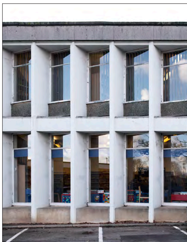
Figure 134. Detail of the east façade of the county library extension, built 1961-4. These windows were designed to light the adult lending library on the ground floor and an adult reference room above. (©Historic England Archive, James O. Davies, DP275690)
