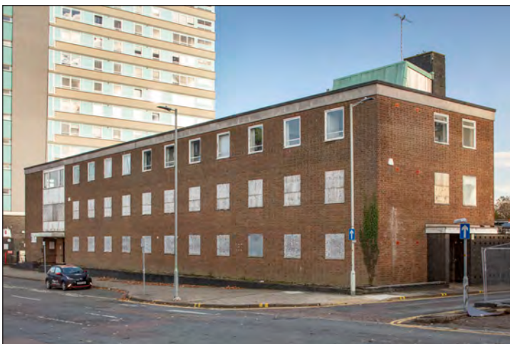
Figure 140. The former police station in Southgate in a photograph of 2020. Permission for its demolition, along with the adjacent garage block, was granted in late 2019. (©Historic England Archive, Patricia Payne, DP278113)
