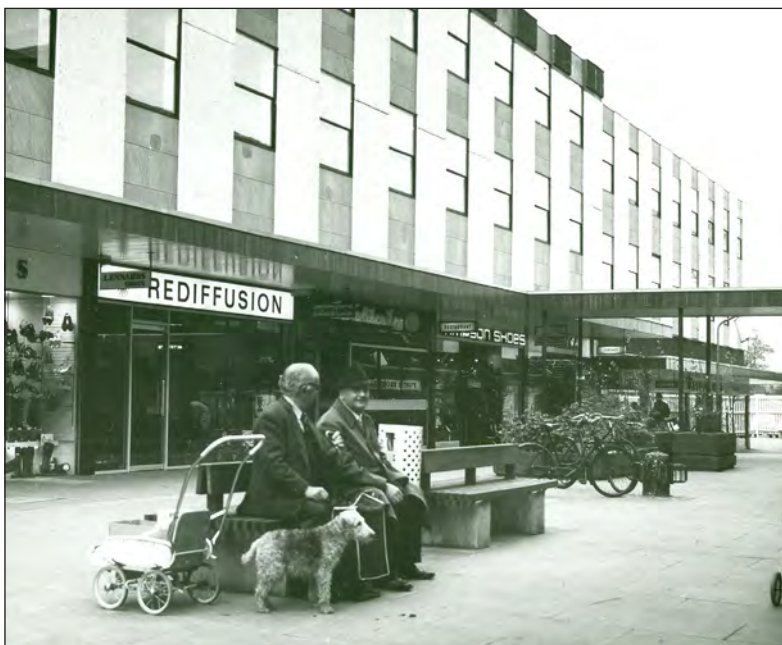
Figure 85. Cross canopies were a unifying feature of all phases of Stevenage's shopping precinct, as built between 1956 and 1976. This photograph shows the cross canopies that formerly existed in the north part of Queensway, built 1967-70. These were removed around 1990. (With kind permission of Stevenage Museum, PP11145)
