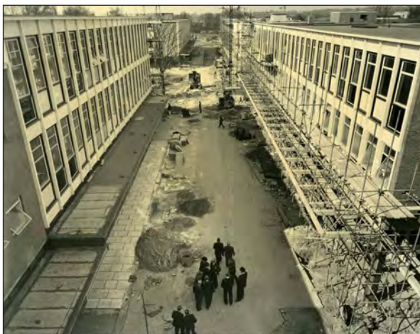
Figure 27. A photograph of 1958 showing construction of Stevenage’s shopping precinct, begun two years earlier. The view looks north along Queensway, towards the Town Square. (With kind permission of Stevenage Museum, P3885)
