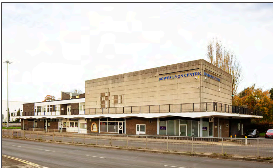
Figure 154. The exterior of Bowes Lyon House youth centre in 2020. There have been alterations since the mid-1960s, but these are comparatively minor, and the building remains in the use for which it was built. (©Historic England Archive, Patricia Payne, DP278137)
