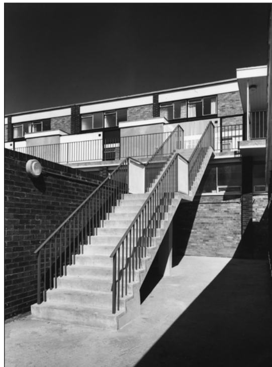
Figure 65. A photograph of 1959 showing rear access stairs to maisonettes placed above the town centre shops. (John Maltby/RIBA Collections)
