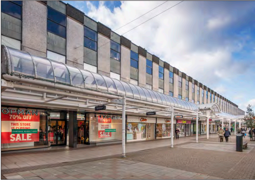
Figure 91. To date, the principal alteration to the north part of Queensway, built in 1967-70, has been the replacement of the canopies with a glazed arcade – work seemingly undertaken in c. 1990, following the opening of the Westgate shopping centre. (©Historic England Archive, James O. Davies, DP275707)
