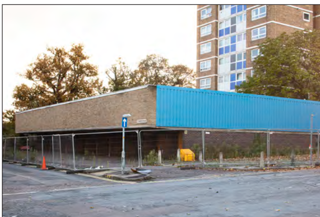
Figure 139. The multi-storey police garage block in Southgate, built in c. 1964-5 and shown here in a photograph of 2020, awaiting demolition. (©Historic England Archive, Patricia Payne, DP278114)
