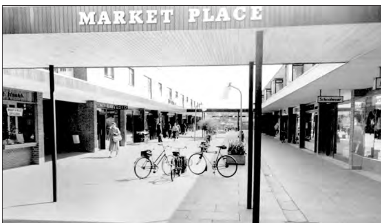
Figure 86. Three cross canopies were built in Market Place, all of which survive. This photograph shows the pedestrian way in c. 1960. (© The Francis Frith Collection)
