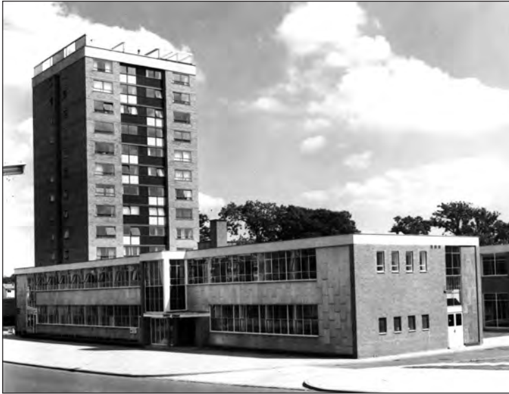
Figure 131. A photograph of c. 1970 showing the integrated county library and health centre, Southgate, built in 1959-60 to designs by the architects of Hertfordshire County Council, with The Towers point block beyond. (With kind permission of Stevenage Museum, P7379)
