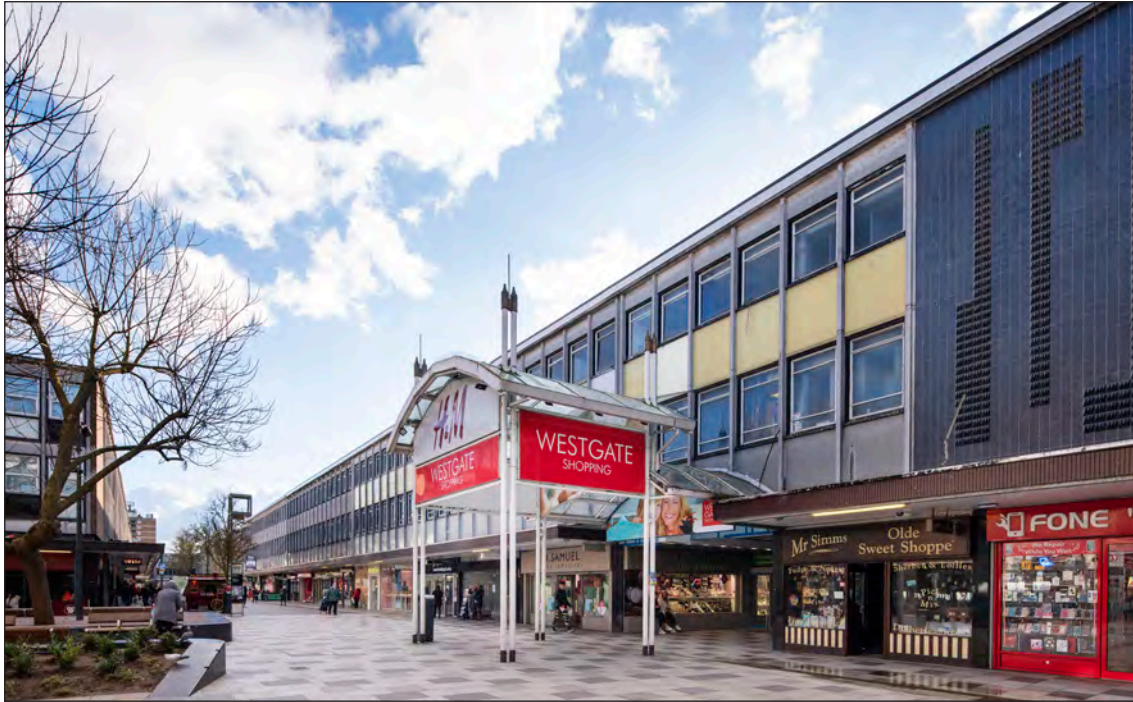
Figure 75. View from Littlewoods Square towards the west block of Queensway. The section with the yellow-coloured second-floor panels dates from 1962-4, and adjoins the 1950s work to the south. The entrance to the Westgate shopping centre was added in c. 1988. (©Historic England Archive, James O. Davies, DP275705)
