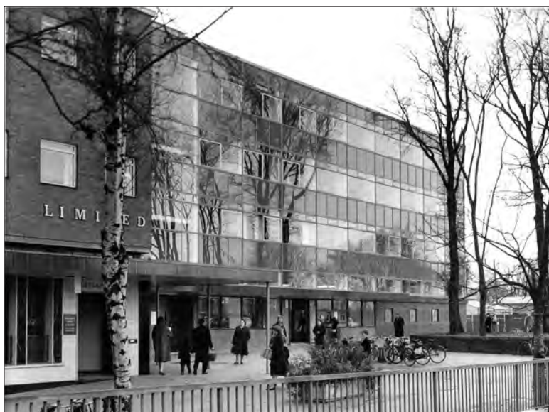
Figure 110. The Head Post Office on the south side of the Town Square, designed by Leonard Vincent and his team and built in 1958-9. The building was demolished in 1999 and replaced by The Plaza development. (With kind permission of Stevenage Museum, P3947)
