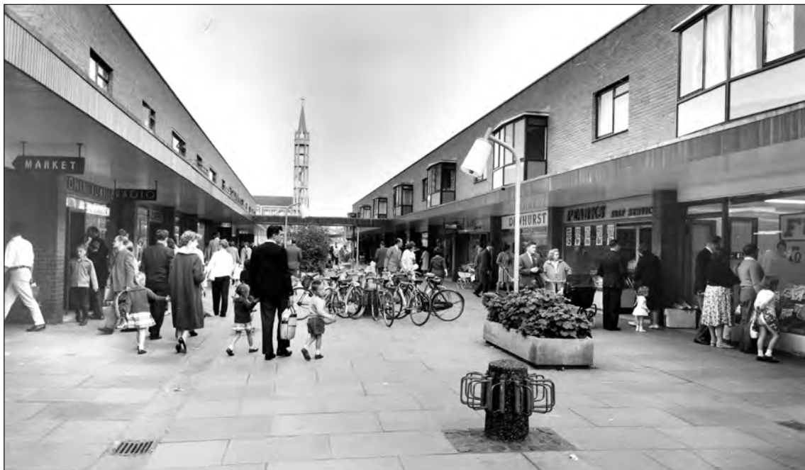
Figure 64. A photo of 1963 showing the two-storey section of Market Place, looking east towards the church, with flats placed above the shops. The whole ensemble, including street furniture, was designed by Leonard Vincent’s team at SDC. (With kind permission of Stevenage Museum, P6857)
