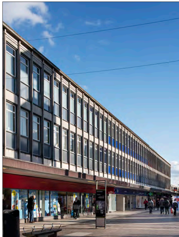
Figure 24. The shopping precinct at Stevenage is notable for being unified in its design. On the rare occasions where companies employed their own architects – as was the case in this part of Queensway, at shops including Woolworth’s and Boots – Leonard Vincent of the Development Corporation adapted their designs to his modular ethos. (©Historic England Archive, James O. Davies, DP275704)
