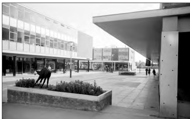
Figure 18. An example of a small-scale pedestrian precinct in a new town is Bush Fair in Netteswell, Harlow, built in 1956-9 and shown here in a photograph of c. 1960. (©Historic England Archive, AA98/06942)
