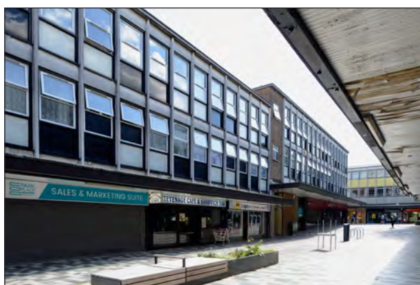
Figure 43. Park Place, looking east towards Queensway. This pedestrian way was extended in the early 1960s to include 'larger standard units', with shops on the ground floors and a mixture of commercial and residential use above. The brick wall towards the centre of the picture represents the end of the first phase work of 1956-9. (© Elain Harwood)
