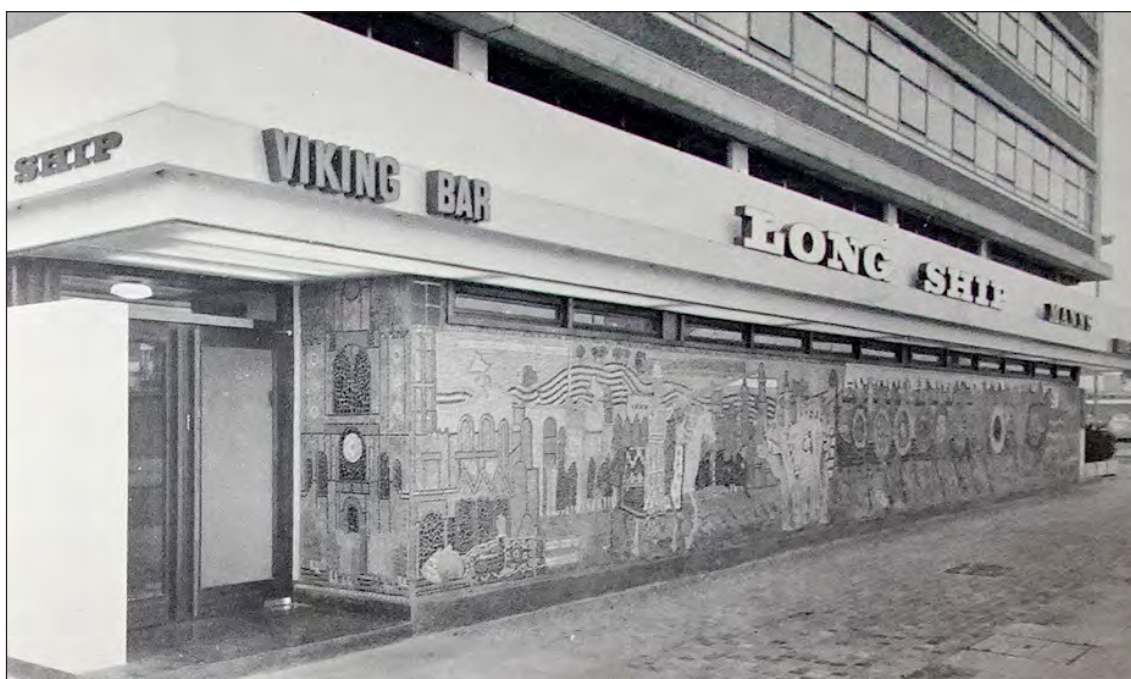
Figure 143. The Viking-themed Long Ship public house, at the base of Southgate House, in a photograph published in the Watney Mann magazine The Red Barrel in 1967. The pub opened in October 1966 and featured on its façade a large mosaic by the artist William Mitchell. This was removed as part of the remodelling of the ground floor in 2001. (Courtesy of Heineken UK)
