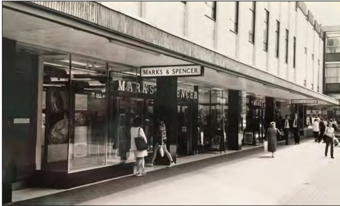
Figure 77. Photo of 1998 showing the Marks and Spencer's store in the north part of Queensway. This was opened in 1970 and closed in 2015. (Courtesy of K. Morrison)
