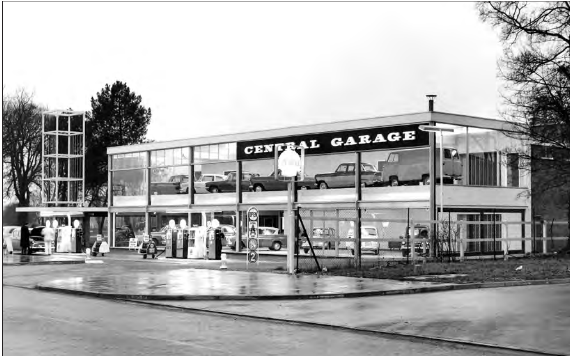
Figure 127. The Central Garage, Danestrete, was the first building of its type in Stevenage town centre. It was built in 1960-1 for Shell Mex BP Ltd, to designs by the respected architect Max Lock, including both a car showroom and a filling station. The site was redeveloped as flats in 2005-6. (With kind permission of Stevenage Museum, P3738)
