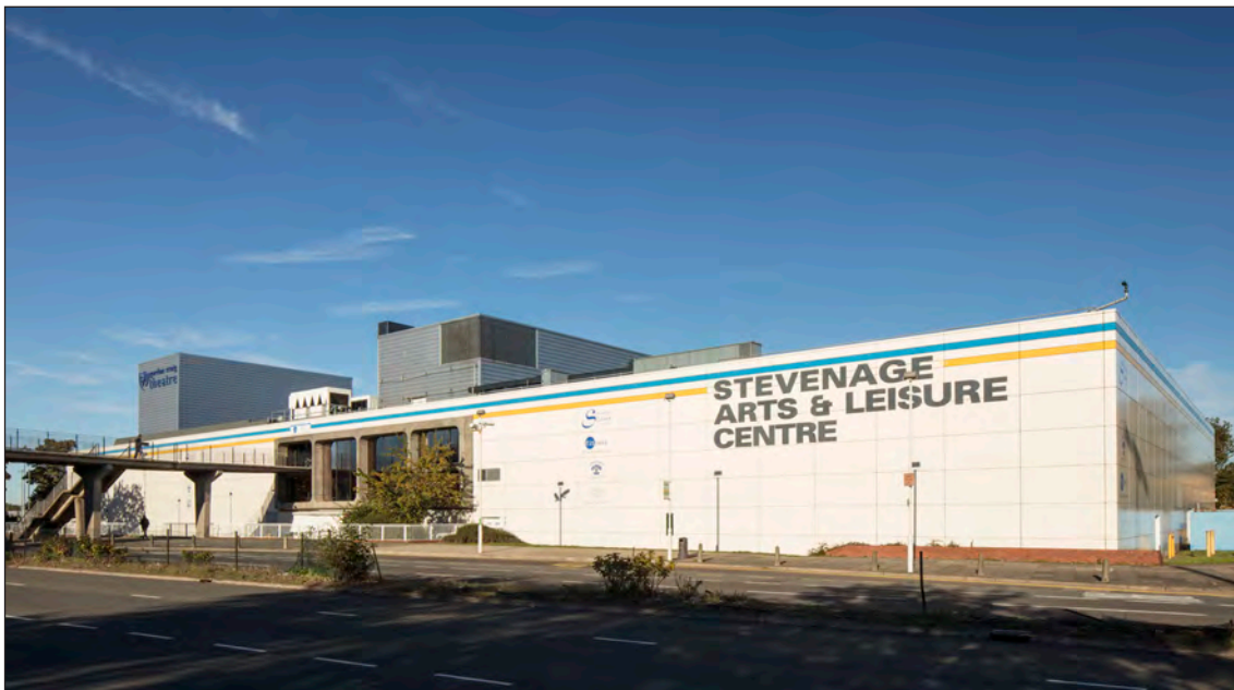
Figure 161. The west front of the arts and leisure centre, facing onto Lytton Way, showing the results of the recladding works undertaken in c. 1993-4. (©Historic England Archive, Patricia Payne, DP237000)
