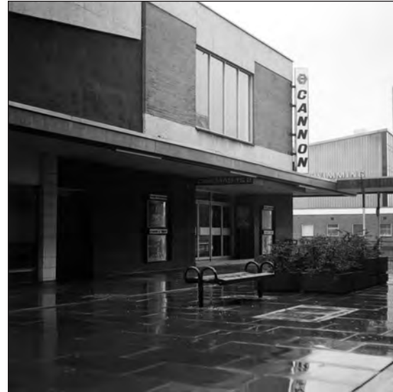
Figure 79. The east part of the 1971-3 block on The Forum contained an ABC cinema. This became part of the Cannon group in 1987, and closed in 1994, at which point the whole block was demolished. Its site is now occupied by a surface car park. (With kind permission of Stevenage Museum, PP1192)
