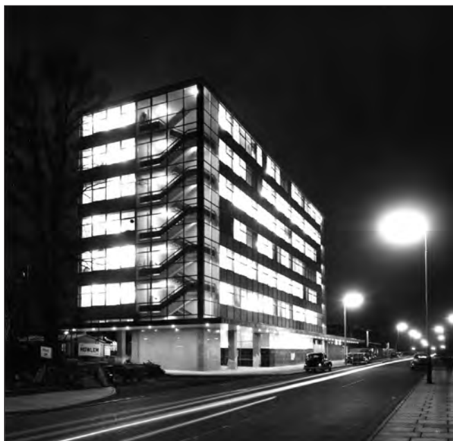
Figure 114. One of the most important offices developments in central Stevenage was Daneshill House, Danestrete. This was built in 1959-61 as Stevenage Development Corporation’s own headquarters, to designs by Leonard Vincent and his team. (With kind permission of Stevenage Museum, P3963)
