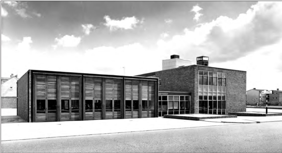
Figure 145. The fire and ambulance station on St George's Way, built in 1961-2 to designs by Hertfordshire County Council. and shown here in a photograph taken shortly after completion. (With kind permission of Stevenage Museum, P7053)
