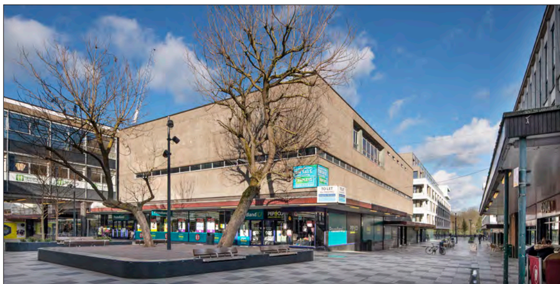
Figure 42. Features of Phase II of the shopping precinct, constructed in 1962-4, included a two-storey glass bridge (left of photo), a Littlewoods department store (centre) – facing onto a 'square' – and new buildings in Park Place (right). (©Historic England Archive, James O. Davies, DP275708)
