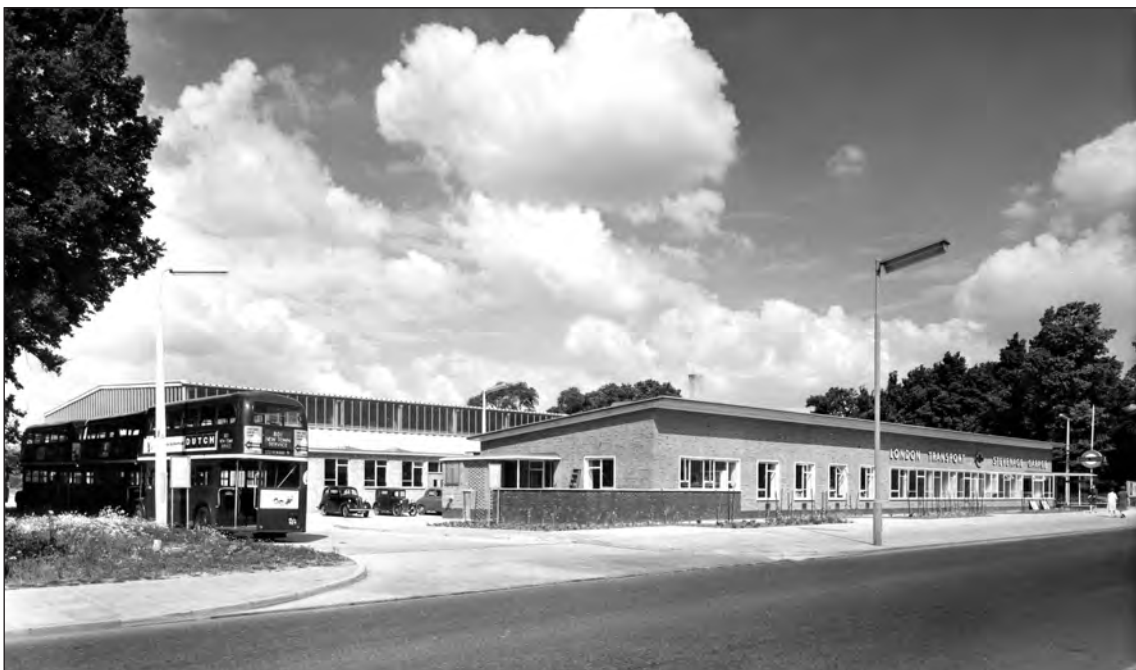
Figure 109. The bus garage on Danestrete, seen from the south-east. The garage was built in 1957-9 to designs by the London Transport Executive, and comprised a low range of offices with taller garage block behind. It was demolished in 1993. (With kind permission of Stevenage Museum, P3777)
