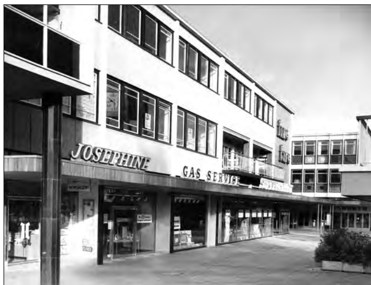
Figure 25. One of the unifying external features of Stevenage town centre is the use of canopies above the ground-floor shopfronts. These connected all shops, and were finished in timber. Shown here is the north side of the Town Square, in a photograph of 1959. (With kind permission of Stevenage Museum, P3945)
