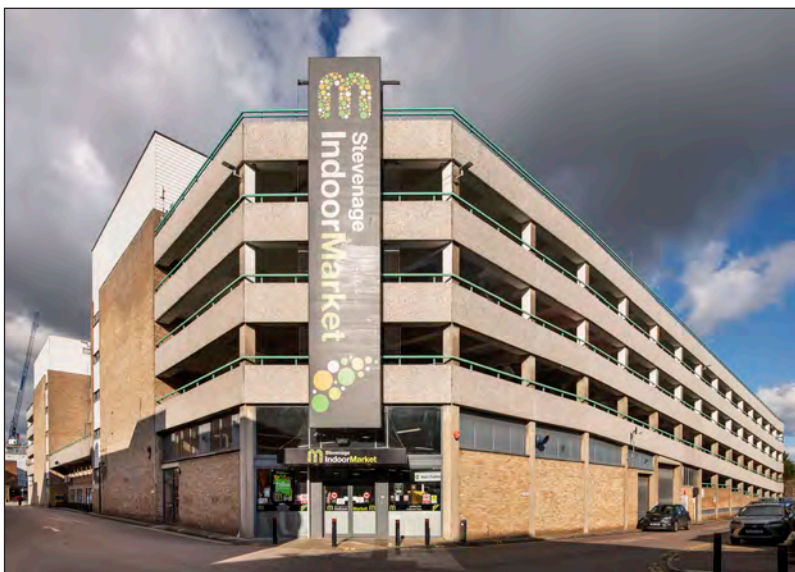
Figure 105. The multi-storey car park on St George's Way, built in 1971-3 on the site of the former Market Square car park. It is viewed here from the south-west, showing the entrance to the ground-floor market. (©Historic England Archive, James O. Davies, DP275699)
