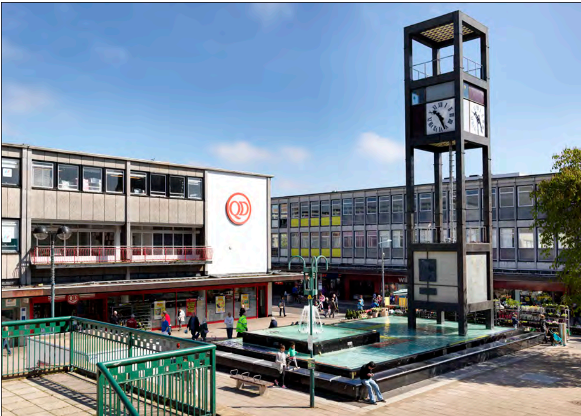
Figure 101. The east part of the Town Square in 2013, with the clock tower and pool, the platform visible on the left and the former Fine Fare supermarket (reworked as QD). The pool was altered in c. 1995. (©Historic England Archive, James O. Davies, DP159947)
