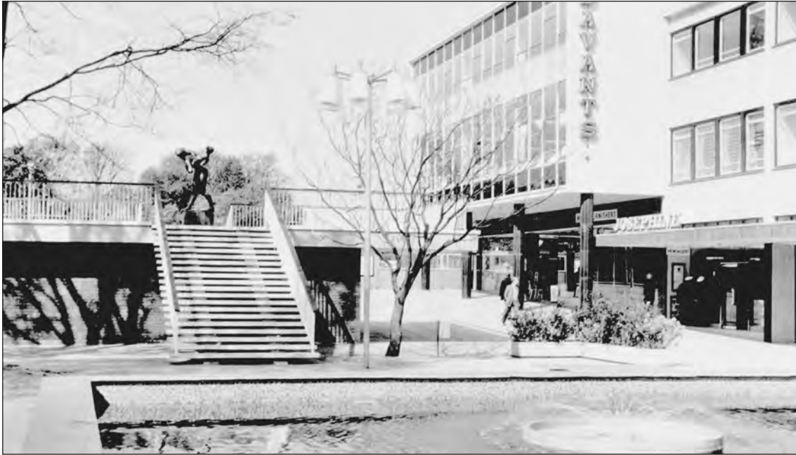
Figure 168. The Town Square – shown here in a photograph of c. 1960, looking west – is the most famous component of Stevenage town centre. It is at the heart of its conservation area, and contains two listed structures: the sculpture Joy Ride and the clock tower. (© The Francis Frith Collection)
