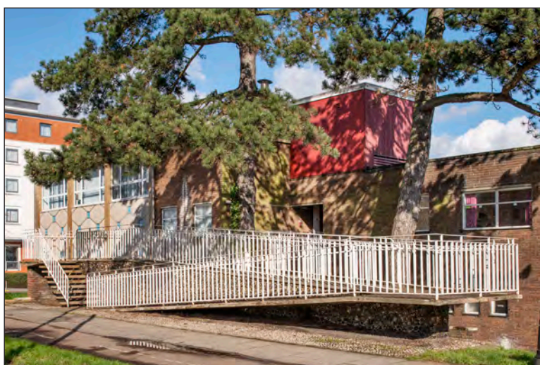
Figure 130. The west (Danestrete) side of the outpatients’ clinic, showing the original ramped entrance way and railings, as well as the mature Scots pines retained by Stevenage Development Corporation when the building was constructed. (©Historic England Archive, James O. Davies, DP275684)
