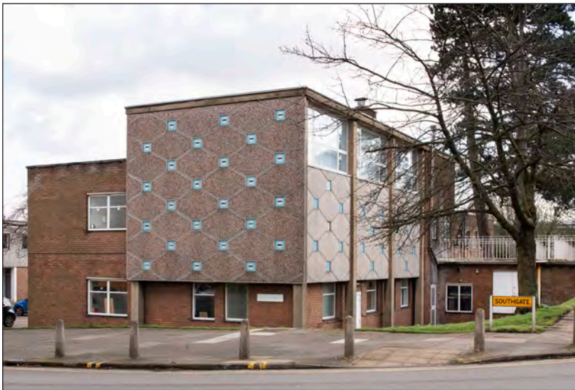
Figure 129. The same view of the outpatients' clinic in 2020, showing how little the exterior of the building has been altered over the past six decades. (©Historic England Archive, James O. Davies, DP275679)
