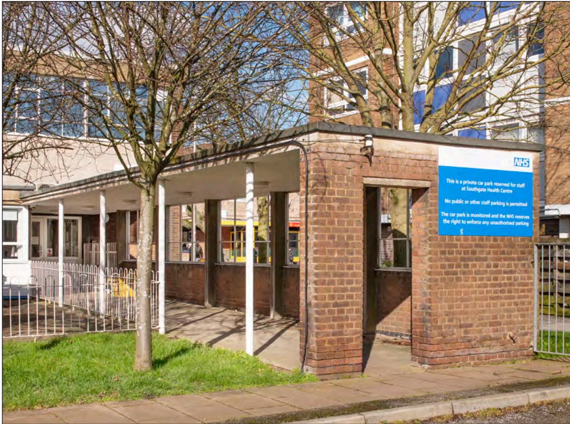
Figure 135. At the rear of the health centre in Southgate a notable surviving feature is the pram shelter, built as part of the construction works of 1959-60. (©Historic England Archive, James O. Davies, DP275688)
