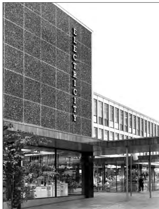
Figure 70. Variety in the design of Stevenage town centre was created by the use of blank walls such as this – faced with concrete aggregate and incised with lines forming a grid. It is opposite the junction of Queensway and Market Place, and is seen here in a photo of 1959. (With kind permission of Stevenage Museum, P3799)
