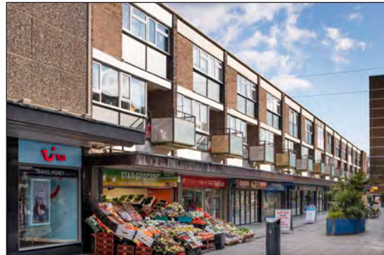
Figure 69. The buildings in the south part of Queensway were designed with residential accommodation placed above the shops, and featured first-floor glass-edged balconies, which survive well. (©Historic England Archive, James O. Davies, DP275696)
