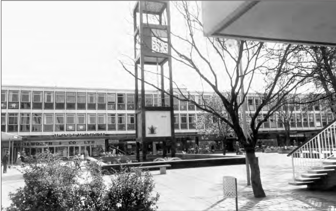
Figure 66. A view of c. 1960 from the Town Square towards Queensway, showing the unified grid design used for the exterior architecture of Stevenage's shopping precinct. This was novel at the time, though has since come to be widespread. (© The Francis Frith Collection)
