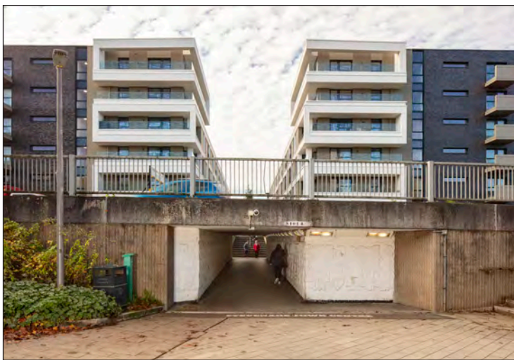
Figure 90. A photograph showing the heavily remodelled Park Place blocks (2017-18) from the east. Also visible are William Mitchell's relief sculptures of 1973, decorating the subway built at that time as part of the alteration of St George's Way as a dual carriageway. (©Historic England Archive, Patricia Payne, DP278119)
