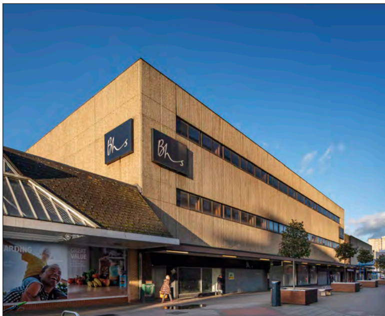
Figure 82. The BHS store in The Forum viewed from the south-west in 2020. The store closed in 2016. (©Historic England Archive, James O. Davies, DP275715)
