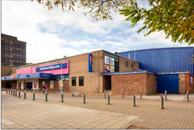
Figure 119. A photograph of 2020 showing the exterior of what is now Stevenage's Mecca bingo hall. The massing of the building is that of 1960-1, but there have been various alterations, such as the remodelling of the canopy. (©Historic England Archive, Patricia Payne, DP278095)
