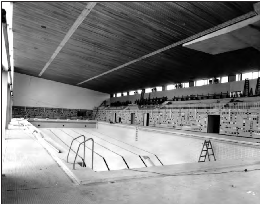
Figure 156. The pool hall of the swimming baths building in St George's Way, in a photograph of 1962. This included a large main pool, a smaller training pool and a gallery for spectators. (With kind permission of Stevenage Museum, P7054)
