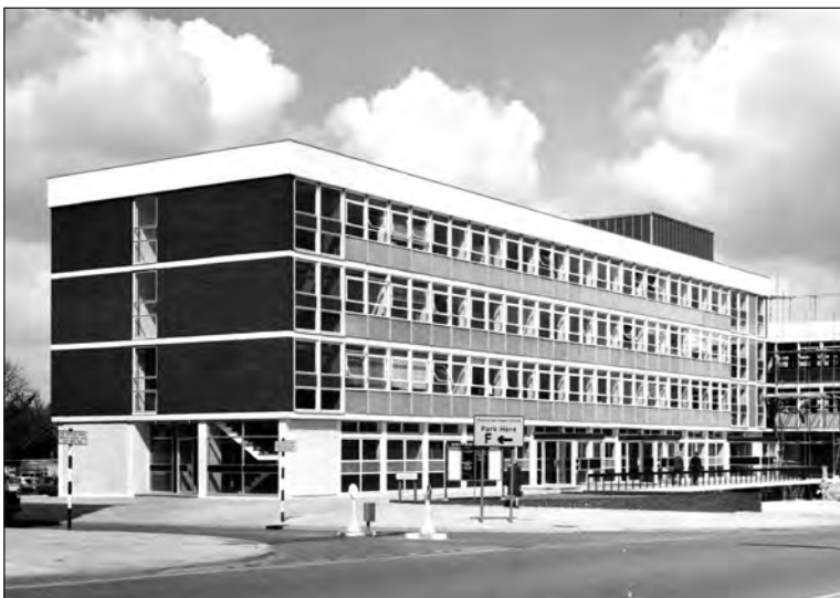
Figure 125. A photo of 1967 showing the recently completed phase one block of Brickdale House, Danestrete (built 1964-6), and work beginning on phase two, to the north. The offices were built to designs by the Ministry of Public Building and Works and housed staff from four government departments. (With kind permission of Stevenage Museum, P7276)
