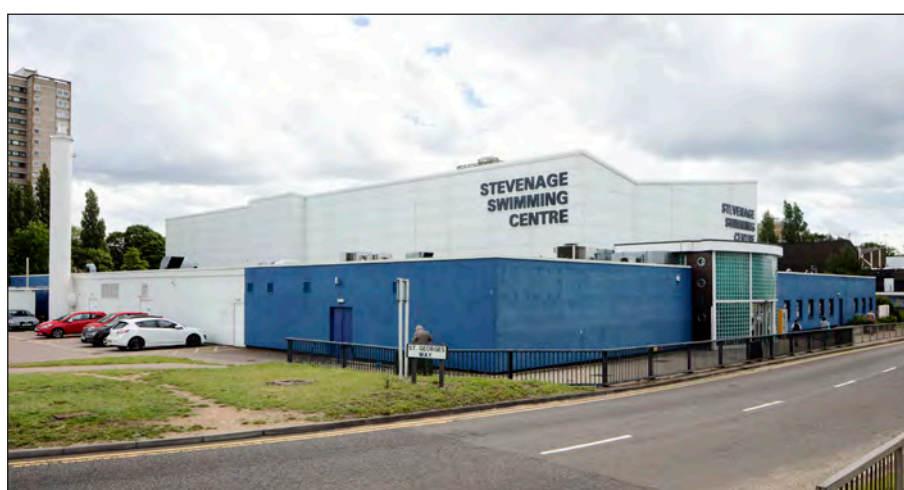
Figure 157. The swimming pool building viewed from the north-west. Alterations undertaken in c. 2000 included the recladding of the structure and a new entrance extension on the west. (©Historic England Archive, Patricia Payne, DP232454)
