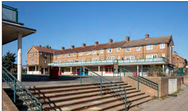
Figure 17. Small-scale pedestrian precincts became increasingly popular in Britain from the early 1950s onwards. Early examples include Park Square, King's Heath, Northampton (1953-4). (©Historic England Archive, Patricia Payne, DP247533)
