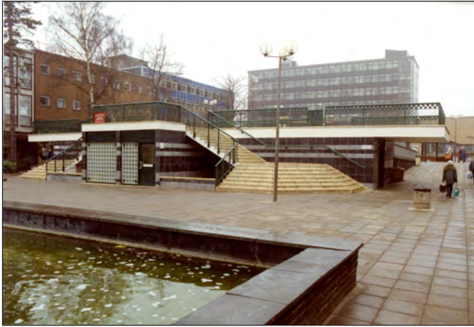
Figure 100. A photograph of February 1993 showing the recently completed alterations to the east side of the raised platform in the Town Square. (With kind permission of Stevenage Museum, PP1203)
