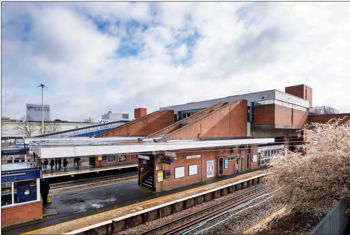
Figure 163. Stevenage railway station, Lytton Way, built in 1971-3 to replace the Victorian station at Old Stevenage. This photograph looks south-east across the tracks and platforms. The building was designed by British Railways Eastern Region. (©Historic England Archive, James O. Davies, DP275655)
