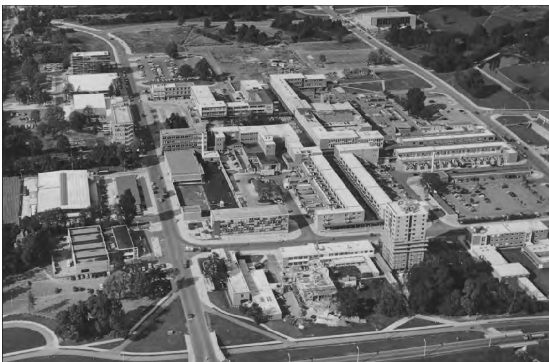
Figure 41. Aerial photograph of 1962 showing clearance work at the north of Queensway (at the top of the picture), in preparation for the building of 'Phase II' of the shopping precinct. The view, looking north, also shows construction underway on The Towers and the library extension (bottom of the picture). (With kind permission of Stevenage Museum, PP1292)
