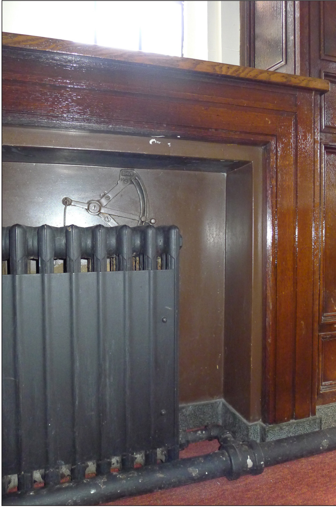
Figure 35: Detail of fresh-air inlet behind radiator at the Cumberland Inn, Botchergate, Carlisle, completed 1930 (© Historic England, photograph: Rebecca Pullen, 2016)
