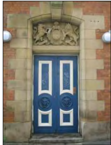
Plate 30: Detail of the Faraday Street entrance into Newton Street Police Station.
