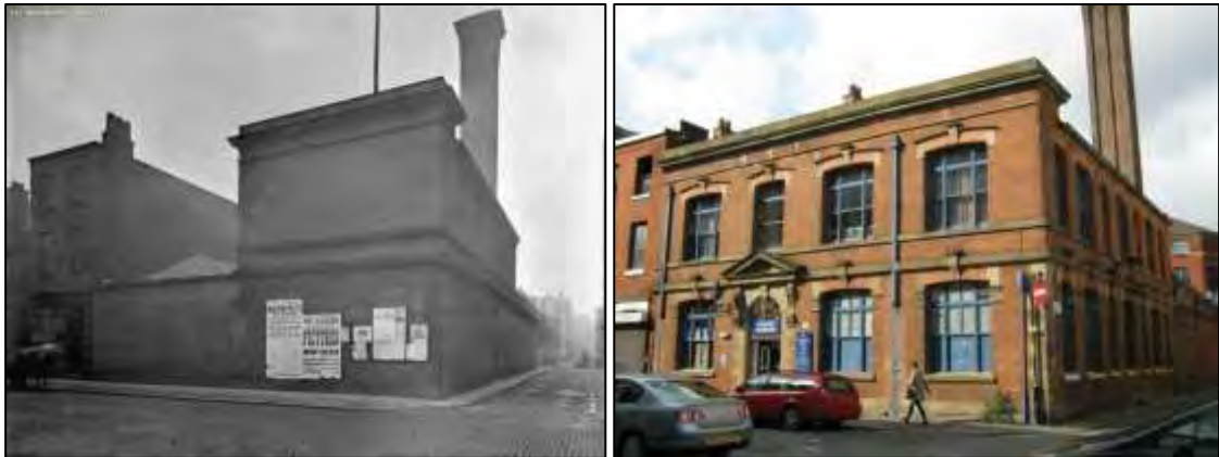
Plate 28-29: Nineteenth century photograph of Newton Street Police Station prior to its expansion (© Manchester Archives) and the station today showing the 1902 alterations.
