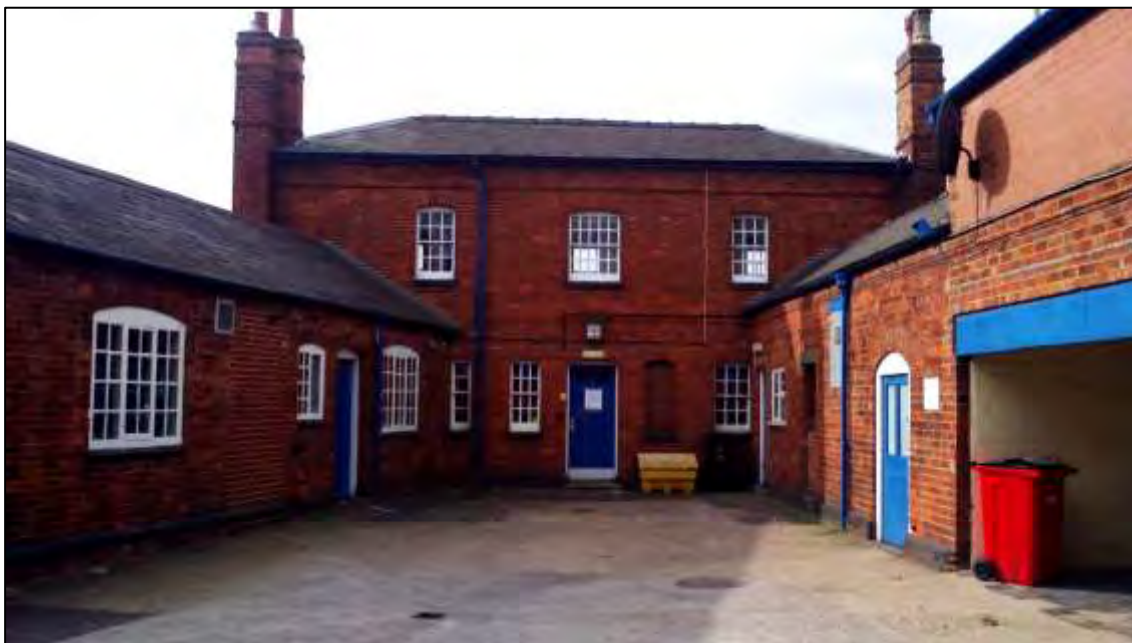
Plate 41: View of the rear of Lutterworth Police Station, looking south.
