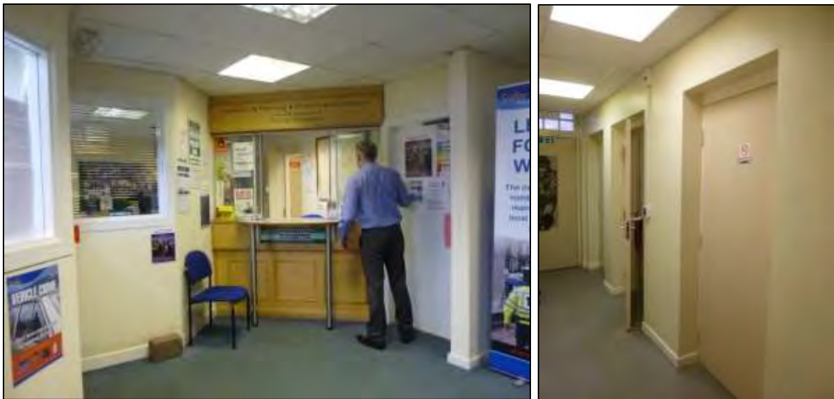
Plates 46-47: Refurbished enquiry desk (left) and cells (now storage; right) in Easingwold Police Station.
