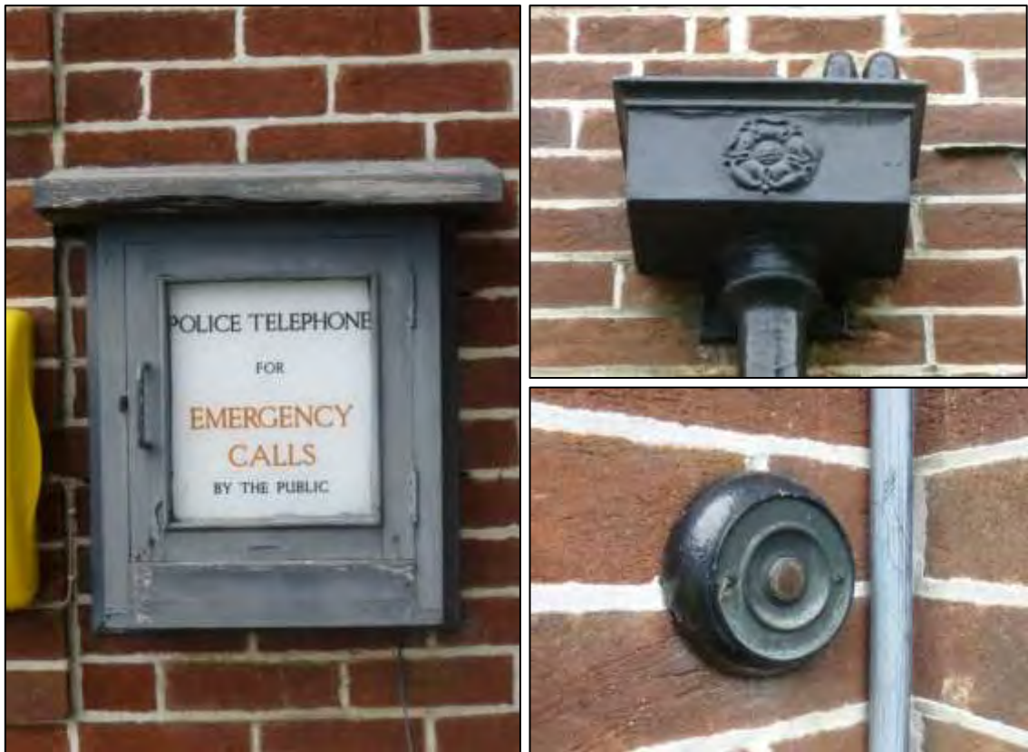
Plate 45: Details of original public police telephone, hopper and bell push at Easingwold.
