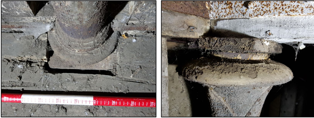
Figure 28: Left: The original flooring has been cut so that the columns sit on the level stone surface below in order to create greater stability. Right: This may have resulted in the columns being too short, so a piece of metal was inserted above each column so that it supported the wall plate and tie beam. The tie beam and wall plate are joined with an iron strap.
