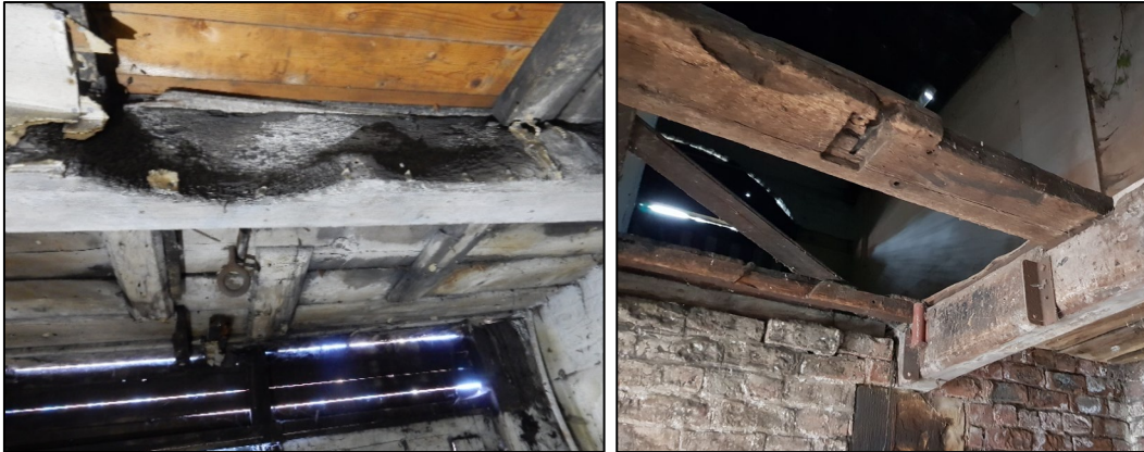
Figure 47: Crescent-shaped wear marks in the waybeam (left) and a reused sleeper (right)
