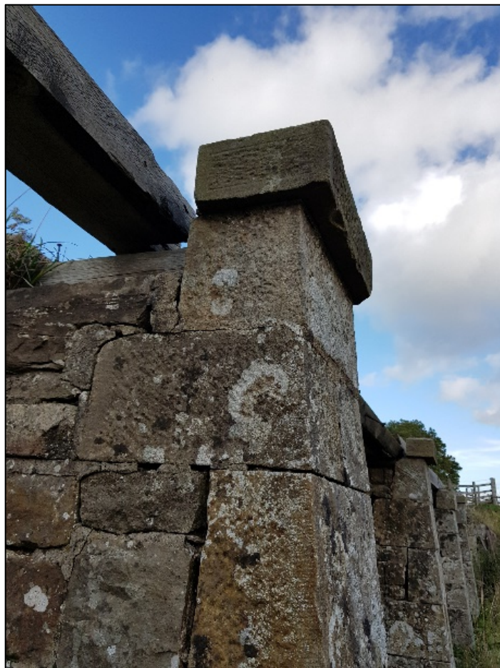
Figure 52: Tooled and margined coping to the cell wall tops at the coal depot, Bowes Station.
