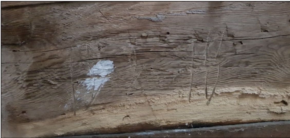
Figure 36: Baltic shipping marks on the underside to the attendants' platform above cell 2. The marks possibly indicate third- or common-grade timber.
