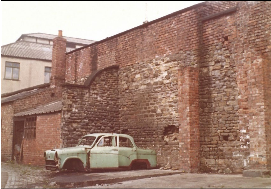
Figure 51: The much altered 1825 Depot walls in 1972 with scarring where garden buildings leaned against them from 1837. The walls have been heightened in brick and reused for subsequent development (photo: John Proud, courtesy of Win Proud)
