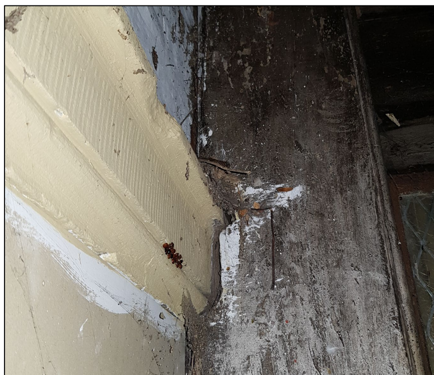
Figure 32: The timber upright supporting the wooden wall plate has been cut around the stone impost bands. This suggests that the impost design was added before the timber frontage added.
