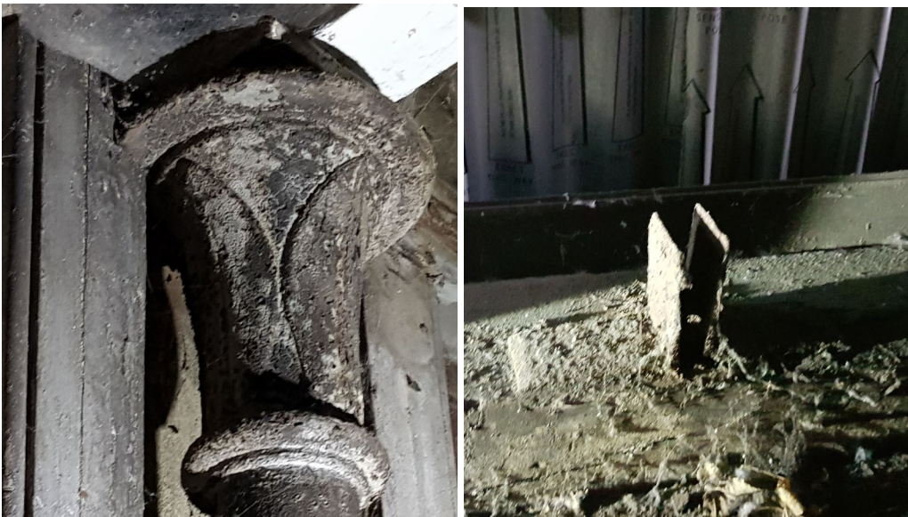
Figure 29: Left: The capitals of the columns are cut into the timber uprights. Right: catches at the base of each louvre opening were presumably part of a mechanism to open and shut the louvres
