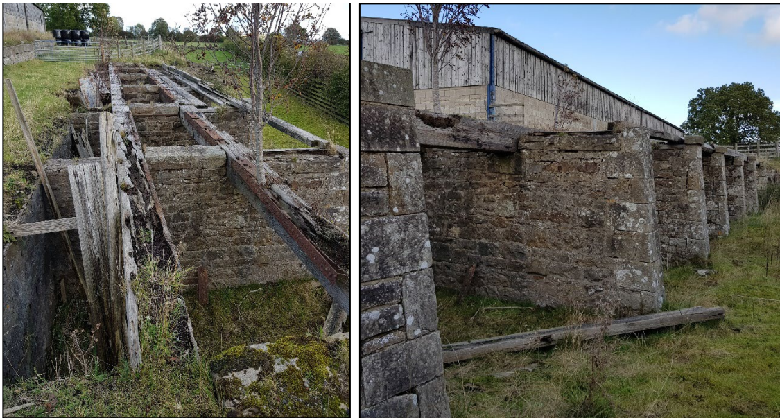
Figure 53: The remains of the coal cells at Bowes Station of 1861 (South Durham & Lancashire Union Railway, formed by the S&DR). No lime depot was provided here but the construction similarities are notable including large sandstone pads to support the waybeams, attendants' platforms either side of the track where the laden waggons would be opened and the coal dropped into the cells below and good ashlar facings to the cell walls creating the appearance of stone piers. To prevent the weight of the waggons pushing the walls outwards, the walls were battened back, and additional support provided with iron bars. No such extra strengthening was required at lime depots which had a first storey and roof structure to resist outward forces. Bowes Station and the coal depot are earmarked for demolition when the A66 is widened.
