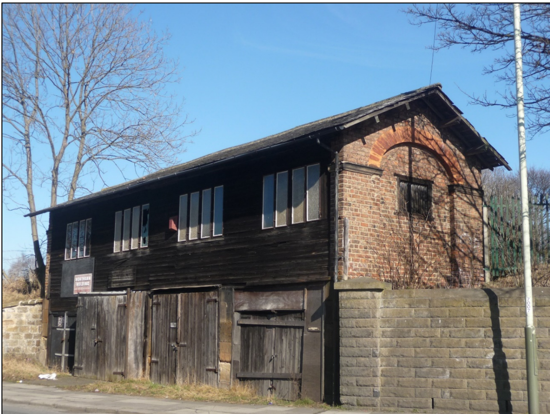
Figure 2: The Lime Depot from the south east in 2010 before the metal security panelling was added to the Hopetown Lane elevation (photo: Archaeo-Environment Ltd)
