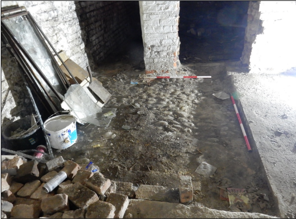
Figure 35: Exposed original stone cobble floor surviving beneath the later concrete.
