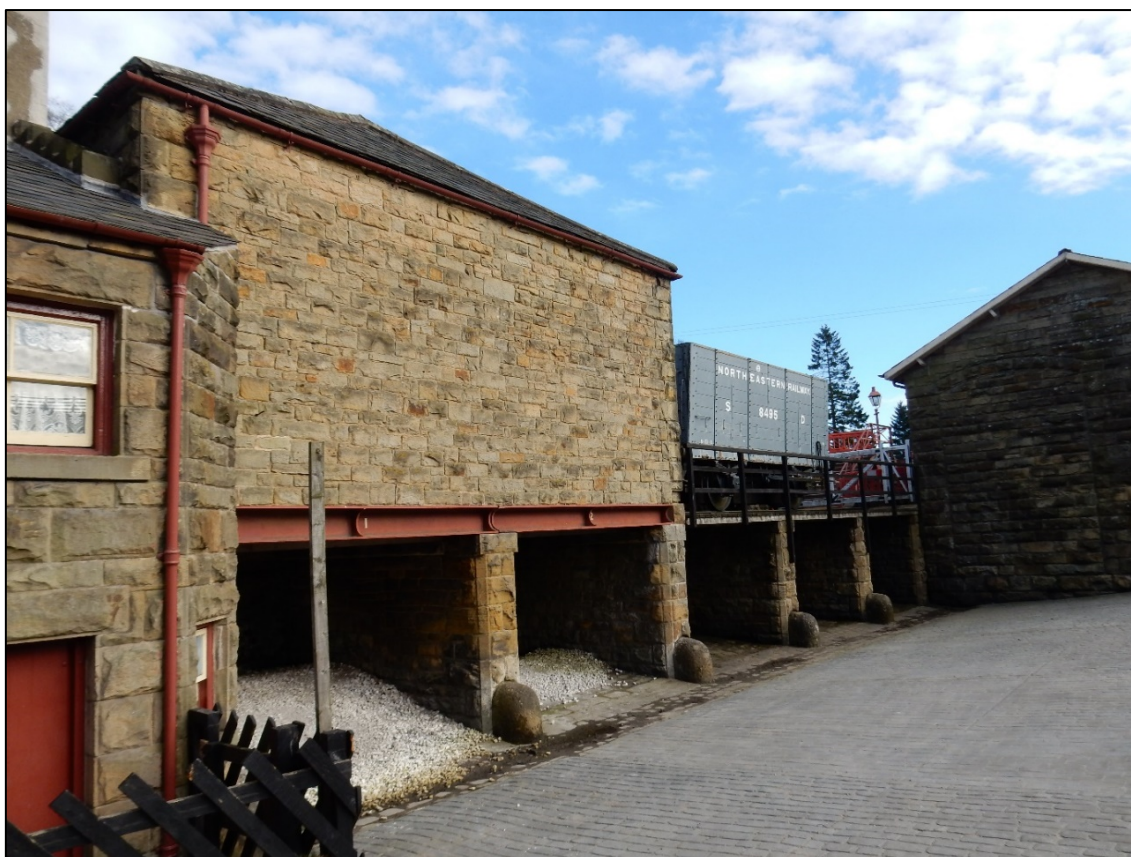
Figure 55: The covered lime depot at Goathland with the exposed coal depot beyond. No doors seem to have been necessary at either set of cells because they were part of a larger goods yard. The boulders to the front protect the dividing walls of the cells from careless reversing.
