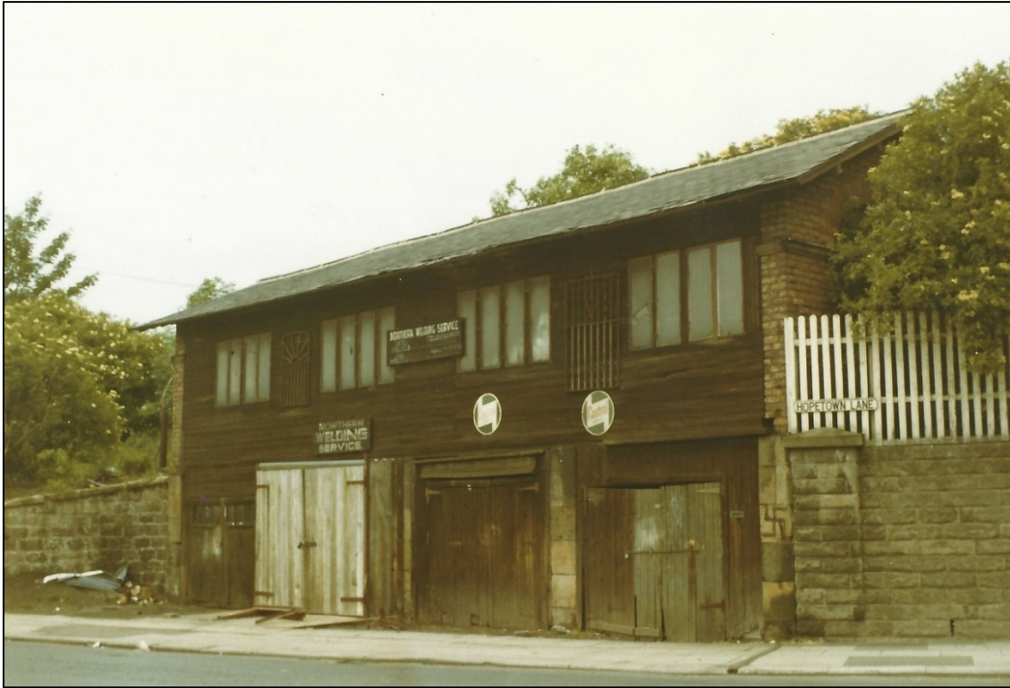
Figure 38: The lime depot in 1971 with new doors in cell 2 replacing the doors shown in the 1960s in fig 16 (photo: John Proud, courtesy of Win Proud)
