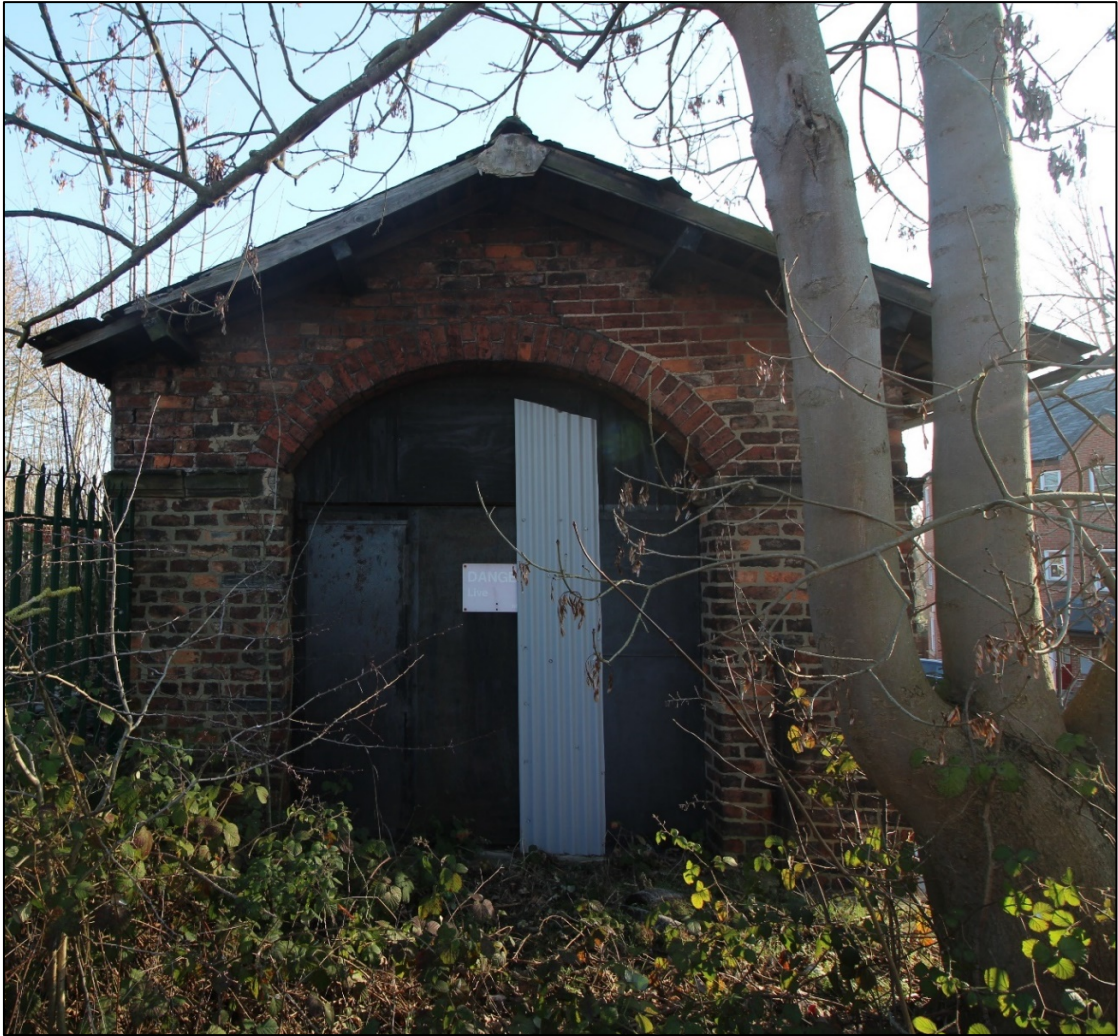
Figure 19: The north-west elevation. This archway was the entrance into the building for fully-laden chaldron waggons containing lime. The doors are a later addition
