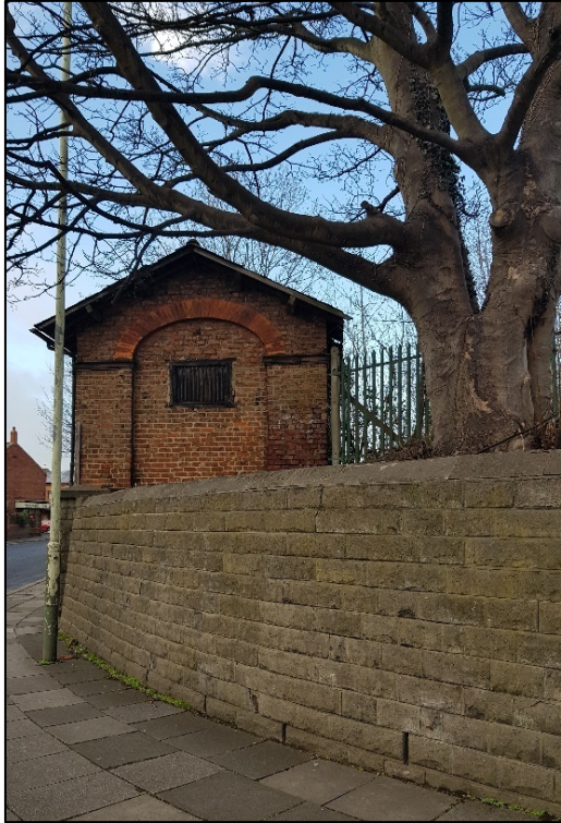
Figure 41: Composite stone walls about the depot. These were probably part of a landscaping scheme from between 1938 and 1950.
