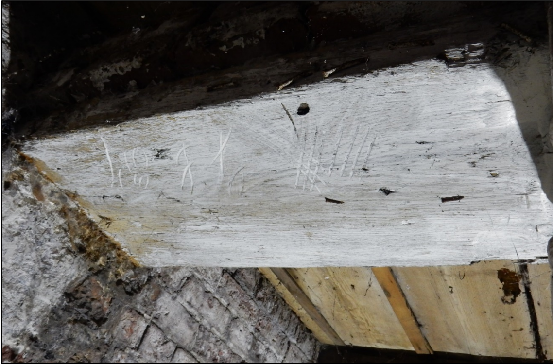
Figure 45: Baltic shipping marks in a later lintel insertion between cells 3 and 4
