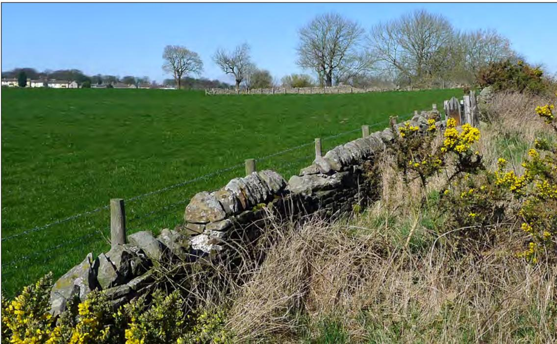
Fig 12: The original railway boundary wall to the south of the Etherley Engine. Ground inspection revealed most of the coping stones are in place. March 2019 © Historic England.
