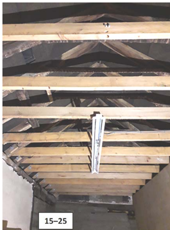
Figure 13: Annotated photograph to help locate sampled timbers from the rear roof of number 45 High Street (viewed looking west to east) (EXT-M15–EXT-M25, photograph Robert Howard)
