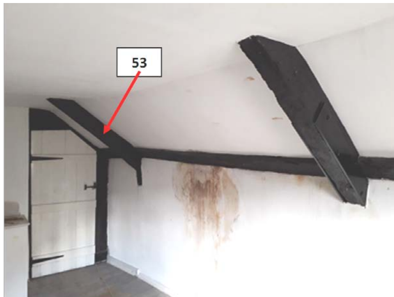
Figure 15d/e: Annotated photographs of the roof space of 41 High Street looking west to east (EXT-M51, EXT-M52, EXT-M54, and EXT-M55; top) and east to west (EXT-M53; bottom) to help identify sampled timbers (photographs Robert Howard)
