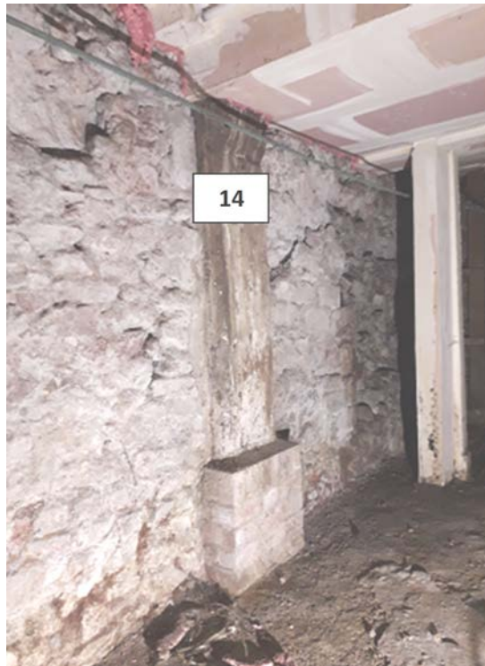
Figure 12c: Annotated photograph to help identify sampled timbers from the south cellar wall of 44 High Street (EXT-M14, photograph Robert Howard)
