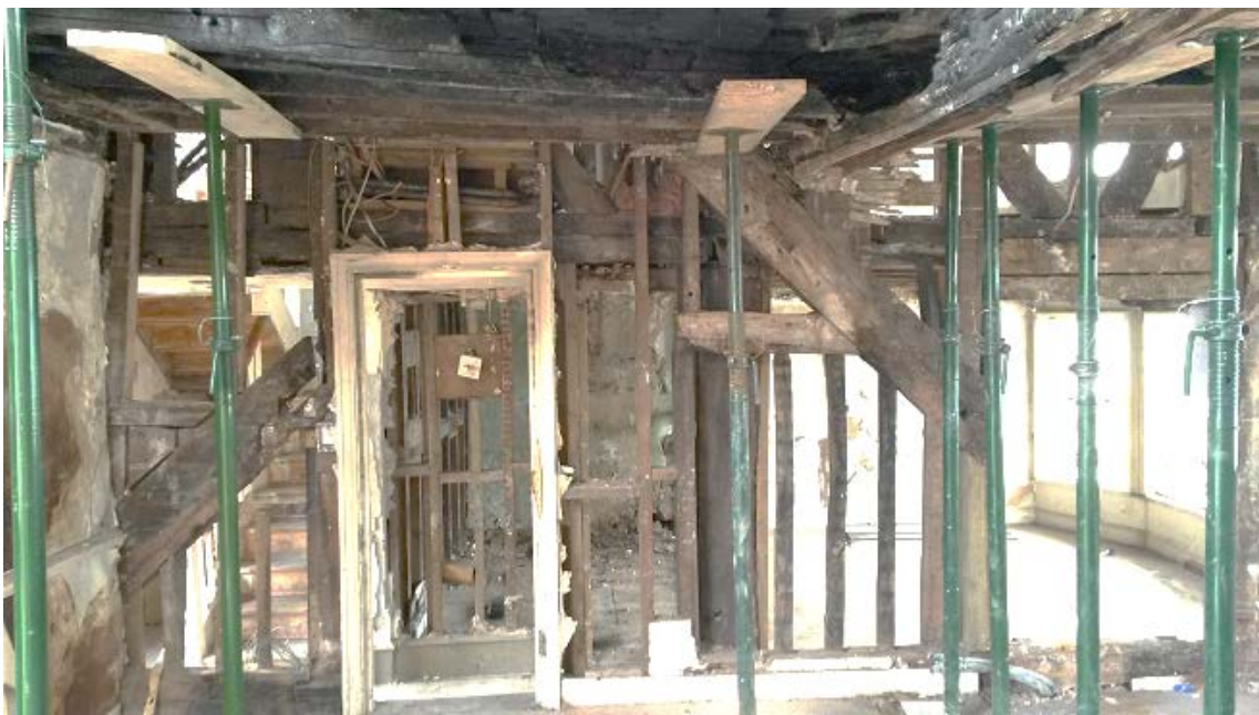
Figure 4a/b: General view of the timber remains to a rear wall of zone 3 (fig. 3) of the Royal Clarence Hotel (top), and the newly revealed truss in zone 1 (fig. 3), the Well House Tavern (16–17 Cathedral Yard, bottom), looking south to north (photographs Robert Howard)
