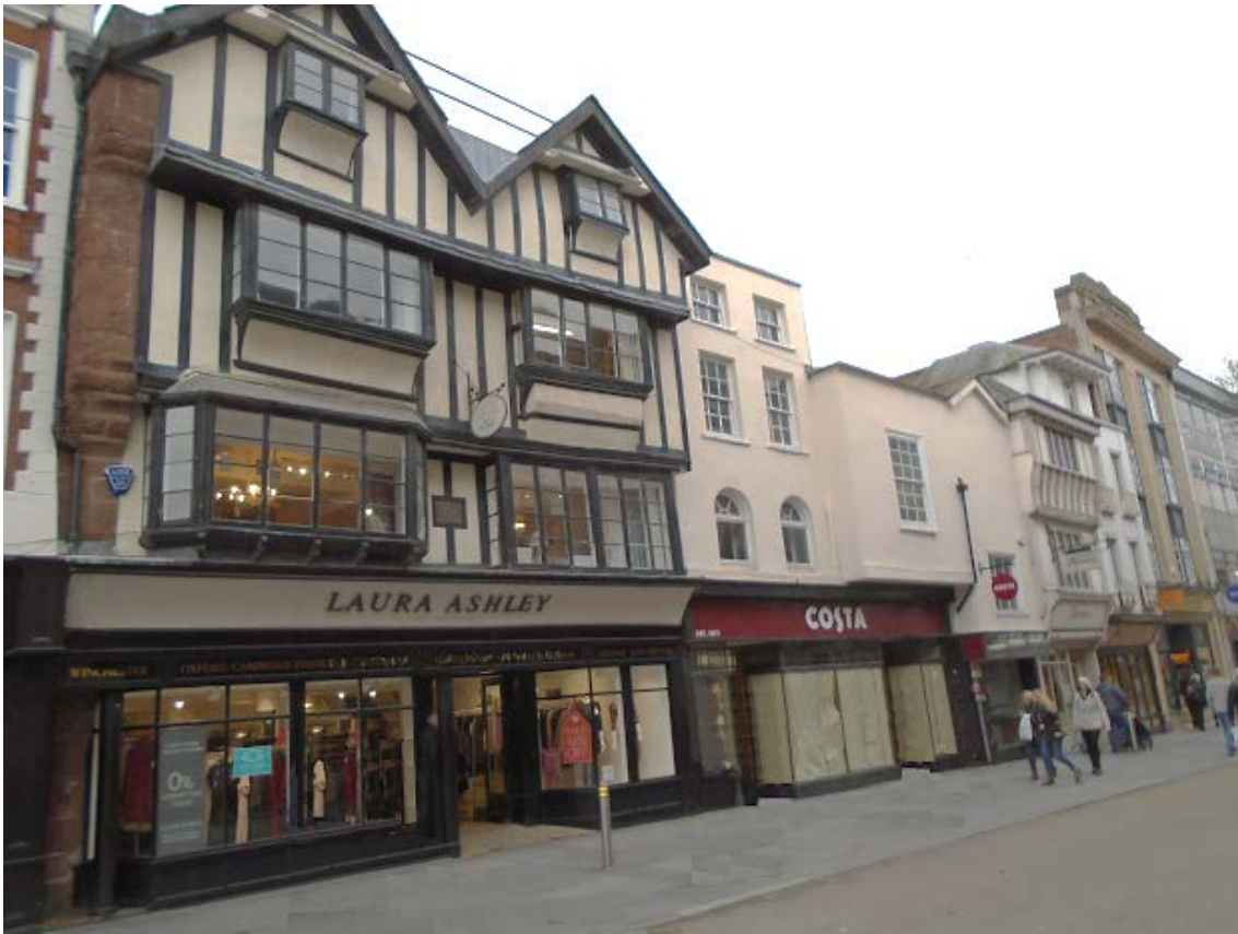
Figure 5: General view looking along the High Street from 41/42 (Laura Ashley), past 43–45 (Costa) towards the still-jettied 47 (L'Occitane, photograph Robert Howard)
