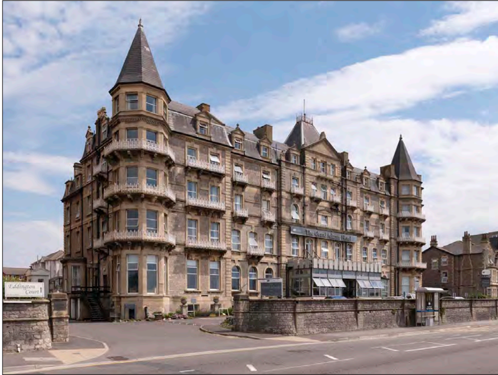
Figure 84: Examination of the Grand Atlantic's facade reveals that the original elevation of the College survives, but the building has been extended on either side by wings with polygonal, corner turrets. It has also been raised to four storeys, with an attic throughout. (DP218759)
