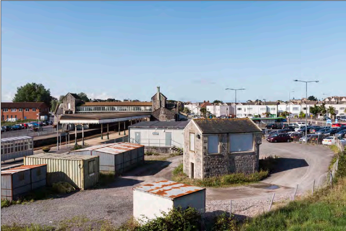
Figure 17: Coinciding with the new station, a new signal box for the branch line was constructed, though it now stands, unused, beside the current station. It is said to be the oldest surviving signal box on the British rail system. (DP218288)
