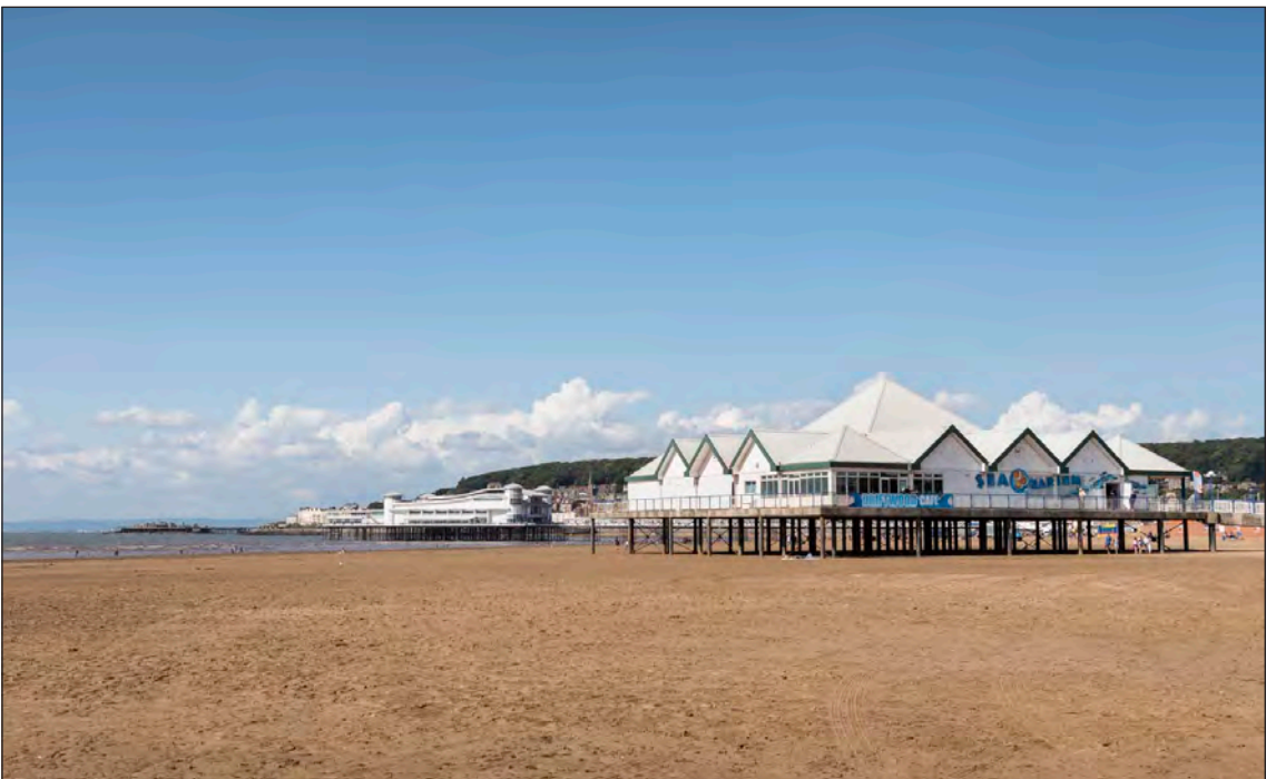
Figure 109: The SeaQuarium is in the foreground, with the Grand Pier in the middle distance and the derelict Birnbeck pier on the horizon. At high tide Weston could be said to have three piers, a claim that only Blackpool can rival. (DP218017)
