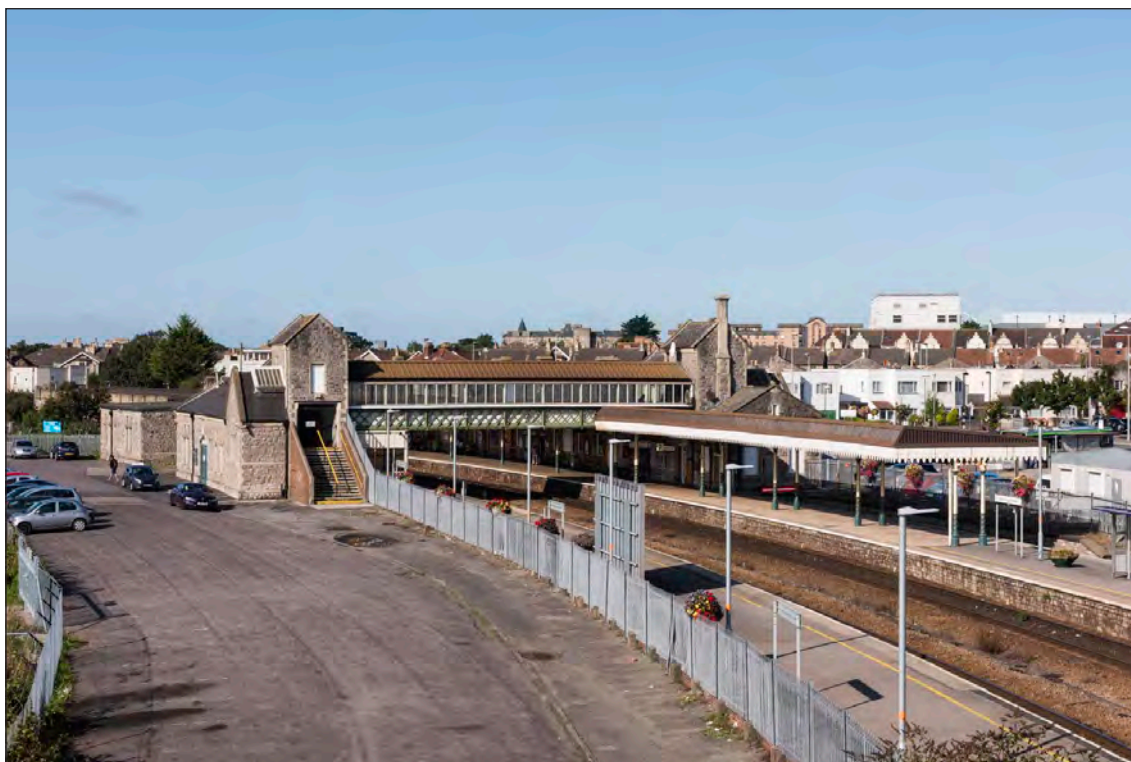
Figure 19: Weston's current railway station is actually relatively small, with only two platforms flanking the twin tracks. (DP218284)
