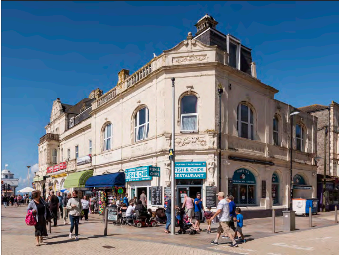
Figure 13: The cluster of buildings at the western end of Regent Street, including the remains of the circulating library in the centre. (DP218266)
