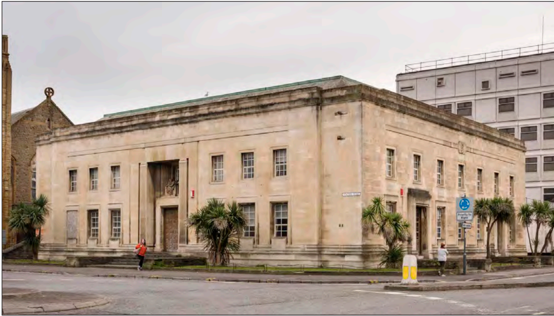
Figure 110: The 1934 Magistrates' Court will be retained and adapted to provide new homes in the centre of Weston, but the 1970 Police Station behind has been demolished to make way for housing. (DP218306)
