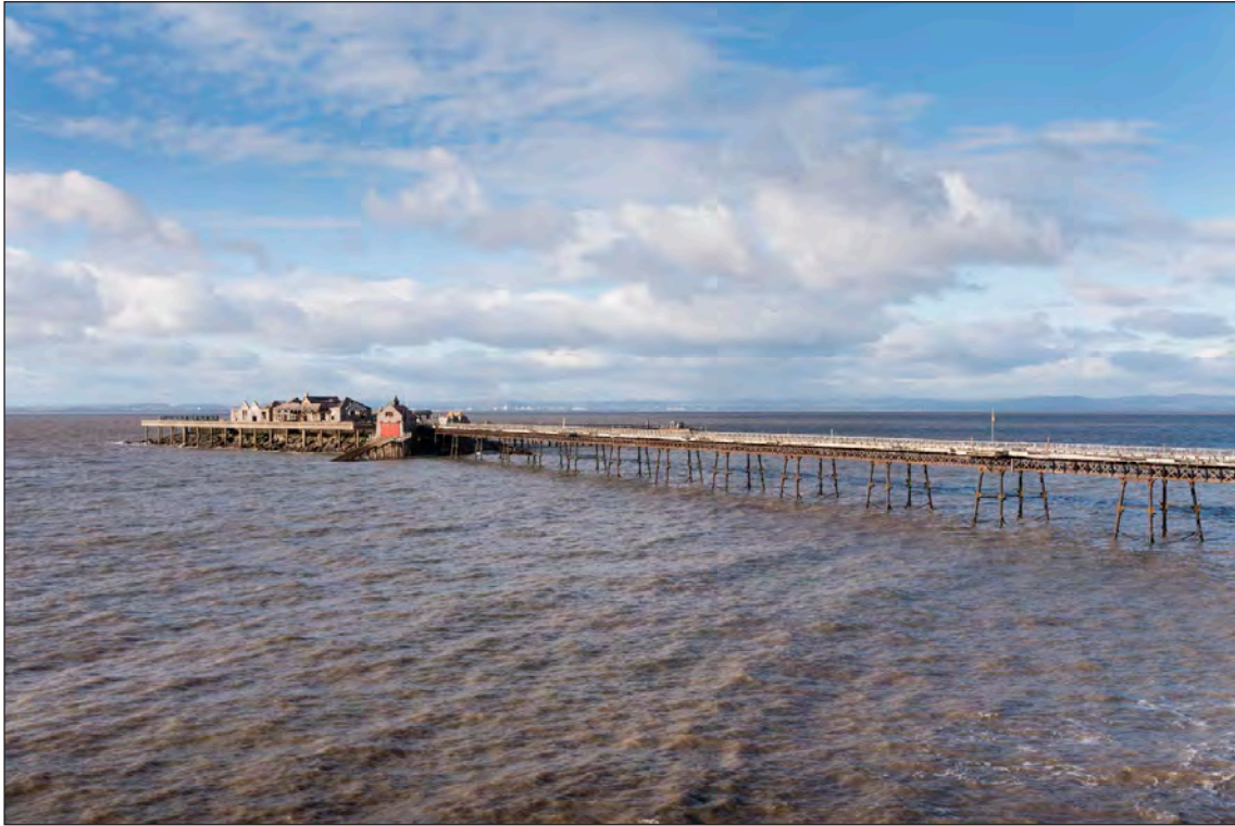
Figure 77: The components of Birnbeck Pier were erected by Messrs Toogood from parts prefabricated at their Isca Foundry across the Severn in Newport (Monmouthshire) and the bridge section was completed by the end of 1866. (DP218350)
