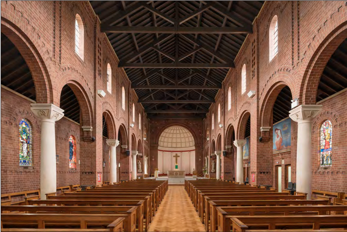
Figure 97: Corpus Christ Roman Catholic Church of 1928-9 has an elegant ashlar exterior and a fine Byzantine-inspired brick interior. (DP218753)
