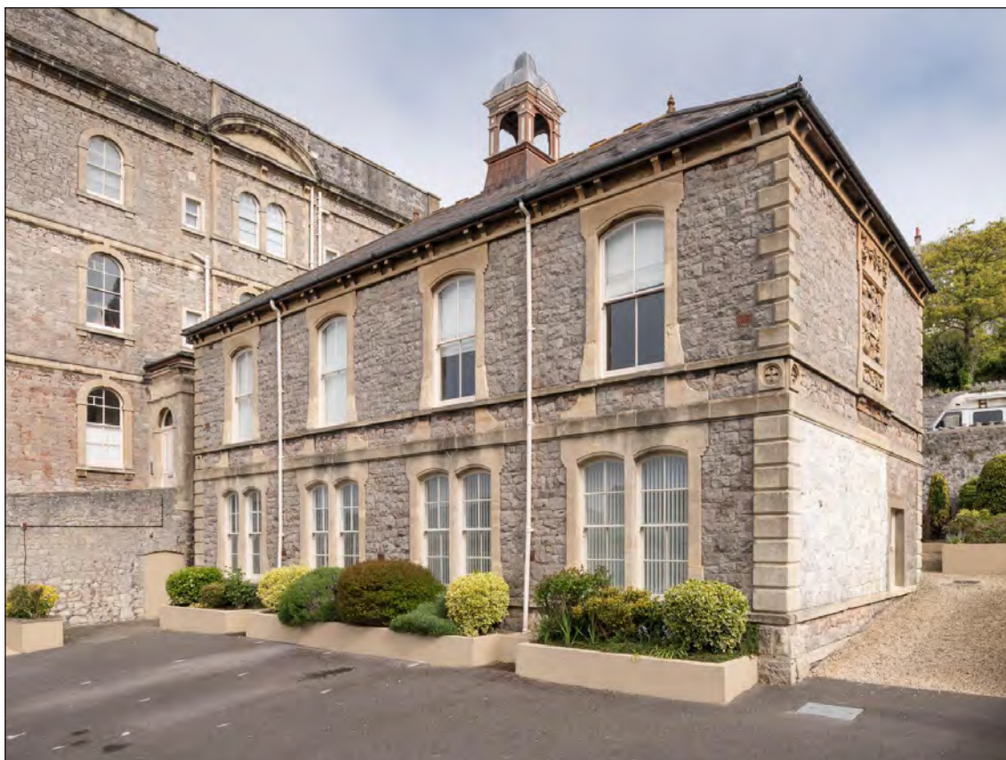
Figure 57: The extension to St Peter's Preparatory School in Atlantic Terrace East by Price & Wooler. (DP218643)
