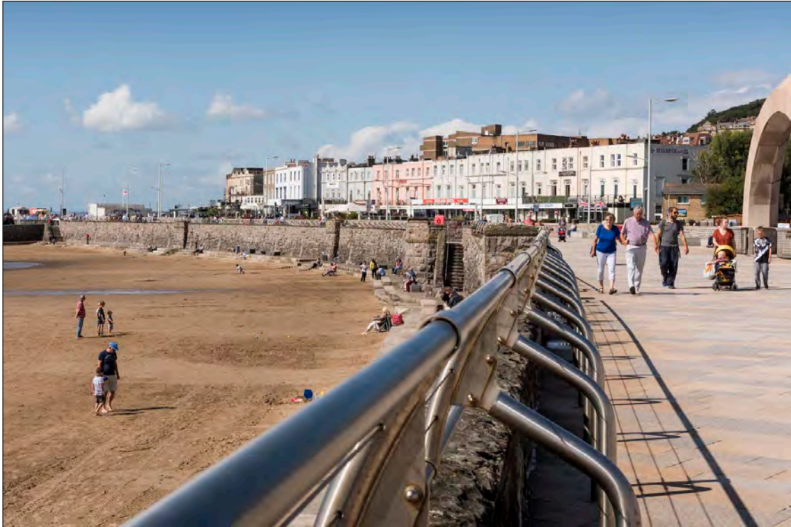
Figure 62: The scheme involved the erection of gently sloping, stone-faced sea walls behind which two miles (3.2km) of seafront promenade was created. Wind-shelters and seats were provided at frequent intervals. The work cost about £35,000 and required 1 million tons of stone. (DP218026)
