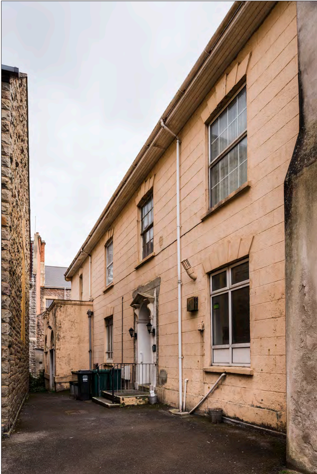
Figure 8: Originally three-bays wide and symmetrical, a fourth bay in a similar style was added to the east of Parsley's Whitecross House between 1903 and 1931, by which time the building was being used as a Sunday School. (DP218260)
