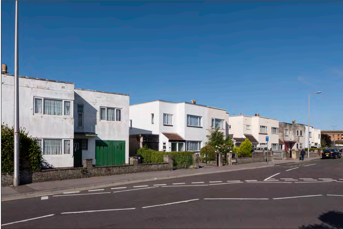
Figure 95: This modern photograph shows some of the Art Deco houses in Station Road, built in around 1934 to designs by Leete & Darby. (DP218280)
