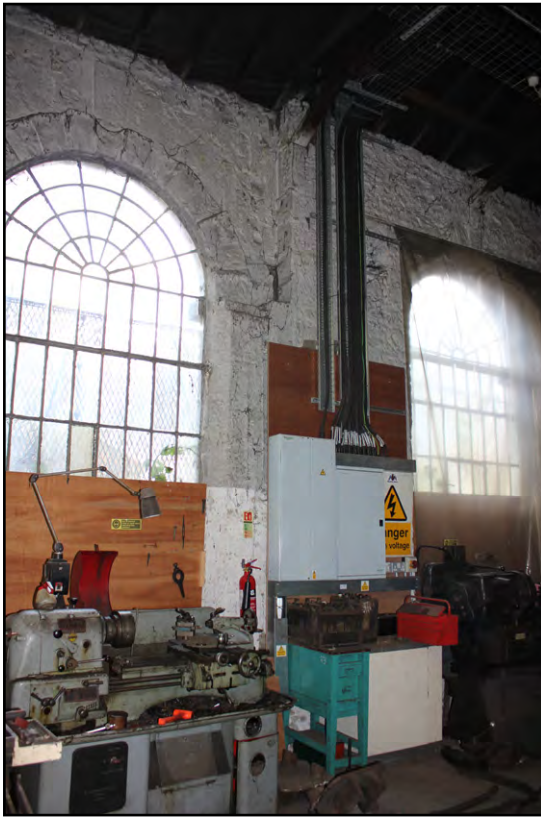
Figure 11: South wall, bays 3 and 4 showing the pattern of thin / thick walls above the arches
