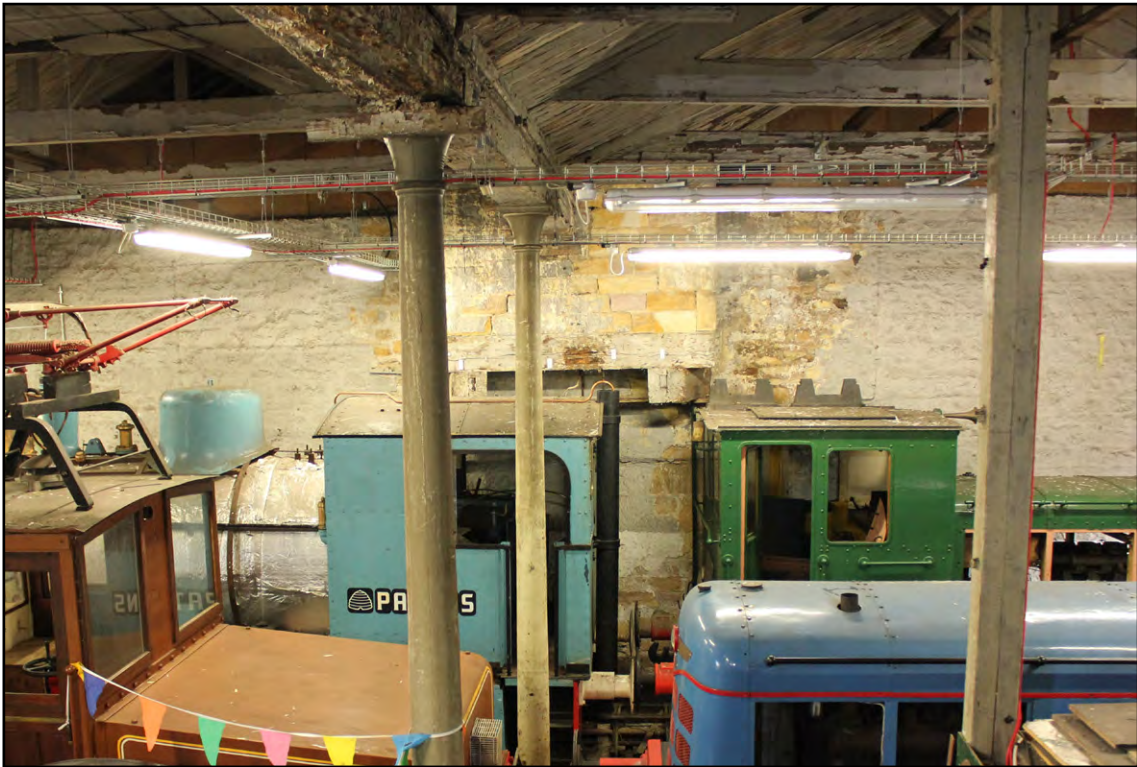
Figure 36: The western cell looking east. Note the slender cast-iron columns, and uppers section of tower cantilevered out on heavy timber beams
