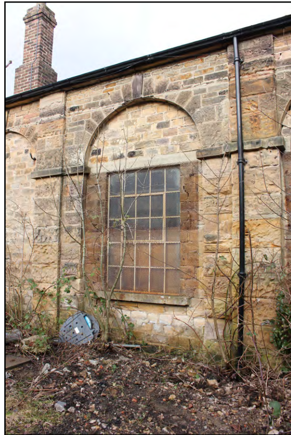
Figure 19: Bay 5. Its different arrangement suggests it may have been for pedestrian or cart access
