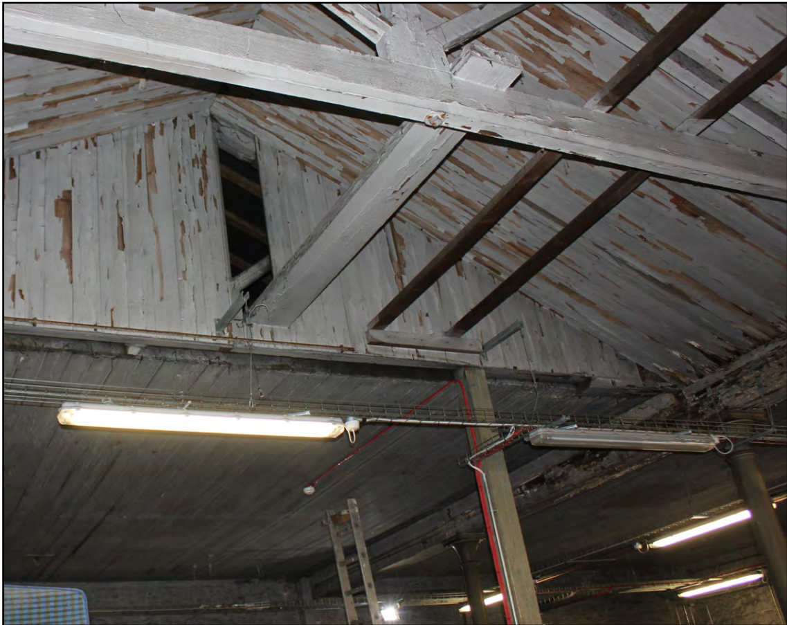
Figure 42: Timber tongue-and-groove ceiling and sarking
