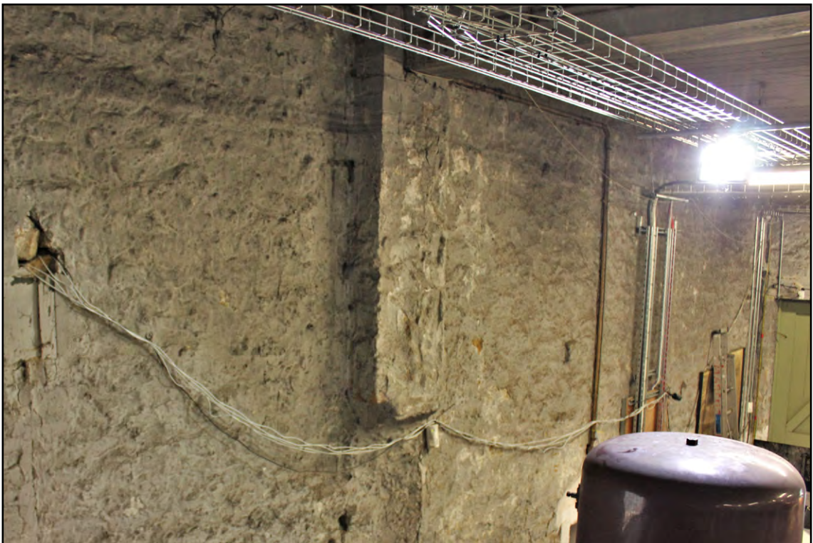
Figure 21: Masonry stub, of what was probably the north wall
