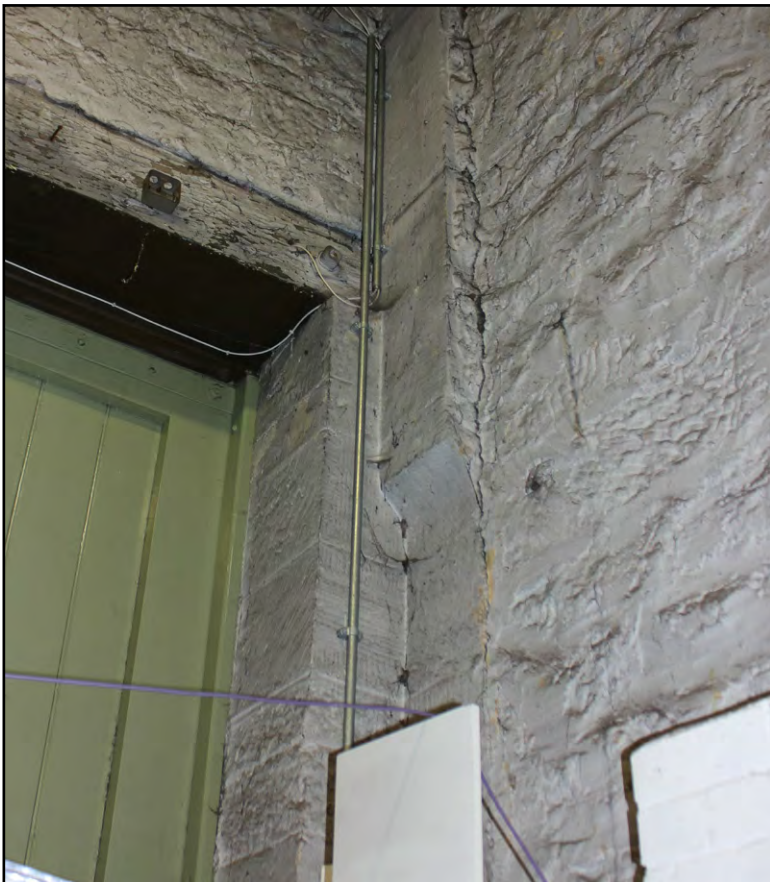
Figure 32. Remnant of shouldered arch to bay 5
