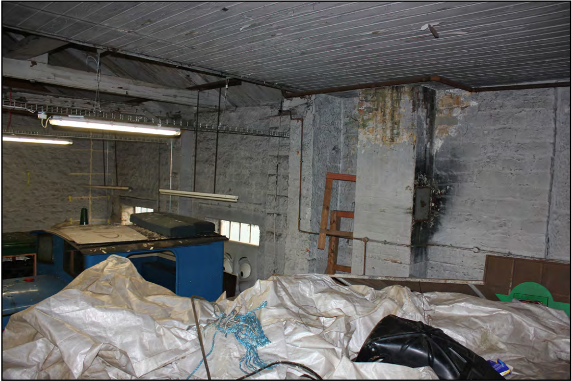
Figure 20: The internal south wall, western wall. The series of rusticated piers, a wall stub with heavy tooling and a chimney flue characterise this elevation
