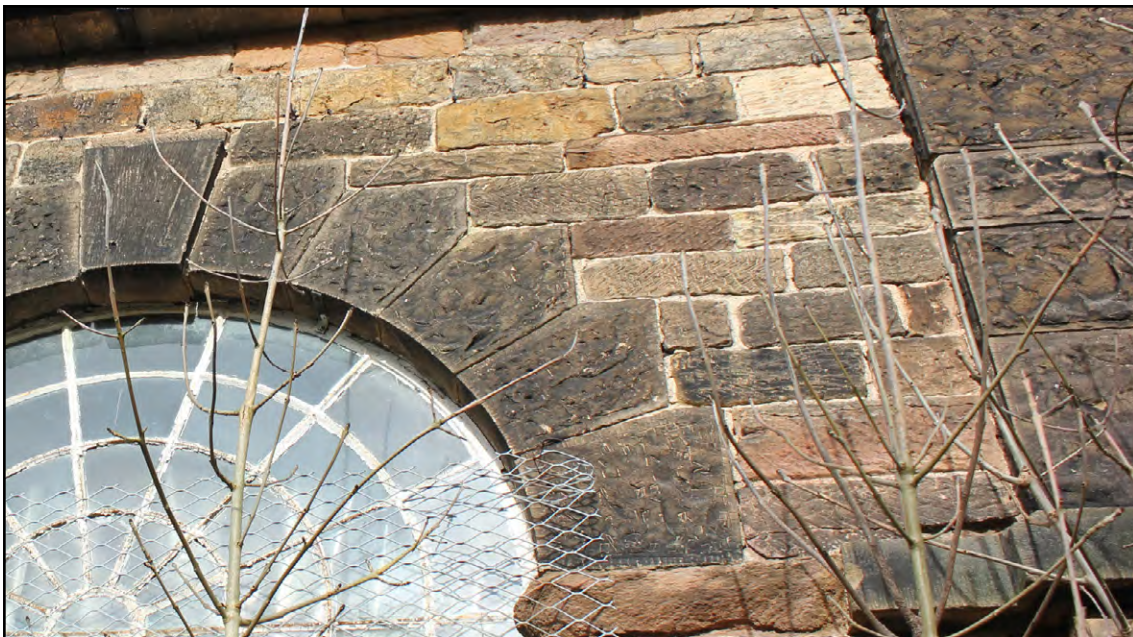
Figure 10: Bay 4 - detail of tooling, south elevation
