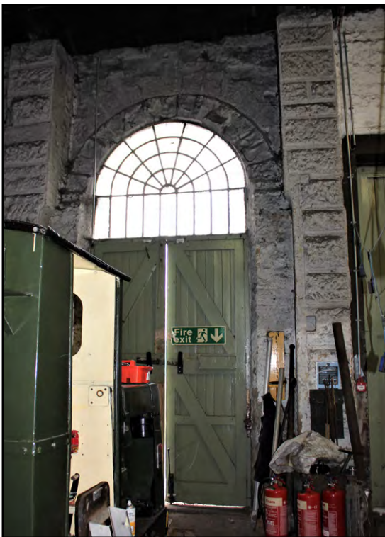
Figure 28: Interior of bay 3 showing rusticated piers
