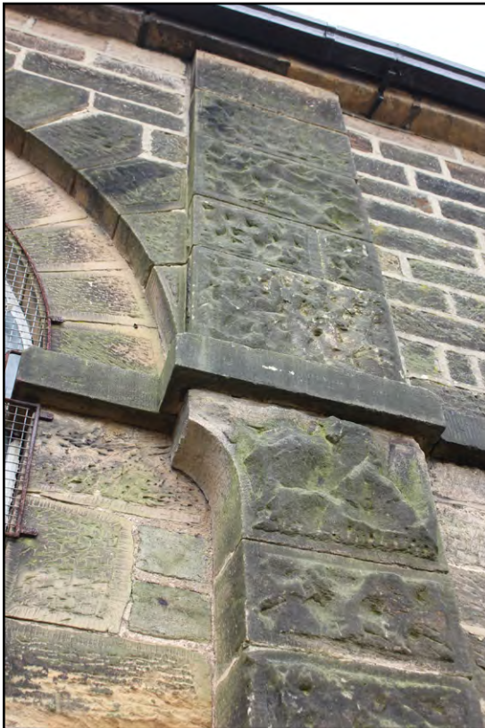
Figure 26: Detail of shouldered arch to bay 3 with later arched infill
