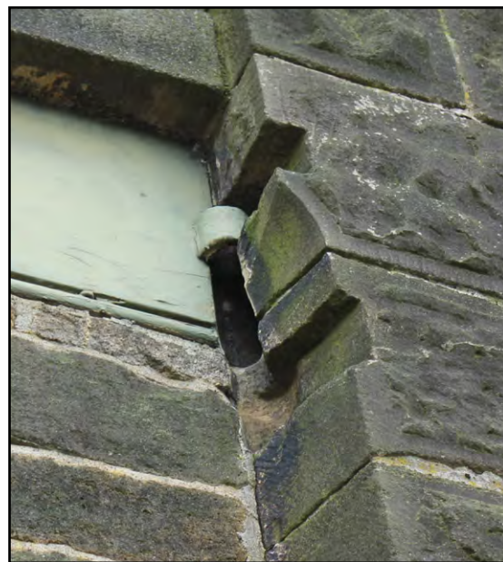
Figure 44: Empty slots and part of a hinge to bay 7. Note the careful tooling
