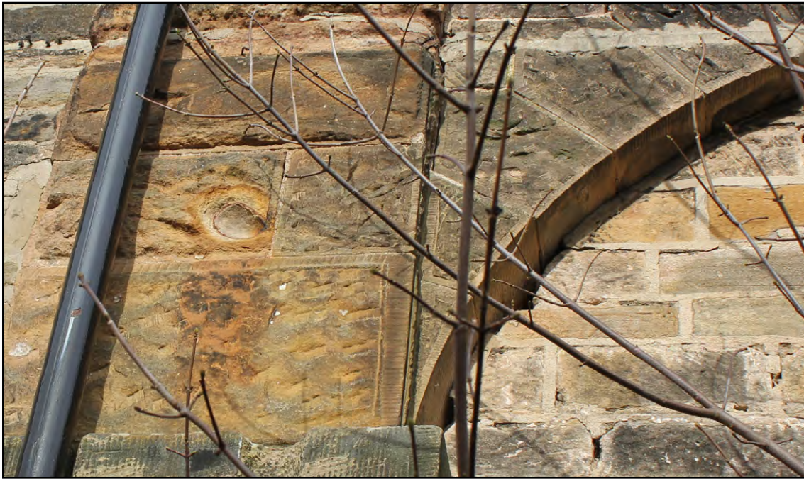
Figure 18: Pier between bay 5 and 6 showing different tooling to that of Phase 1
