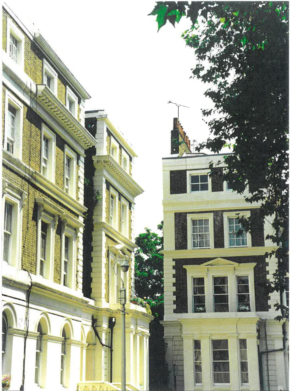
Fig. 33 The upper stages of No. 33 Albert Square shows distinct signs of having been rebuilt at some stage. The brick is of a different type, there is a loss of the upper entablature, and the topmost cornice is also of reduced form.
