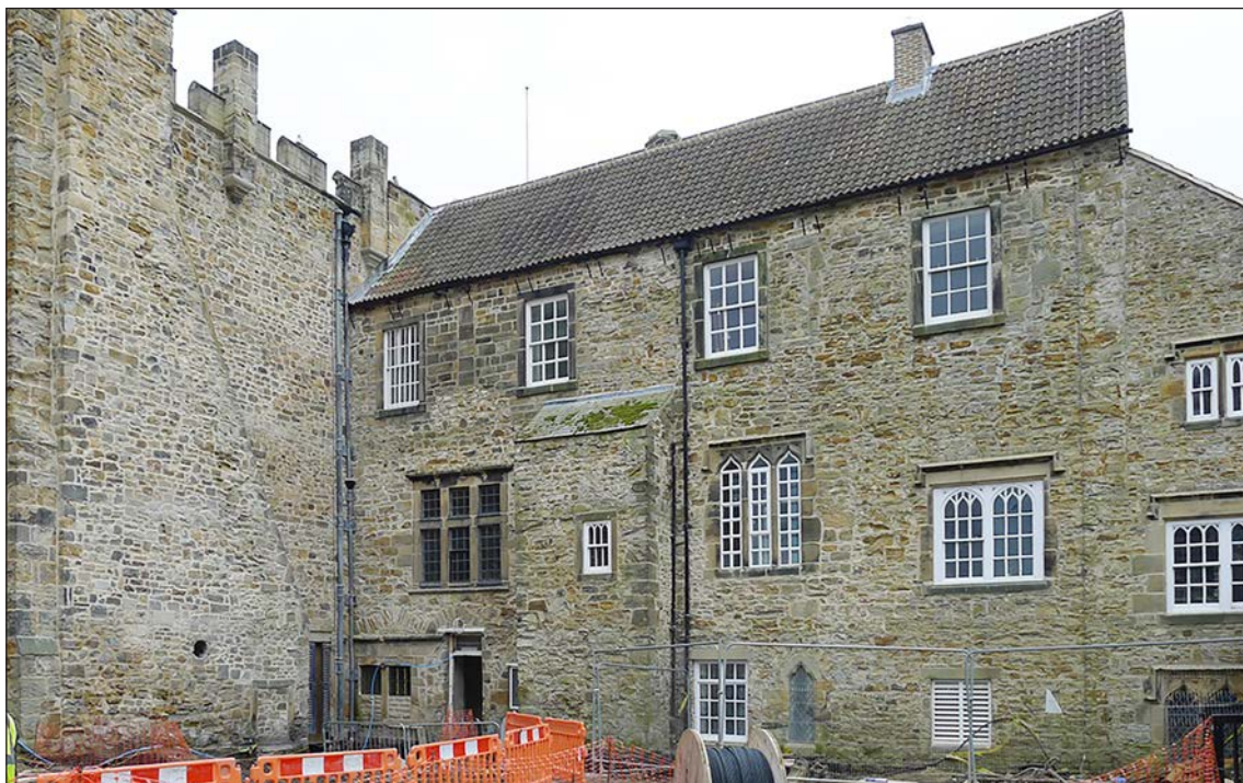
Figure 48: The L-shaped range at Auckland Castle, from the north-west, probably built in the early 14th century and much adapted in successive centuries, viewed from the north-west (© Historic England, photograph taken by Rebecca Pullen, 2019)
