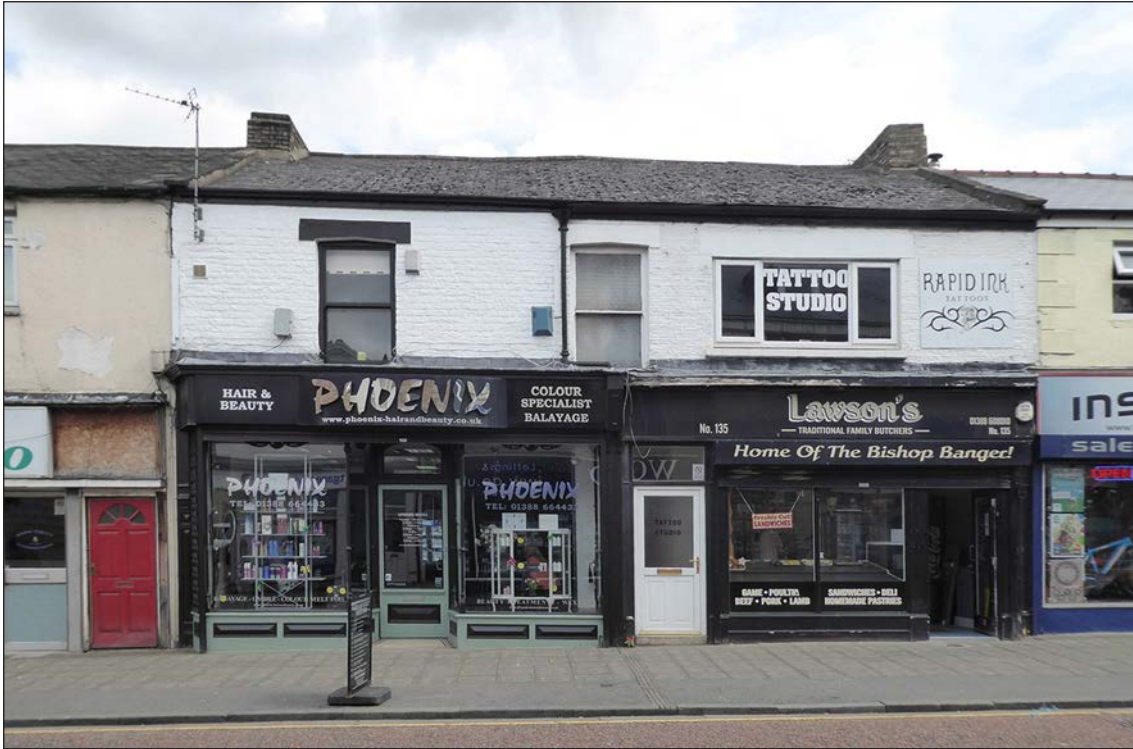
Figure 151: No. 131 Newgate Street (Phoenix Hair and Beauty) with an altered later 19th-century shopfront; viewed from the west (© Historic England, photograph taken by Hilary Gould, 2019)
