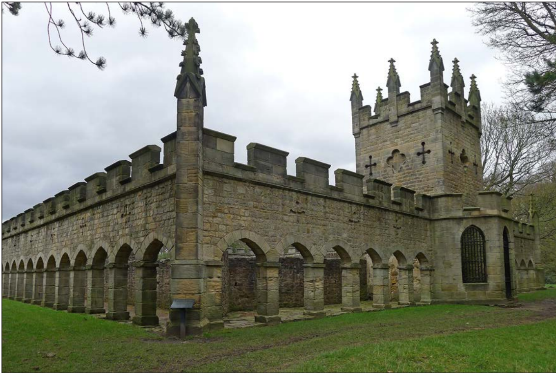
Figure 56: The 18th-century deer shelter, designed by Thomas Wright for Bishop William Trevor, viewed from the west (© Historic England, photograph taken by Rebecca Pullen, 2019)
