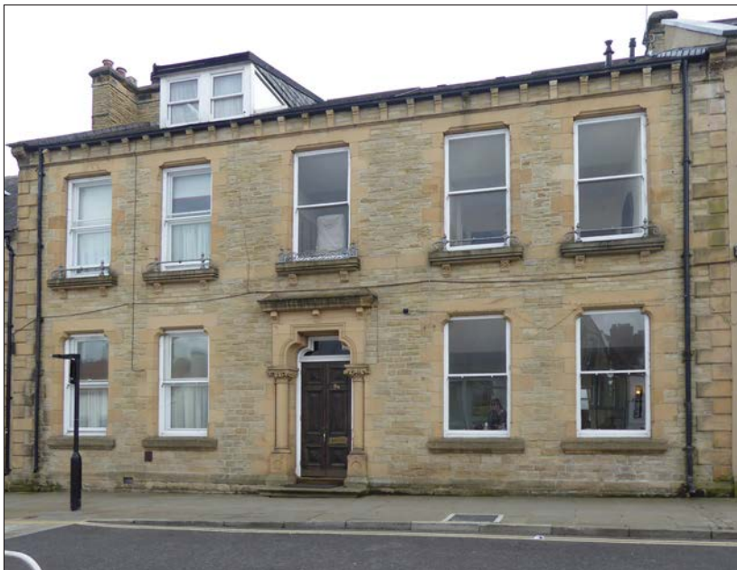
Figure 84: No. 9a Market Place, the former Mount School, viewed from the north (© Historic England, photograph taken by Jayne Rimmer, 2019)
