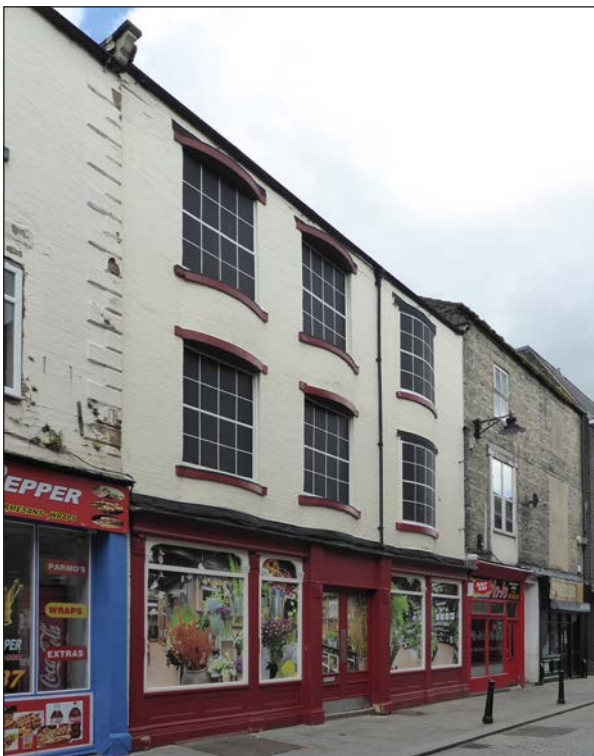
Figure 102: Nos. 65-66 Fore Bondgate (formerly Bar Mondo), a late 18th century former house that was later converted into a public house; viewed from the south-west (© Historic England, photograph taken by Clare Howard, 2019)
