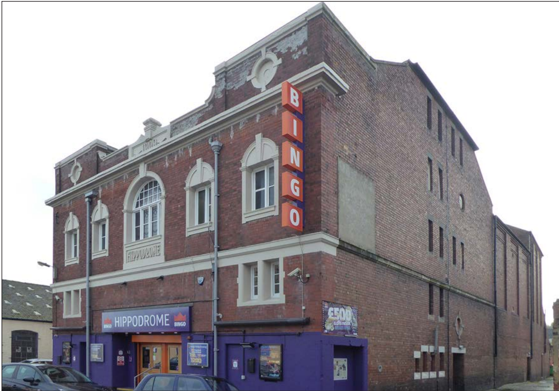
Figure 171: The Hippodrome, Railway Street, former cine-variety theatre, viewed from the north-west (© Historic England, photograph taken by Clare Howard, 2019)
