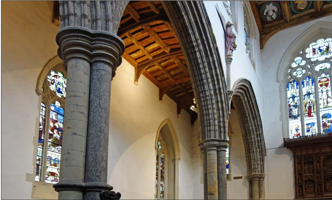
Figure 5: View of the north arcade inside the Chapel of St Peter, Auckland Castle, showing the mixed use of different stone for the columns, intended to create visual interest (© Historic England, photograph taken by Rebecca Pullen 2019)
