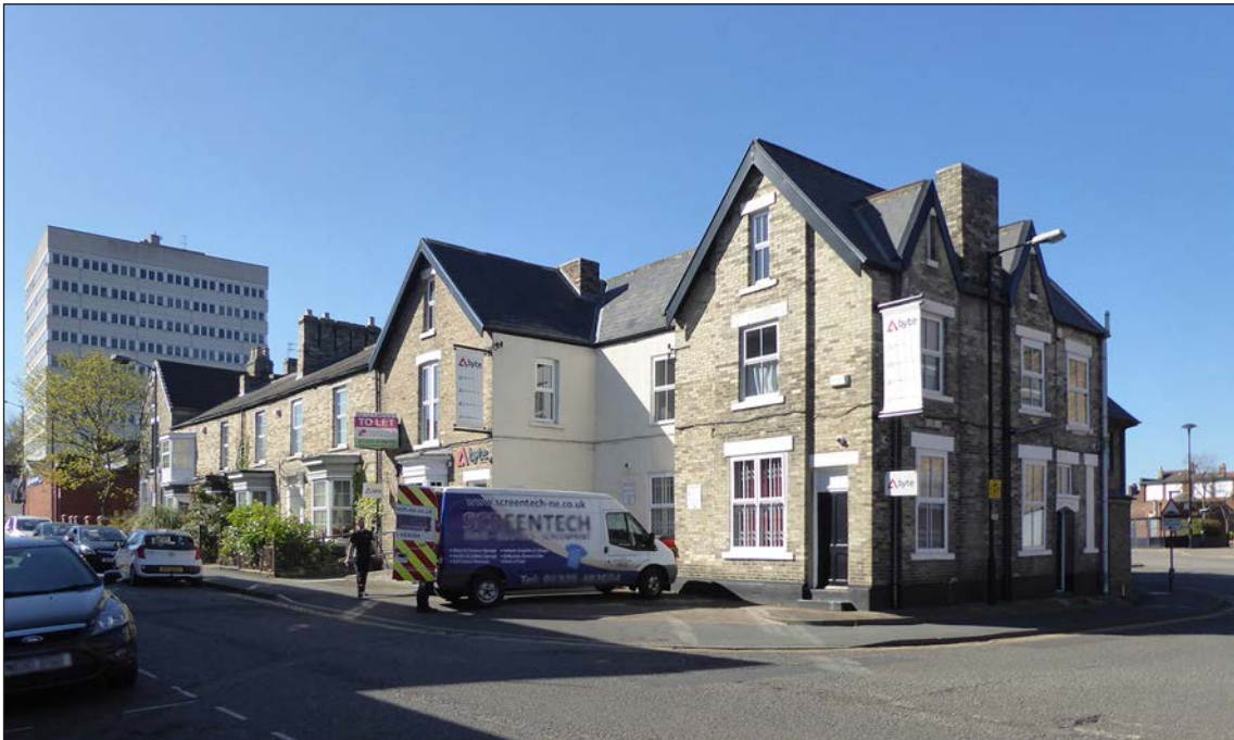
Figure 143: Nos. 13 to 16 Tenters Street, built as a row of houses in cream brick with pitched slate roofs; viewed from the south-east (© Historic England, photograph taken by Clare Howard 2019)
