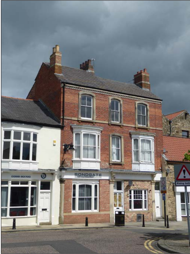
Figure 103: No. 36 Fore Bondgate, a tall three-storey building to the north of the road; viewed from the south-west (© Historic England, photograph taken by Clare Howard, 2019)
