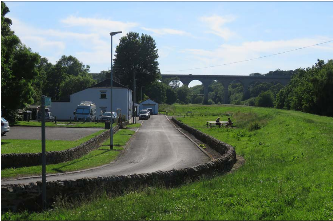
Figure 97: General view along Batts Terrace, looking west towards Newton Cap Viaduct, with the flood embankment seen to the right; viewed from the east (© Historic England, Clare Howard, 2020)
