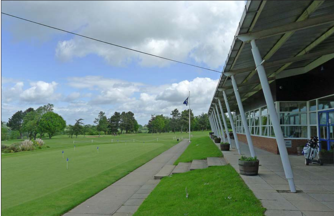
Figure 66: The north-west frontage of the club house at Bishop Auckland Golf Club with the course extending out in front; viewed from the south-west (© Historic England, photograph taken by Rebecca Pullen, 2019)
