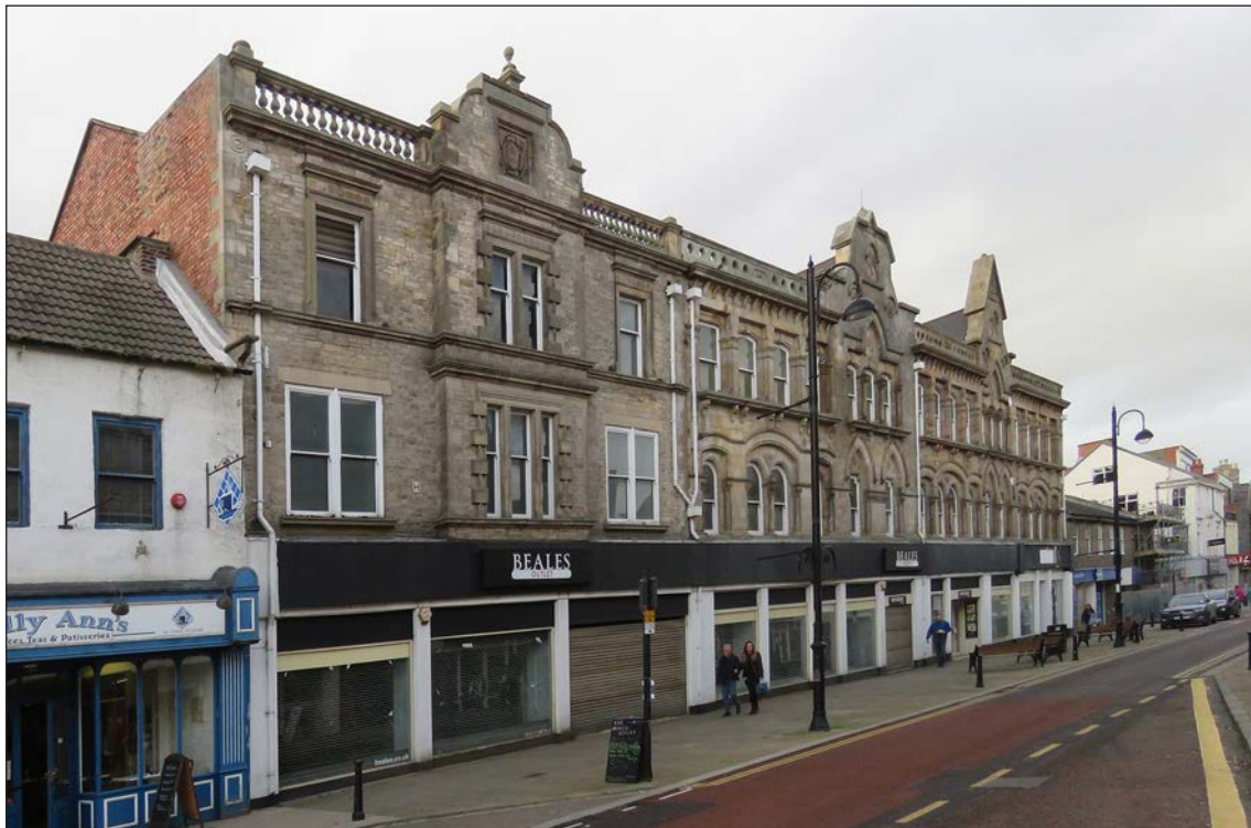
Figure 139: The imposing three-storey row of the former Co-operative Central Stores at no. 80 Newgate Street, viewed from the south-east (© Historic England, photograph taken by Clare Howard, 2018)
