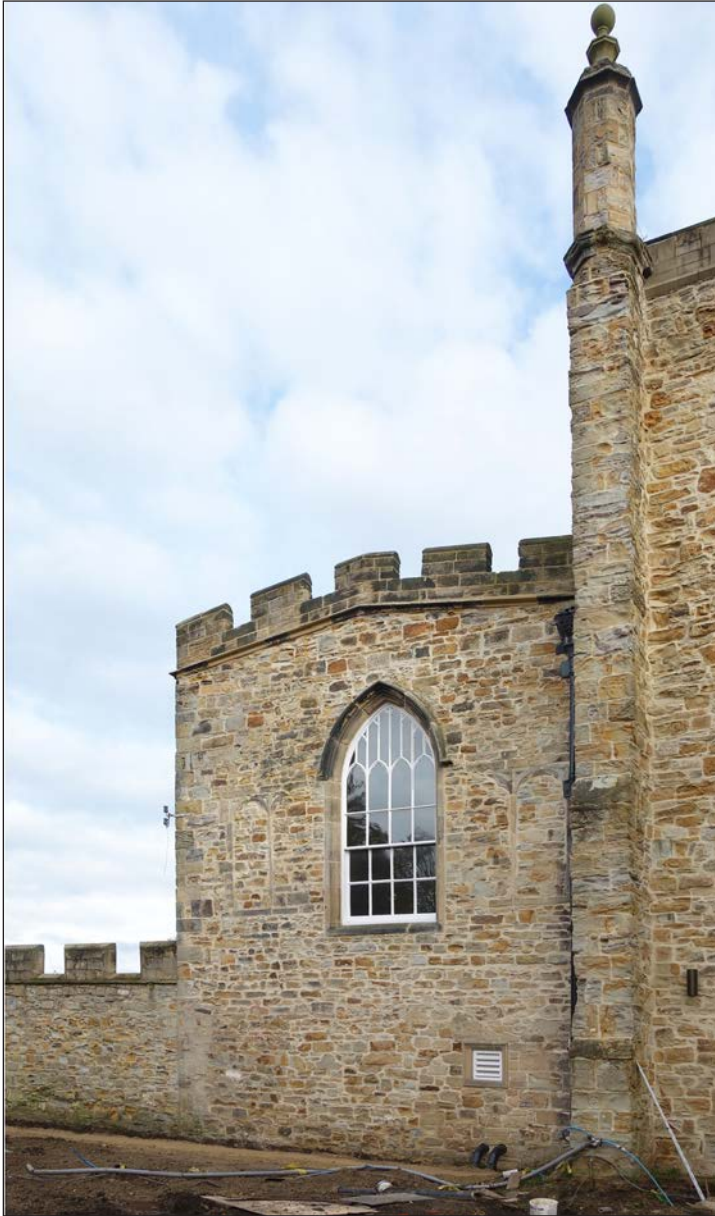
Figure 49: The link block on the north side of Bishop Bek's two-storey chamber block, viewed from the west (© Historic England, photograph taken by Rebecca Pullen, 2019)
