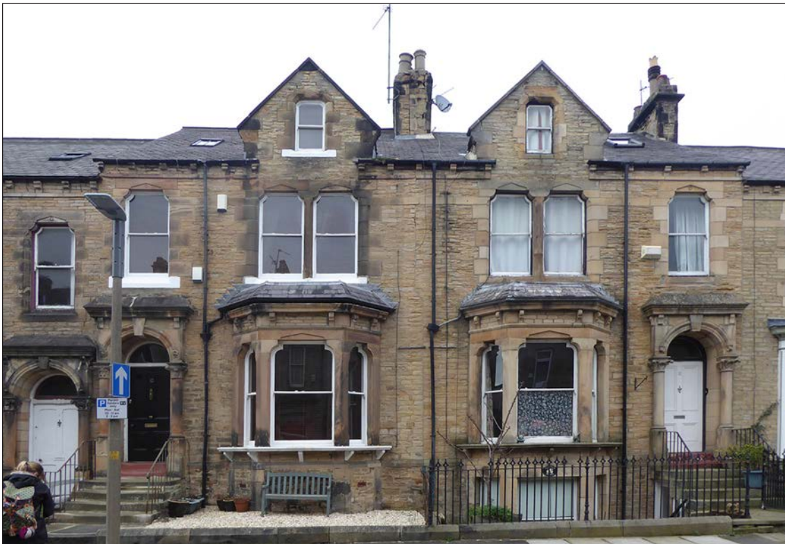
Figure 182: Nos. 10 and 11 Victoria Avenue, viewed from the south (© Historic England, photograph taken by Clare Howard, 2019)
