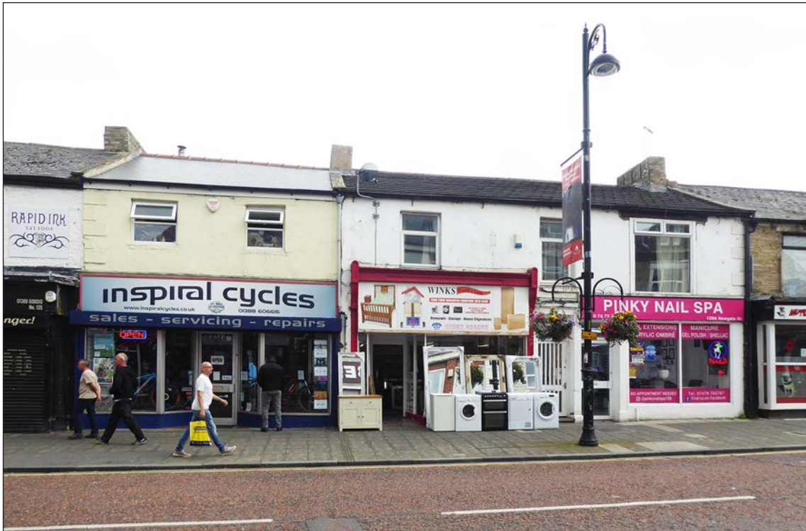
Figure 149: Nos. 137-139a Newgate Street, former terraced housing to the east side of the street, viewed from the west (© Historic England, photograph taken by Hilary Gould, 2019)
