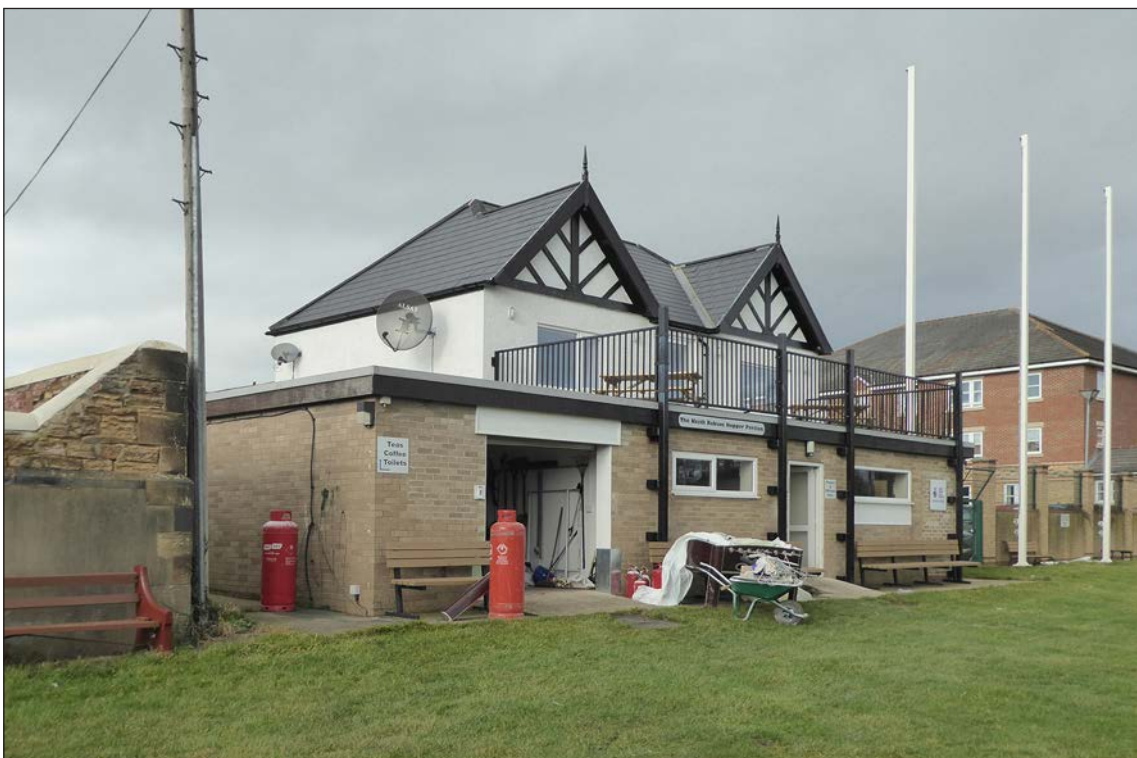
Figure 185: Bishop Auckland Cricket Club was built in the early 20th century and extended in the late 20th century; viewed from the south-east (© Historic England, photograph taken by Clare Howard, 2019)
