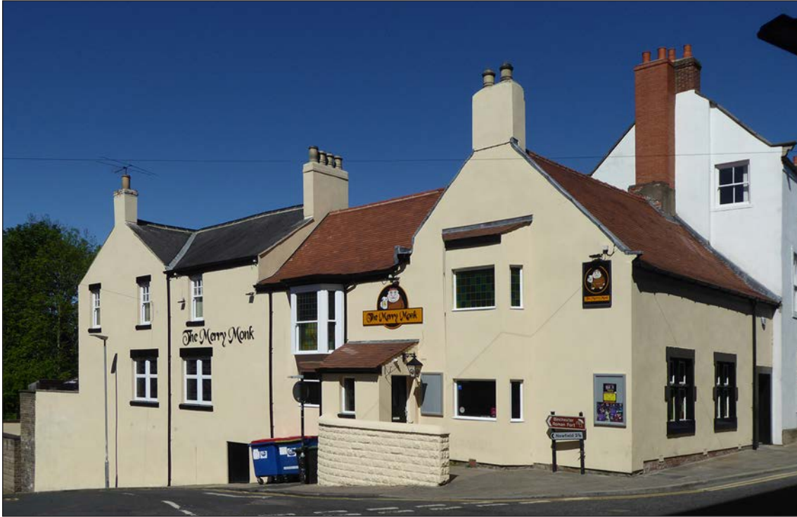
Figure 75: No. 30 Market Place, The Merry Monk public house has a front range which may date to the late 17th century; viewed from the south-west (© Historic England, photograph taken by Clare Howard, 2019)
