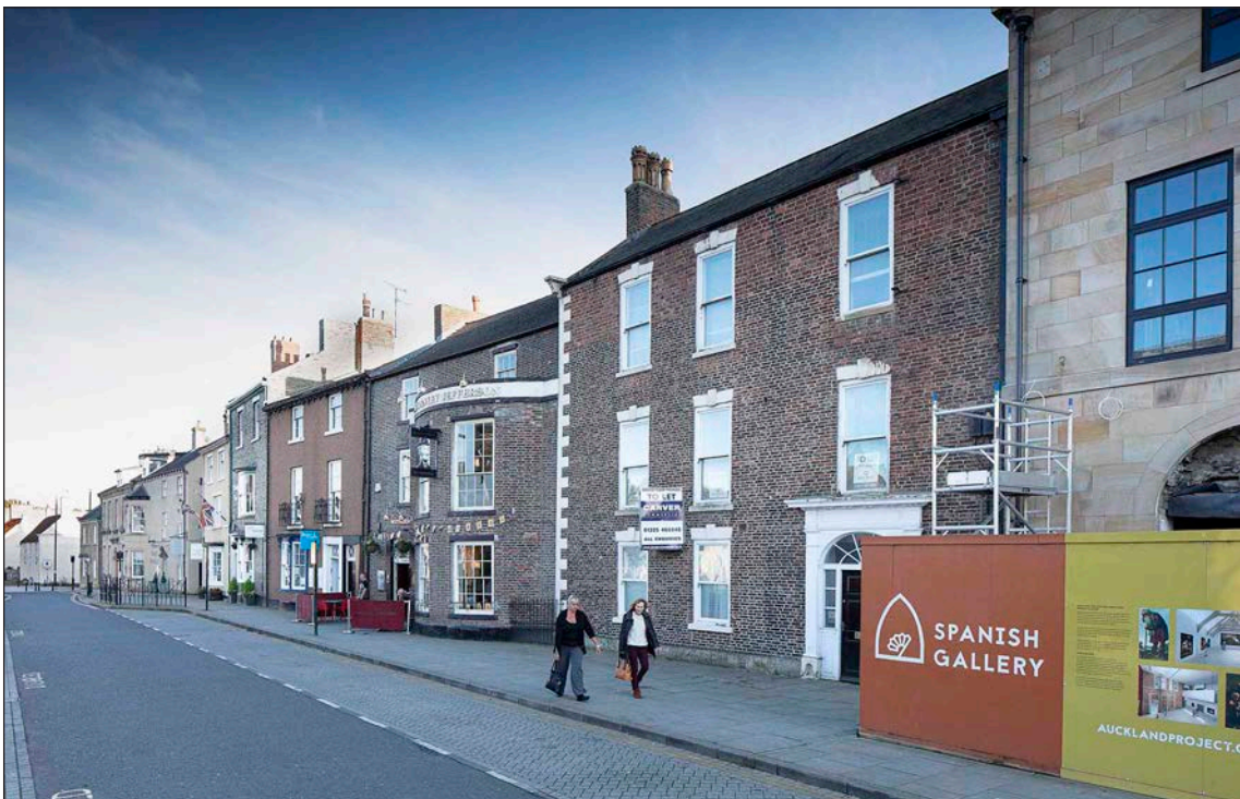
Figure 77: Buildings to the south side of the Market Place, including no. 4 Market Place, the former vicarage of the Church of St Andrew and no. 5 Market Place, the Stanley Jefferson public house; viewed from the north-west (DP234521 © Historic England Archive, photograph taken by Alun Bull, 16 October 2019)
