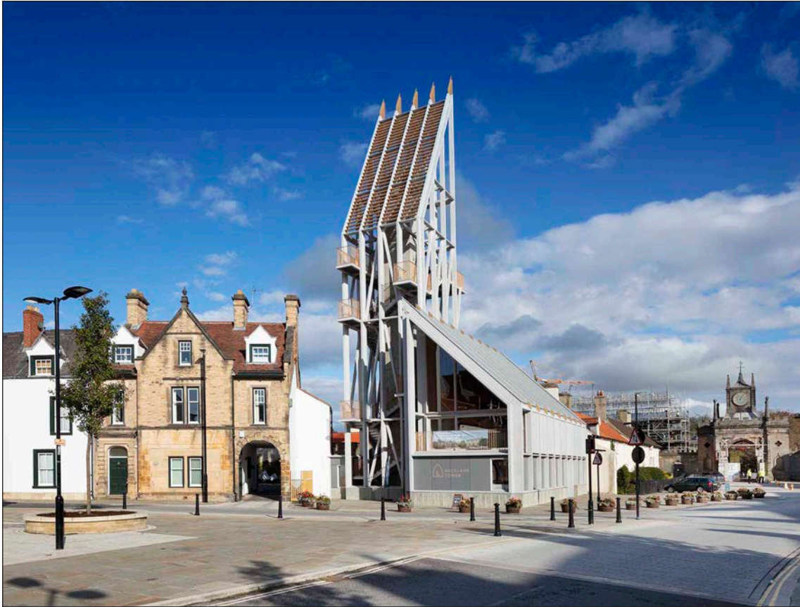
Figure 32: Auckland Tower, viewed from the west, with the entrance to Auckland Castle far right (DP234729 © Historic England Archive, photograph taken by Alun Bull, 16 October 2019)
