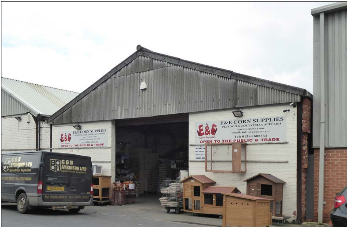
Figure 165: No. 19 Peel Street (E & E Corn Supplies), viewed from the north-west (© Historic England, photograph taken by Hilary Gould, 2019)
