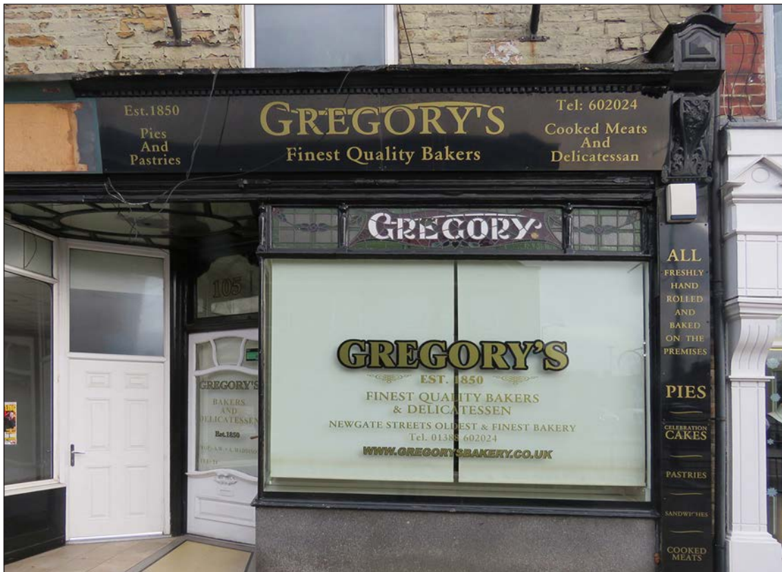
Figure 135: Nos. 103 and 105, partly occupied by Gregory's butchers who have occupied the same building since at least 1871. The shopfront complete with stained glass is a significant survival. Viewed from the west (© Historic England, photograph taken by Clare Howard, 2018)
