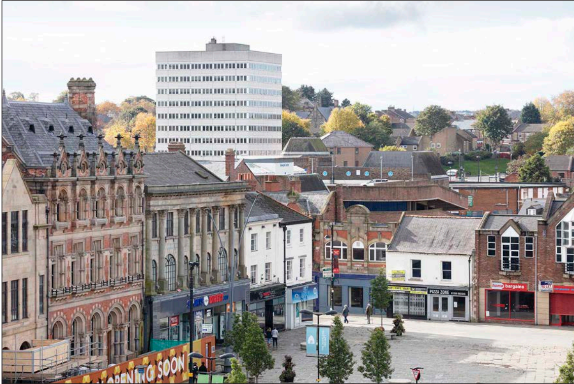
Figure 30: The former Department of Health and Social Security building dominating the skyline behind the buildings of the Market Place, viewed from the north-east (DP234719 © Historic England Archive, photograph taken by Alun Bull, 16 October 2019)
