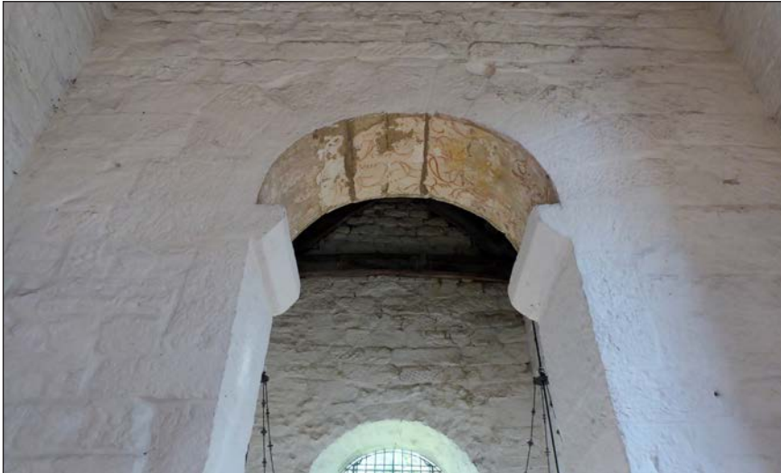
Figure 6: The chancel arch at Escomb church possibly built using Roman stone (© Historic England, photograph taken by Clare Howard, 2019)
