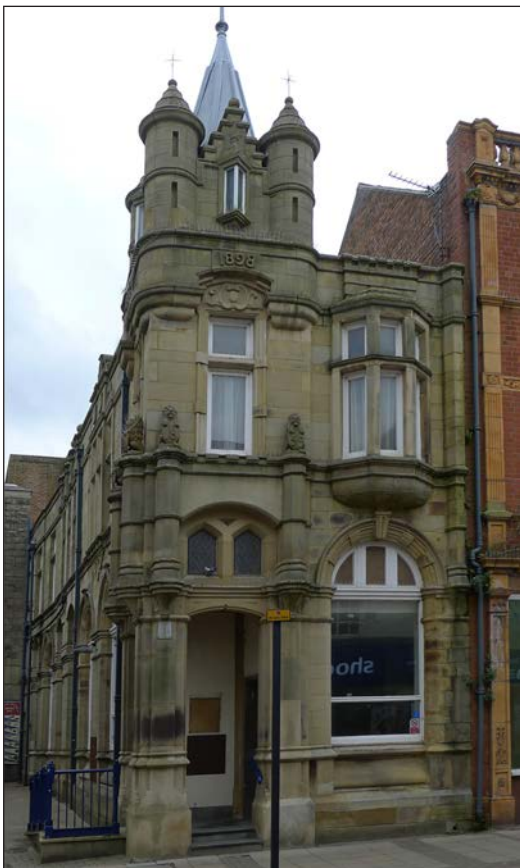
Figure 116: Former Yorkshire Penny Bank (no. 18 Newgate Street), built 1898; viewed from the east (© Historic England, photograph taken by Hilary Gould, 2019)
