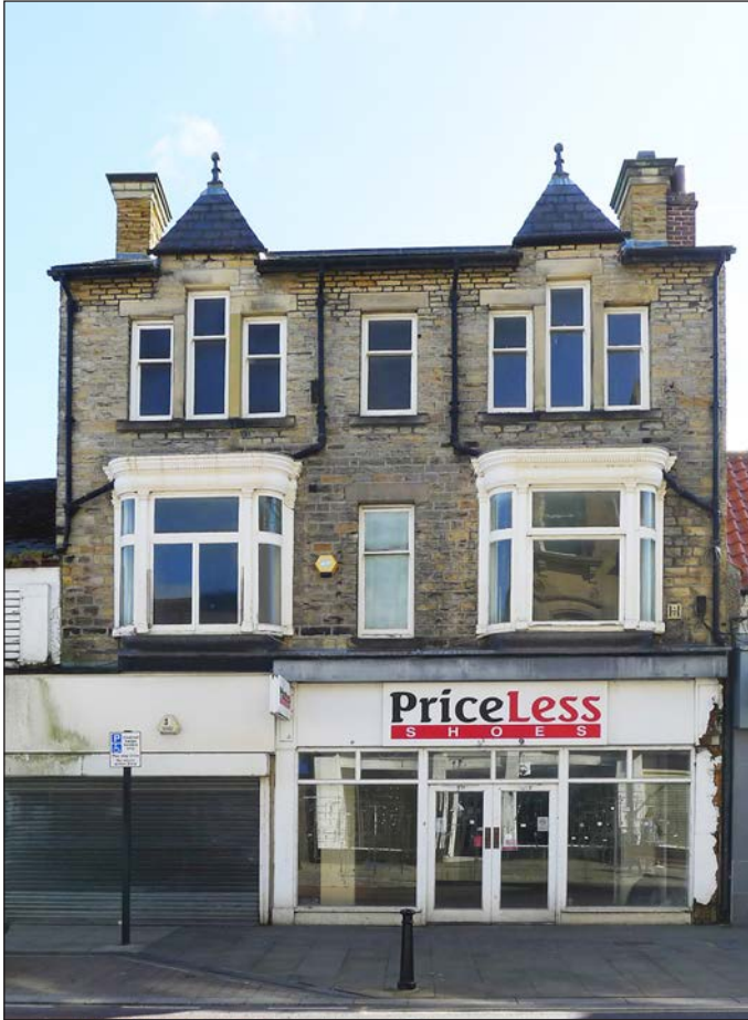
Figure 133: No. 67 Newgate Street built in the late 19th or early 20th century; viewed from the east (© Historic England, photograph taken by Hilary Gould, 2019)
