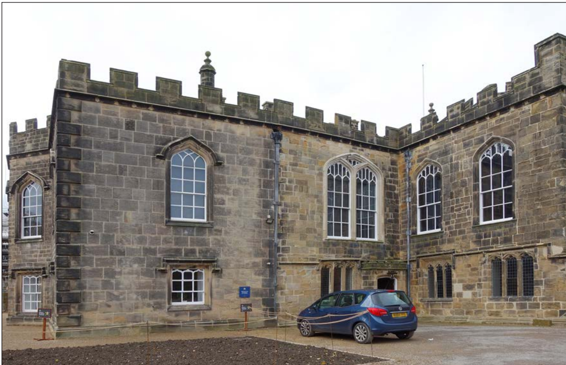
Figure 51: The east elevation of the south range showing the construction break between the 16th-century extension to the right and the mid-18th century addition by Bishop Trevor to the left (© Historic England, photograph taken by Rebecca Pullen, 2019)
