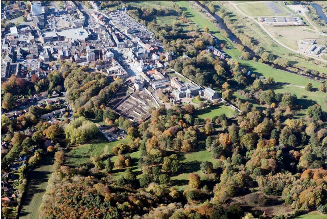
Figure 36: Oblique aerial photograph showing Auckland Castle, adjacent formal gardens, and the distinctive terraces of the walled garden, during major refurbishment to the ground and building in 2018, viewed from the south-east and showing the close physical link with the town (Detail from 34095_029 © Historic England Archive, photograph taken by Emma Trevarthen, 18 October 2018)
