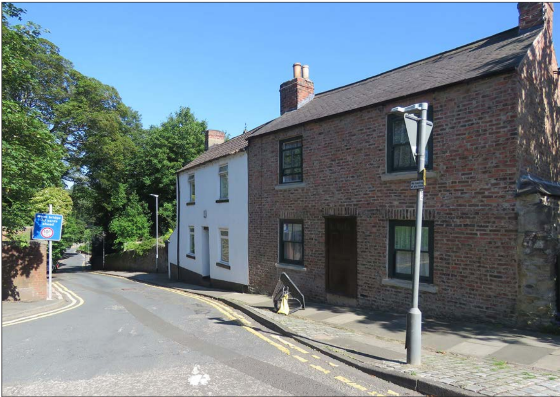
Figure 178: Cottages at the west end of Durham Chare (nos. 23 and 24), viewed from the west (© Historic England, photograph taken by Clare Howard, 2019)
