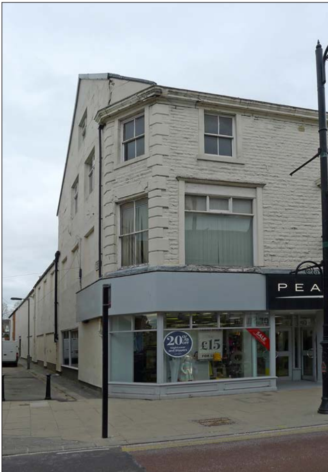
Figure 126: No. 70 Newgate Street has a late 19th-century façade fronting an earlier building perhaps of early 19th-century date; viewed from the east (© Historic England, photograph taken by Hilary Gould, 2019)
