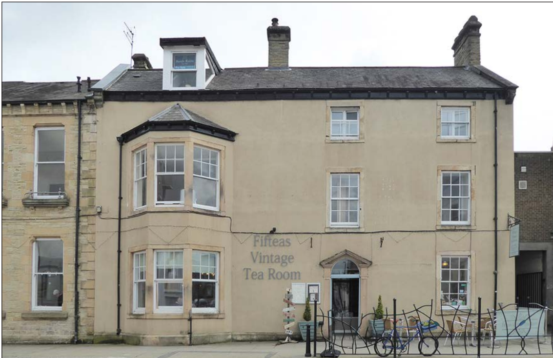
Figure 78: No. 9 Market Place (Fifteas Vintage Tea Room) which became a girls' school from 1864; viewed from the north (© Historic England, photograph taken by Jayne Rimmer, 2019)
