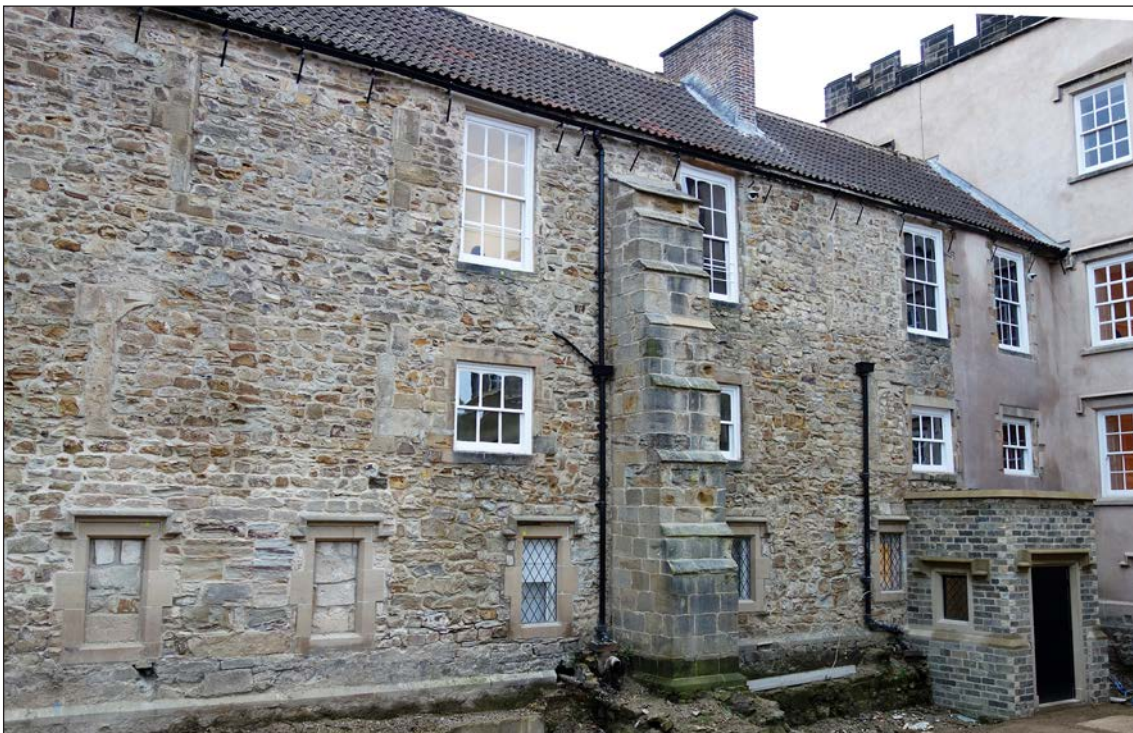
Figure 52: The south elevation of the Scotland Wing, viewed from the south-west showing the blocked multi-light windows and later inserted windows to create a mezzanine and long gallery (© Historic England, photograph taken by Rebecca Pullen, 2019)
