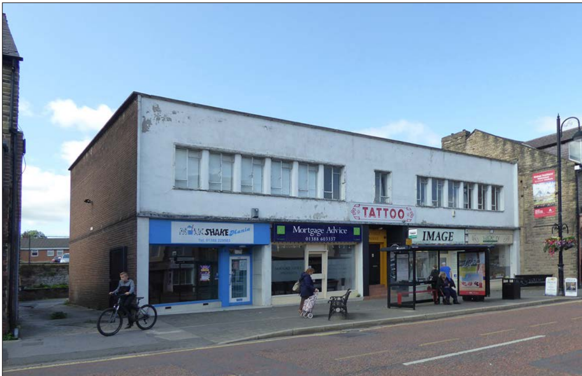
Figure 154: Victoria House, Newgate Street, built in the mid-20th century; viewed from the south-east (© Historic England, photograph taken by Hilary Gould, 2019)
