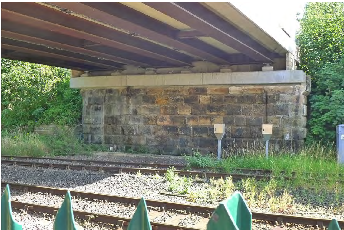
Fig 69. The south abutment of railway overbridge DAE2/10 (Cockton Hill Road). Note the ends of the abutment break forward slightly and are surmounted by large ashlar blocks that corbel out on both sides, suggesting they initially comprised free-standing piers. (© Historic England/Marcus Jecock)
