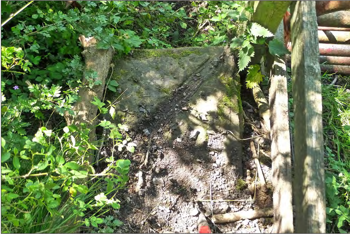
Fig 42. Detail of one of the end pier caps to the retaining walls of railway accommodation bridge BIF/10, showing the 'half-saltire' channelling. (© Historic England/Marcus Jecock)
