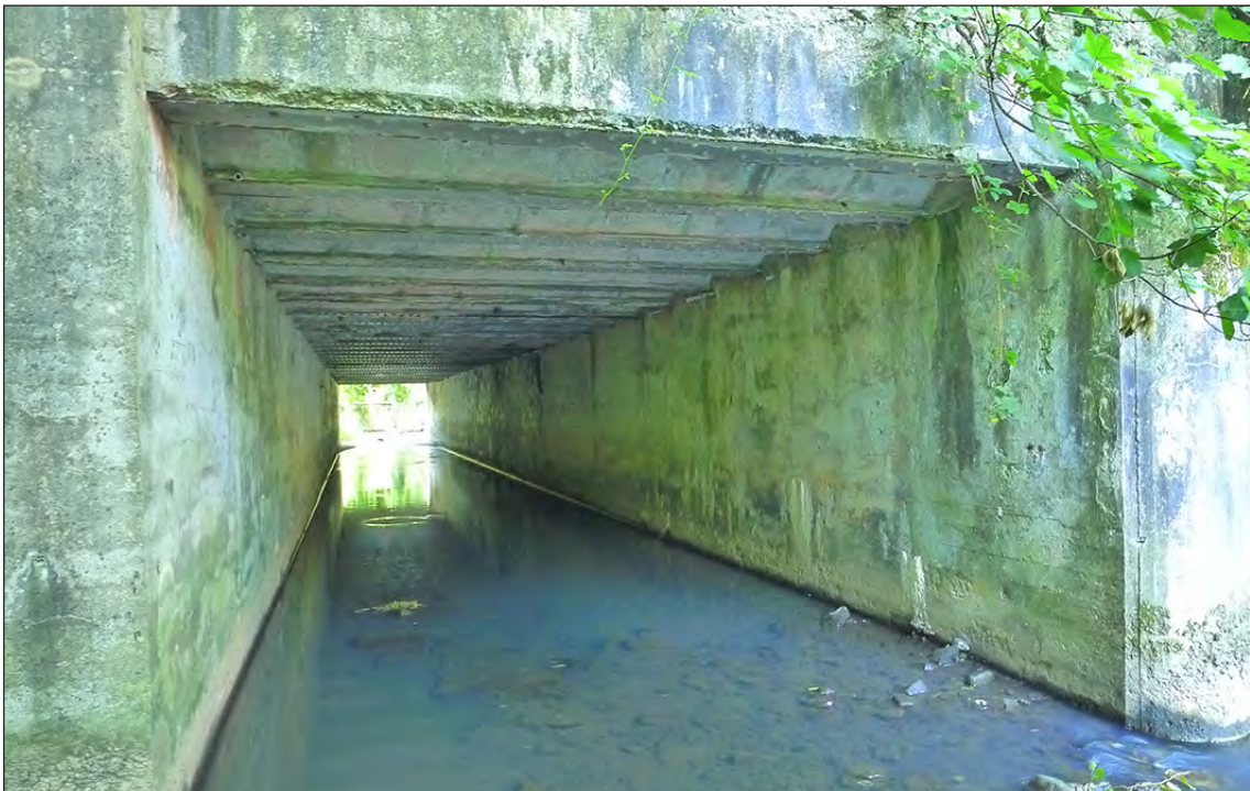
Fig 14. The eastern of the two box conduits of the bridge carrying Durham Road across the River Gaunless., seen from the north. The central spine wall with its bullnose cutwater is at right of frame. Note the soffit formed from steel joists and concrete jack arches. (© Historic England/Marcus Jecock)
