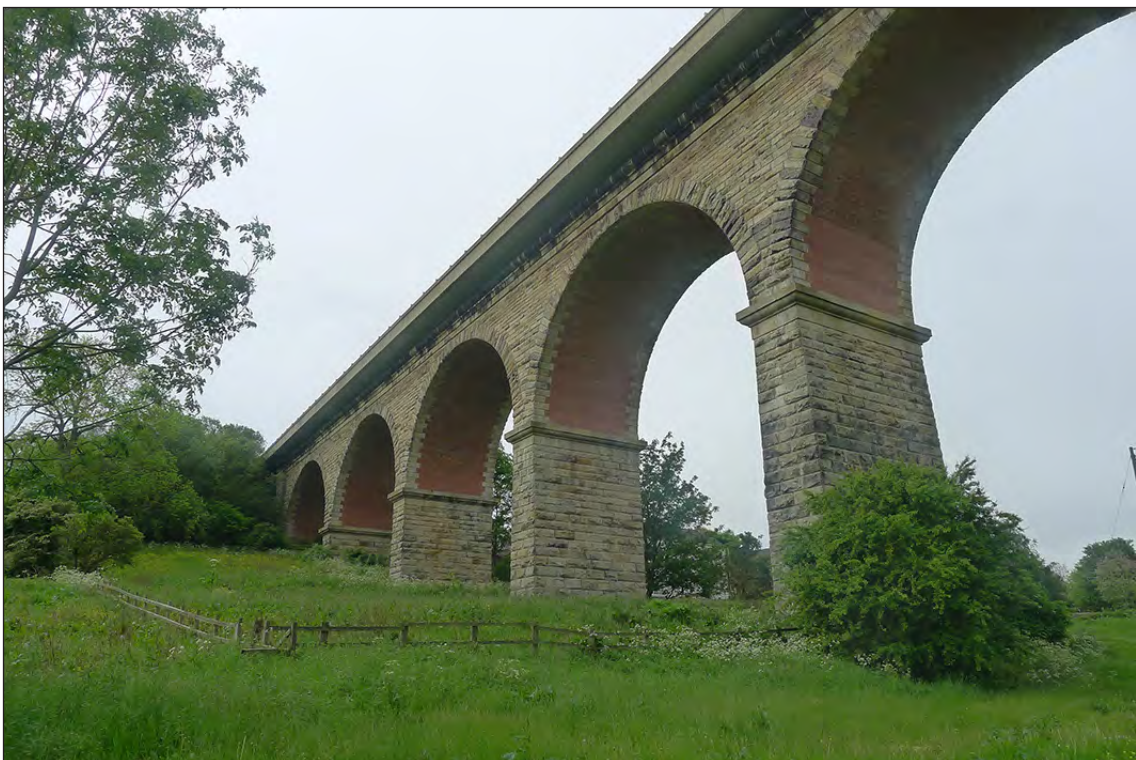
Fig 50. The southern end of Newton Cap Viaduct from the east. Note the modern cantilevered road deck. (© Historic England/Marcus Jecock)
