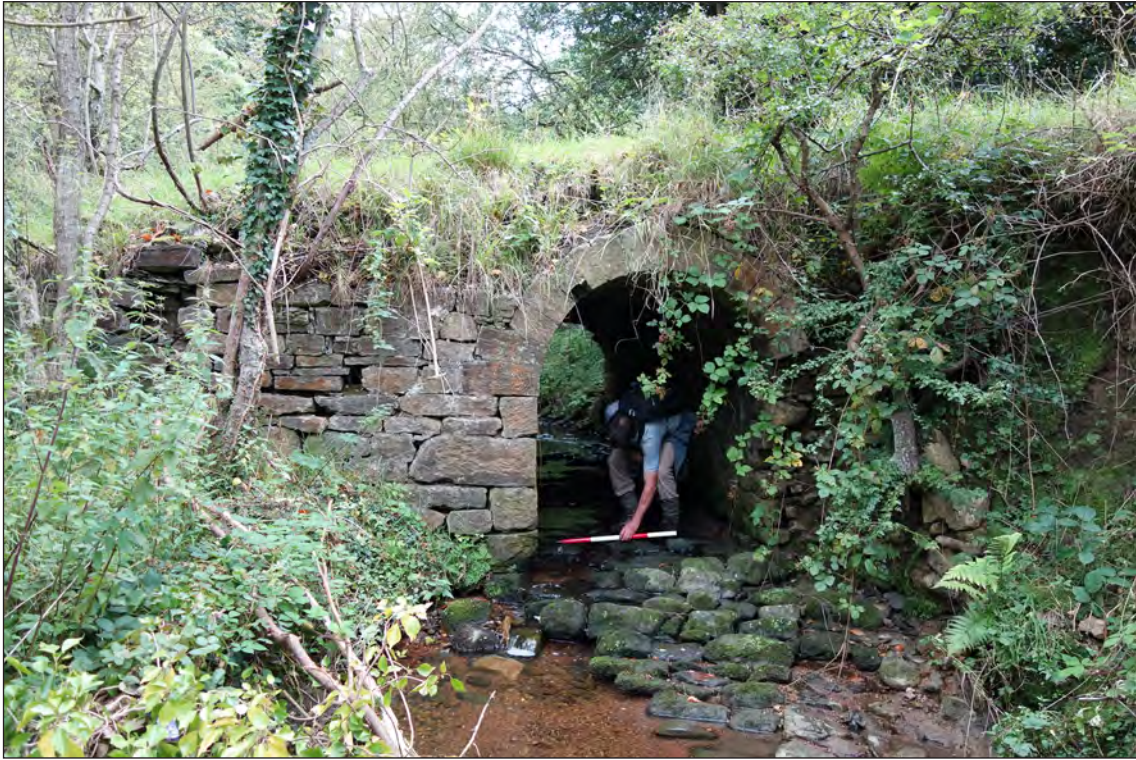
Fig 88. The downstream (western) headwall of 'footbridge no. 3' across the Coundon Burn in Auckland Park. (© Historic England/Rebecca Pullen)
