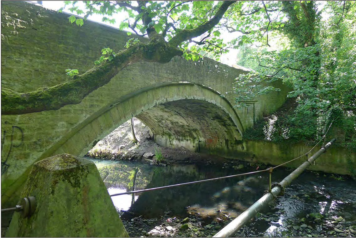
Fig 17. The northern (downstream) elevation of the phase-2 Gaunless Bridge. (© Historic England/Marcus Jecock)
