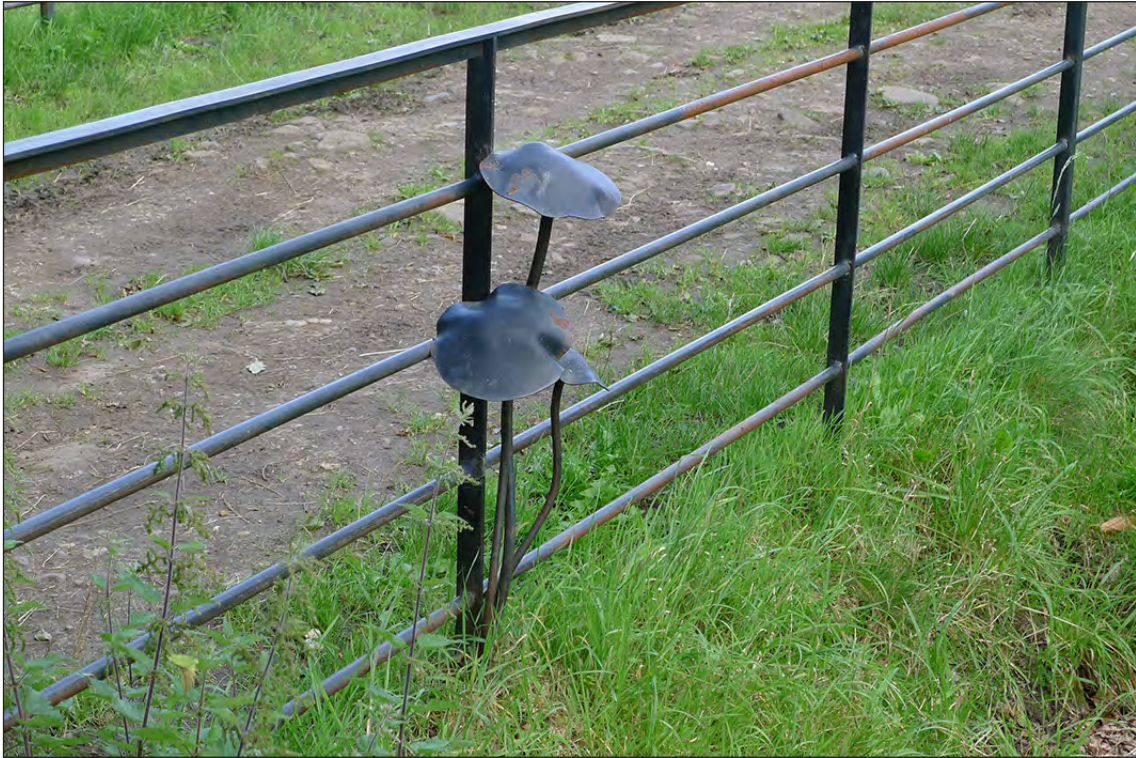
Fig 82. Detail of the modern railings to 'Bishop Trevor's' culvert for the Coundon Burn in Auckland Park. (© Historic England/Marcus Jecock)
