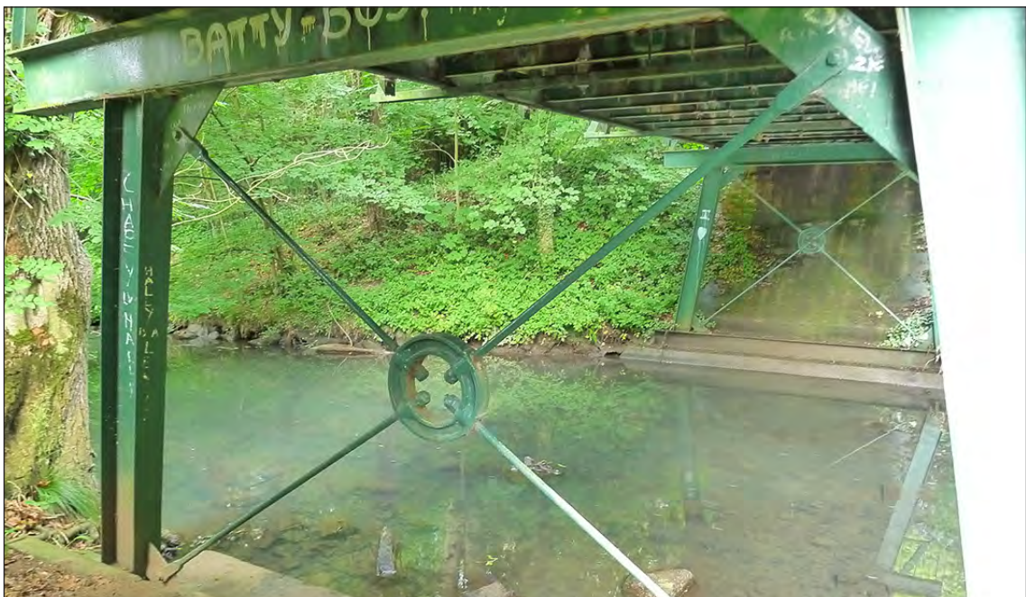
Fig 21. The support trestles to the pony truss in Bishop Auckland Cemetery (© Historic England/Marcus Jecock)
