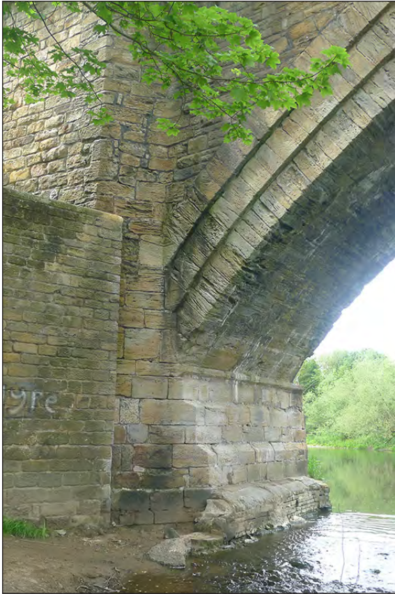
Fig 9. The face of the southern abutment of Newton Cap Bridge. (© Historic England/Marcus Jecock)
