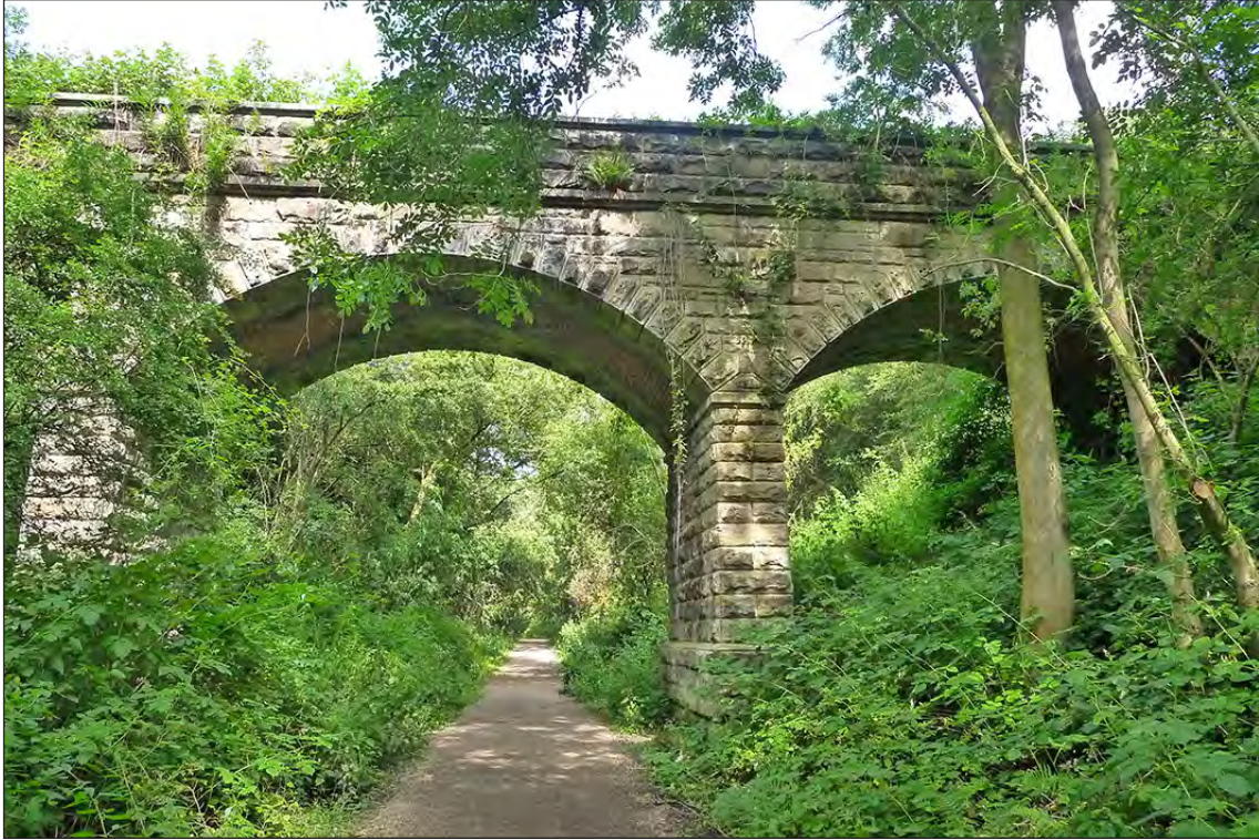
Fig 28. The south-western elevation of railway accommodation bridge BIF/5, showing the central and eastern spans. (© Historic England/Marcus Jecock)
