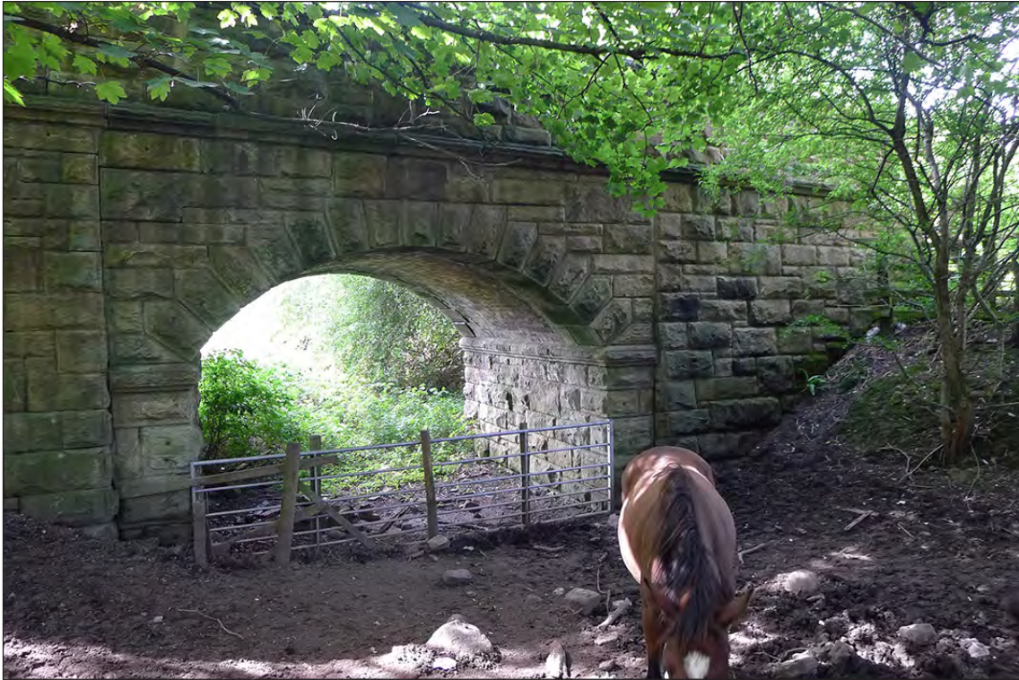
Fig 30. Eastern elevation of railway accommodation bridge BIF/7. (© Historic England/Marcus Jecock)
