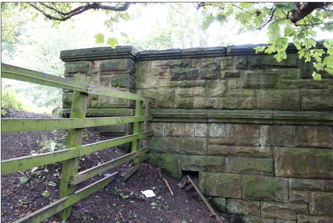
Fig 31. Detail of railway accommodation bridge BIF/7, showing string course, end pier and coping. (© Historic England/Rebecca Pullen)
