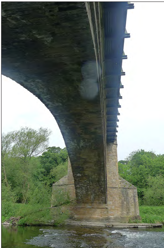
Fig 8. The underside of the southern arch and the central pier of Newton Cap Bridge seen from the south. (© Historic England/Marcus Jecock)
