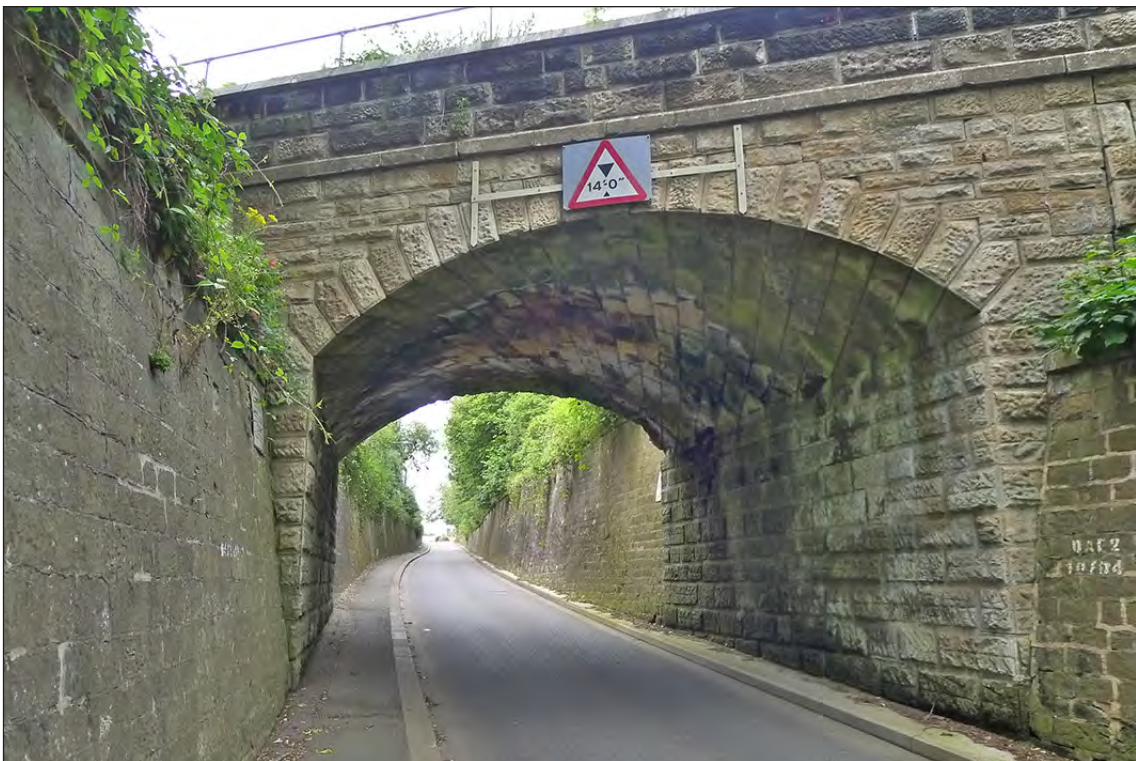
Fig 62. The south-western (downhill) elevation of railway underbridge DAE2/7 (Bone Mill Bank). (© Historic England/Marcus Jecock)
