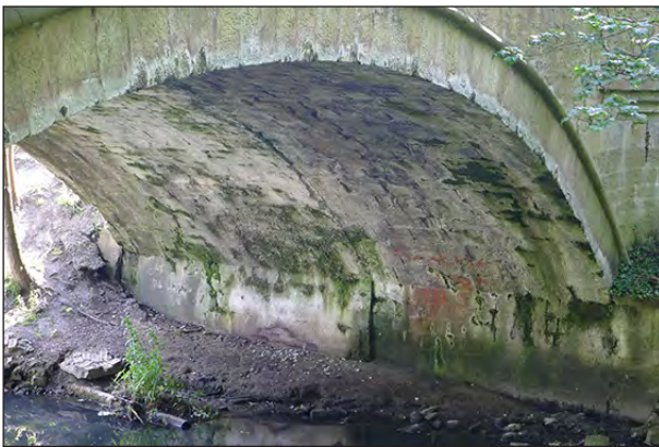
Fig 15. The construction joint visible in the barrel of Gaunless Bridge. (© Historic England/Marcus Jecock)
