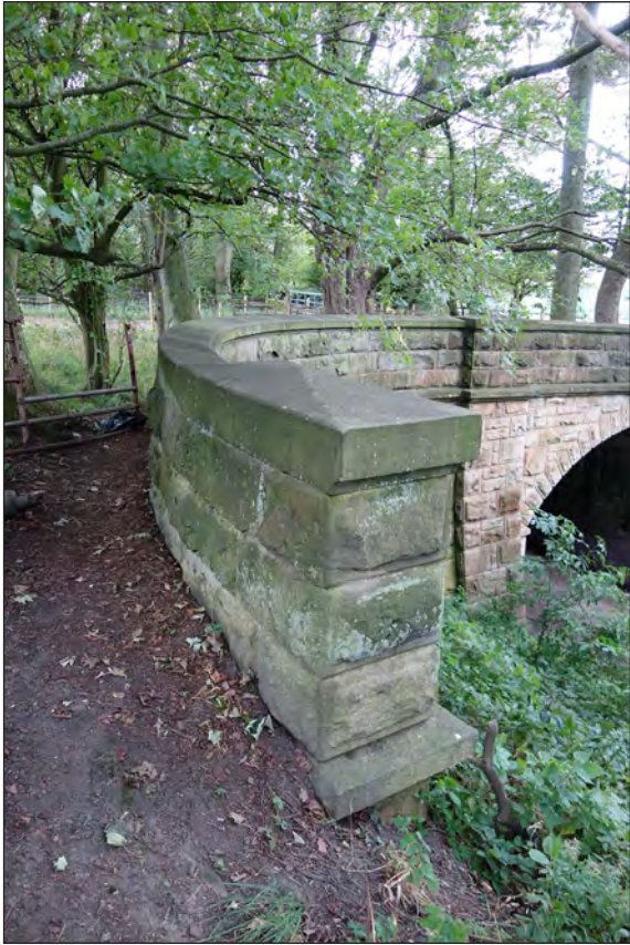
Fig 45. Detail of parapet and curving wing wall to railway accommodation bridge BIF/11 ('Bishop's Bridge'). (© Historic England/Rebecca Pullen)
