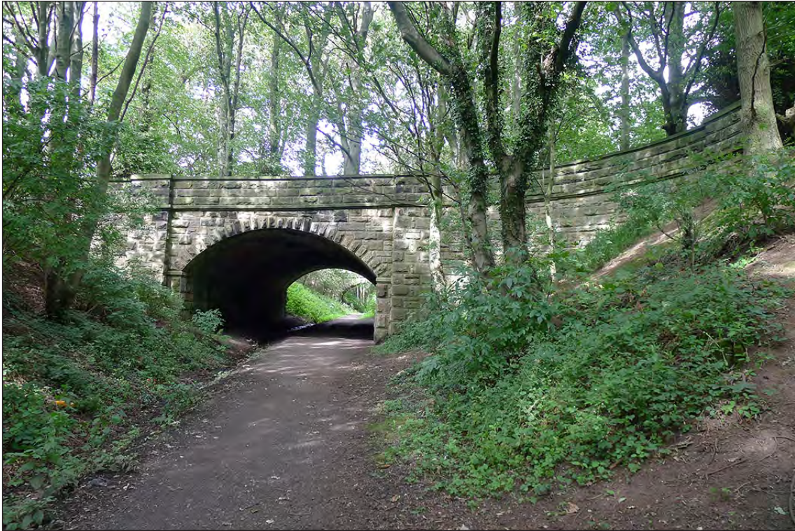
Fig 43. The south elevation of railway accommodation bridge BIF/11 ('Bishop's Bridge'). Note the great width (or length) of the arch barrel. (© Historic England/Marcus Jecock)
