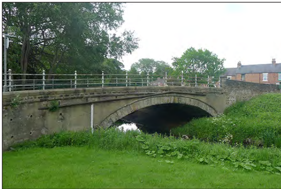
Fig 22. The southern (upstream) elevation of the phase-1 B6282 bridge over the River Gaunless at South Church (© Historic England/Marcus Jecock)
