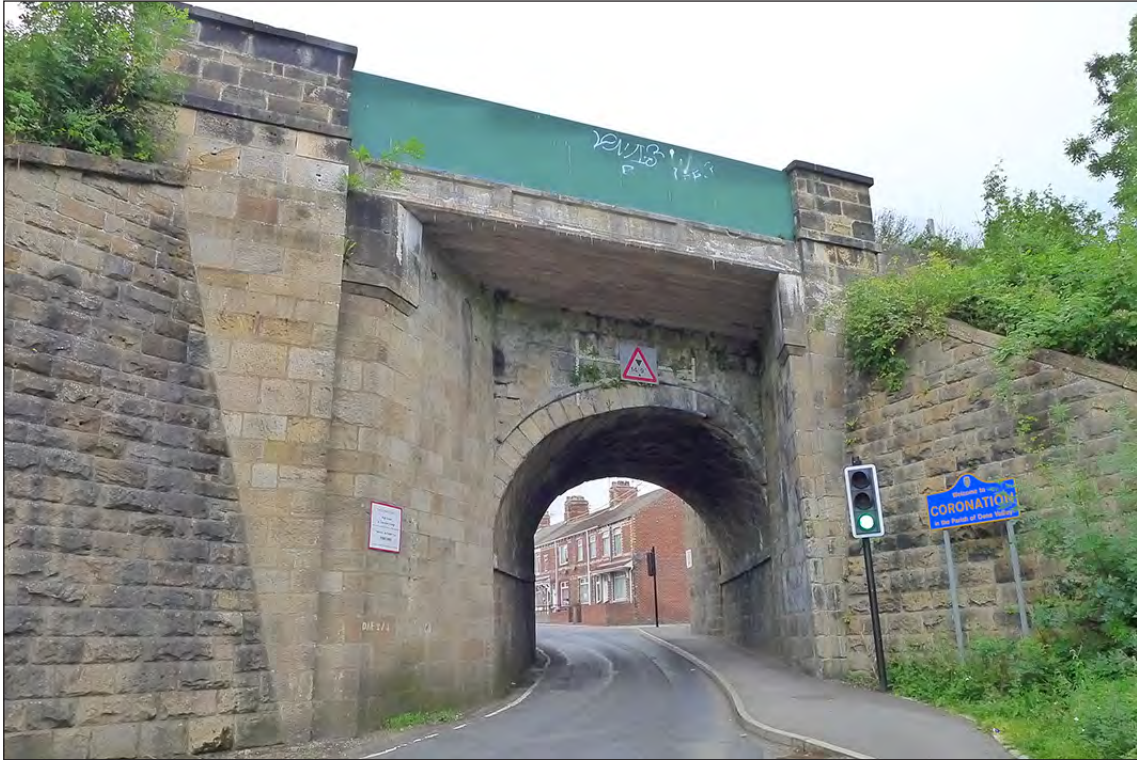
Fig 52. The eastern elevation of railway underbridge DAE2/4 (High St, Coundon Grange), showing the original skew arch and one half of the later widening. (© Historic England/Marcus Jecock)
