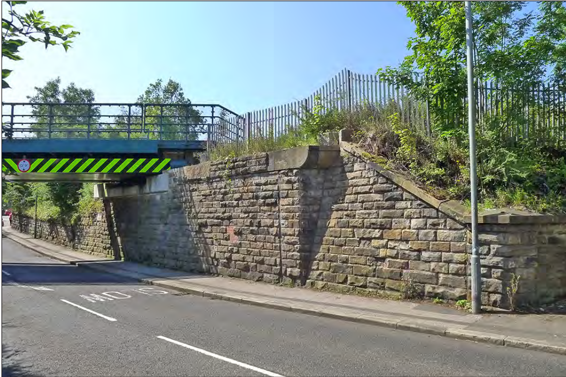
Fig 65. The north elevation of railway underbridge DAE2/9 (South Church Lane). (© Historic England/Marcus Jecock)
