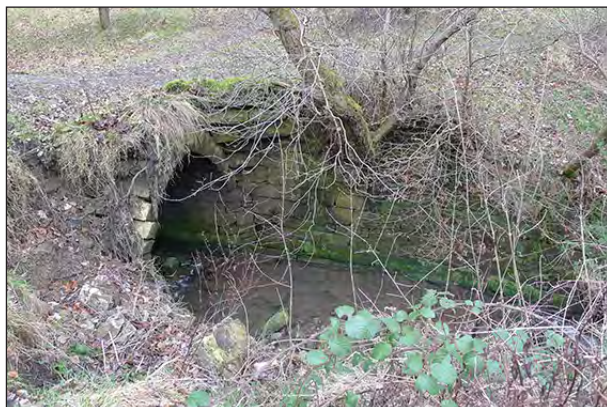
Fig 85. The eastern elevation of 'footbridge no. 1' across the Coundon Burn in Auckland Park. Note the corbelling in the north-east spandrel to ease the passage of the footpath on to the bridge, and the short length of training wall. (© Historic England/Marcus Jecock)
