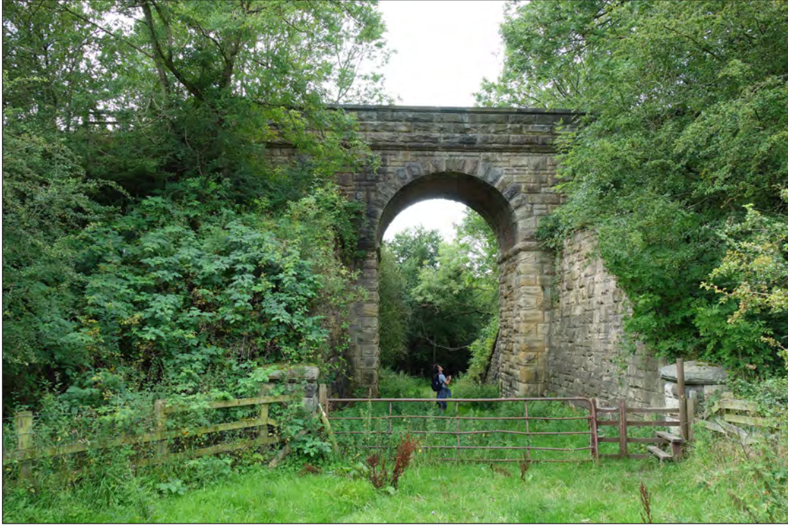
Fig 35. Eastern elevation of railway accommodation bridge BIF/9. (© Historic England/Rebecca Pullen)
