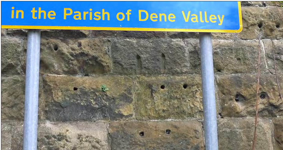
Fig 55. Detail of S&DR stone sleepers re-used in the north-east retaining wall of railway underbridge DAE2/4 (High Street, Coundon Grange). (© Historic England/Marcus Jecock)
