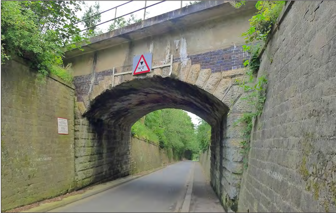
Fig 59. The north-east (uphill) elevation of railway underbridge DAE2/7 (Bone Mill Bank). Note the brick repair to the spandrel and the later concrete parapet. (© Historic England/Marcus Jecock)
