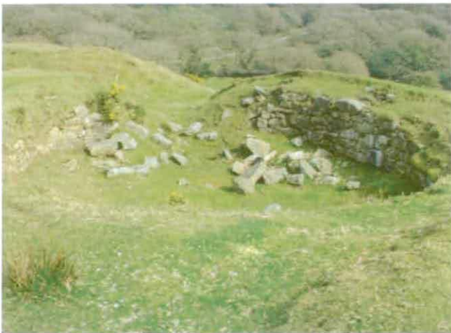
Plate 5. Settling pit (15) with surviving masonry lining.
