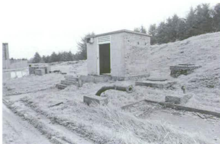
Figure 126 Switch House B2.3 © Crown copyright NMR (AA94/1940)
