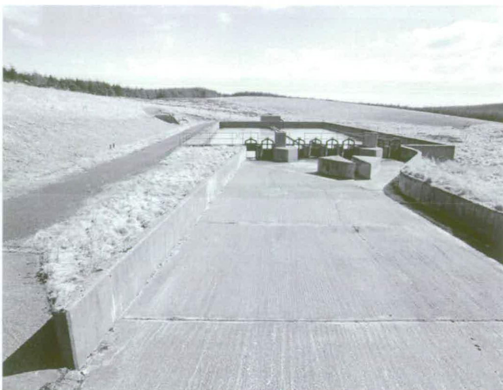
Figure 237 A broad concrete lined spillway extends eastward from Missile Test Stand C3 to an Effluent Lagoon C31.3 © Crown copyright NMR (AA94/2029)
