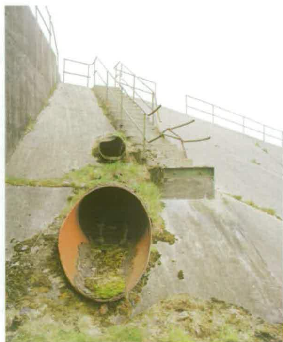
Figure 154 Large bore steel pipes on the east side of Engine Test Stand A2 poured vast quantities of cooling water onto the hot steel deflector bucket to prevent it from melting during test firings © English Heritage NMR (DP003884)
