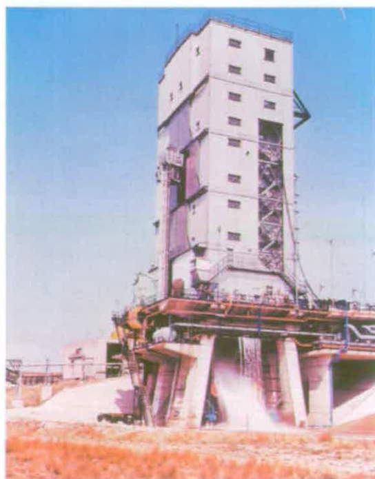
Figure 222 Contemporary photograph of Missile Test Stand C3 showing cooling water pouring from the efflux deflector bucket © Rolls-Royce plc
