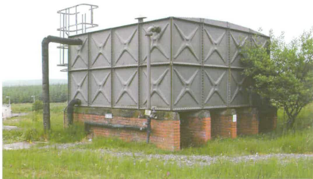
Figure 305 Braithwaite Water Tank containing the domestic supply for the Meteorological Station © English Heritage (AF00134/metstation water)
