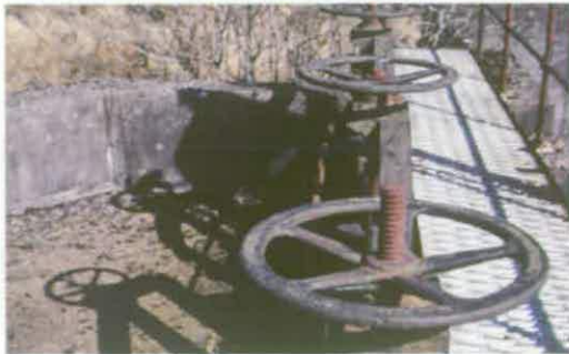
Figure 122 A series of four metal sluice gates controlled the flow of effluent from the main channel into the Settling Tank B6 © English Heritage (AF00134/B6 sluice)
