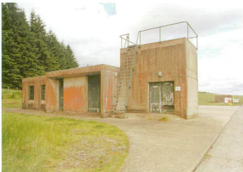
Figure 291 Control Building K1 © English Heritage NMR (DP003988)
