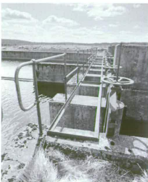
Figure 238 Eight sluice gates at the west end of the Effluent Lagoon controlled the flow of waste water and unspent fuel © Crown copyright NMR (AA94/2032)
