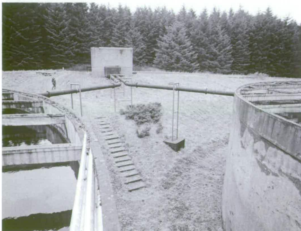
Figure 284 Before entering storage tanks, water from the main Intake Plant Q26 was screened through a Micro Screening Chamber © Crown copyright NMR (AA94/1976)
