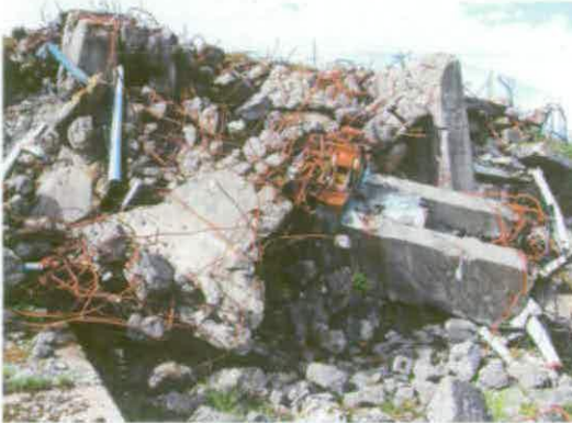
Figure 174 Engine Test Stand A42 was demolished with explosives after being decommissioned © English Heritage (AF00134/A42)
