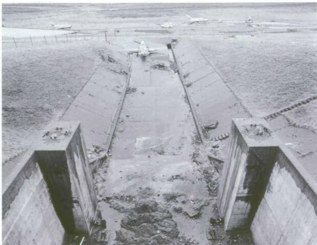
Figure 145 Concrete spillway of Test Stand A1 which channelled cooling water and unspent fuel into drainage conduits to the south © Crown copyright NMR (AA94/1960)
