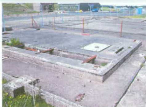
Figure 165 Concrete floor slab of the former Electrical Control Station A17.3 © English Heritage (AF00134/A17.3)
