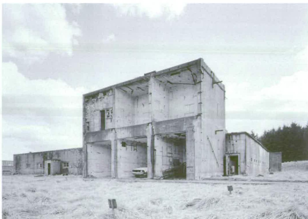
Figure 106 Gas Generator Test Cells B1.4, B1.5 and B1.6 looking south- east. Above these were further cells one of which has been bricked up © Crown copyright NMR (AA94/2943)
