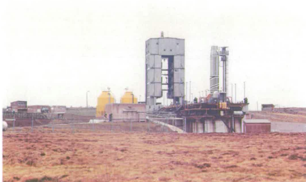
Figure 230 Contemporary photograph of Missile Test Stand C3 showing two large yellow LOX storage tanks to the west of the causeway © Rolls-Royce plc
