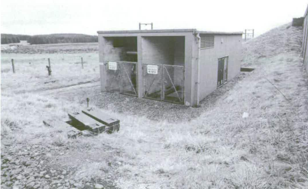
Figure 175 Electricity Sub-station A10.1 © Crown copyright NMR (AA94/1945)
