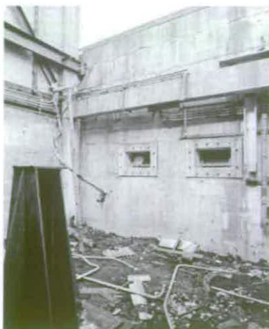
Figure 103 Interior of the derelict Pump Test Cells B1.1 © Crown copyright NMR (AA94/1936)
