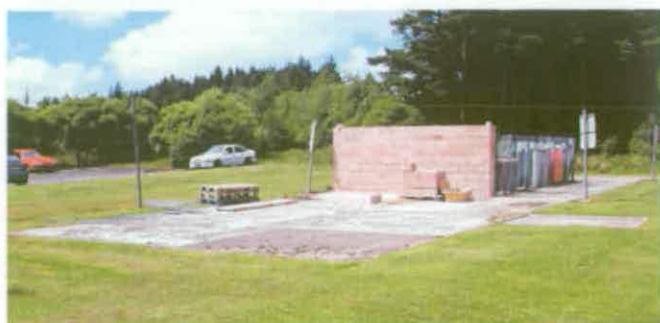
Figure 61 Gas Cylinder Store F111 © English Heritage (AF00134/F111)
