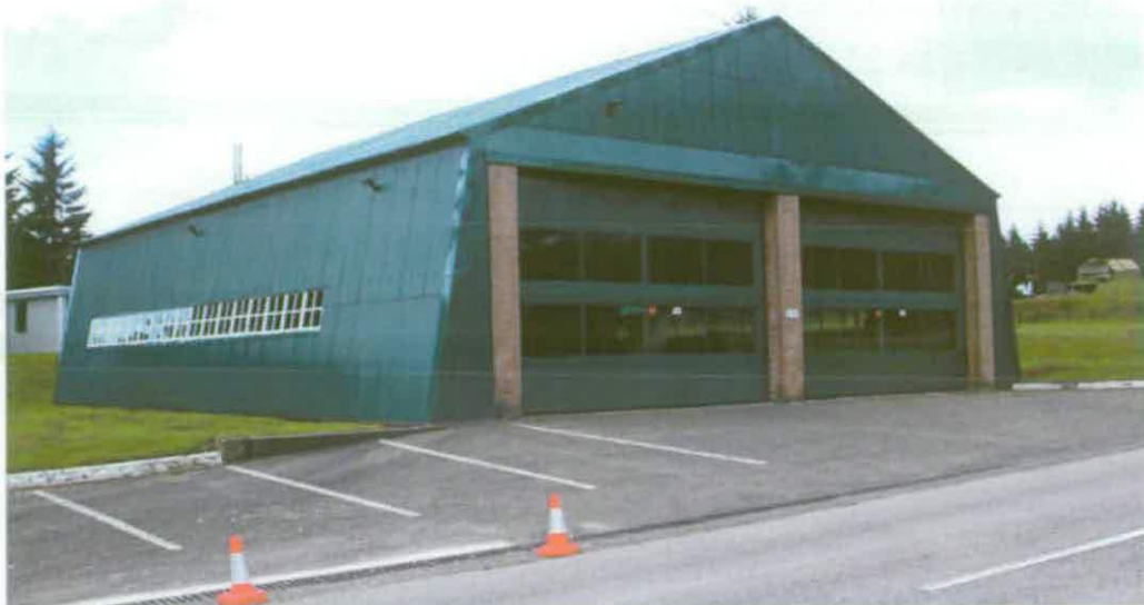
Figure 70 Fire Station Q2.19 © English Heritage (AF00134/Q2.19)
