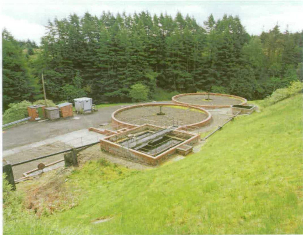
Figure 32 Sewage Plant © English Heritage NMR (DP003933)
