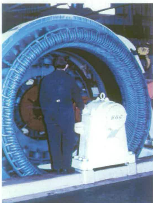
Figure 82 Compressor housed in building D1 © Rolls-Royce plc
