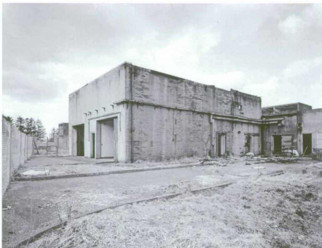
Figure 102 Pump Test House B1.1 comprised two brick test cells - one for kerosene pump callibration and the other for liquid oxygen pumps © Crown copyright NMR (AA94/2941)
