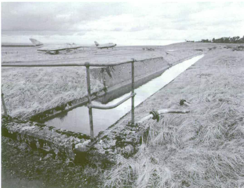
Figure 200 A concrete lined drain that flanks the south side of the test stands carried cooling water and unspent fuel to an Effluent Lagoon A14 © Crown copyright NMR (AA94/1968)
