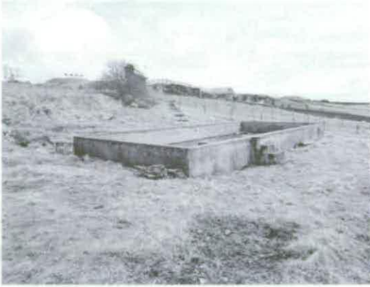
Figure 173 Kerosene Dump Tank to the west of Engine Test Stand A42 © Crown copyright NMR (AA94/2930)
