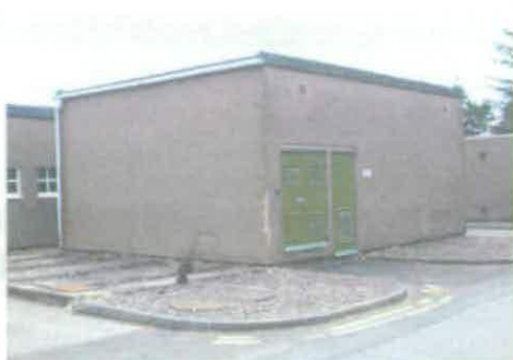
Figure 47 Sub-station F42.2 © English Heritage (AF00134/F42.2)
