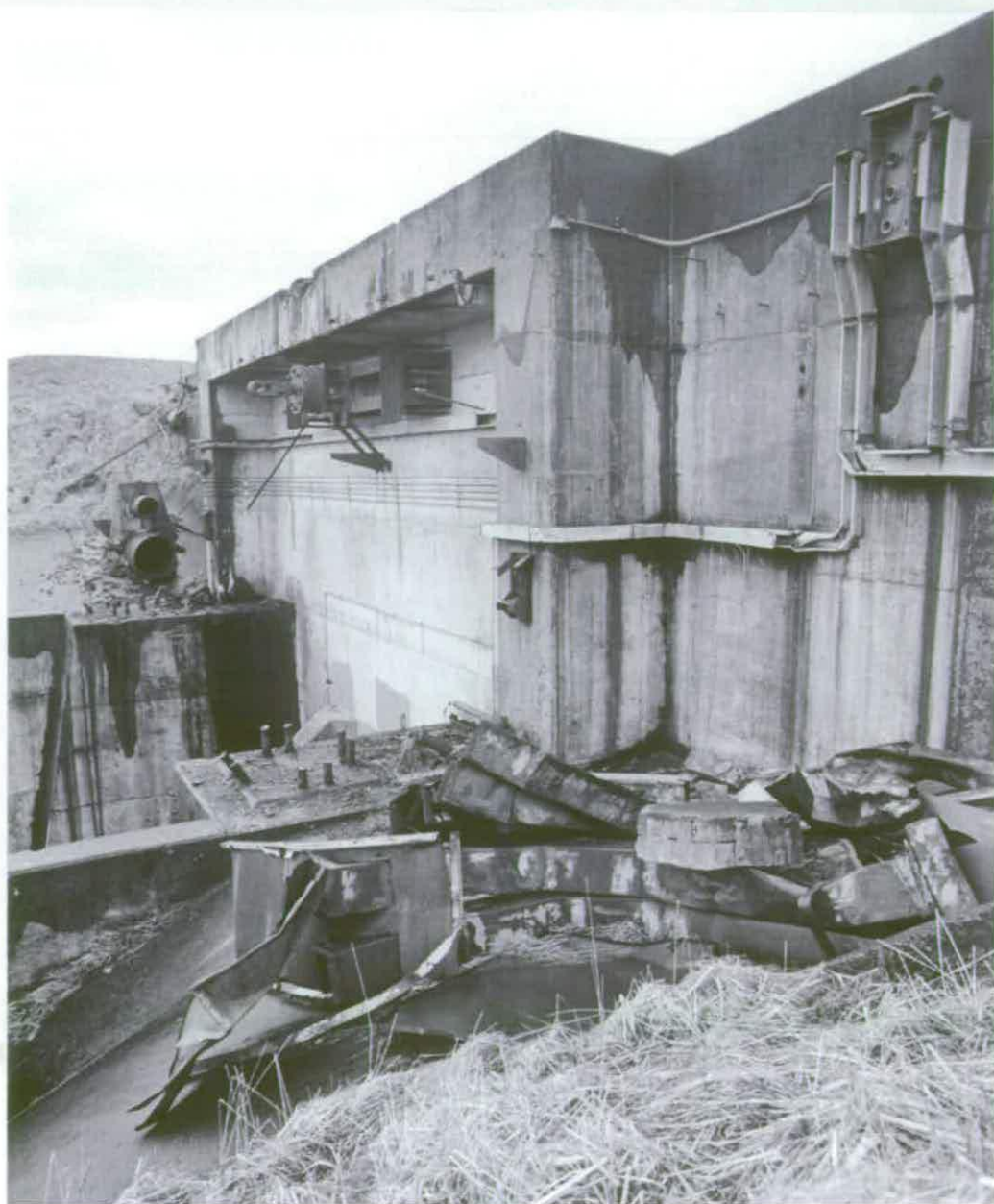
Figure 139 Rear wall of Engine Test Stand A1 with a gimballed mounting for the efflux deflector still in place © Crown copyright NMR (AA94/1957)
