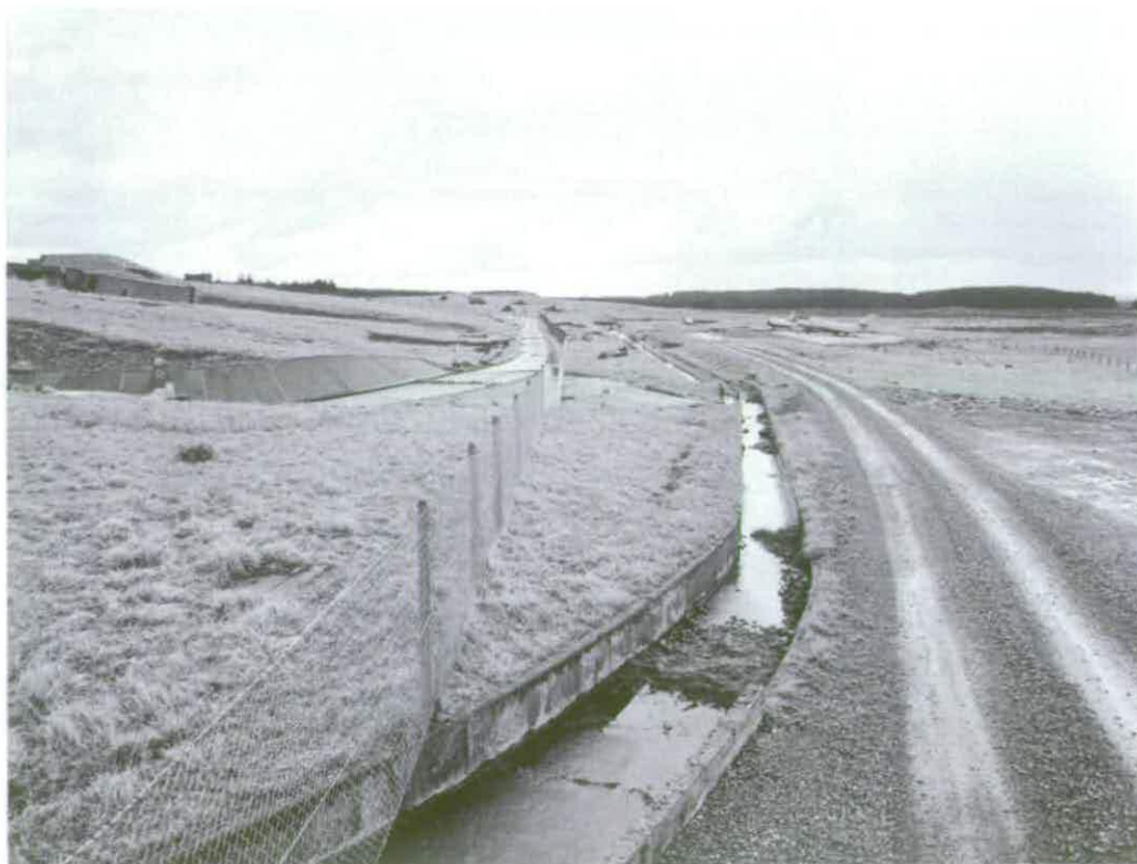
Figure 172 Cooling water and inspent fuel from Engine Test Stand A42 drained into a channel that flanked the south side of the test stands © Crown copyright NMR (AA94/2929)
