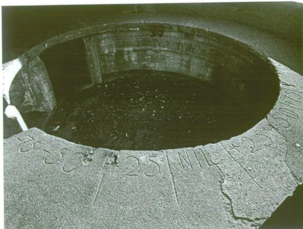
Figure 15 Photograph showing detail of the gun quadrant arcs for the southern 6-inch Mark VII gun (NMR: BB97/5388)
