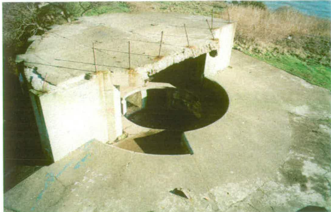
Figure 13 Photograph showing the southern 6-inch Mark VII gun emplacement with Second World War casemate over
