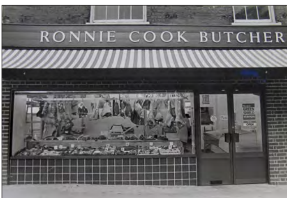
Figure 34. 41 High Street as seen on the 10 th March 1976 – a typical post-war butcher's shop with large plate-glass display window and a tiled stallriser. SROL: 1176/1/13/7/3/13. Reproduced by kind permission of the Lowestoft Journal
