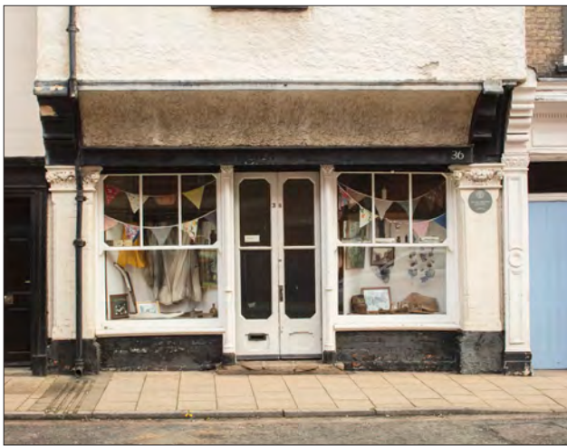
Figure 28. 36 High Street. A late 19 th -century shopfront with cast-iron columns set below the jetty of a 15 th -century house. © Historic England DP247553
