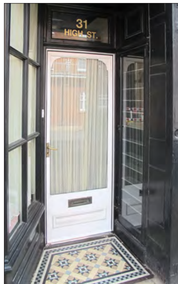
Figure 25. Late 19 th -century encaustic tiles and a shallow display case within the lobby of 31 High Street. © Historic England, Katie Carmichael
