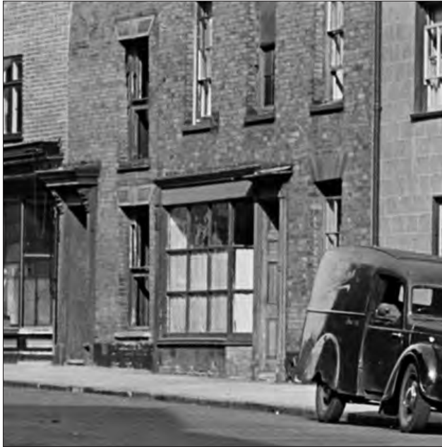
Figure 27. 33 High Street in 1949, showing a lost shopfront of c.1840. © Historic England bb50/00217 (detail)
