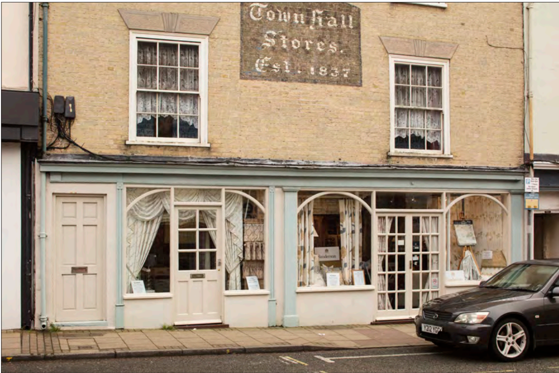
Figure 36. 43-44 High Street, a modern shopfront of c.2003 in a traditional style. © Historic England DP247561
