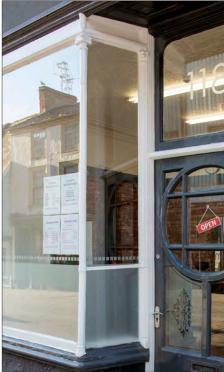
Figure 122. 118 High Street – slender timber colonettes with Ionic capitals are a typical feature of Edwardian shopfront design. © Historic England DP236888
