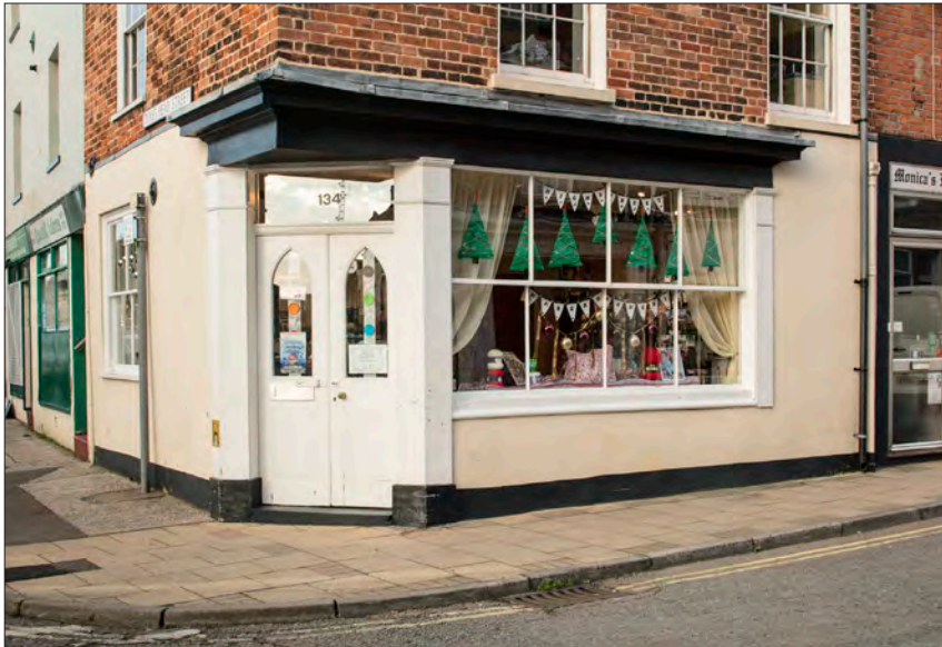
Figure 141. 134 High Street retains a typical late 19 th -century sash window (with later repairs) for the sale of consumable goods. © Historic England DP236909
