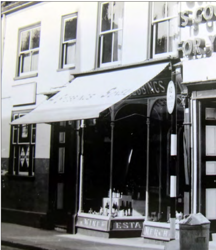
Figure 158. 149 High Street, c.1960. Now hidden, it is possible that the surviving fascia and stallboard retain the 'brilliant' lettering seen here. Reproduced by kind permission of Suffolk Record Office, ref SROL: 1504/1/4/2 (detail)
