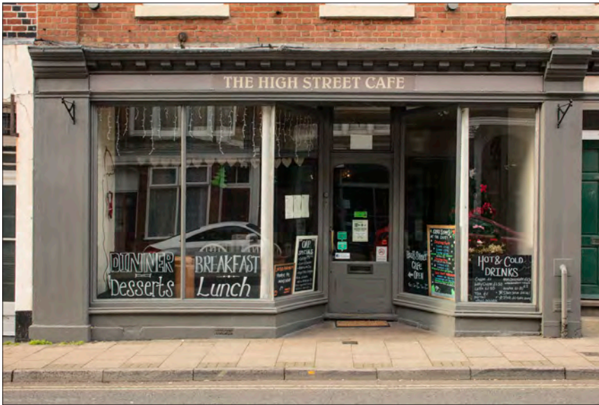
Figure 145 138 High Street – a typical shopfront of c.1900 with later modifications. © Historic England DP236913
