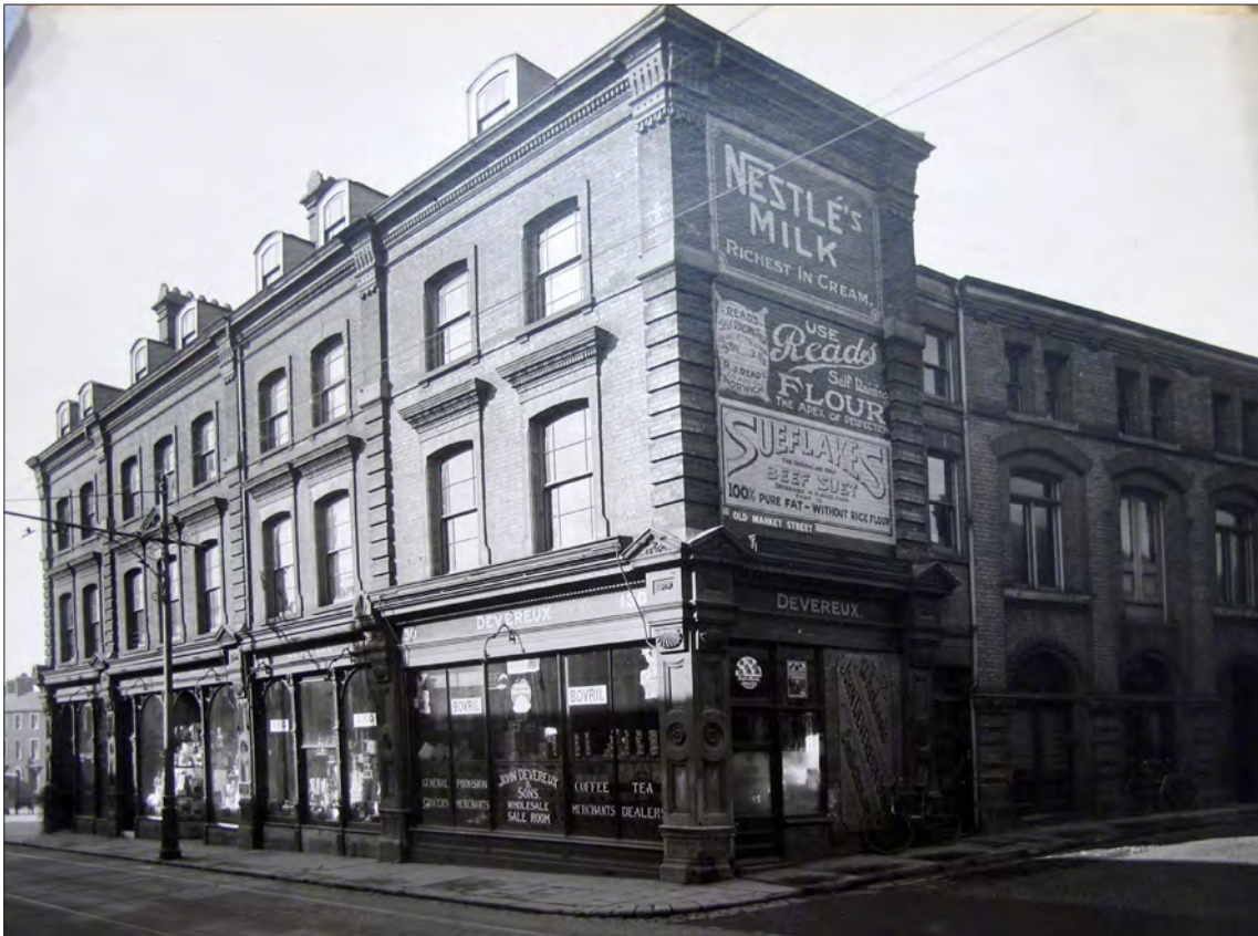
Figure 130. Devereux's store was built in at least two phases, the two styles of shopfront clearly visible in this undated photograph. Reproduced by kind permission of Suffolk Record Office, ref SROL: 598/7/23
