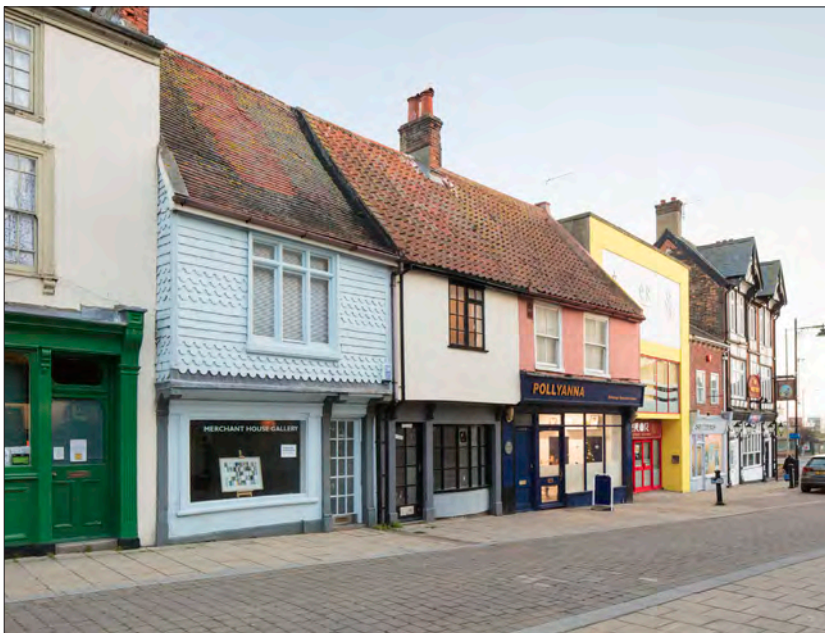
Figure 106. 102-107 High Street. The shopfronts of 102, 103 and 104 are set beneath the jetty of a 16 th -century building. © Historic England DP236875
