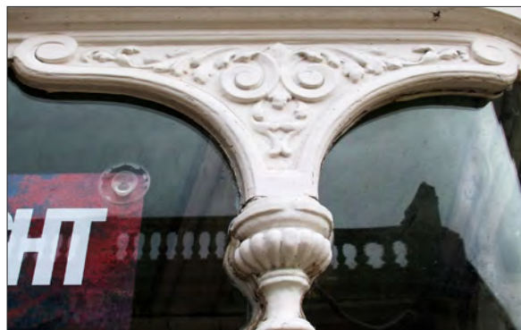
Figure 16 (below). A carved timber spandrel and delicate colonette with decorative capital at 2 Sheepgate, Beccles. © Historic England, Katie Carmichael
