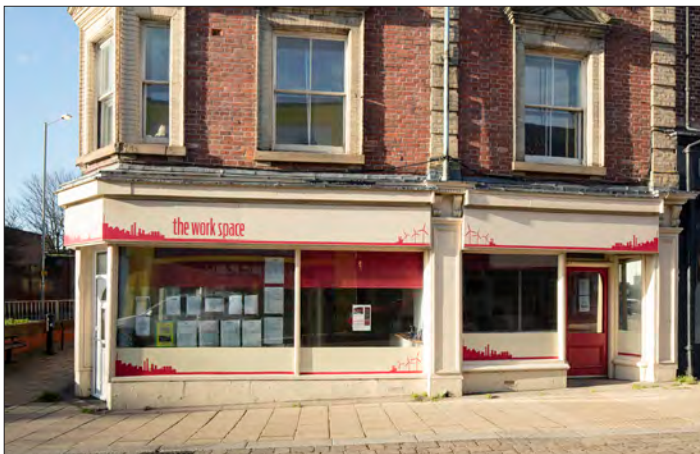
Figure 111. 113-114 High Street, a c.1900 shopfront with later alterations. © Historic England DP236880
