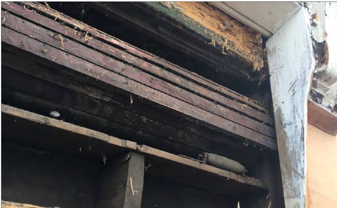
Figure 172. A wooden roller shutter was uncovered at 17 Station Square, Lowestoft, in spring 2019 and may be similar to those just visible at 36 High Street. © Private Collection
