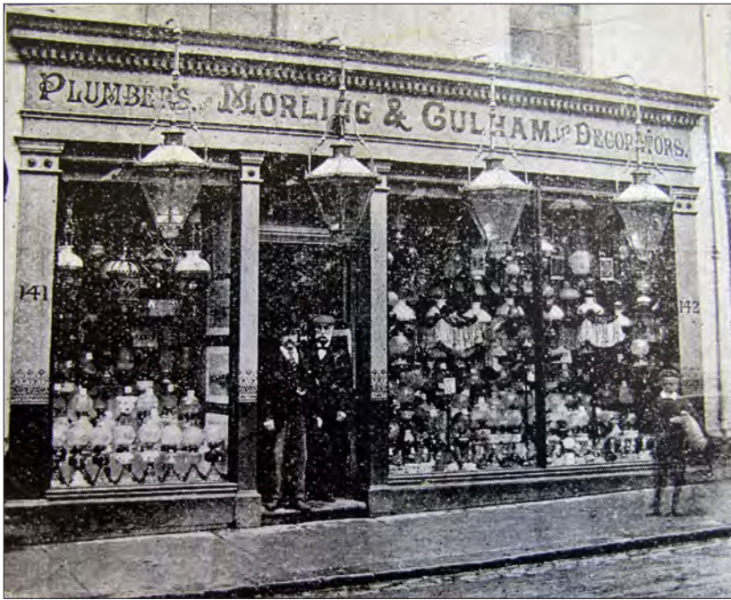
Figure 150. 141 High Street as seen in c.1900 when it had an eye-catching shopfront complete with gas lanterns. Reproduced by kind permission of Suffolk Record Office, ref SROL: 1300/72/46/6
