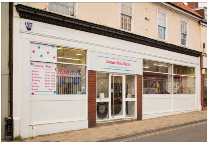
Figure 149. 141-142 High Street, a plain modern frontage beneath a dentilled cornice. © Historic England DP236917
