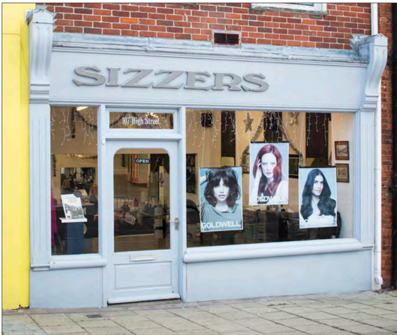
Figure 108. 107 High Street – a mid-20 th -century (or later) shopfront in a traditional style. © Historic England DP236878
