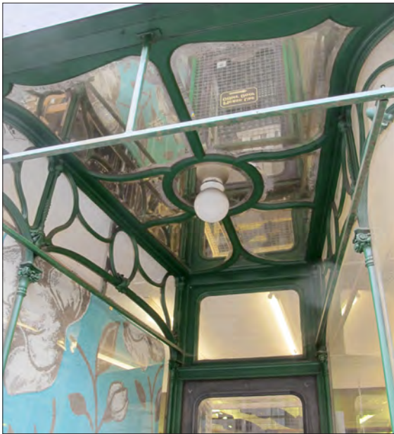
Figure 6. A mirrored soffit at 10-11 Regent Street, Great Yarmouth, Norfolk. © Historic England, Katie Carmichael
