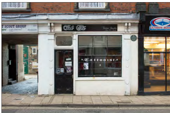
Figure 64. 64 High Street, which retains a typical example of a wide sash window for the sale of perishable goods. © Historic England DP236852
