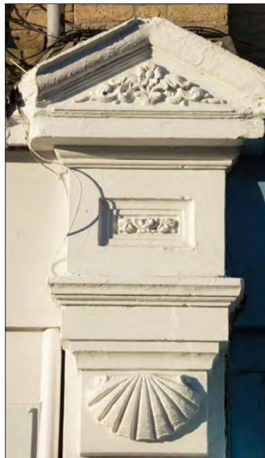
Figure 132. Delicately carved triangular pediments to the consoles at 128 and 130 High Street. © Historic England DP236895
