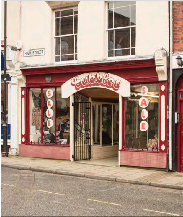
Figure 41. 47 High Street is unusual in having a largely post-war 'arcaded' lobby, although it may have 19th-century origins. © Historic England DP247564
