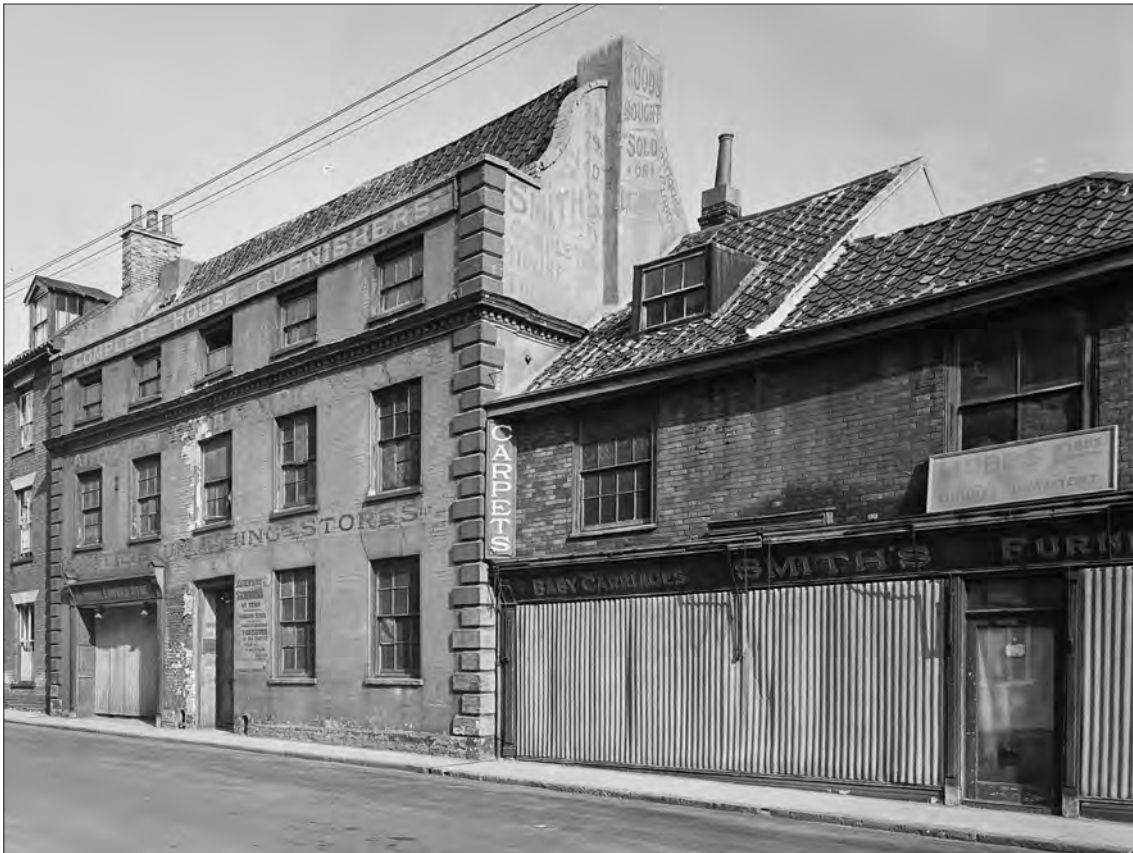
Figure 32. The former Smith's Furnishing Stores at 38-40 High Street – demolished in 1957, pictured in 1949. © Historic England bb50/00217 (detail)
