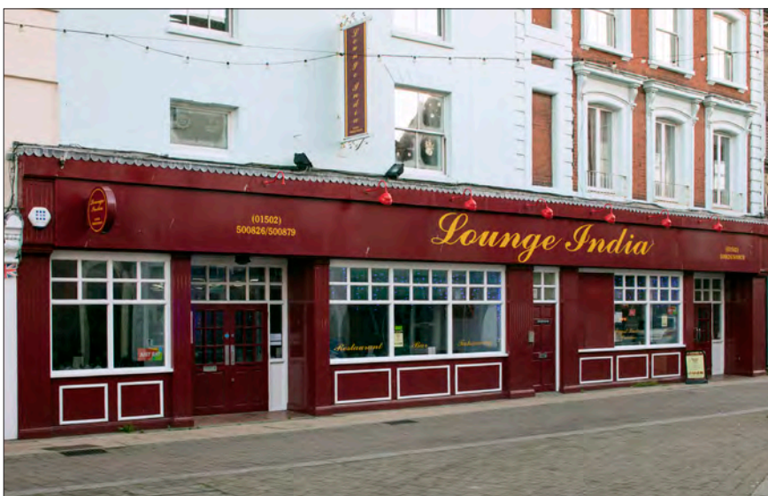
Figure 96. 95-98 High Street. The current frontage spans three buildings and dates to c.1998. © Historic England DP236869
