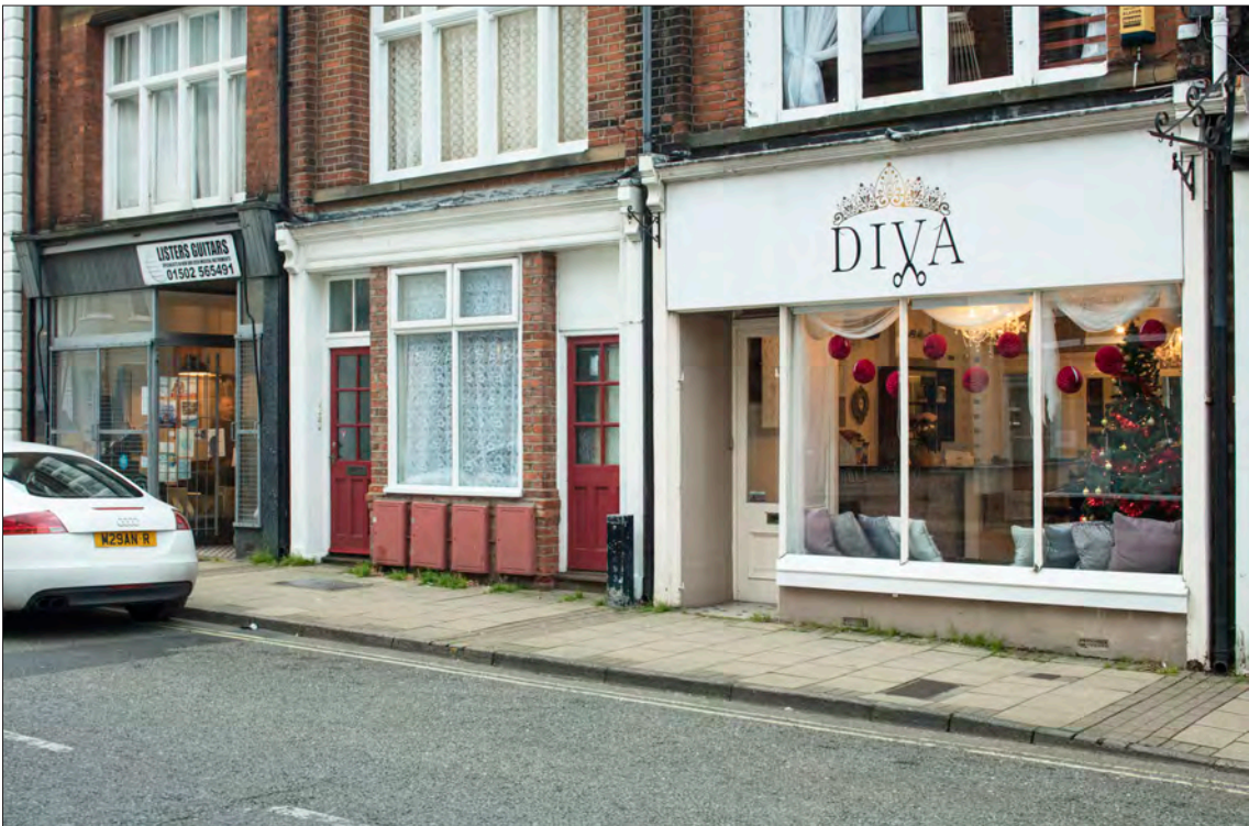
Figure 60. 64, 65 and 66 High Street – built as a single development, though the shopfront of 65 has been entirely removed. © Historic England DP236851
