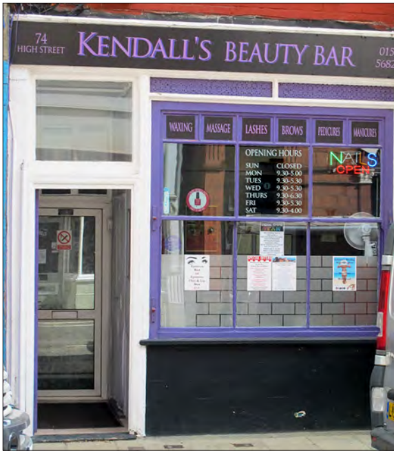
Figure 76. 74 High Street retains a typical example of a shop window designed for the sale of consumable goods, with a wide sash window and a decorative ventilator strip above. © Historic England, Katie Carmichael
