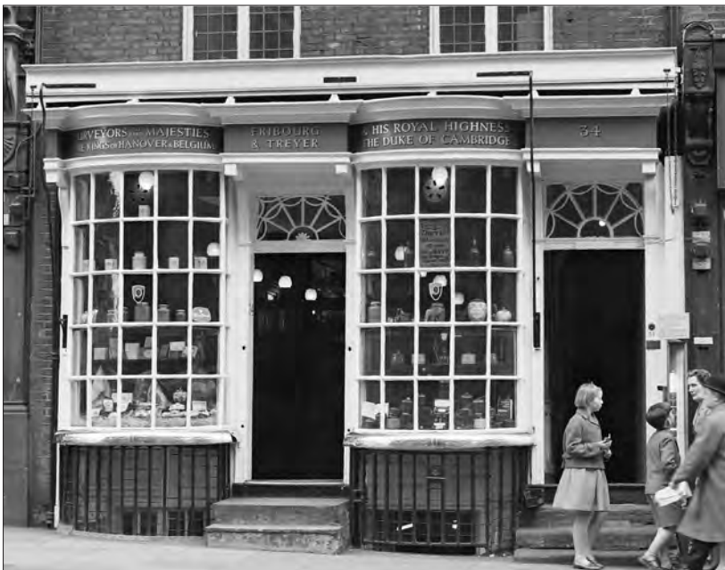
Figure 14. 34 Haymarket, London. Occupied from 1754 until 1982 by the tobacconists Fribourg and Treyer, it is a good example of a mid-18th-century double-bow shopfront. © Historic England AA60/02974 (detail)
