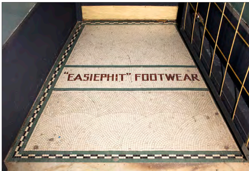
Figure 10. The lobby of 115 High Street, showing the mosaic floor of c.1930. The small holes in the foreground show where a shop gate was fitted out of hours. © Historic England DP236883
