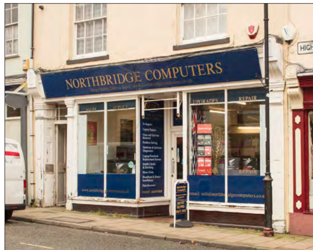
Figure 40. 46 High Street retains a largely unaltered c.1900 shopfront with thin, deep, astragal-moulded glazing bars. © Historic England DP247563
