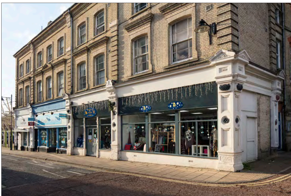
Figure 129. 127-130 High Street, built in c.1869 and extended c.1890. Constructed for the grocery and provisions merchant John Devereux, with a shop to the High Street and extensive warehouses behind. © Historic England DP236901
