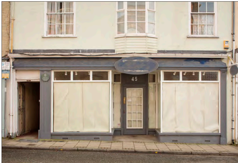
Figure 39. 45 High Street – 20 th -century glazing within an early Victorian frame with unusual scooped ends to the fascia. © Historic England, DP247562
