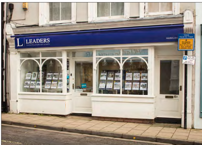
Figure 80. 81 High Street – modern 'traditional' display windows and doorways are set within an apparently older framework. © Historic England DP247579
