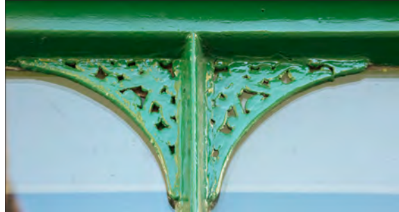
Figure 105. Decorative pierced spandrels at 101 High Street, a feature which may well have been seen on local shopfronts of a similar date. © Historic England DP236874
