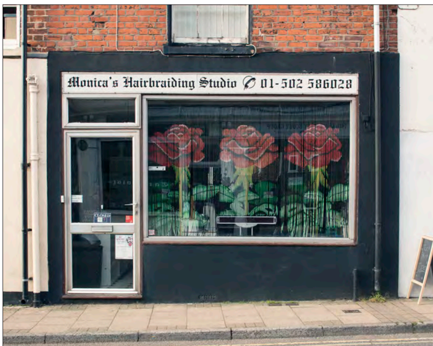
Figure 142. 135 High Street – the simplicity of design and the use of aluminium is typical of the 1970s. © Historic England DP236911
