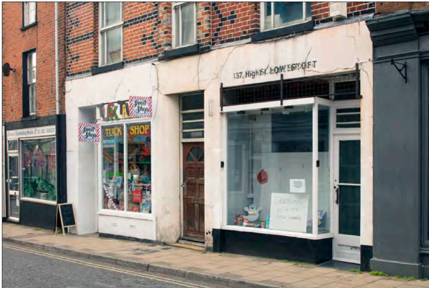
Figure 143. 136 and 137 High Street. The use of shallow, truncated display cases is unusual and suggests an inter-war date. © Historic England DP236912
