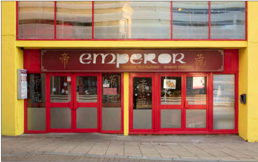
Figure 107. 105-106 High Street, a post-war building with typically minimal detail. © Historic England DP236877
