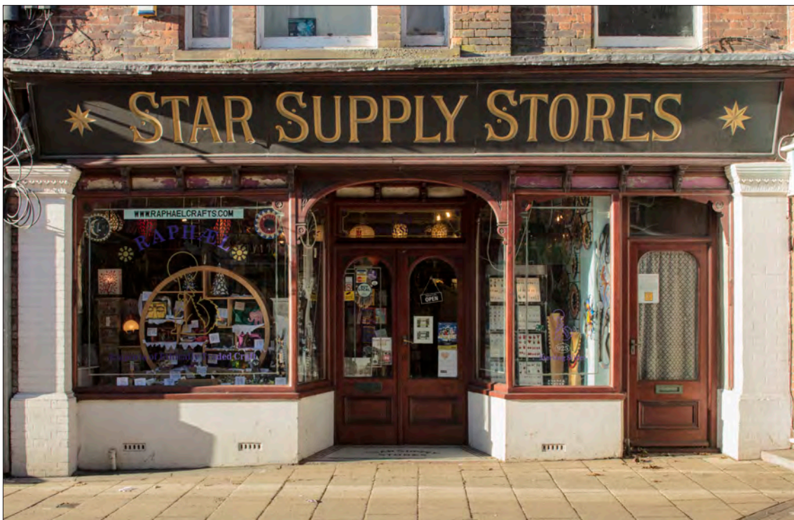
Figure 123. 119 High Street. The Star Tea Company has a complicated history in Lowestoft, and this shopfront appears to date from c.1934. © Historic England DP236889
