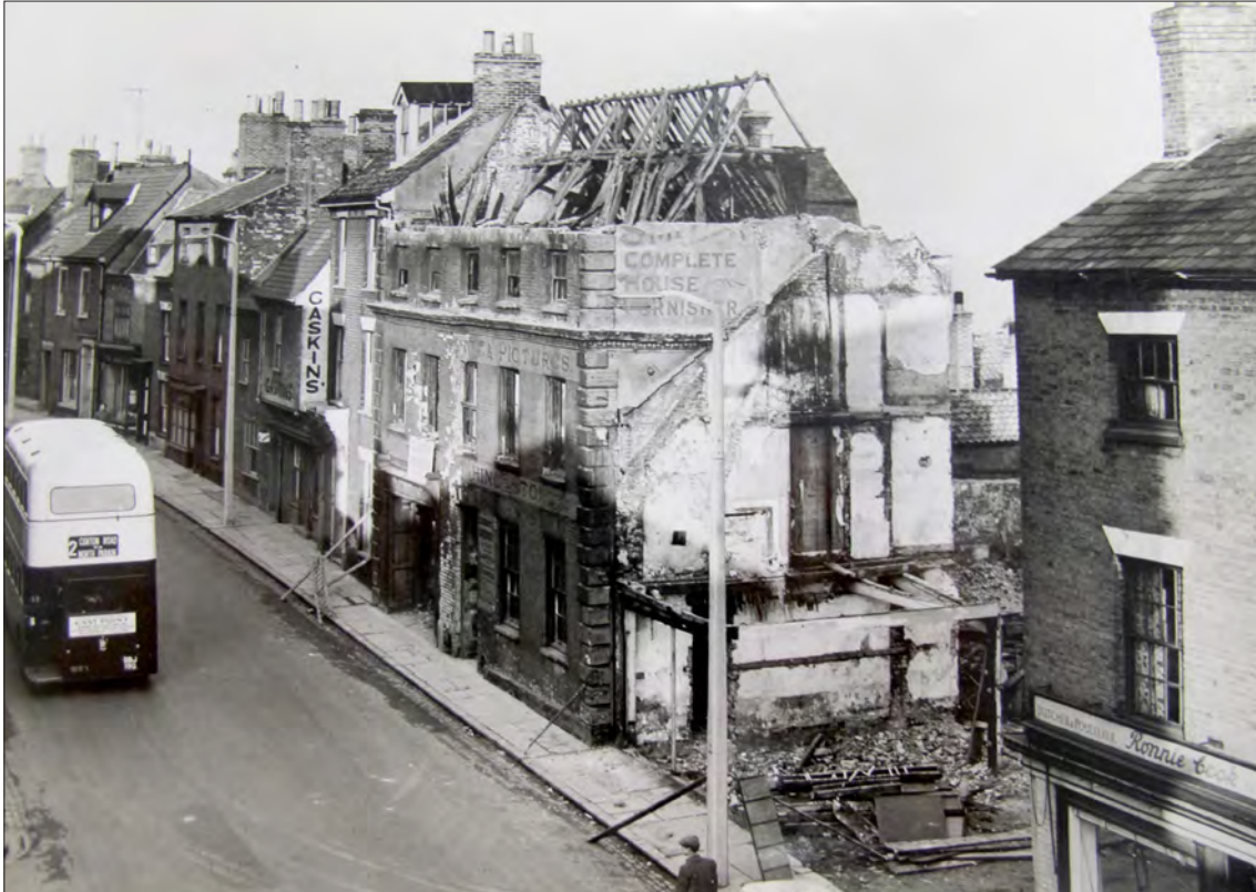
Figure 13. The demolition in 1957 of 38 High Street, a distinctive three-storey 18th-century building. Reproduced by kind permission of Suffolk Record Office, ref SROL: 1300/72/41/34
