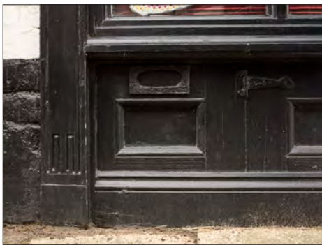
Figure 24 (above). Victorian panelling and letterbox below the shop window of 31 High Street. The stylised Greek key design to the base of the narrow pilasters suggests a date of c.1840. © Historic England, DP247551
