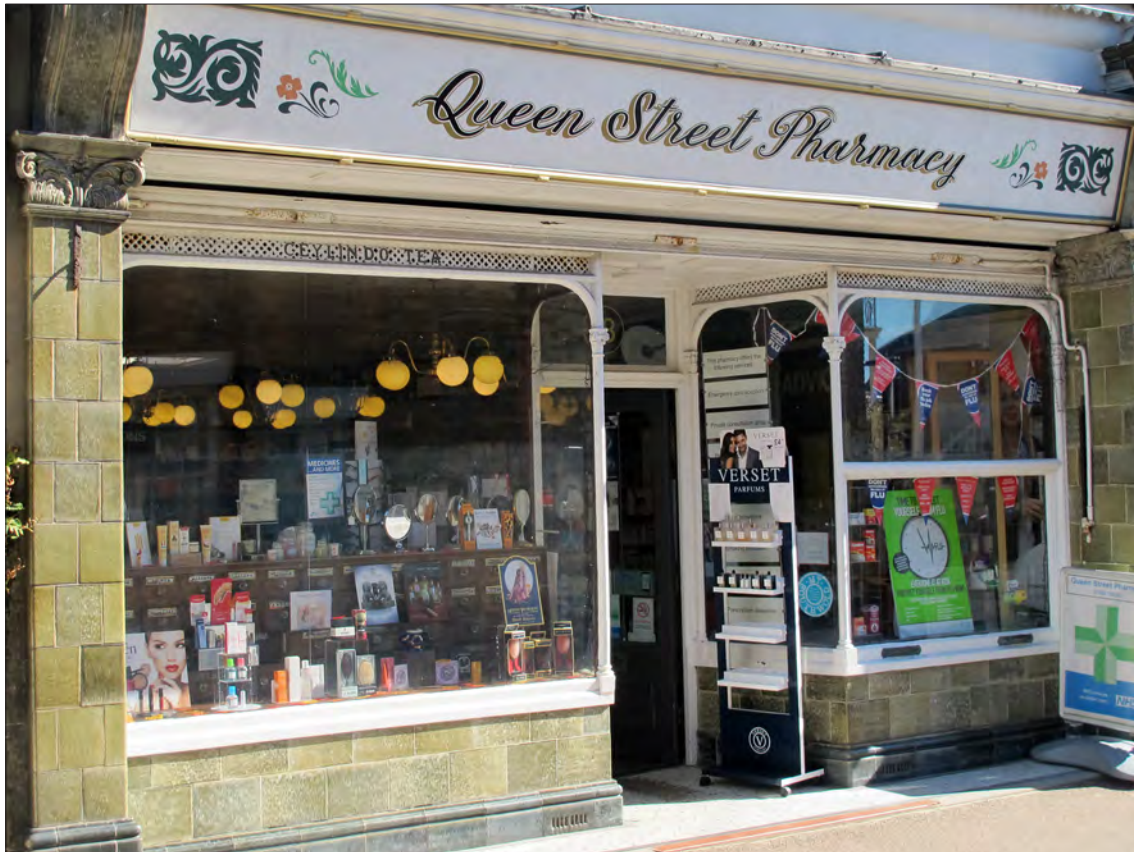
Figure 11. A former International Tea Company shopfront at 18 Queen Street, Southwold, Suffolk. The layout of a sash window to one side of the entrance and fixed glazing to the other was a particular feature of chain grocers' stores. © Historic England, Katie Carmichael
