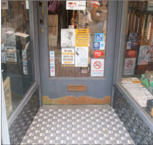
Figure 61. The lobby of 64 High Street, with polished grey granite stallrisers, geometric floor tiles and brass fittings on the door suggesting an inter-war date. © Historic England, Katie Carmichael
