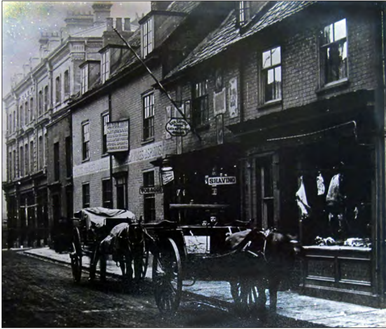
Figure 135. An undated photograph of c.1890 shows the buildings previously on the site of 131-133A High Street. Reproduced by kind permission of Suffolk Record Office, ref SROL: 1828/3/1/15
