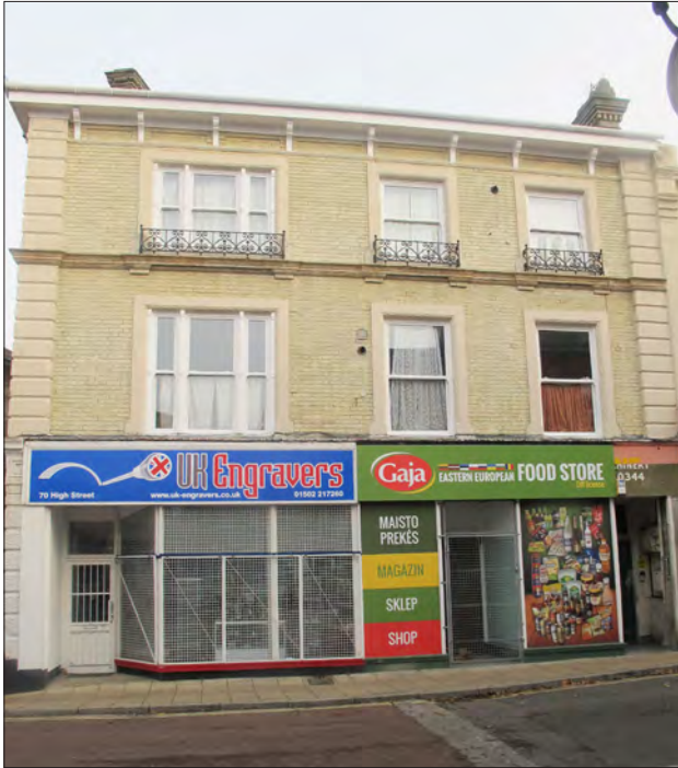
Figure 68. 70-71 High Street, divided into two units; the shop on the right retains an inter-war lobby. © Historic England, Katie Carmichael
