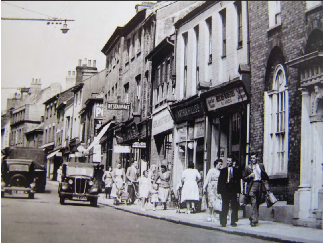
Figure 51. An undated photograph from the 1960s shows both 53 High Street (centre, flat white fascia) during renovation work and 54 High Street when it was still divided into two shops. Reproduced by kind permission of Suffolk Record Office, ref SROL: 1504/1/4/1
