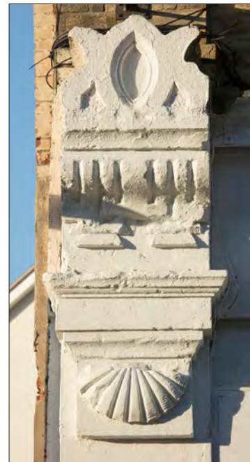
Figure 133. Shaped consoles at 127-129 High Street mark the extent of Devereux's original c.1869 shopfront. © Historic England DP236894
