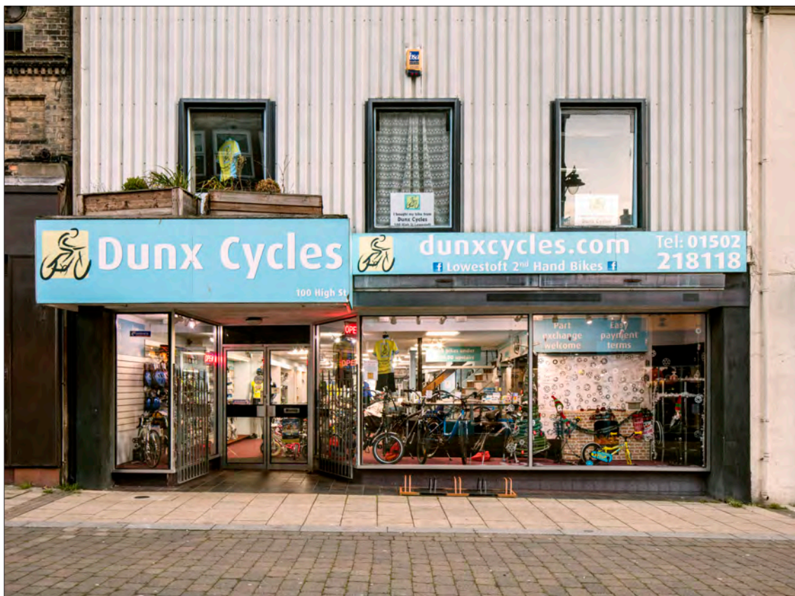
Figure 103. 100 High Street has a typical post-war shopfront, with aluminium-framed display windows and salient surrounds to the first-floor windows. © Historic England DP236872
