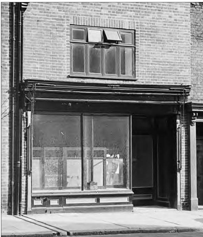
Figure 23. A photograph of 31 High Street taken in 1949, showing a late 19 th -century plate-glass window with 20 th -century brickwork above. © Historic England bb50/00216 (detail)
