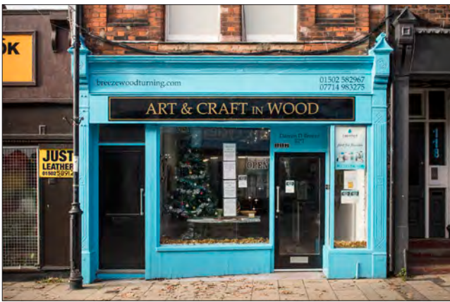
Figure 119. The present shopfront of 117 High Street is a post-war design with asymmetrically splayed lobby and simple plate-glass windows set within the decorative framework of the 1870s. © Historic England DP236885
