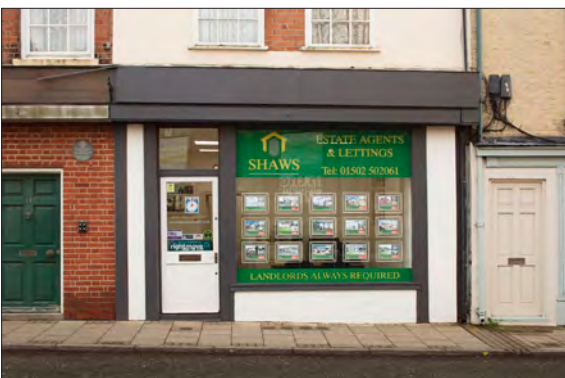
Figure 35. 42 High Street, another plain post-war shopfront lacking details such as pilasters, a cornice or consoles. © Historic England DP247560
