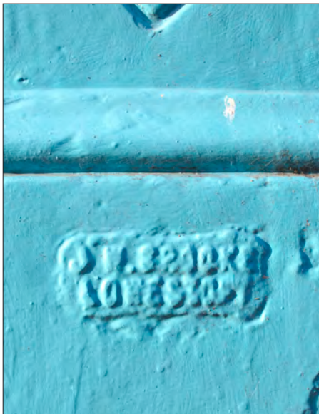
Figure 120. Plaques reading 'JW BROOKE LOWESTOFT' are affixed to the base of both pilasters at 117 High Street, for reasons unknown. © Historic England DP236886
