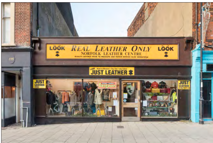
Figure 115. 116 High Street – a modern shopfront with ‘traditional’ style details including dentils. © Historic England DP236884
