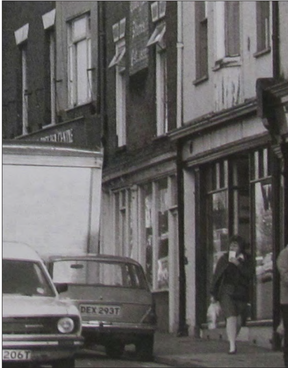
Figure 38. 43-44 High Street, 26th November 1982. All traces of the former early Victorian shopfront were removed and replaced by plain plate-glass windows in c1978. SROL: 1176/1/14/3/11/54 (detail). Reproduced by kind permission of the Lowestoft Journal
