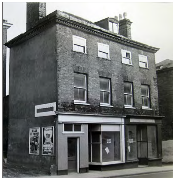
Figure 46. Former shopfronts at 50 High Street, as seen on 28 th April 1978. SROL: 1176/1/13/9/4/18 (detail). Reproduced by kind permission of the Lowestoft Journal
