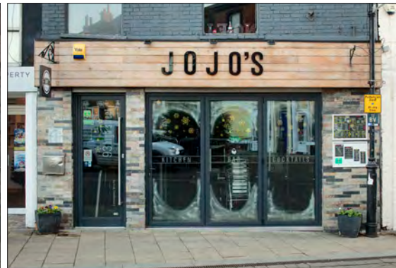
Figure 94. 93 High Street, any former shopfront has been replaced by modern folding doors. © Historic England DP236865
