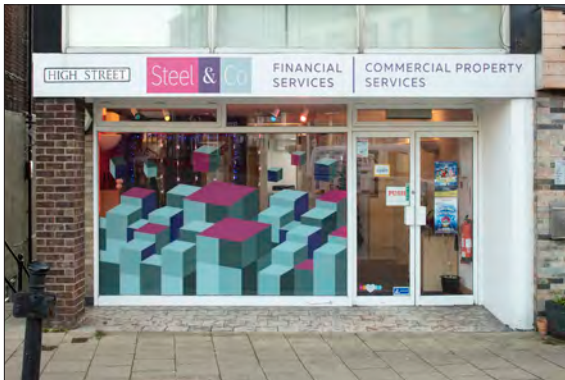
Figure 93. 92 High Street – a post-war commercial property with a large plate-glass window. © Historic England DP236864
