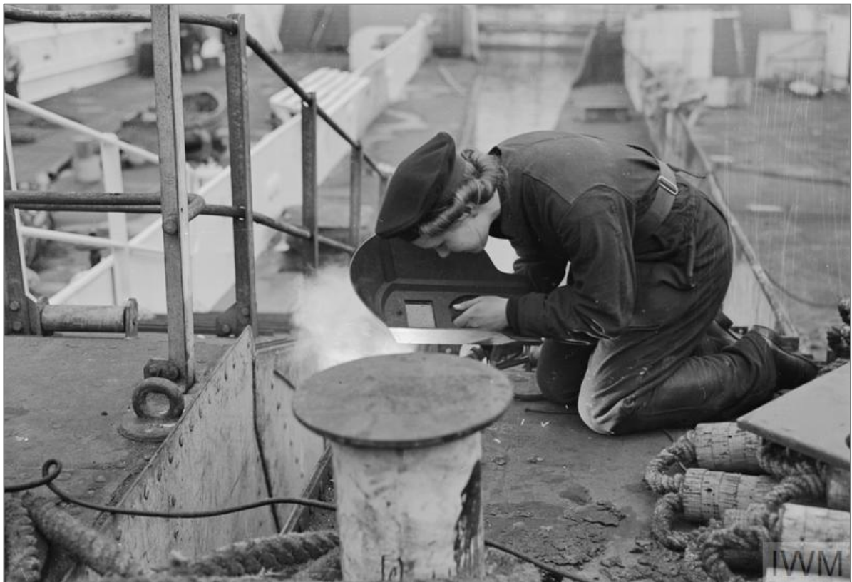
Figure 27: WRNS ship mechanic welding on the deck of a Landing Craft. The location is not specified. © IWM D 18163.
