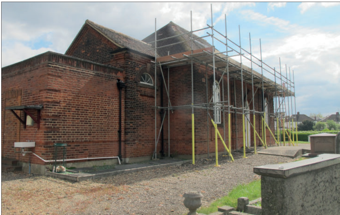
Figure 241: Rear (south-west) view, with the two-part extension in the foreground
