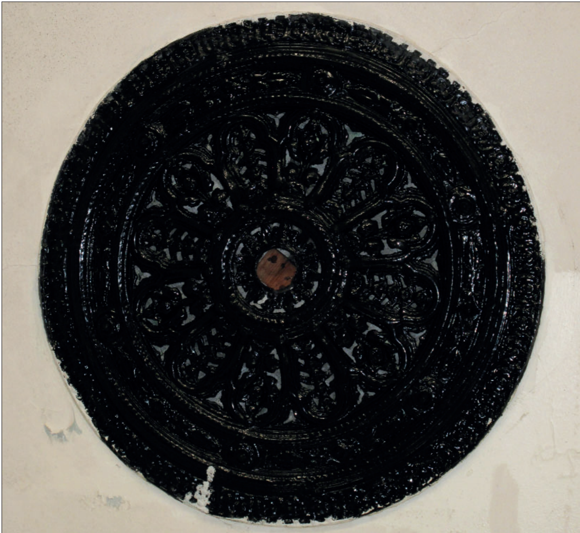
Figure 301: One of two decorative iron ceiling roundels
