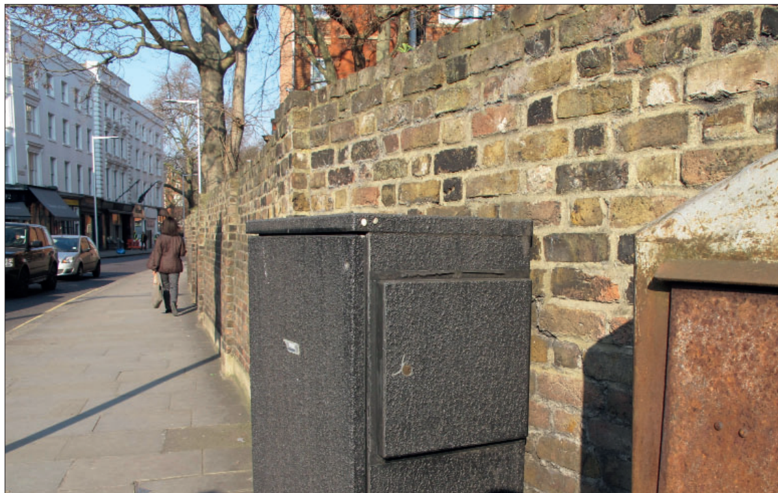
Figure 181: The boundary wall on Fulham Road
