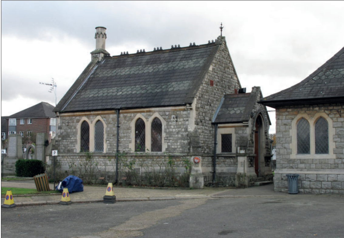
Figure 277: Cohanim room from the north-west
