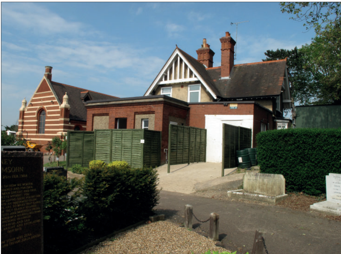
Figure 194: Entrance lodge rear view, mortuary to the right
