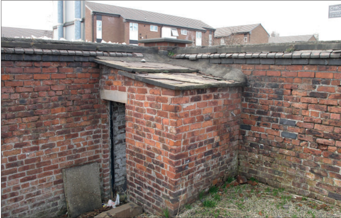
Figure 358: Lean-to privy in the south-western corner of the cemetery
