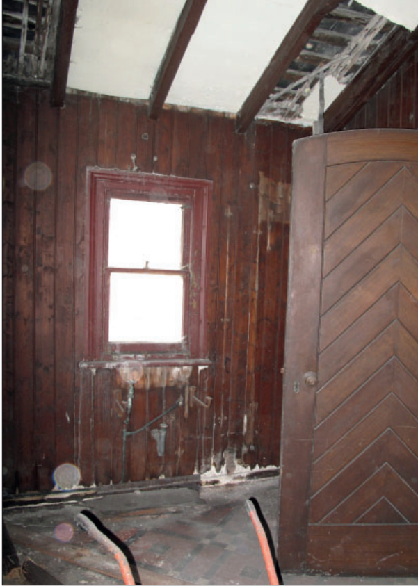
Figure 364: Rear annexe interior
