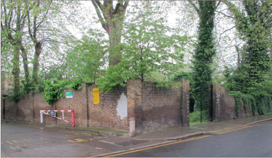
Figure 133: Cemetery wall, from the south-east
