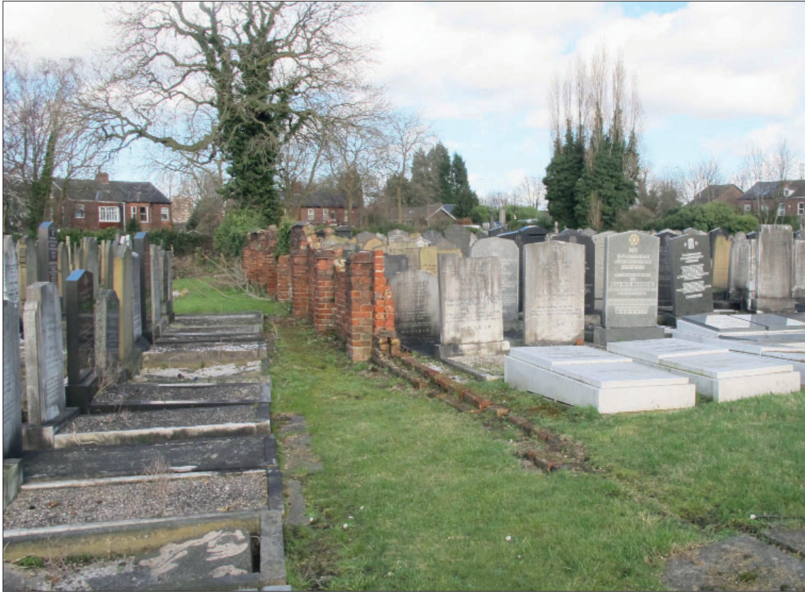
Figure 320: Partially demolished wall between the two Ashkenazi burial grounds
