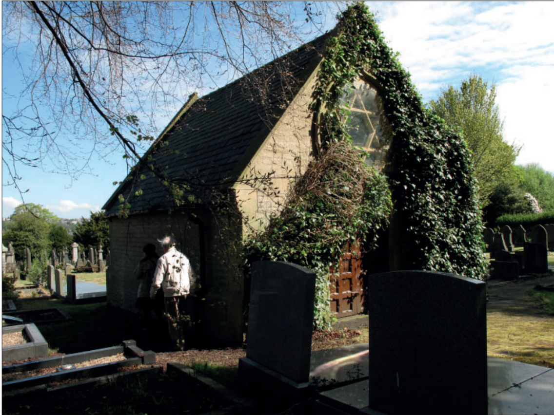
Figure 23: The Reform prayer hall, viewed from the south-west
