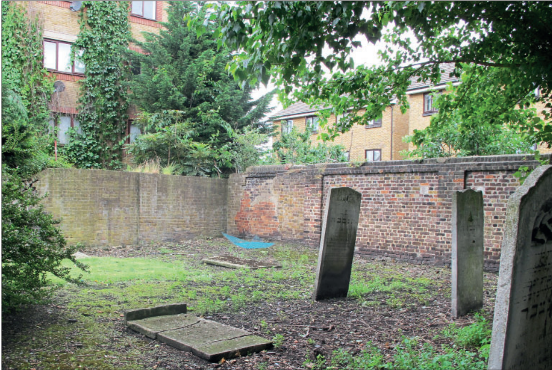
Figure 157: North-west corner where the 19th-century boundary wall (right) is joined by a later section
