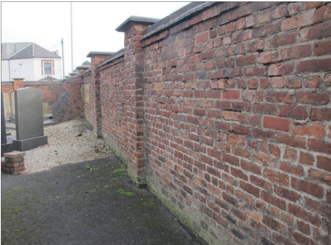
Figure 355: South boundary wall
