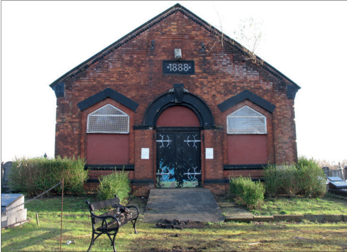
Figure 296: The Ohel north elevation with the main entrance and date stone
