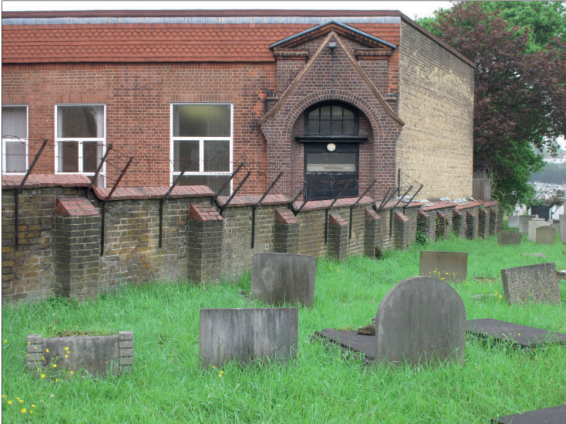
Figure 197: West boundary wall
