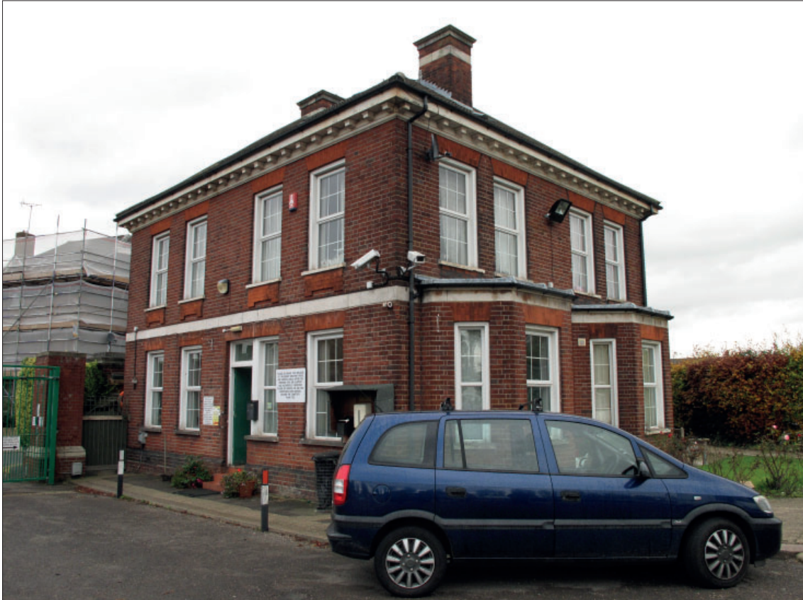
Figure 280: Entrance lodge 1909-10, by Lewis Solomon
