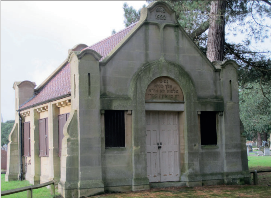
Figure 7: The Ohel viewed from the north
