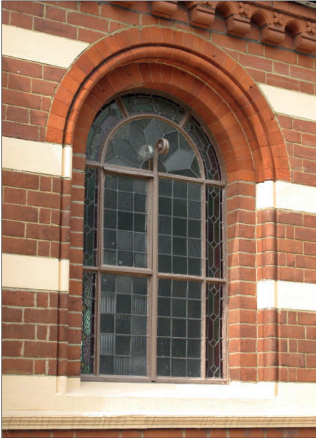
Figure 190: Prayer hall window external detail
