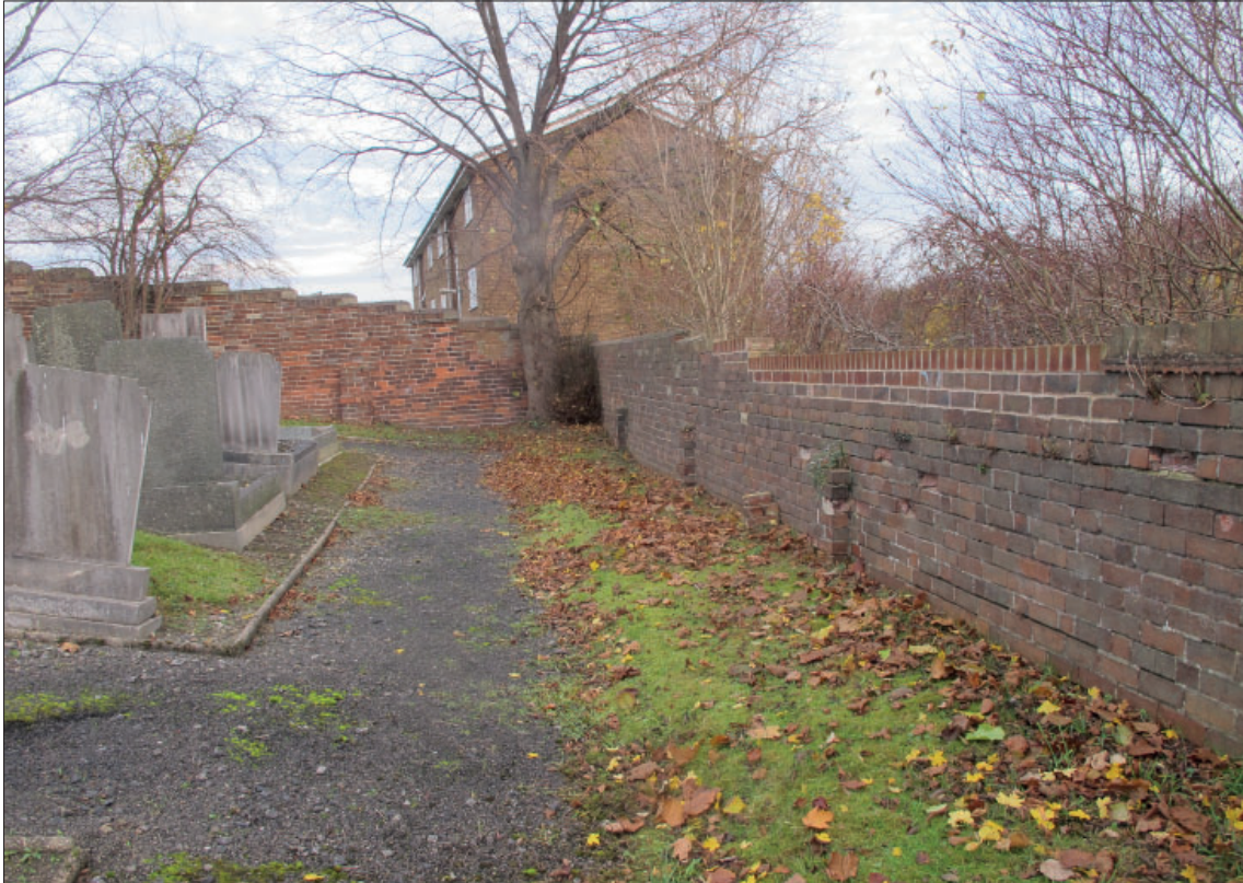
Figure 105: Southern boundary wall on the right, eastern boundary wall ahead
