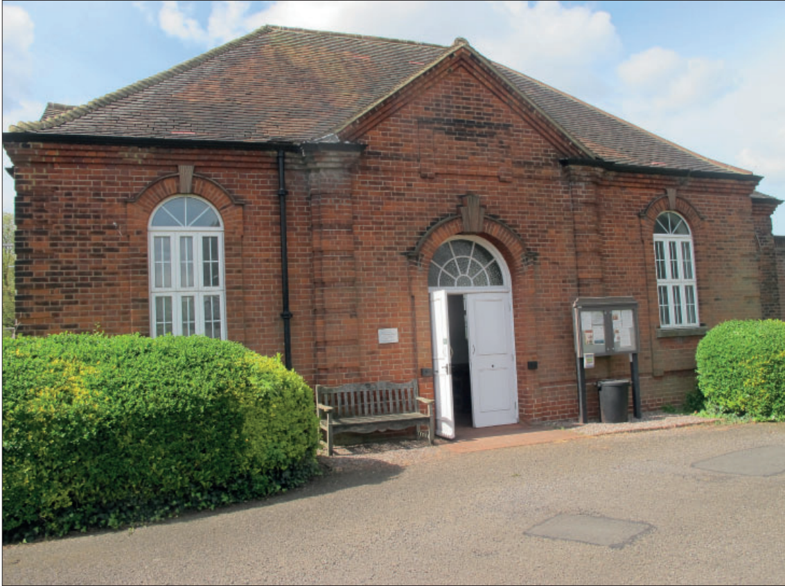
Figure 240: Prayer hall front, view from the north-east
