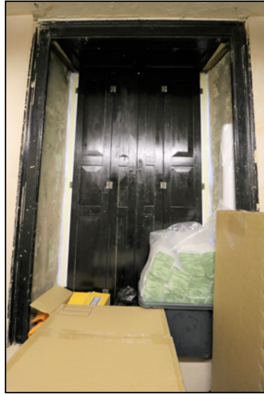
Figure 41. Room G1 window shutters.
