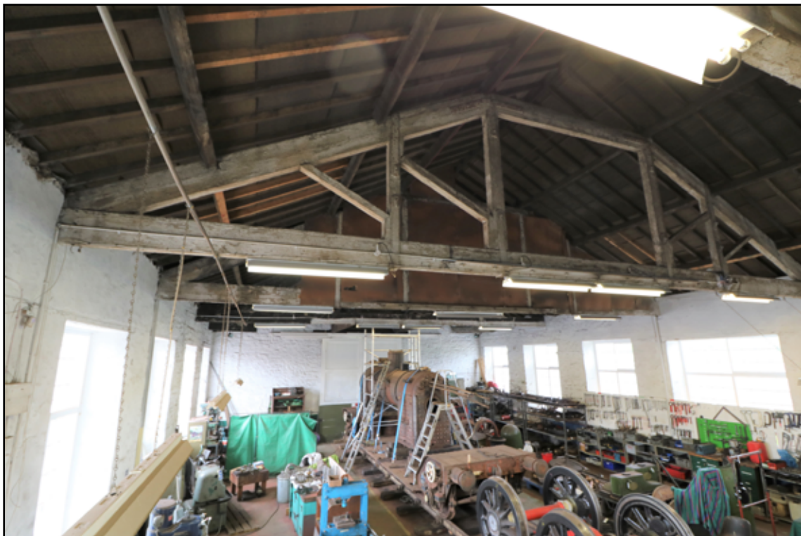
Figure 25. Interior of the north workshop.
