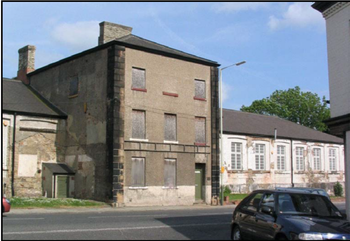
Figure 22. The Hopetown elevation in 2004 . Note to the left are the scars of various outbuildings visible in the rendered walls. (Grenville et al 2004, fig.137, 228). Reproduced by kind permission of Department of Archaeology, University of York.
