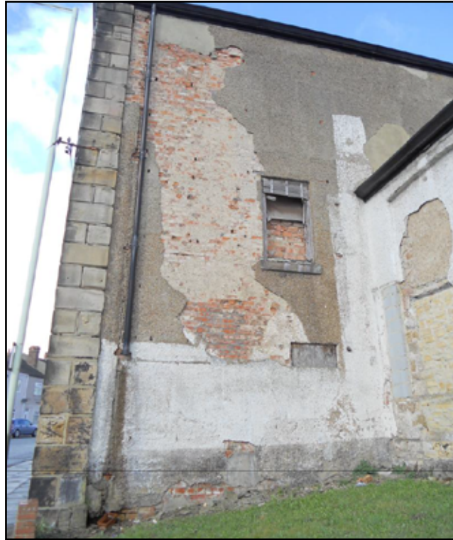
Figure 23. The south elevation of the 'Cottage' with blocked doorway to the right. Reproduced by kind permission of Head of Steam Railway Museum, Darlington.
