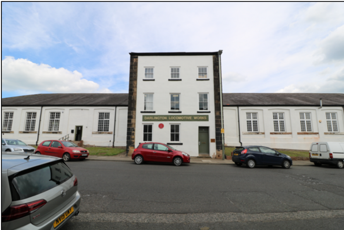
Figure 21. Central block, west elevation seen from Hopetown Lane.
