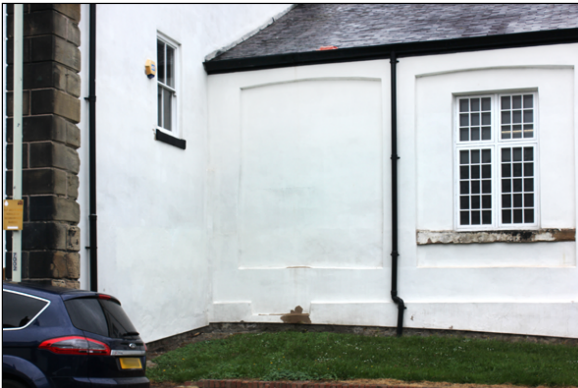
Figure 24. Stepped plinth, west elevation of the southern workshop.
