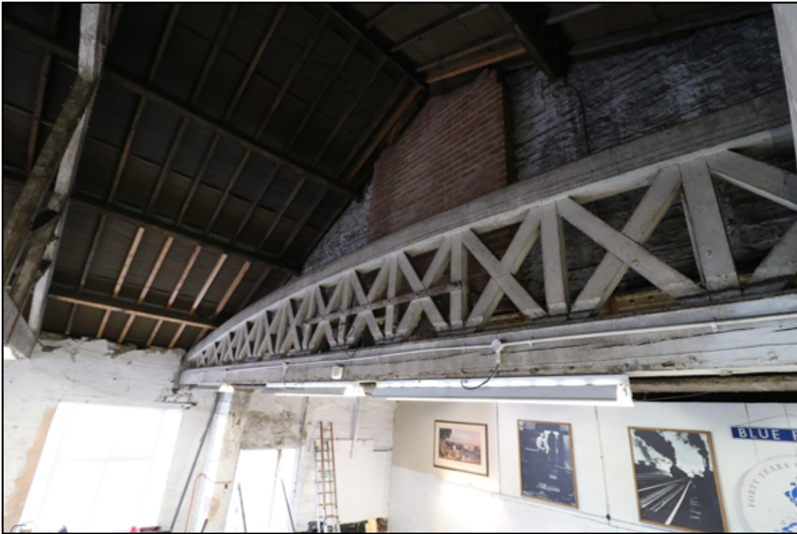
Figure 44. Bow string truss, north workshop.
