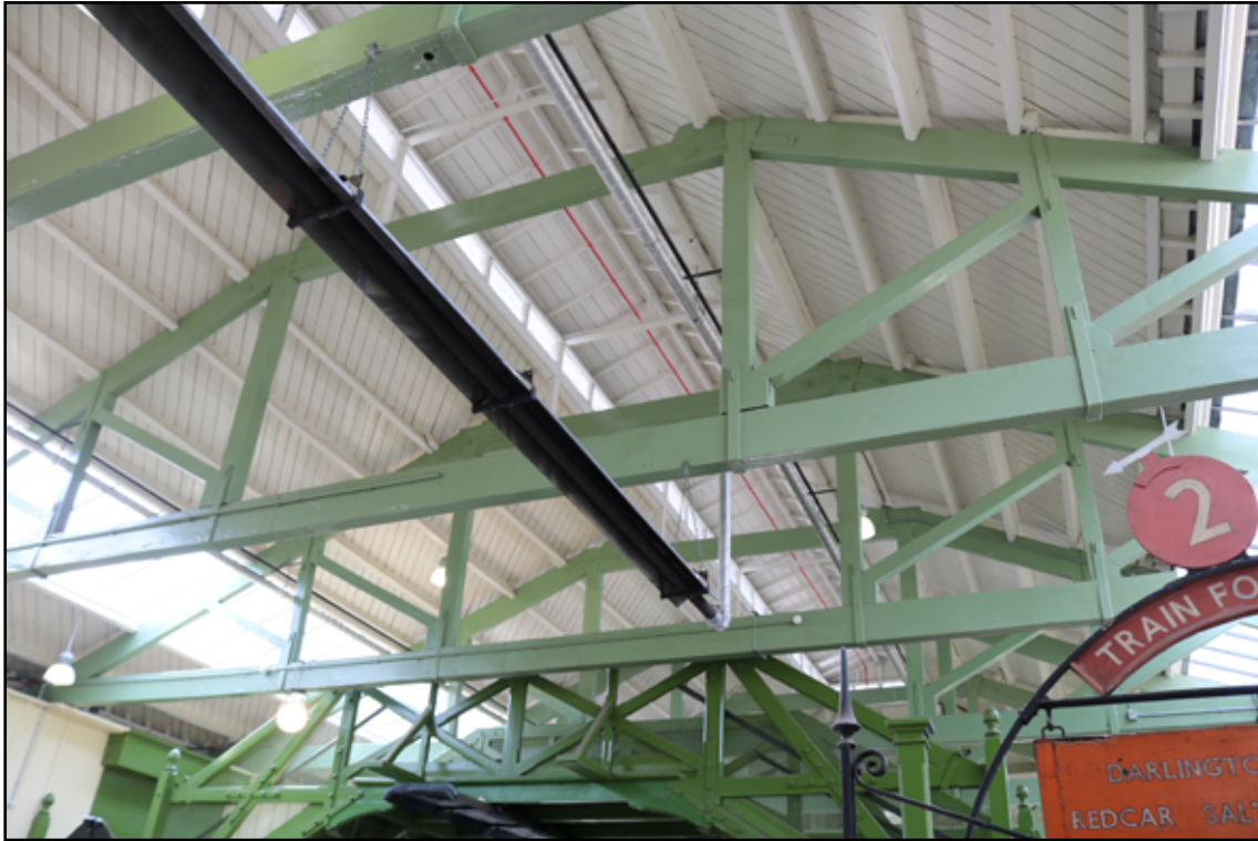
Figure 28. North Road Station roof structure.
