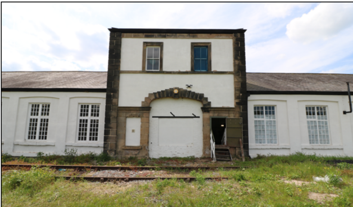
Figure 12. Central block, east elevation today.
