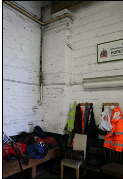
Figure 26. Wall nib with modern wall to the right.
