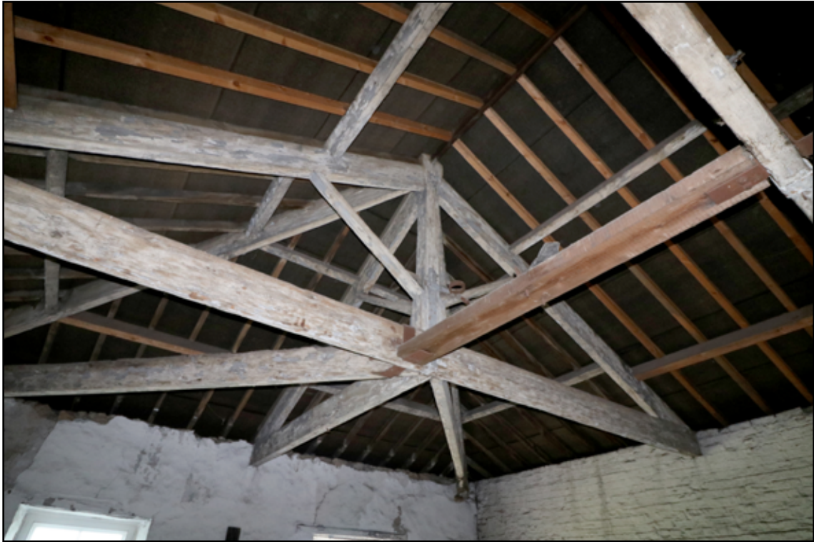
Figure 30. Roof structure in S2.
