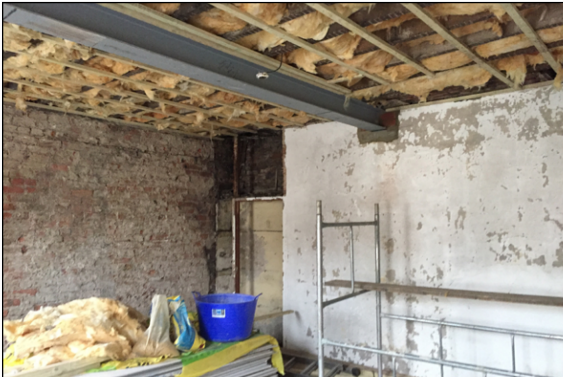
Figure 42. View looking north east into room F1 in 2017 before the walls were plastered and a new ceiling introduced. Signs of the original lath and plaster ceiling are visible on the underside of the ceiling joists, and the faint outline of a blocked fireplace is to the right. The cupboard in the corner has since been plastered over. Reproduced by kind permission of Tony Lord A1/SLT.
