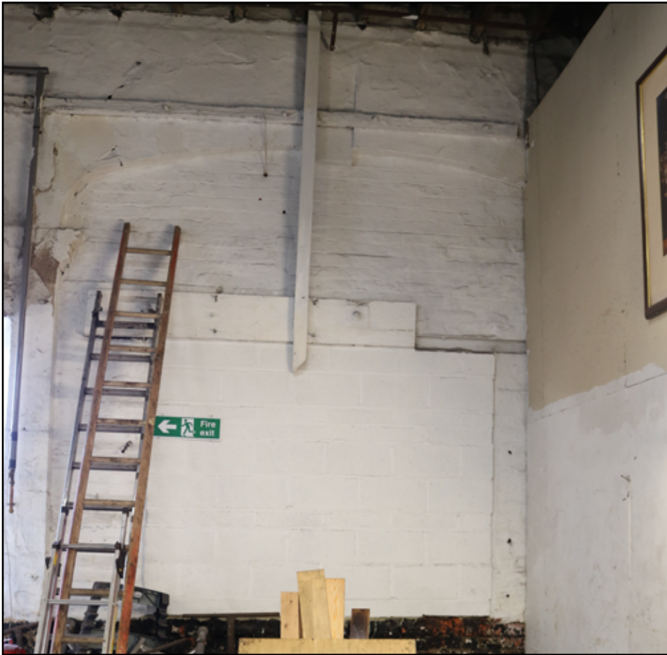
Figure 13. Archway, now blocked, (looking east) as seen in G2.
