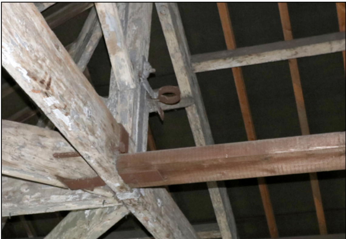
Figure 31. Detail of metal bracket attached to the king post truss which may have formed part of a hoist or lifting gear.
