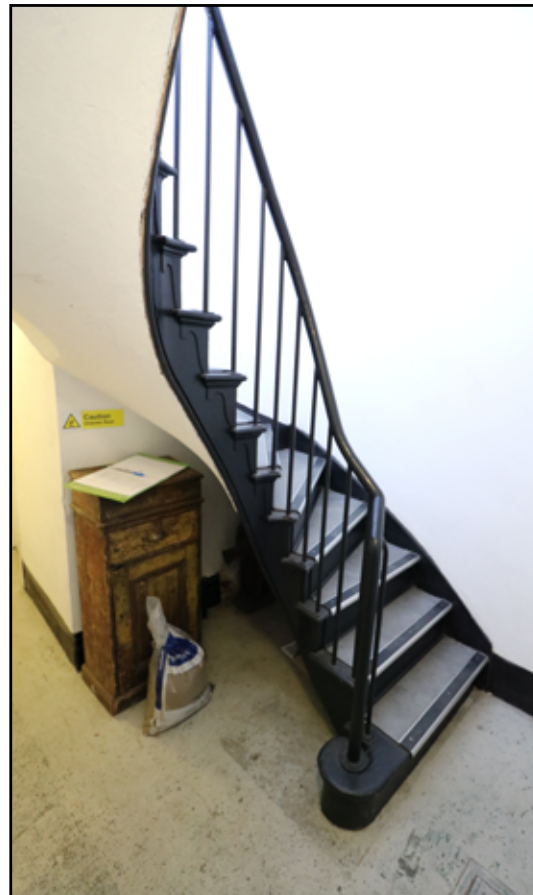
Figure 38. Staircase with modern handrail.
