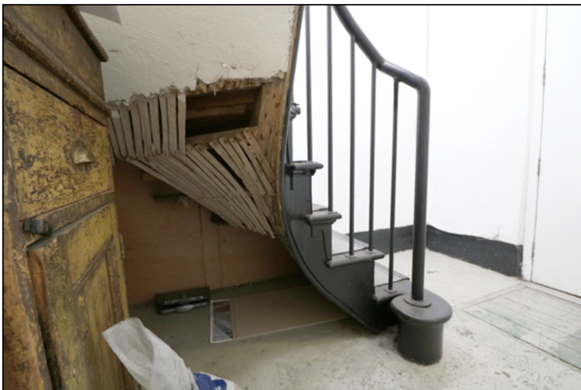
Figure 39. Lath and plaster to underside of staircase.
