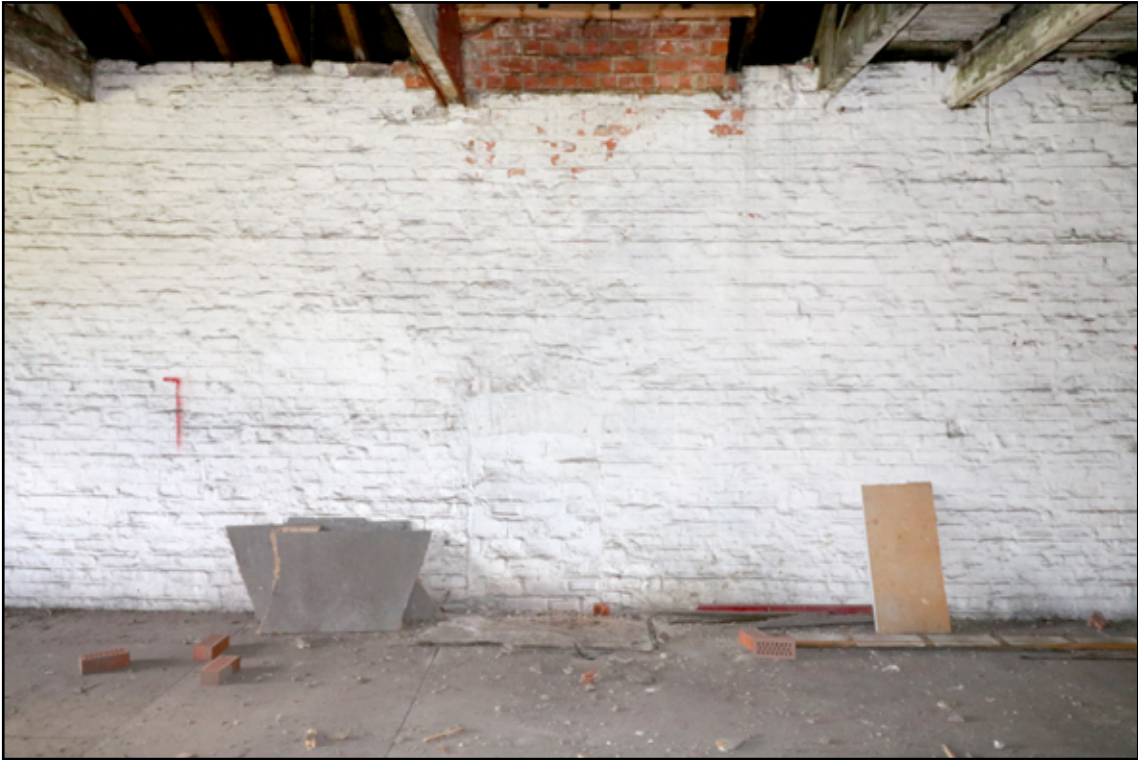
Figure 32. Blocked fireplace with rebuilt stack above.
