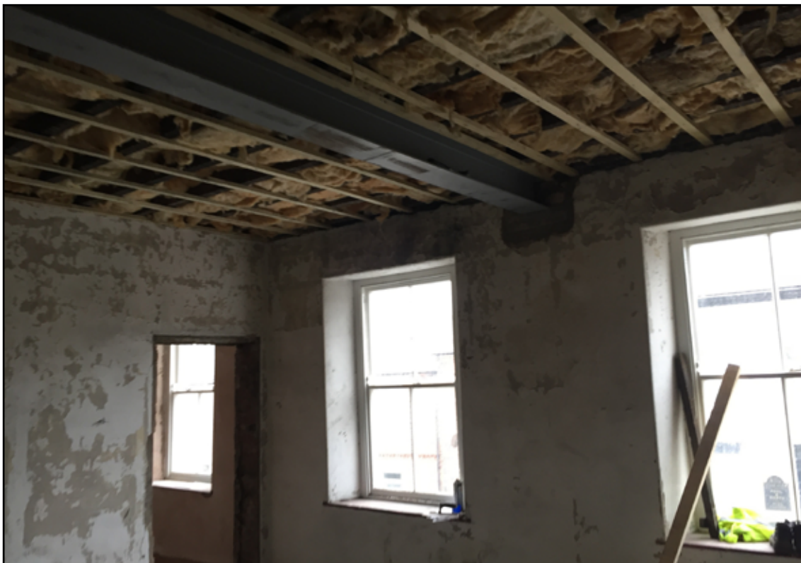
Figure 57. View looking south west in room F1 in 2017 before the walls were plastered and a new ceiling introduced. Reproduced by kind permission of Tony Lord A1/SLT.
