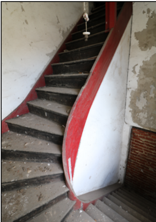
Figure 34. Staircase to workshop and S2.
