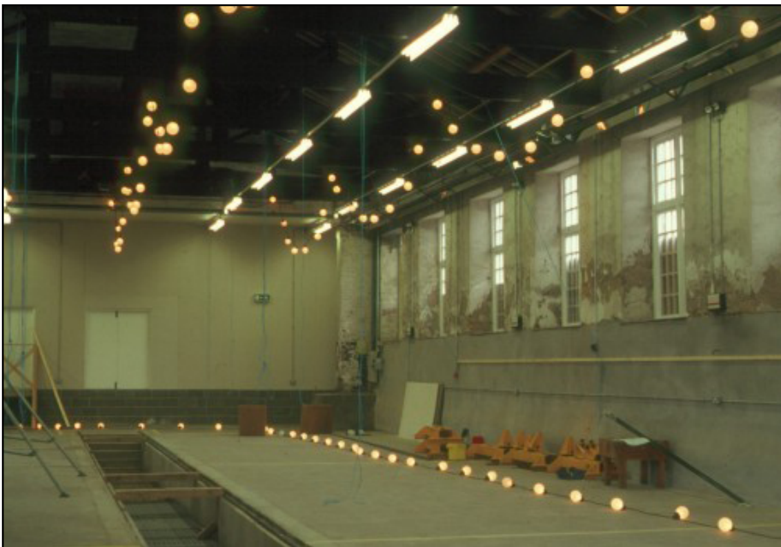
Figure 55. View taken in 1997 of the southern workshop, looking north, showing the new inspection pit. ( https://www.a1steam.com/darlington-locomotive-works/ ).
