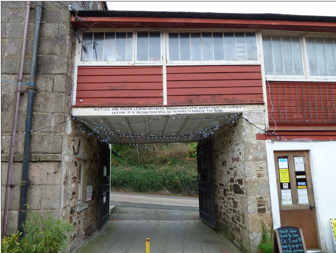
Figure 30: The carriageway in the south-east courtyard range beside the two-storey market house. The weatherboarding is a like-for-like replacement of the previous and possibly of the original arrangement. [Johanna Roethe]
