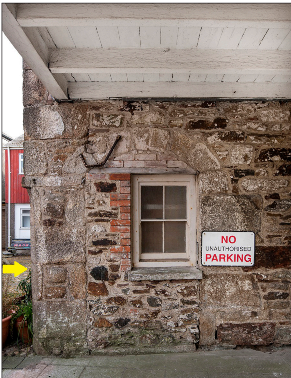
Figure 19: The arches on the south-west elevation (left) and on the north-east elevation (right) of the market house. The arrow in the image to the left indicates a later chamfer. [Left: James O. Davies, DP275887; right: Johanna Roethe]
