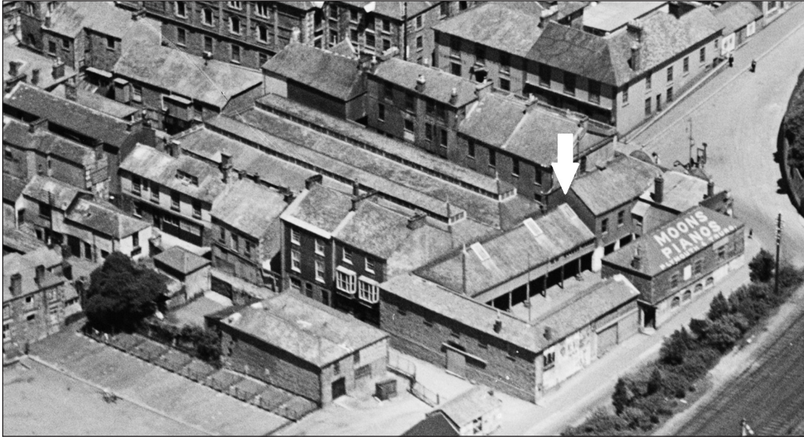
Figure 13: Detail of an oblique aerial photo taken on 24 June 1928, looking north-east. The arrow indicates the north-east end of the north-west range with the inserted first-floor rooms. [© Historic England Archive (Aerofilms Collection), EPW021734]
