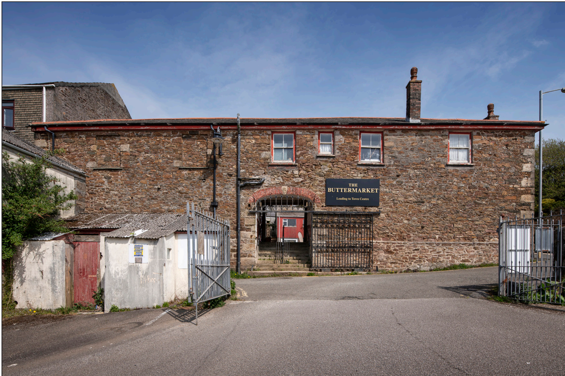
Figure 22: The south-west elevation of the south-west courtyard range, seen from the Fair Meadow carpark. [James O. Davies, DP275878]
