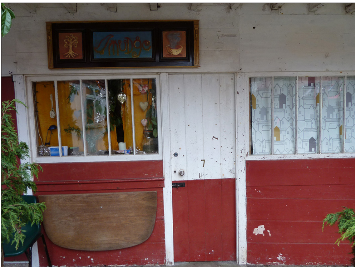
Figure 28: Unit 7 on the ground floor of the south-west courtyard range, with the window of unit 8 to the right. All of the panelling, the window surrounds and the door date from the original date of the building. [Johanna Roethe]
