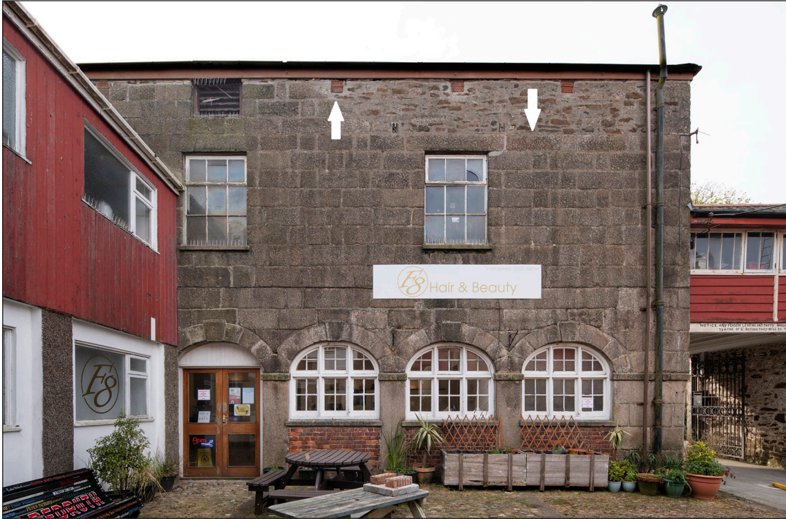
Figure 18: The north-west elevation of the market house, seen from the courtyard. The left arrow indicates the line of the former cross gable, that to the right the line of the original eaves height. [James O. Davies, DP275883]
