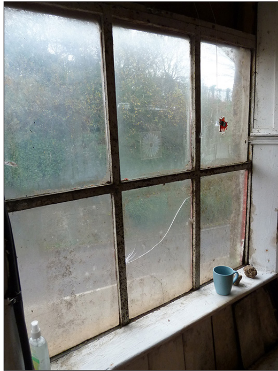
Figure 44: First-floor metal window in the south-east elevation of the market house. [Johanna Roethe]
