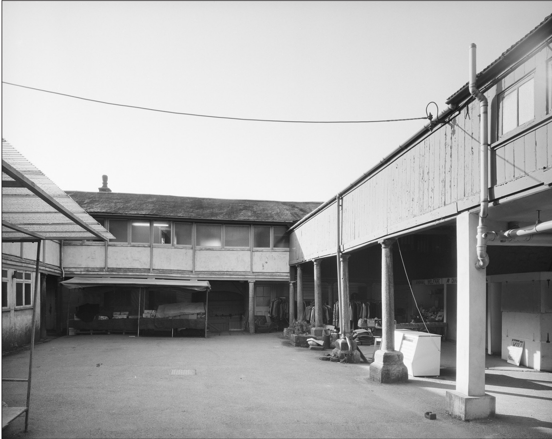
Figure 15: The courtyard in February 1989, looking north-west. [© Crown copyright. Historic England Archive, BB057063]
