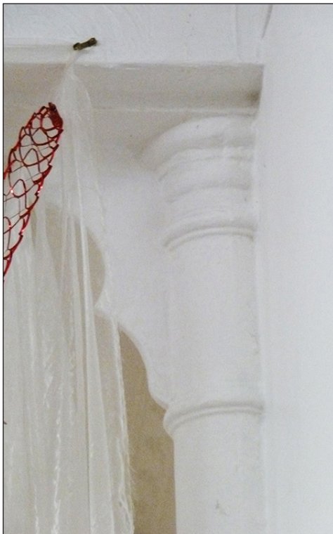
Figure 43: A capital (left) and the maker's mark of the cast-iron columns on the ground floor of the market house. [Johanna Roethe]
