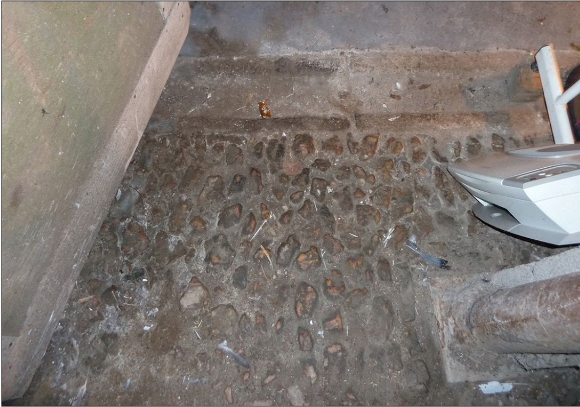
Figure 37: Historic cobbles and granite drain just inside the current entrance to the lower ground floor of the Mining Exchange. [Johanna Roethe]
