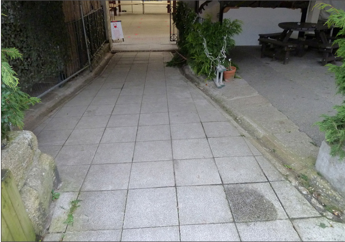
Figure 36: The late 19th-century floor drains lining the remaining (western) entrance from the meat market into the courtyard. The paving between the drains is a modern replacement. [Johanna Roethe]
