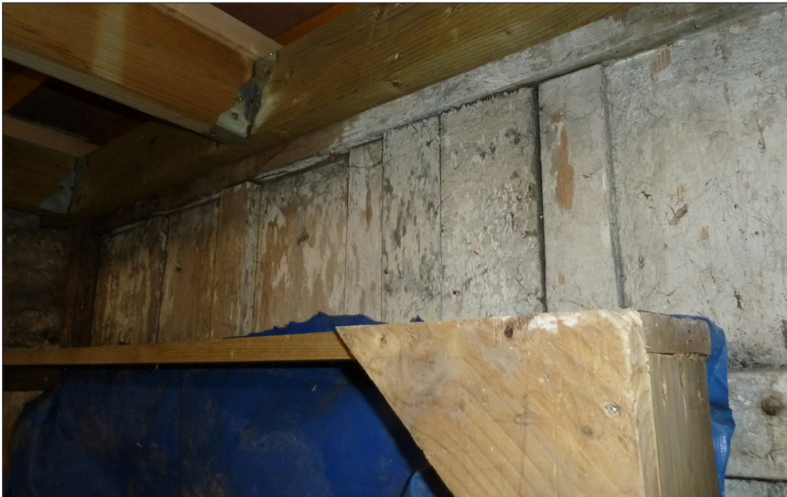
Figure 27: Example of historic boarding between stalls in unit 10 at the north end of the south-west courtyard range. [Johanna Roethe]
