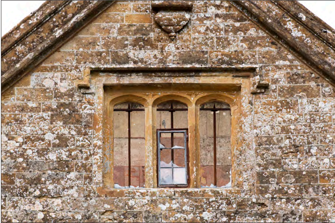
Appendix Two Figure 27: Exterior north wing, east elevation, detail of gable-end window, looking west (DP275917)
