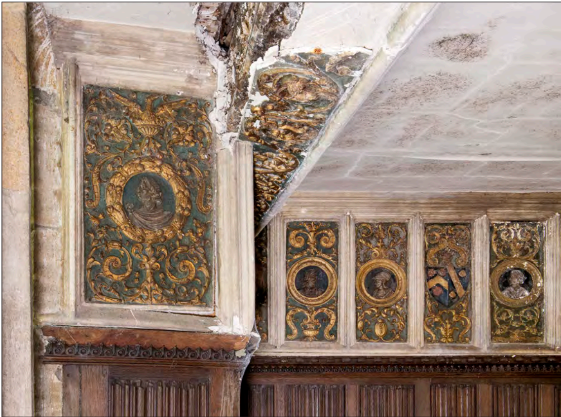
Appendix Two Figure 92: Interior, north wing, ground-floor room, detail of frieze, looking south (DP275982)
