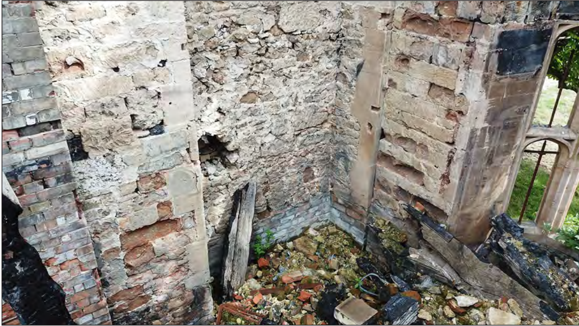
Figure 19 The eastern end of the north wall of the south wing, showing recess infilled with rubble stone (Drone survey image © Historic England)
