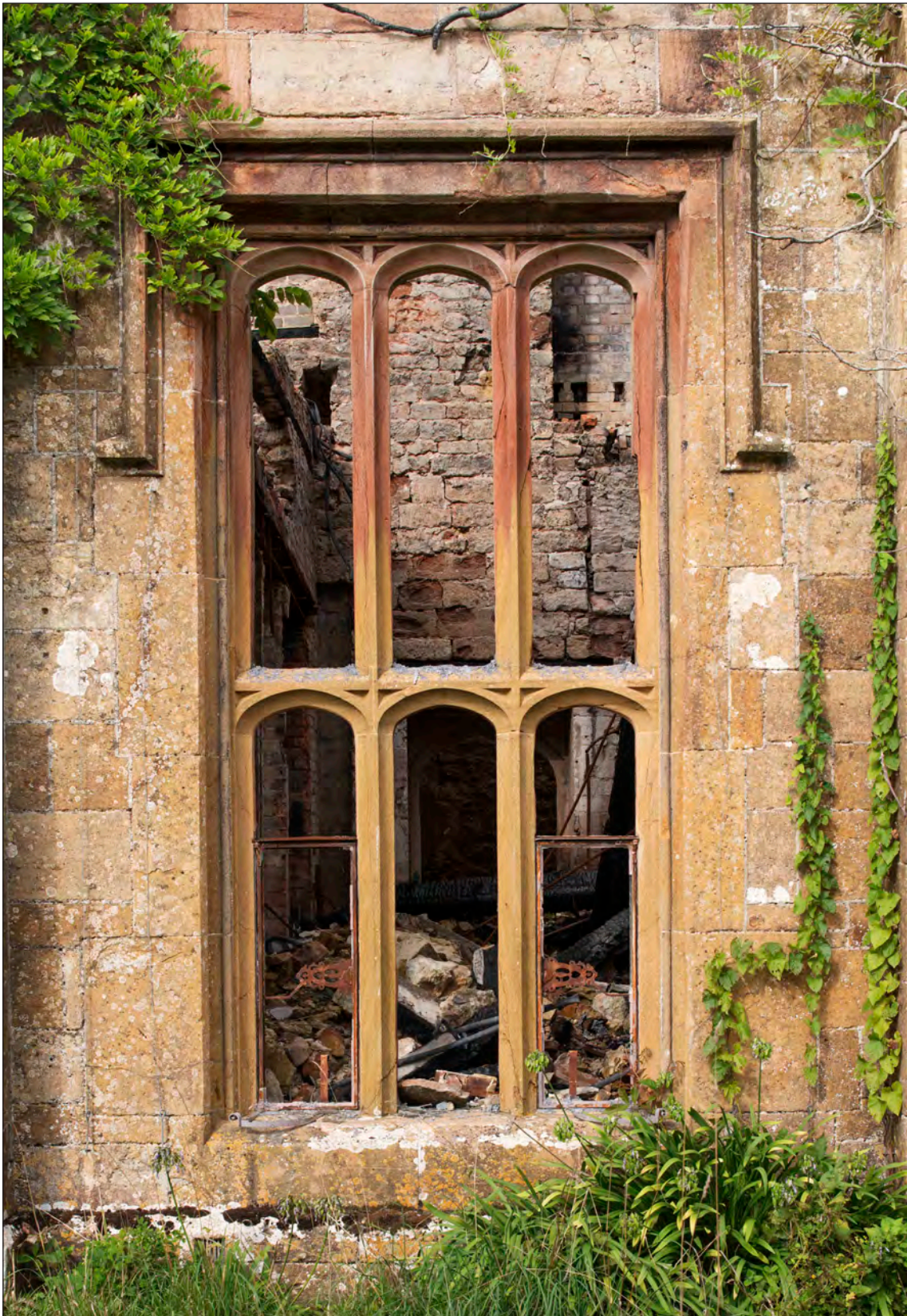
Appendix Two Figure 50: Exterior, south wing, south elevation, detail of window to the east of the central partition, looking north (DP275940)
