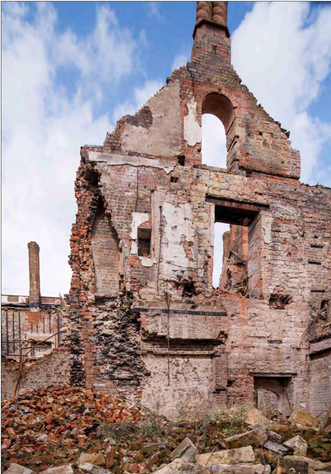
Appendix Two Figure 46: Interior, south wing, west end, looking north (DP275936)
