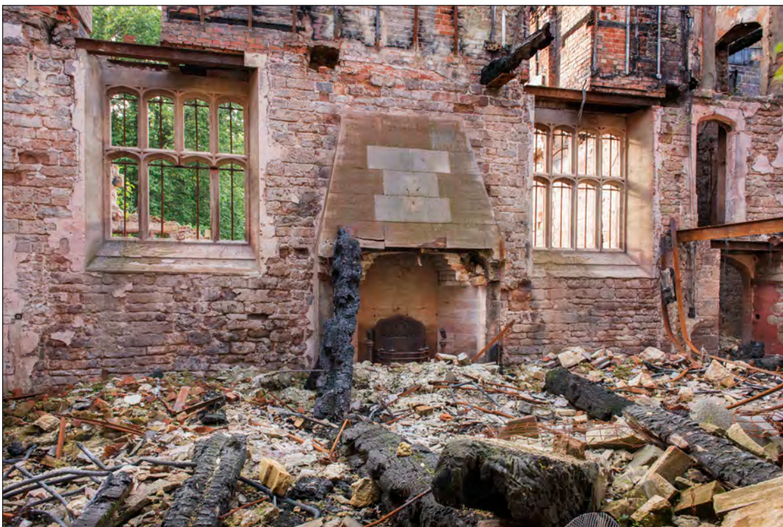
Appendix Two Figure 71: Interior, main range, hall, detail of west elevation, looking west (DP275961)
