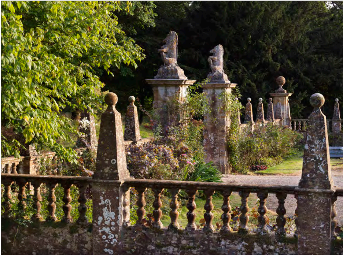
Appendix Two Figure 129: Exterior, forecourt, looking south (DP276019)
