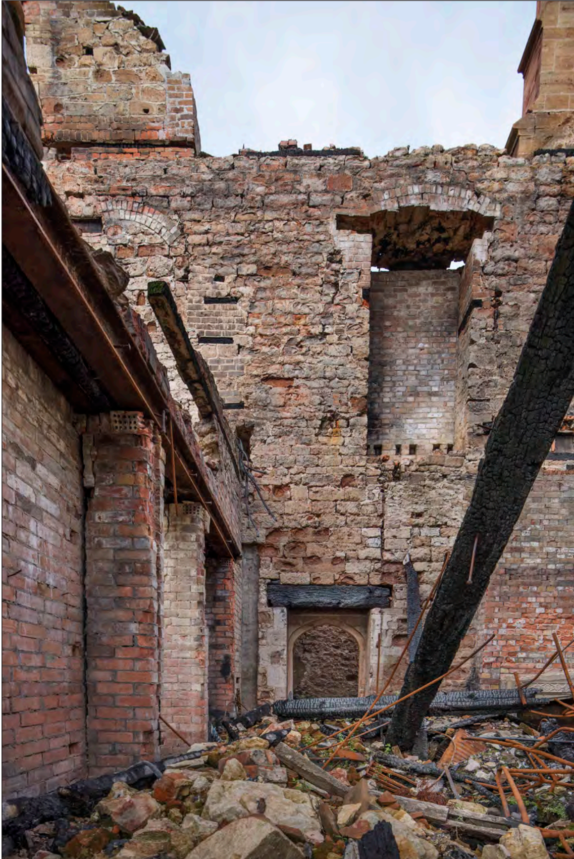
Appendix Two Figure 116: Interior, south wing, centre of north elevation, looking north (DP276006)
