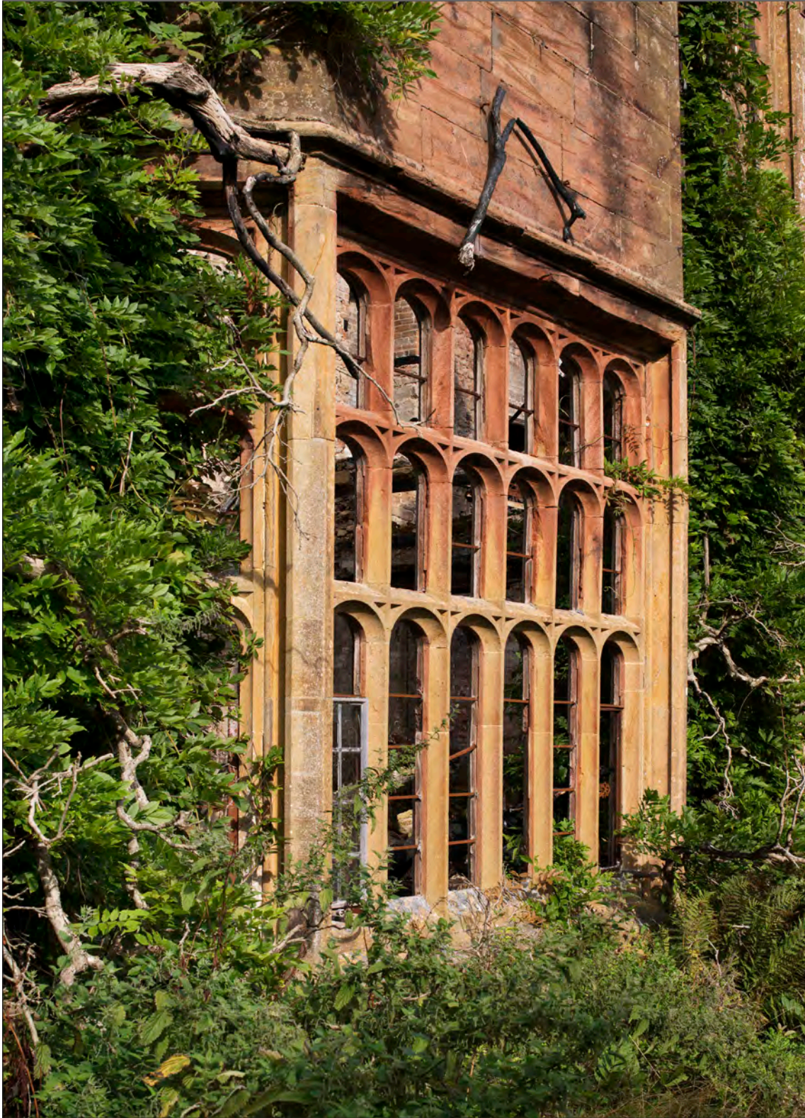
Appendix Two Figure 58: Exterior, south wing, south elevation, detail of bay window, looking north east (DP275948)
