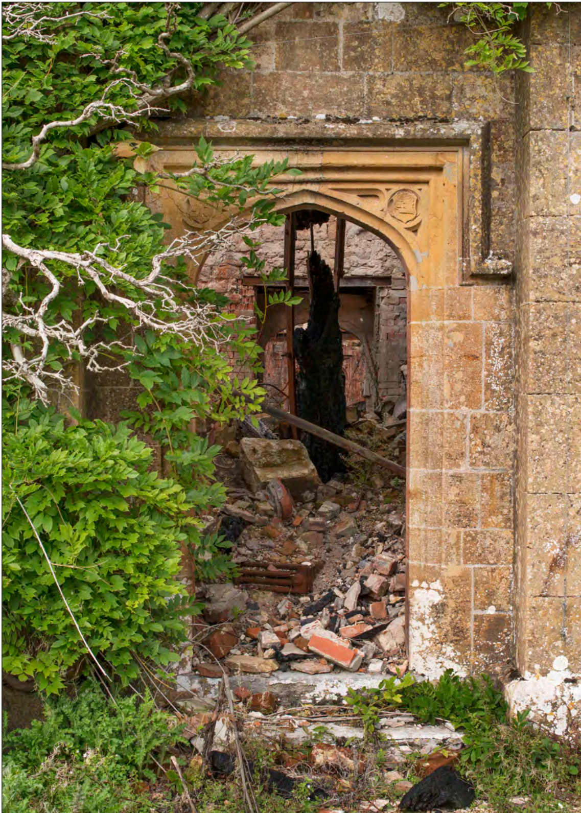
Appendix Two Figure 49: Exterior, south wing, south elevation, detail of doorway, looking north (DP275939)
