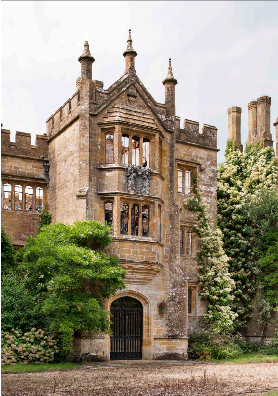
Appendix Two Figure 36: Exterior, east porch and north stair, east elevation, looking north west (DP275926)
