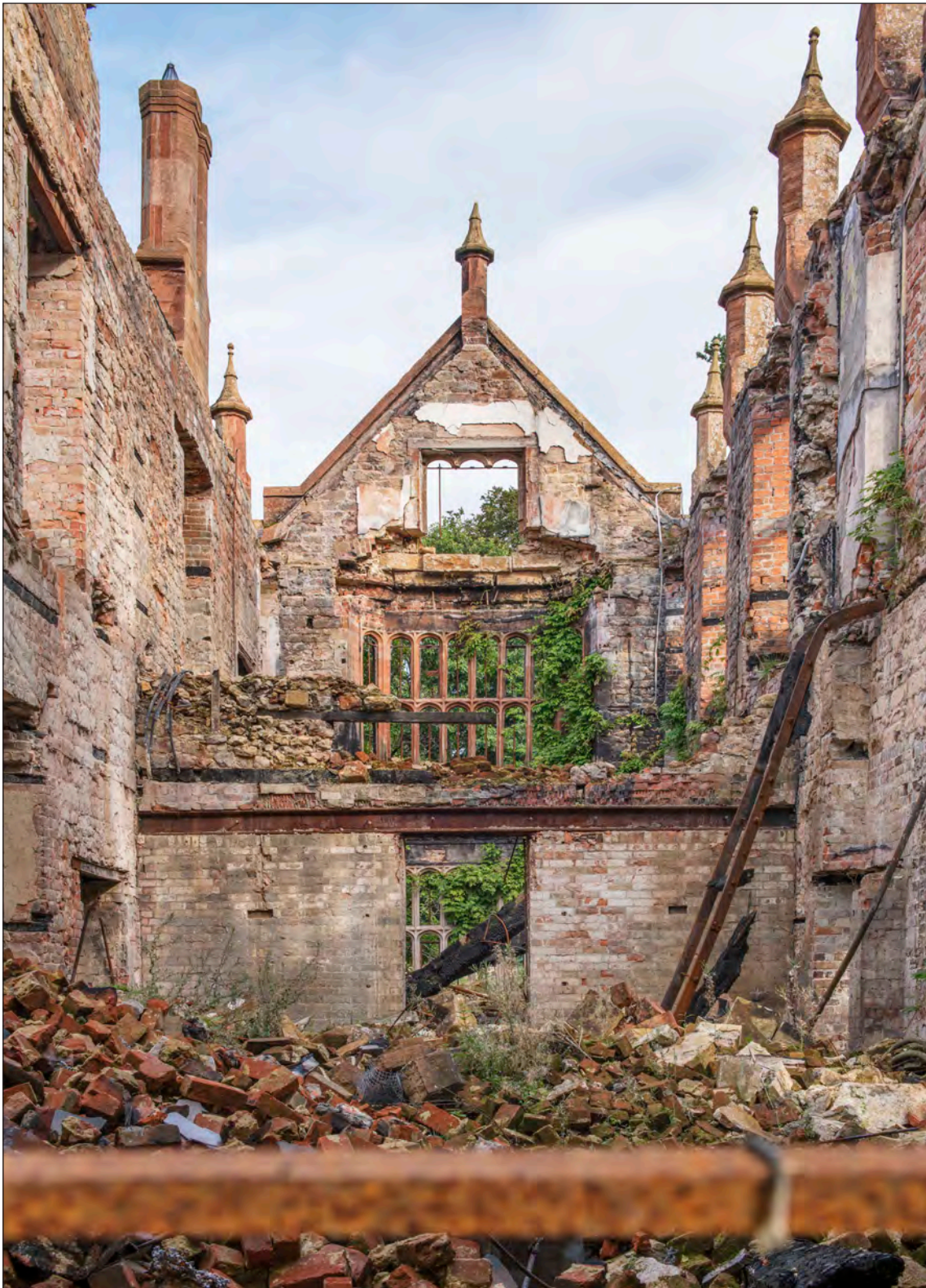
Appendix Two Figure 66: Interior, south wing, looking east (DP275956)
