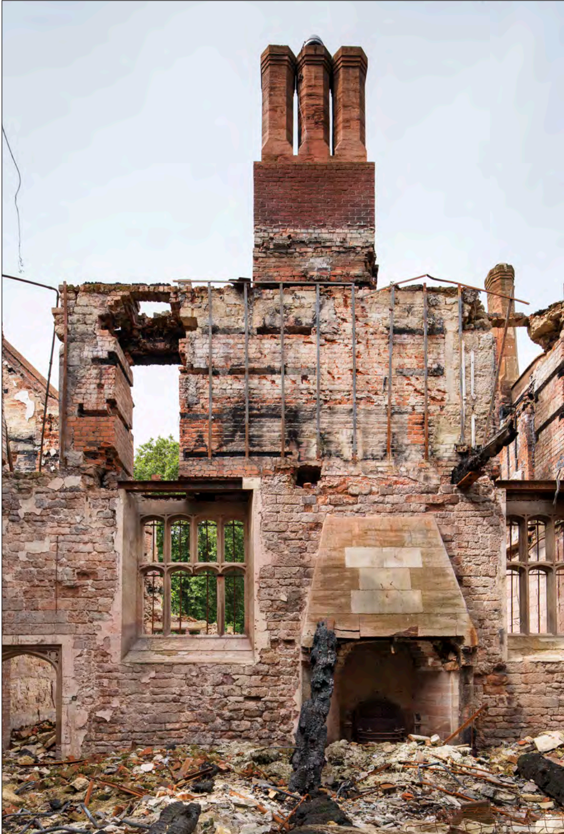
Appendix Two Figure 84: Interior, main range, hall, west elevation, looking west (DP275974)
