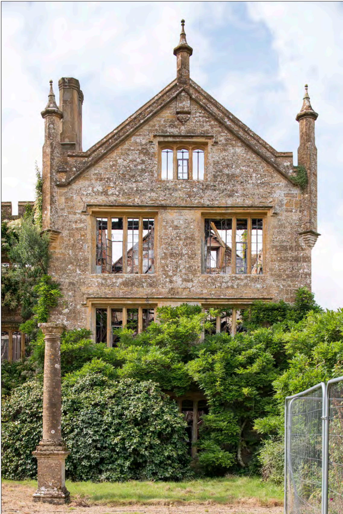
Appendix Two Figure 30: Exterior, north wing, east elevation, looking west (DP275920)
