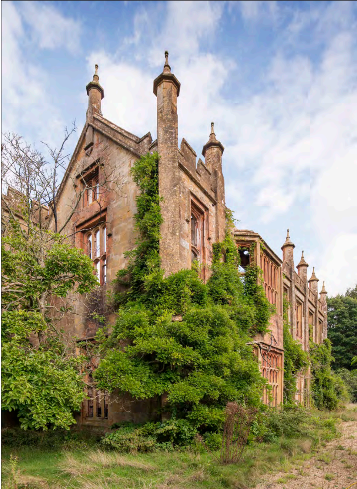
Appendix Two Figure 45: Exterior, south wing, west and south elevations, looking north east (DP275935)
