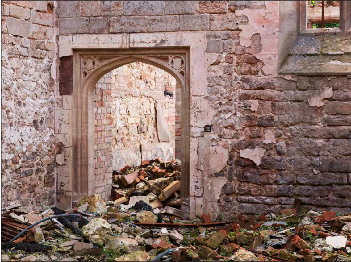
Appendix Two Figure 72: Interior, main range, hall, detail of doorway to dining room, looking west (DP275962)
