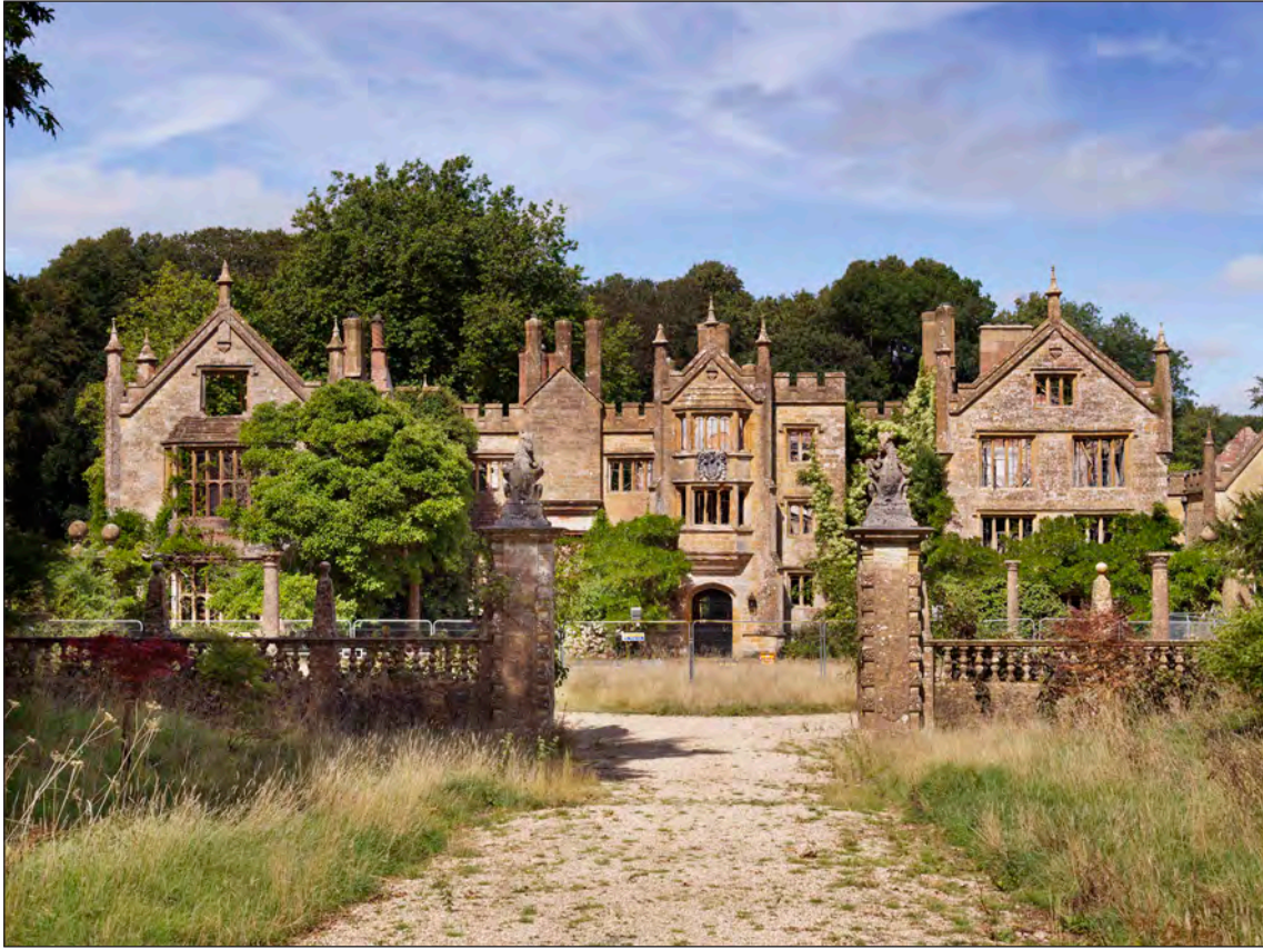
Appendix Two Figure 128: Exterior, east elevation and forecourt, looking west (DP276018)
