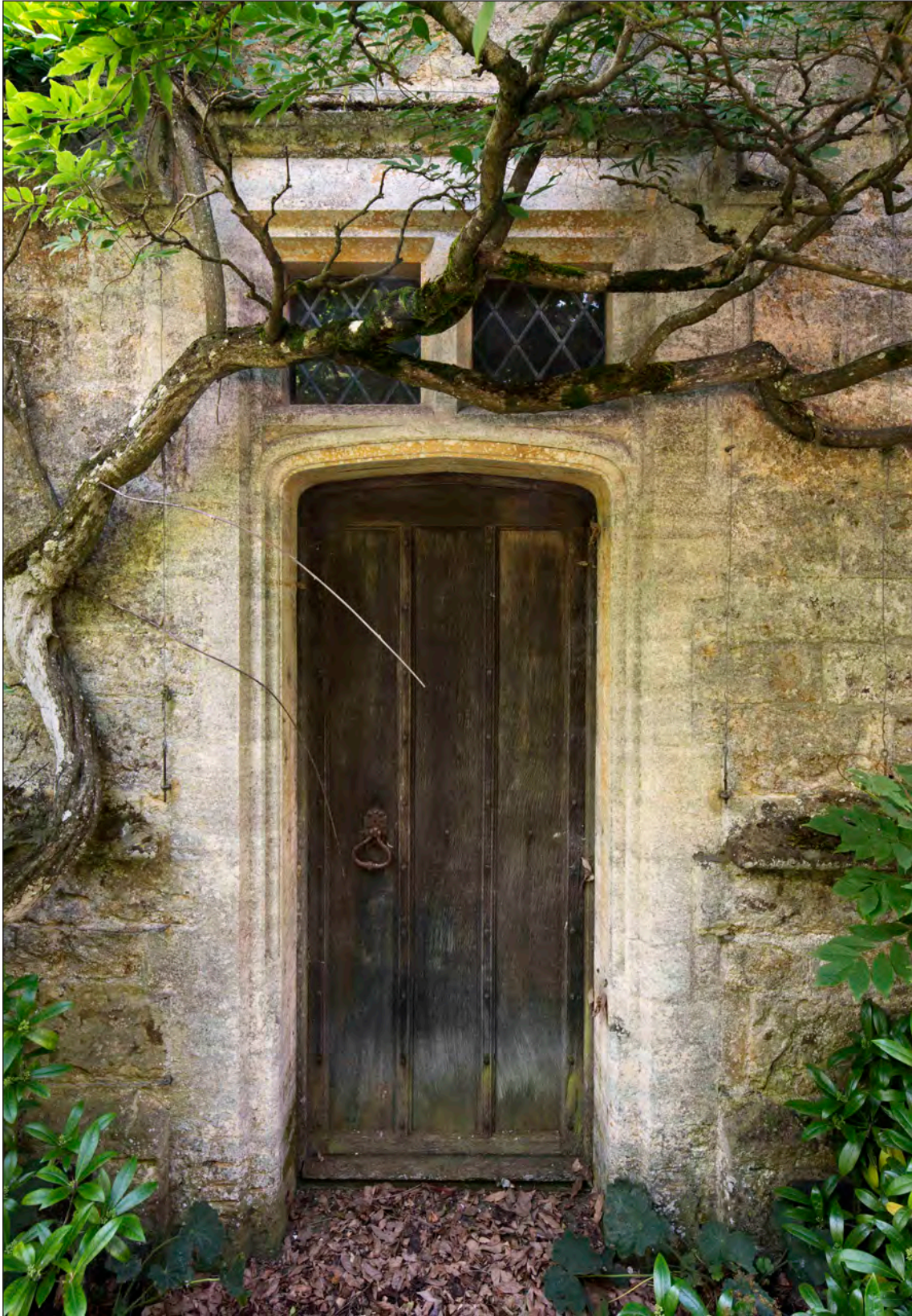
Appendix Two Figure 20: Exterior, north wing, north elevation, detail of door, looking south (DP275910)
