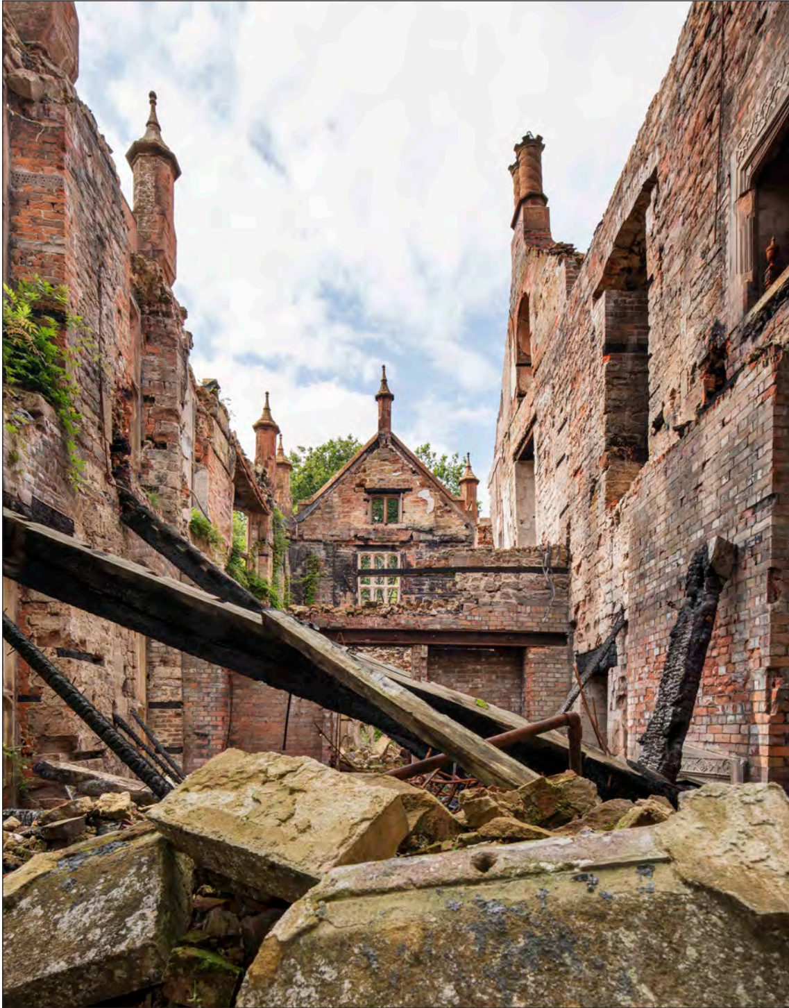
Appendix Two Figure 41: Interior, south wing, looking west (DP275931)
