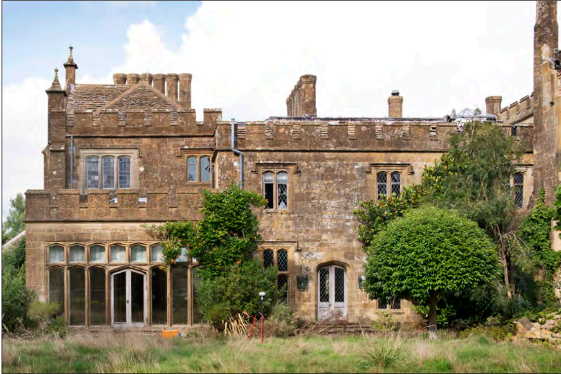
Appendix Two Figure 57: Exterior, service range, south elevation, looking north (DP275947)
