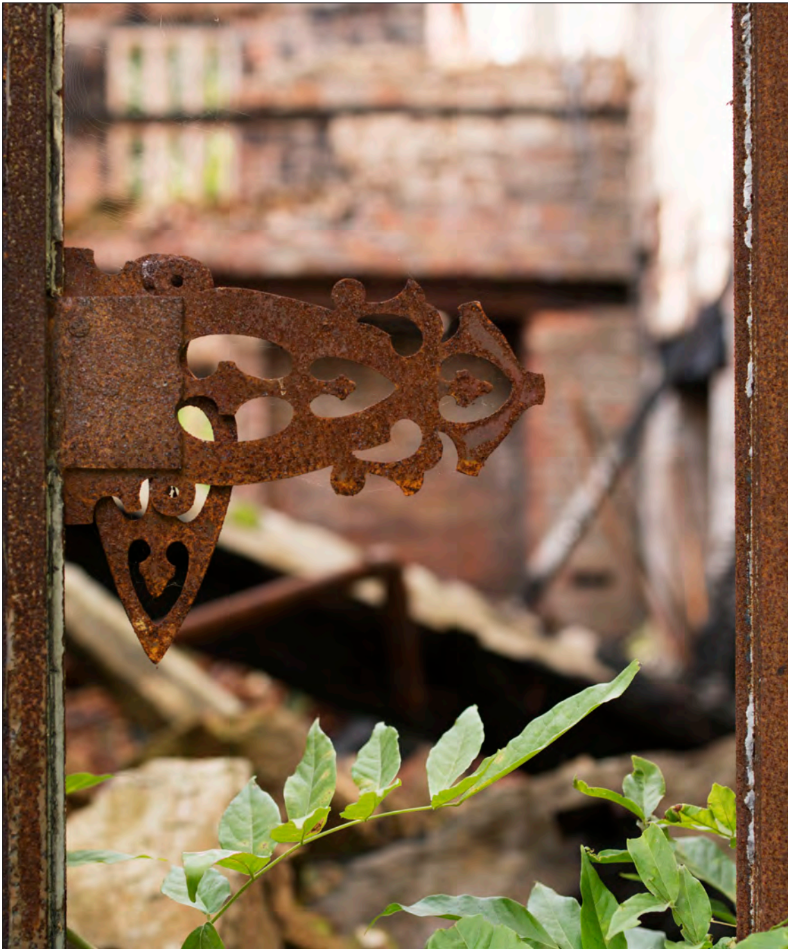
Appendix Two Figure 39: Exterior, south wing, east elevation, detail of ground floor of bay window showing window latch, looking west (DP275929)
