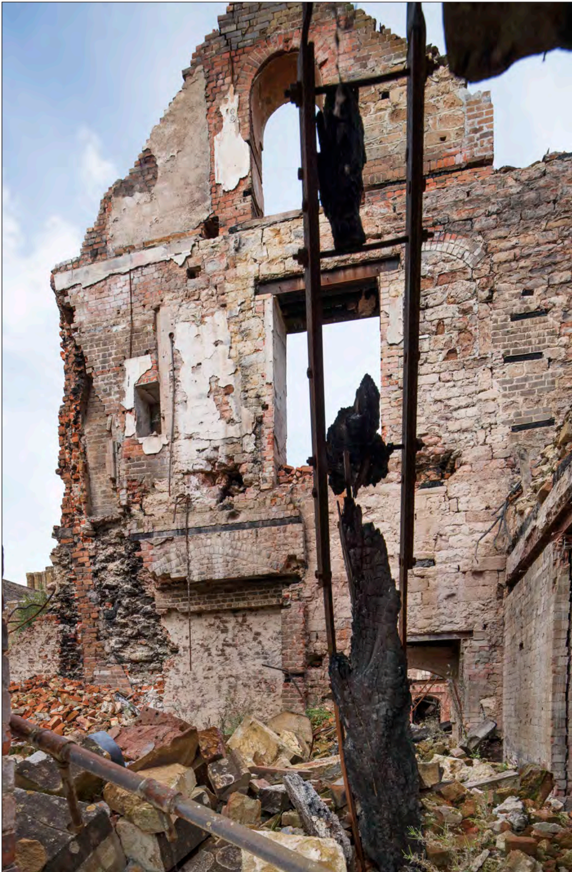
Appendix Two Figure 115: Interior, south wing, west end of north elevation, looking north (DP276005)
