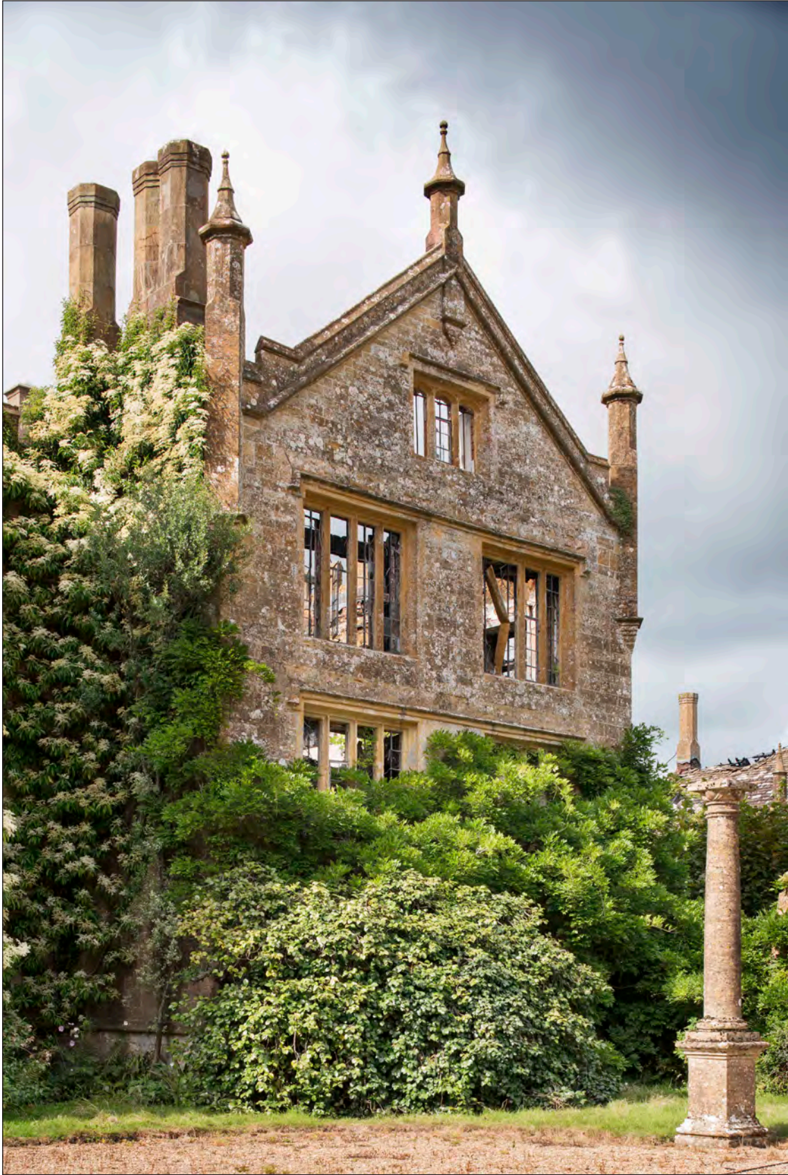
Appendix Two Figure 35: Exterior, north wing, east elevation, looking north west (DP275925)
