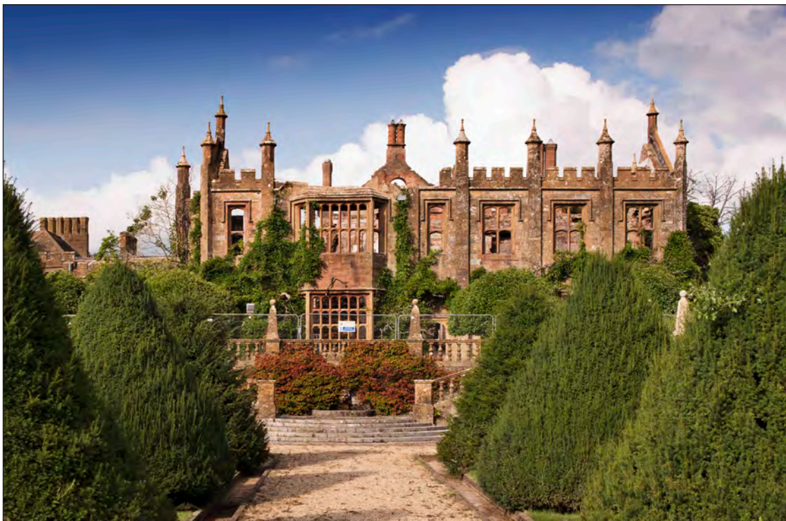
Appendix Two Figure 60: Exterior, south wing, south elevation, looking north (DP27950)
