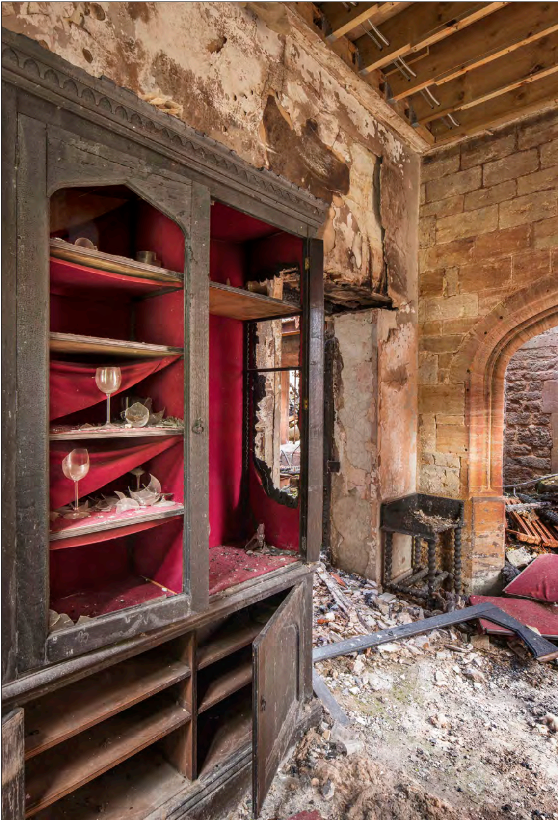
Appendix Two Figure 126: Interior, west porch, north and east elevations, looking north east (DP276016)
