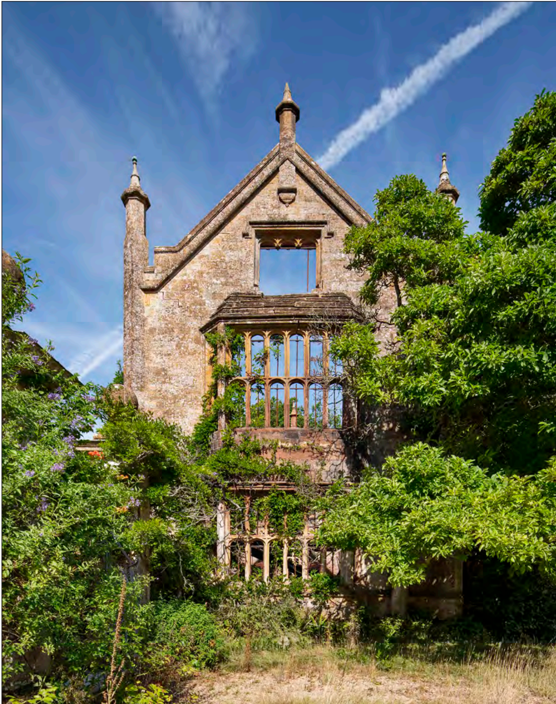
Appendix Two Figure 5: Exterior, south wing, east elevation, looking west (DP275895)
