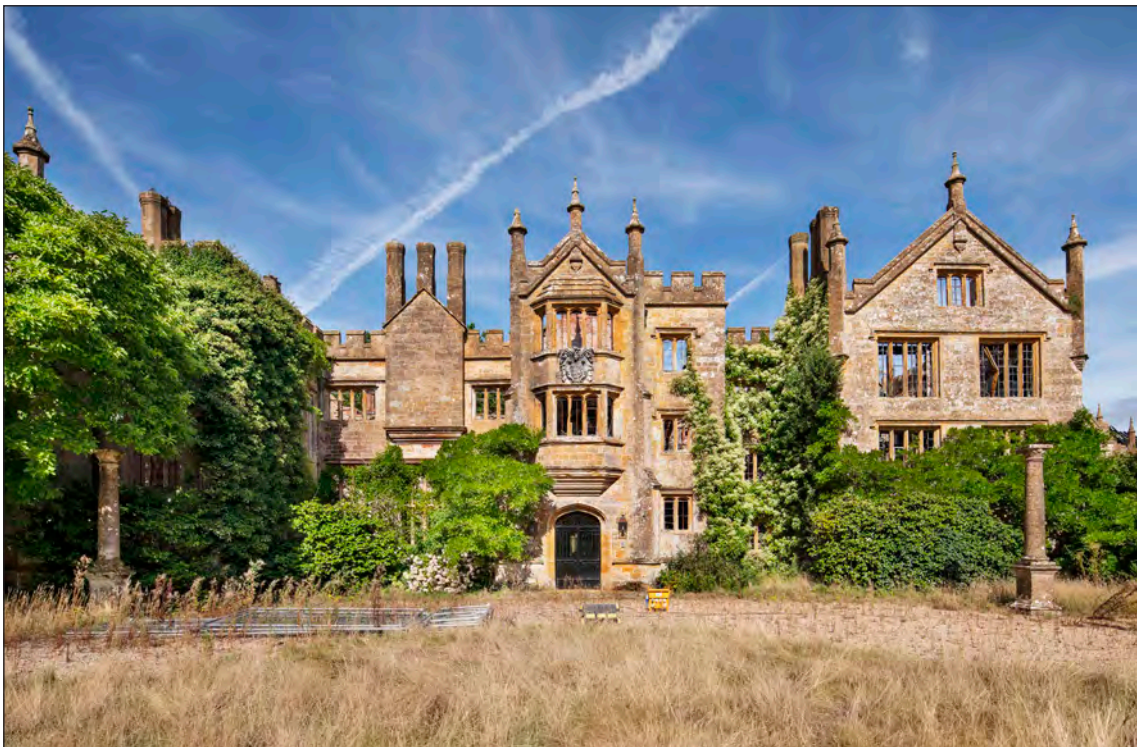
Appendix Two Figure 7: Exterior, main range and north wing, east elevation, looking west (DP275897)
