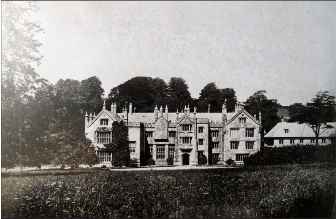
Figure 3 Parnham in 1874, showing the stable block to the north (HEA BB80/883)
