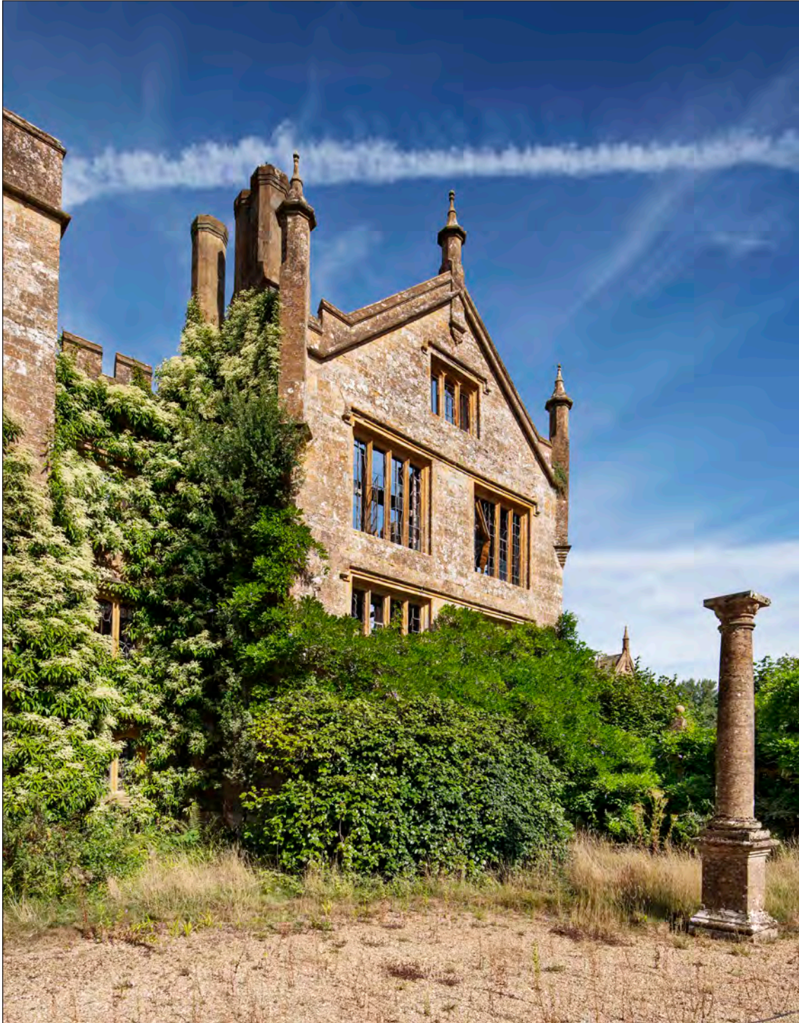
Appendix Two Figure 9: Exterior, north wing, east elevation, looking north west (DP275899)
