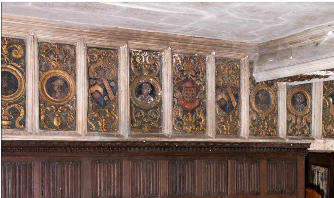
Appendix Two Figure 91: Interior, north wing, ground-floor room, detail of frieze, looking south west (DP275981)
