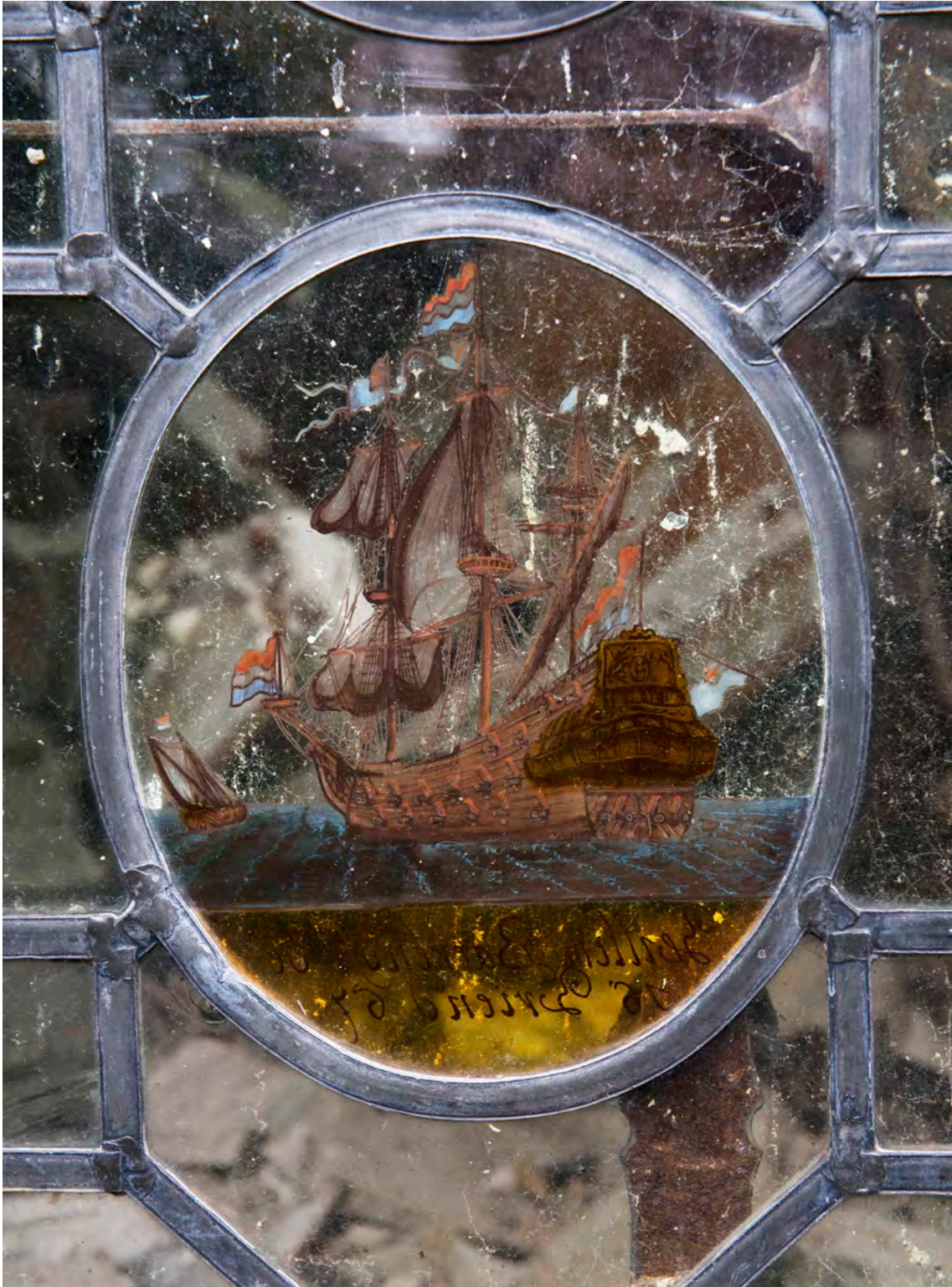
Appendix Two Figure 101: Exterior, north wing, north elevation, detail of stained glass in central ground-floor window, looking south (DP275991)
