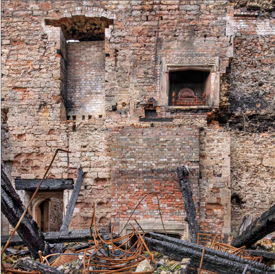
Appendix Two Figure 119: Interior, south wing, western portion of north elevation, showing fireplaces, looking north (DP276009)
