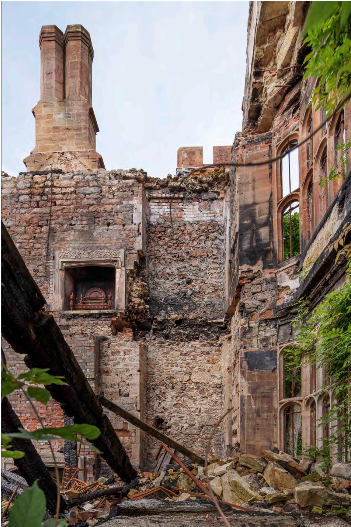
Appendix Two Figure 118: Interior, south wing, eastern end of north elevation, looking north (DP276008)
