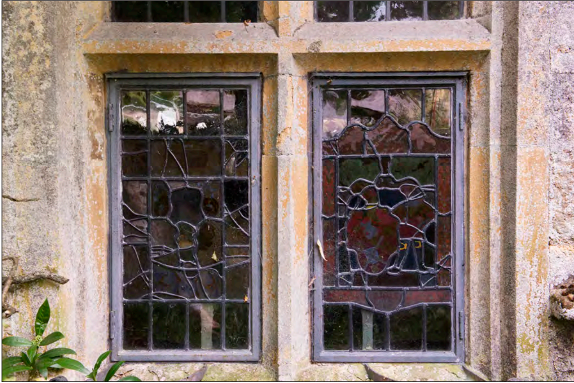
Appendix Two Figure 98: Exterior, north wing, north elevation, detail of stained glass in eastern ground-floor window, looking south (DP275988)
