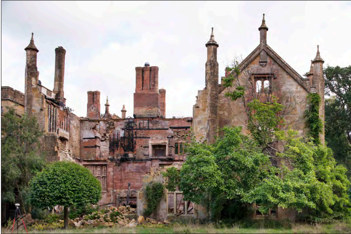
Appendix Two Figure 47: Exterior, dining room and south wing, west elevation, looking east (DP275937)
