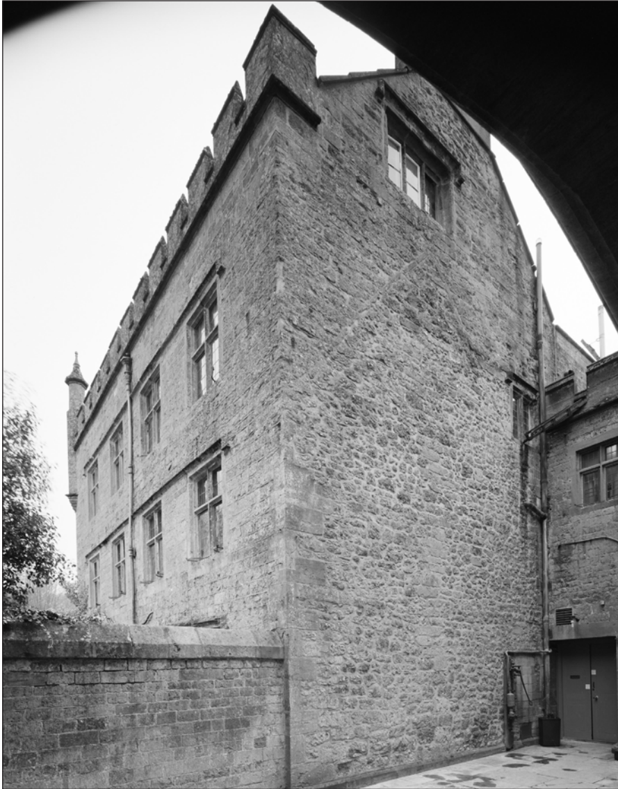
Figure 20 West wall of north wing, showing the earlier, lower roof line visible in 1998, prior to the construction of the Bertram Stair (HEA BB99/04424)
