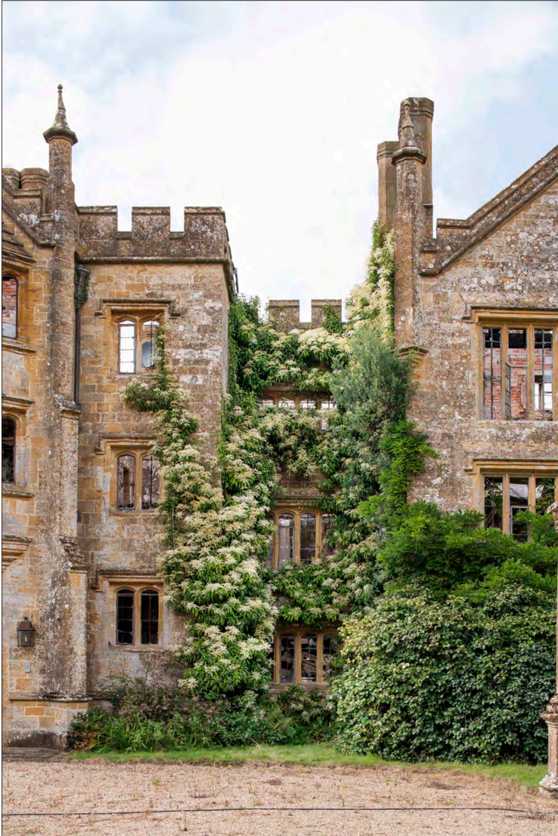
Appendix Two Figure 31: Exterior, main range and north stair, east elevation, looking west (DP275921)
