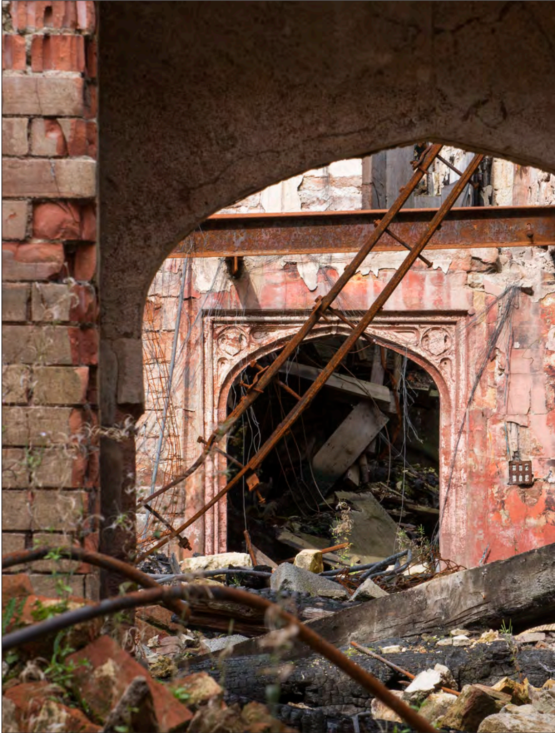
Appendix Two Figure 108: Interior, main range, hall, north elevation, detail of west doorway, seen through the doorway from the south wing, looking north (DP275998)
