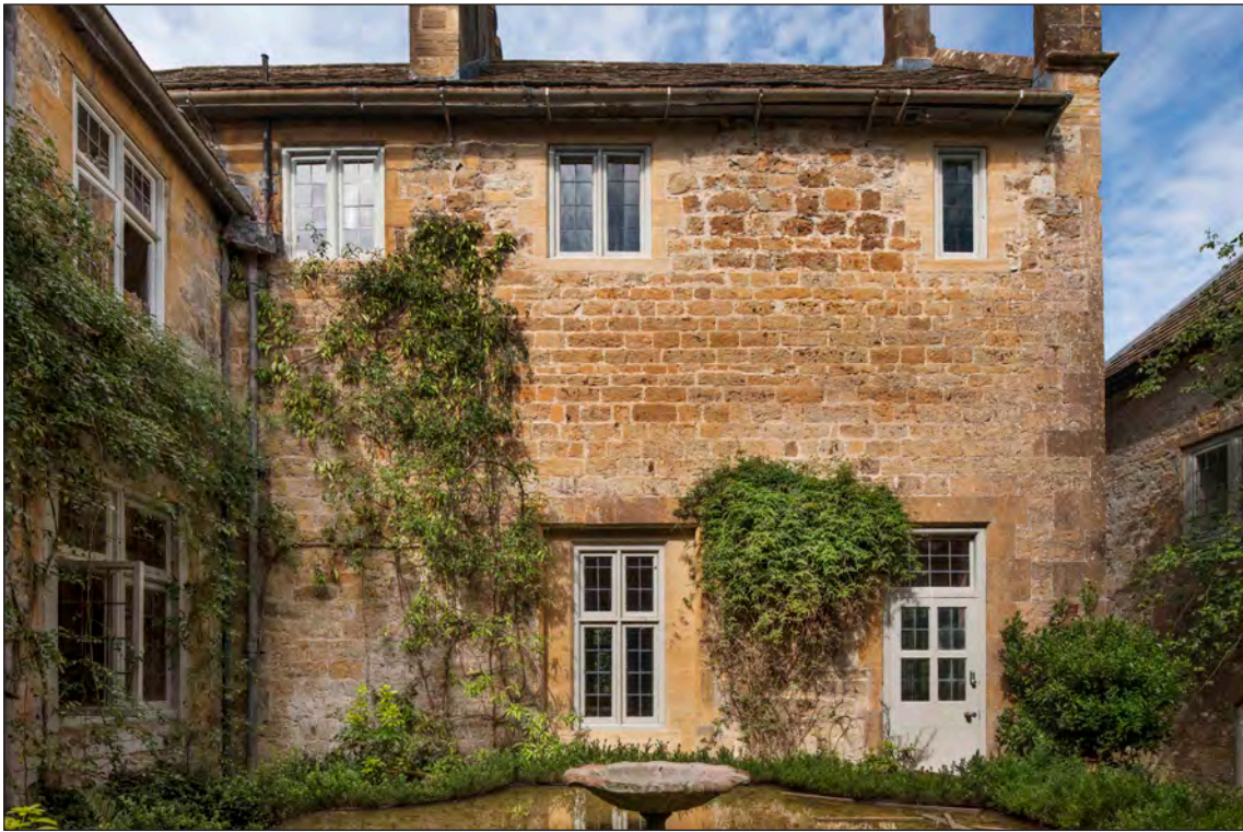
Appendix Two Figure 79: Exterior, service courtyard, service range, east elevation looking west (DP275969)
