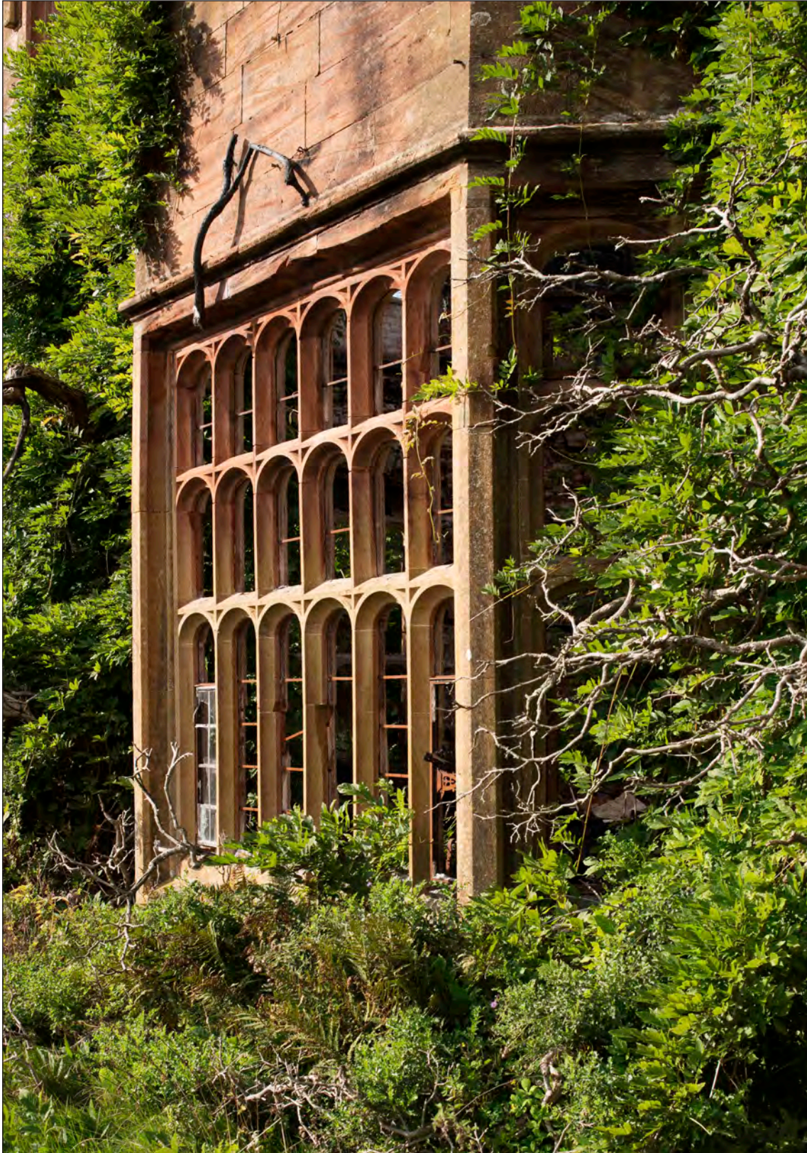
Appendix Two Figure 63: Exterior, south wing, south elevation, detail of bay window, looking north west (DP275953)
