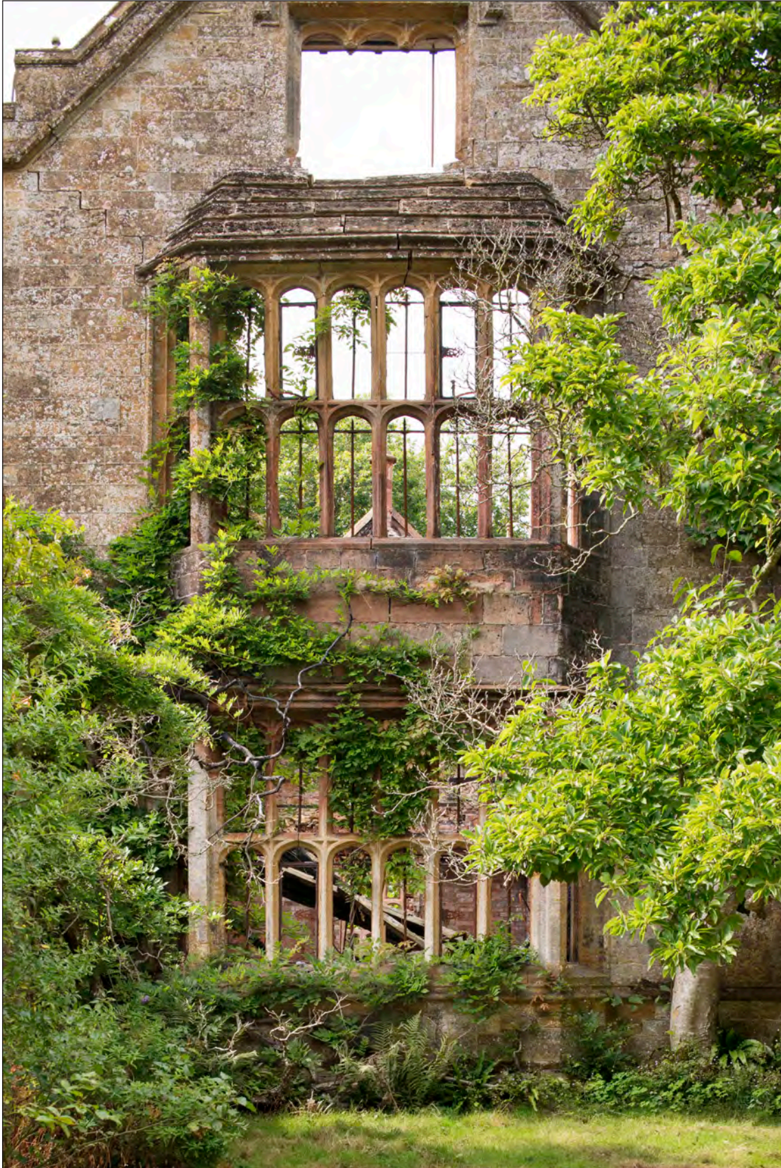
Appendix Two Figure 37: Exterior, south wing, east elevation, detail of bay window (DP275927)
