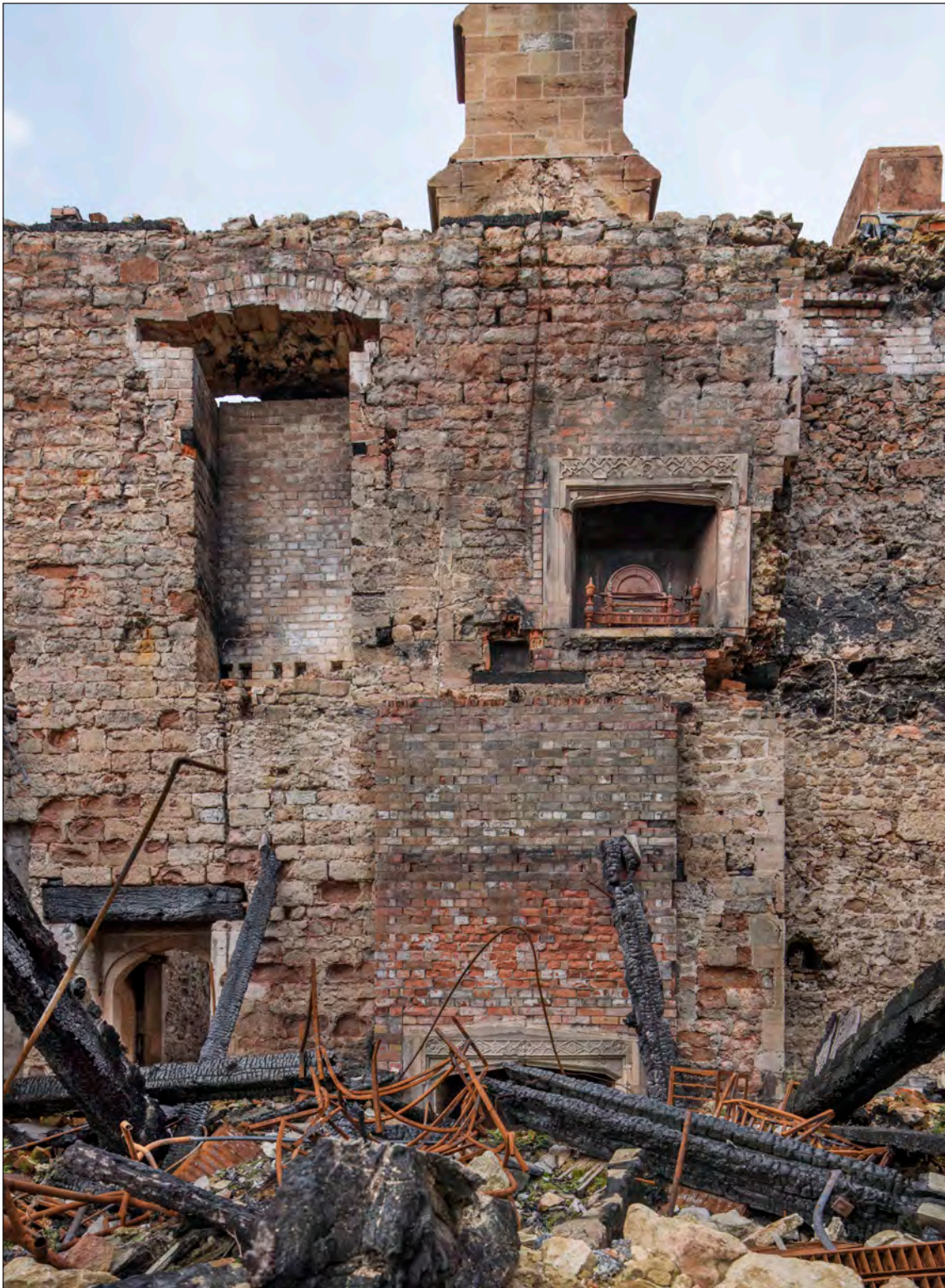
Appendix Two Figure 117: Interior, south wing, eastern portion of north elevation, looking north (DP276007)
