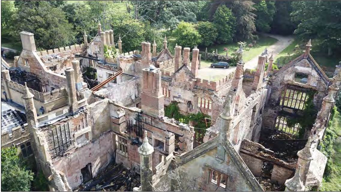
Figure 23 Surviving roof line, showing the pinnacles added by Nash, and the chimney stacks of the same overall form (Drone survey photograph © Historic England)
