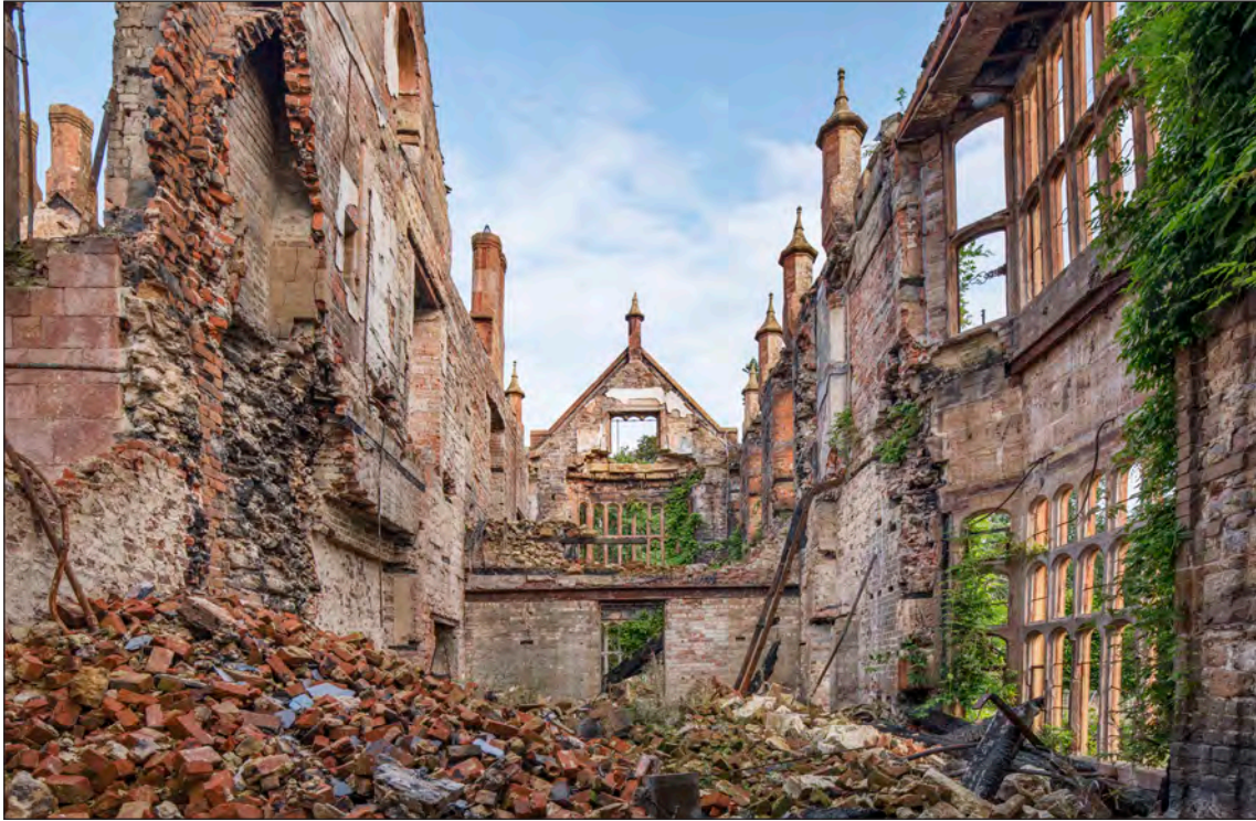
Appendix Two Figure 77: Interior, south wing, looking east (DP275967)
