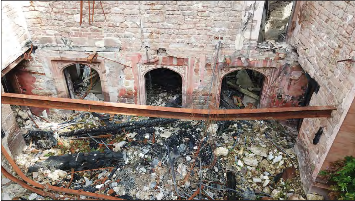
Figure 16 North end of the great hall, showing the service doorways to the north of the original screens passage (Drone survey image © Historic England)
