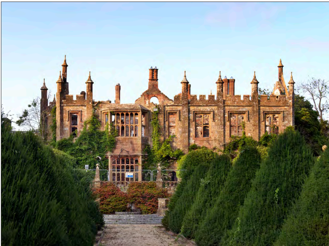
Appendix Two Figure 130: Exterior, south elevation, looking north (DP276020)
