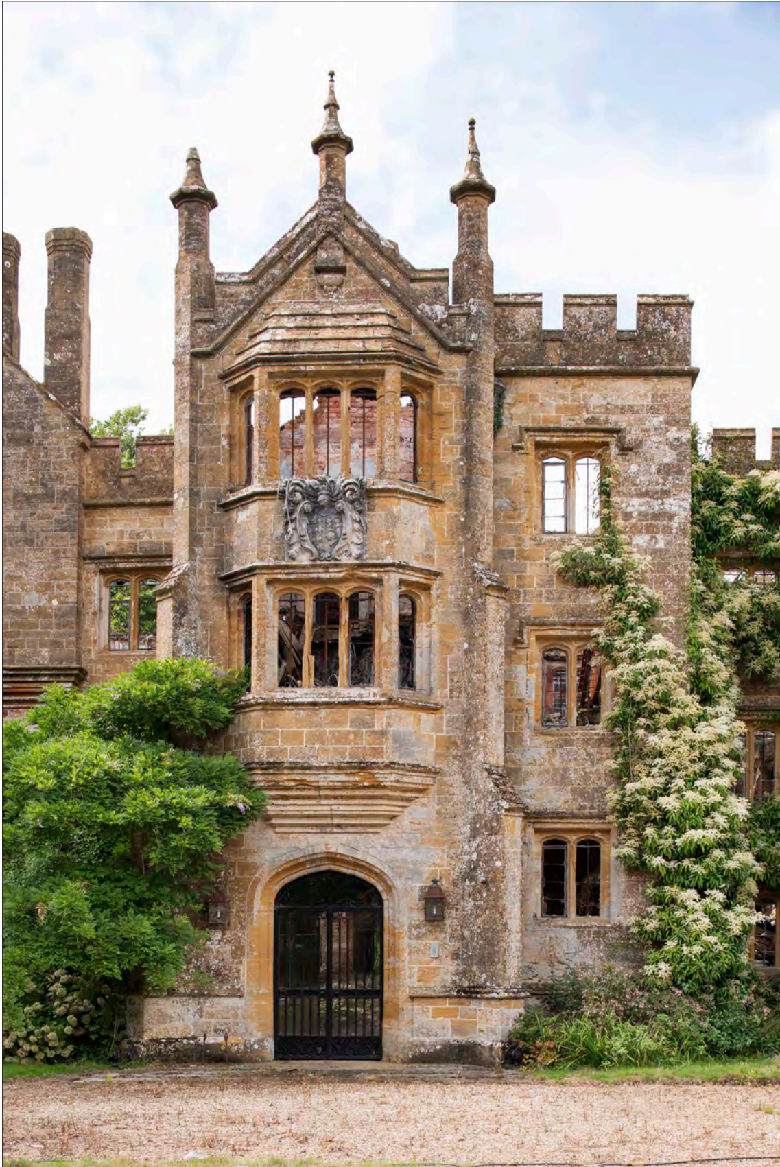
Appendix Two Figure 32: Exterior, north stair and east porch, east elevation, looking west (DP275922)
