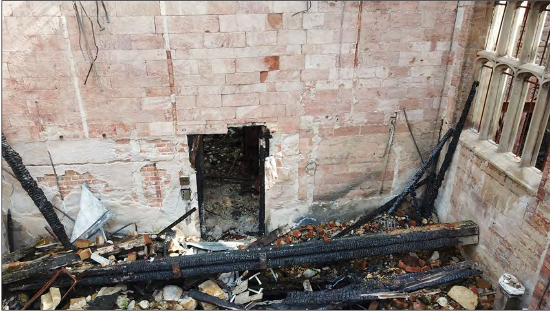
Figure 25 Stonework of the north elevation of the dining room, showing the original ashlar of the west porch to the east of the doorway, and added ashlar carefully pieced in (Drone survey image © Historic England)
