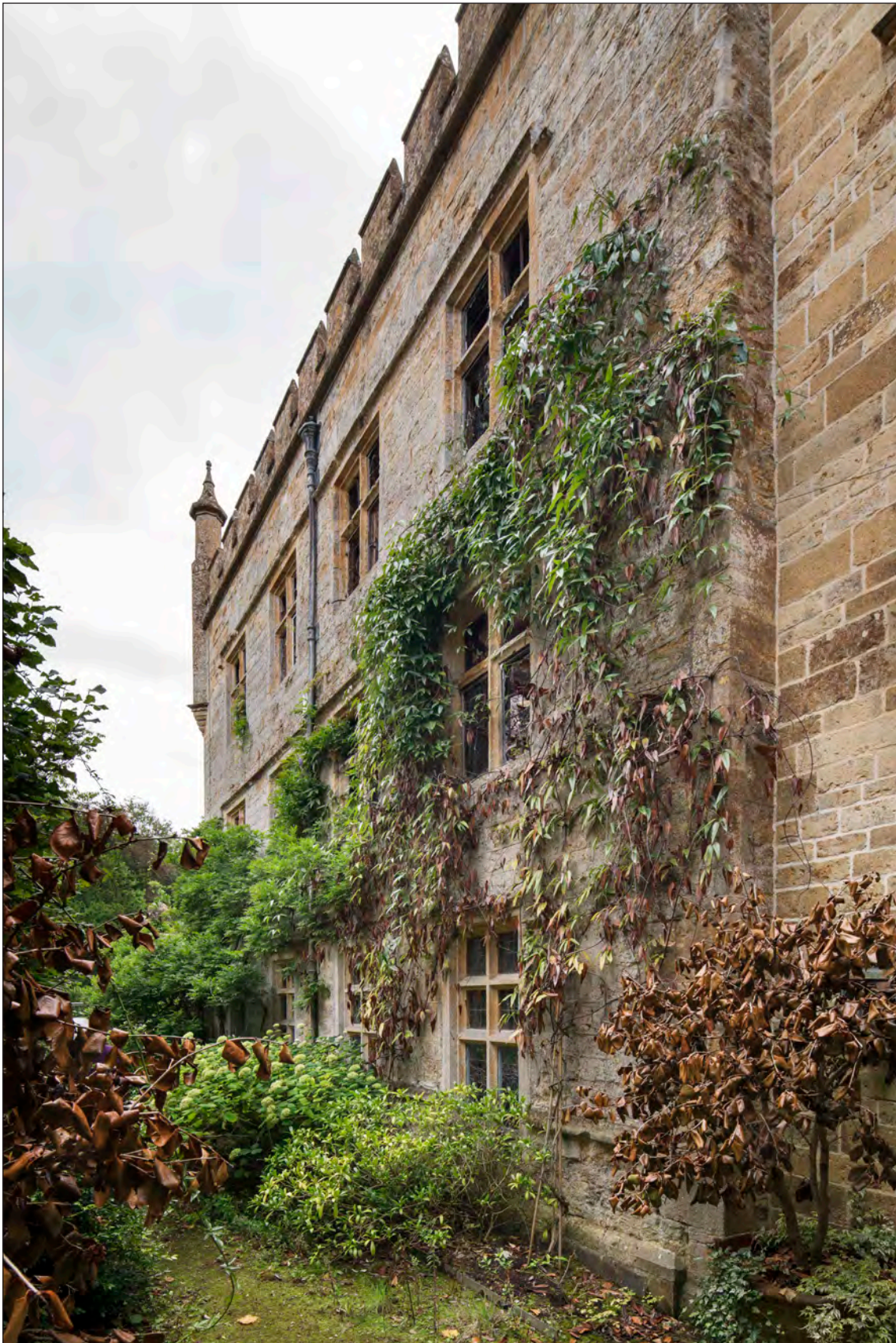
Appendix Two Figure 16: Exterior, north wing, north elevation, looking south east (DP275906)
