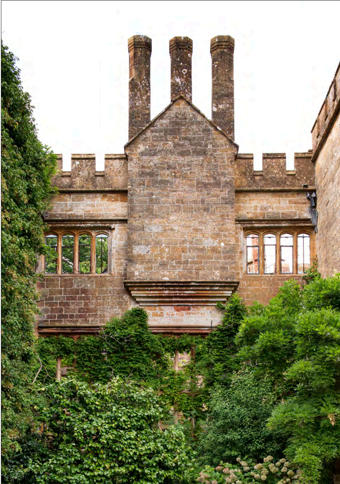
Appendix Two Figure 34: Exterior, main range, hall, east elevation, looking west (DP275924)
