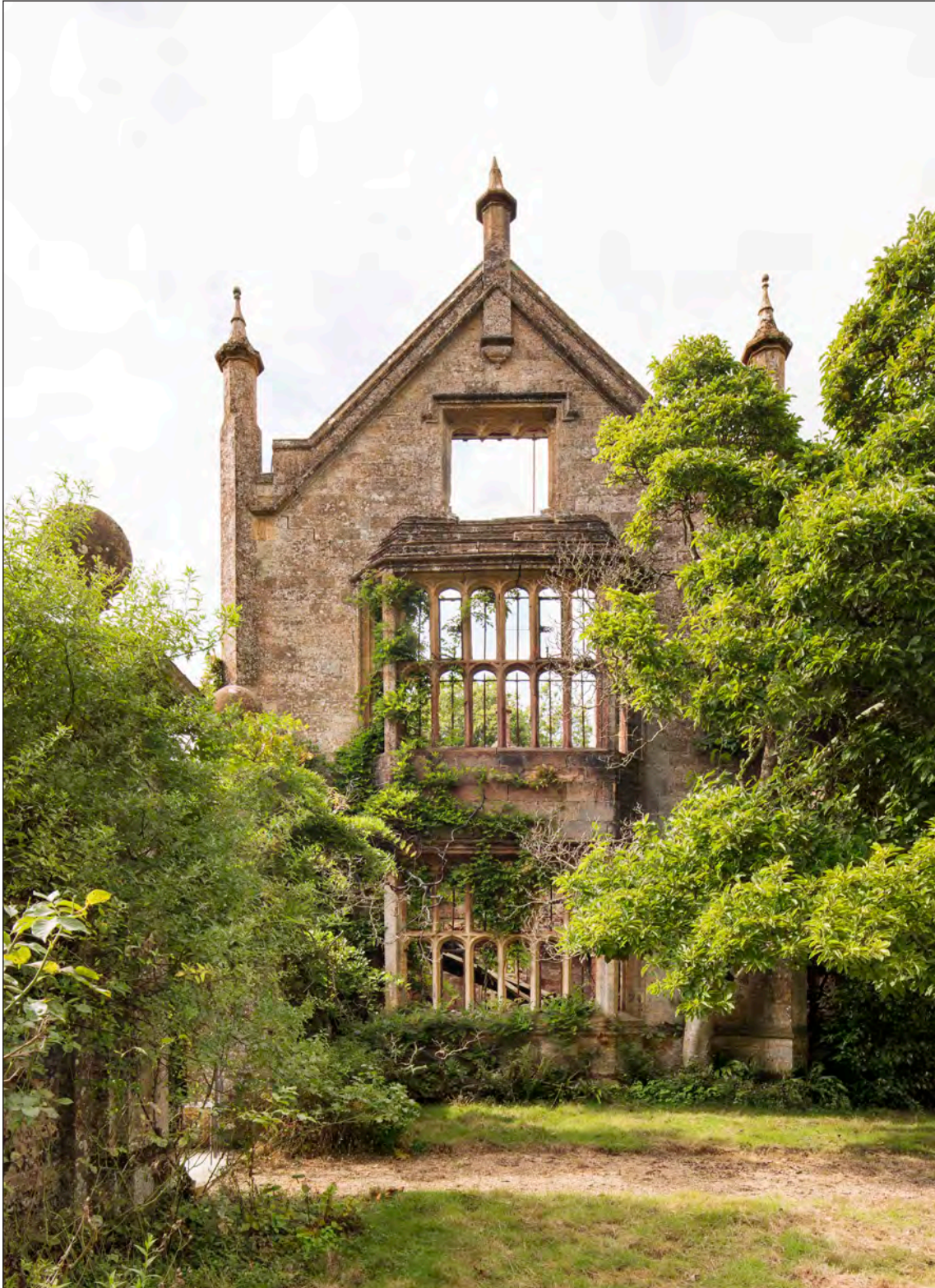
Appendix Two Figure 40: Exterior, south wing, east elevation, looking west (DP275930)
