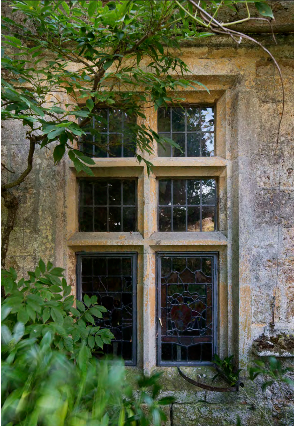
Appendix Two Figure 19: Exterior, north wing, north elevation, detail of eastern ground-floor window, looking south (DP275909)
