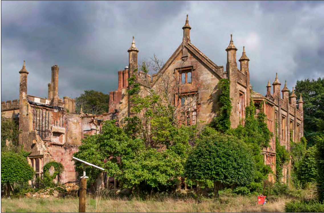
Appendix Two Figure 54: Exterior, south wing and dining room, west and south elevations (DP275944)
