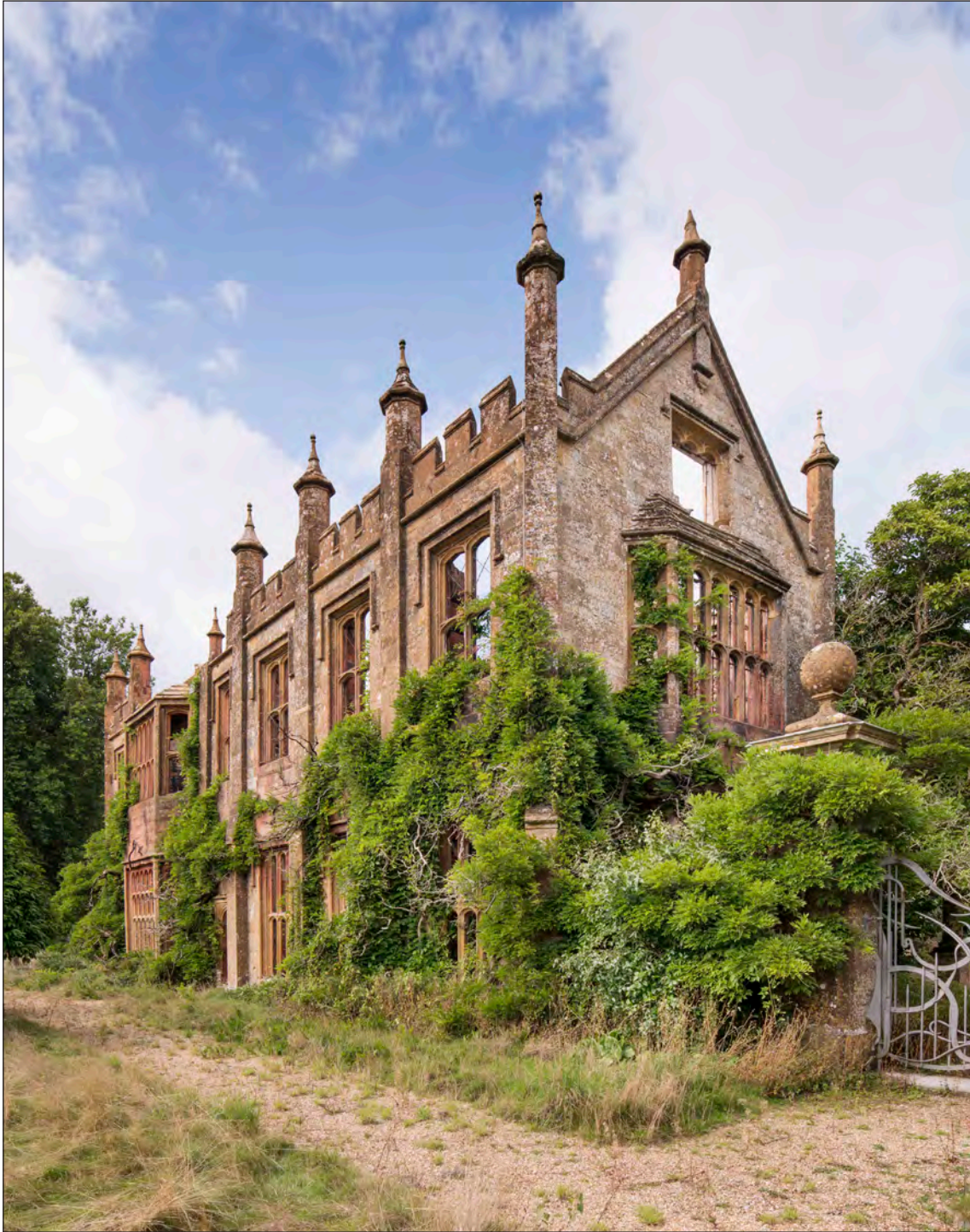
Appendix Two Figure 42: Exterior, south wing, south and east elevations, looking north west (DP275932)
