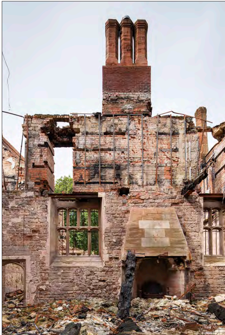
Figure 15 The great hall in the main range, showing the west elevation of the room including the original west window openings (DP275974)
