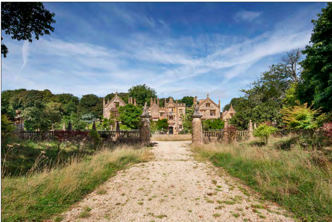
Appendix Two Figure 14: Exterior, east elevation, forecourt and drive, looking west (DP275904)
