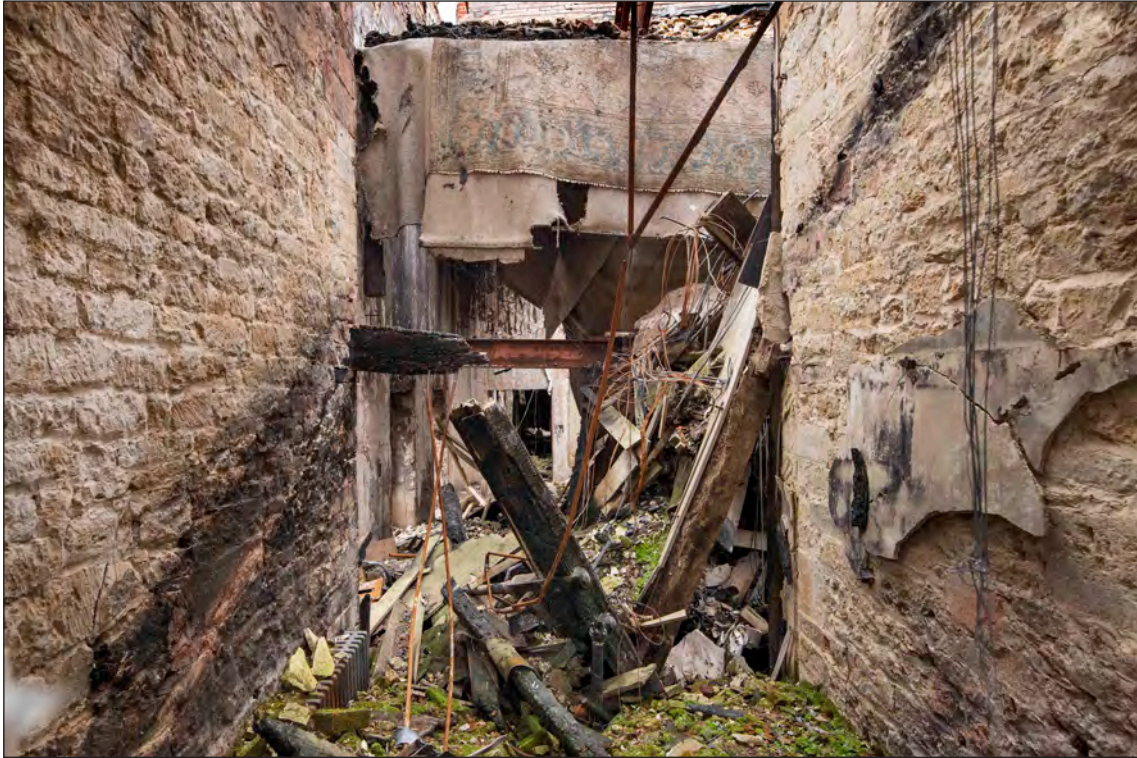
Appendix Two Figure 86: Interior, north stair, looking west (DP275976)
