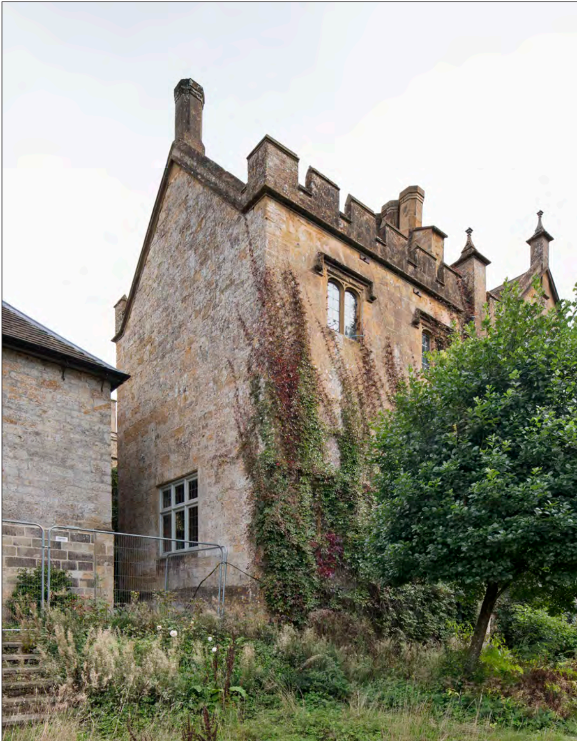
Appendix Two Figure 111: Exterior, service range, north and west elevations, looking south east (DP276001)
