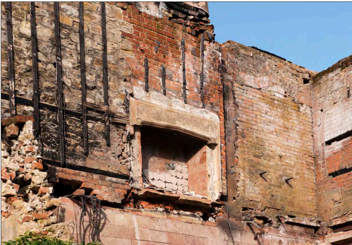
Appendix Two Figure 65: Interior, first floor over dining room, north elevation, looking north east (DP275955)
