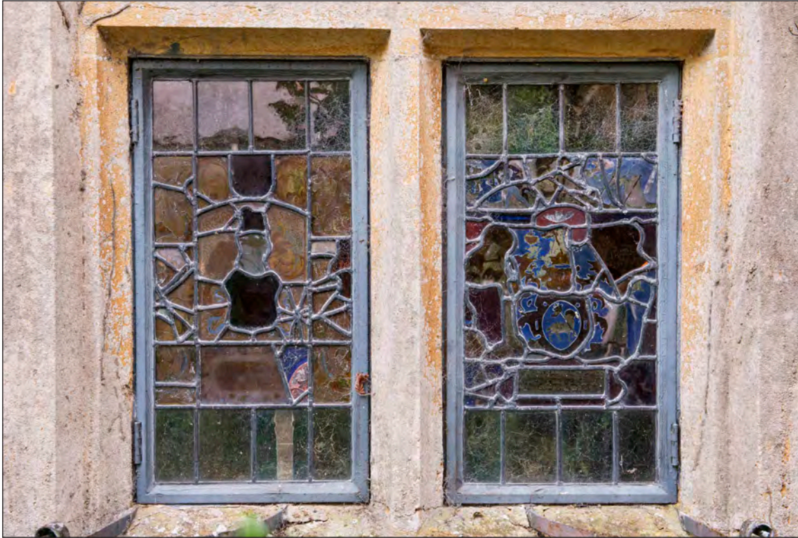
Appendix Two Figure 104: Exterior, north wing, north elevation, detail of stained glass in western ground-floor window, looking south (DP275994)
