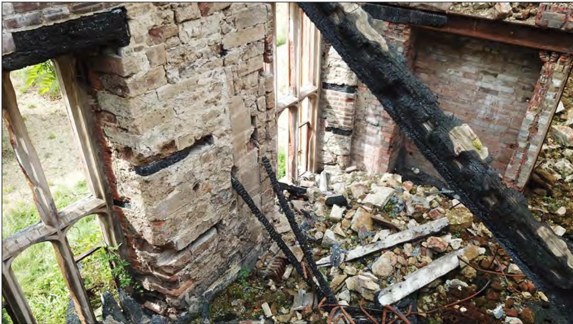
Figure 18 The south wall of the south wing, showing residual jamb from an original window opening between two of Nash's inserted windows (Drone survey image © Historic England)
