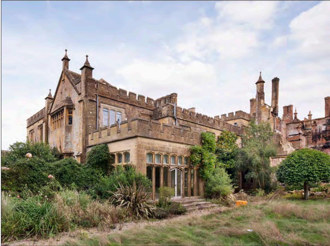
Appendix Two Figure 123: Exterior, service range and orangerie, west and south elevations, looking north east (DP276013)
