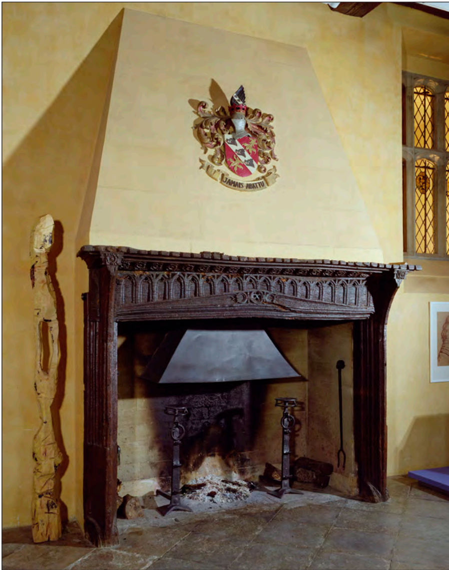
Figure 24 Fireplace in the great hall photographed in 1999 (HEA BB99/04437)
