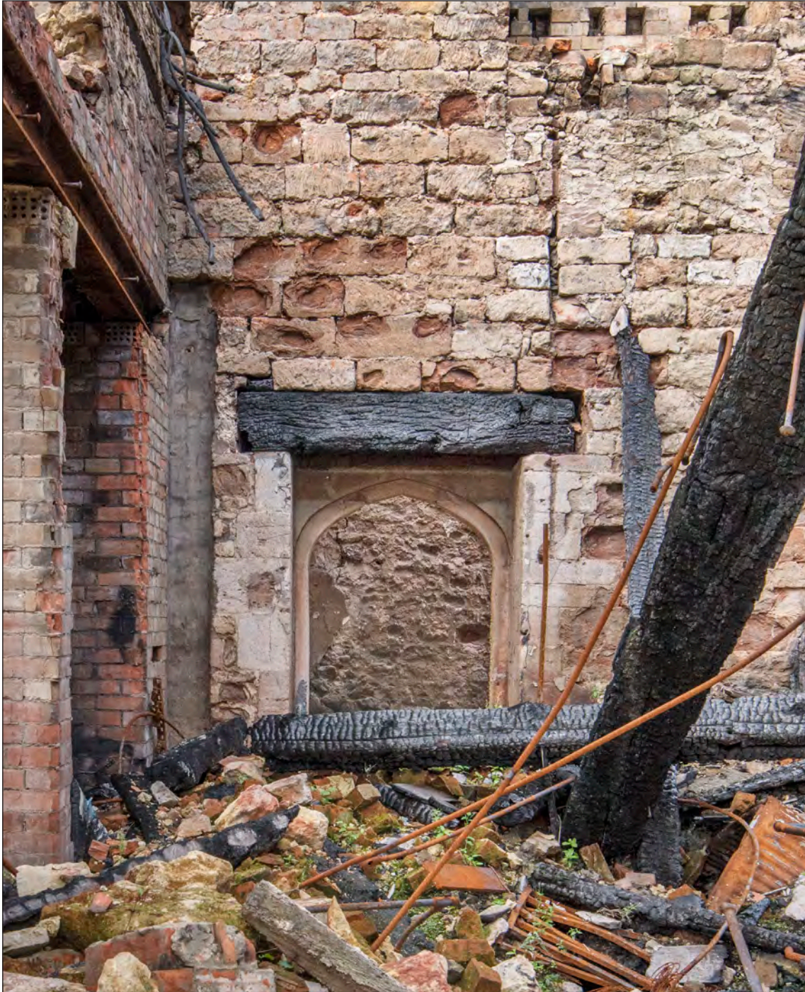
Appendix Two Figure 120: Interior, south wing, central portion of north elevation, detail of door to south stair, looking north (DP276010)
