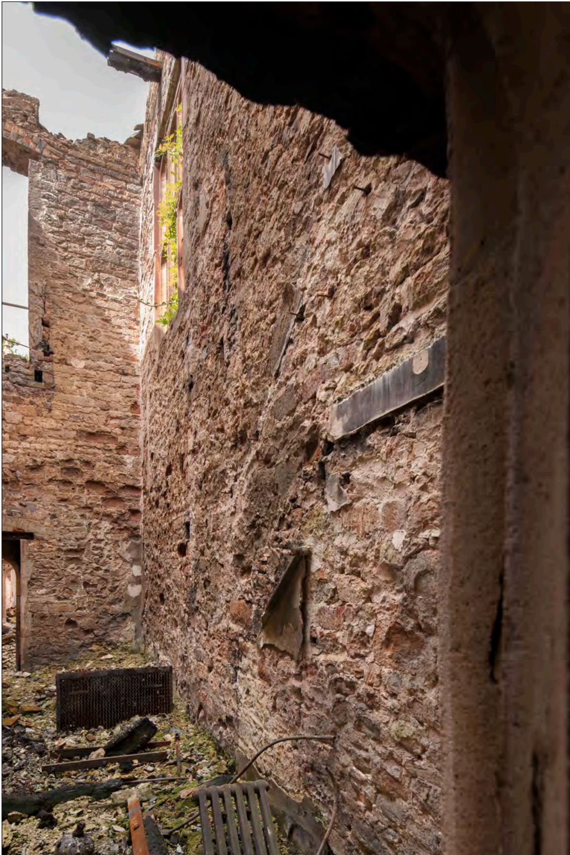
Appendix Two Figure 83: Interior, south stair, looking north west (DP275973)
