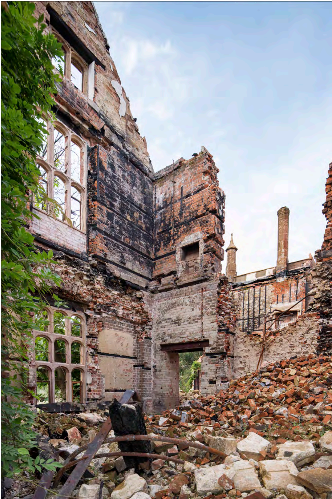
Appendix Two Figure 122: Interior, south wing, north and west elevations, looking north west (DP276012)
