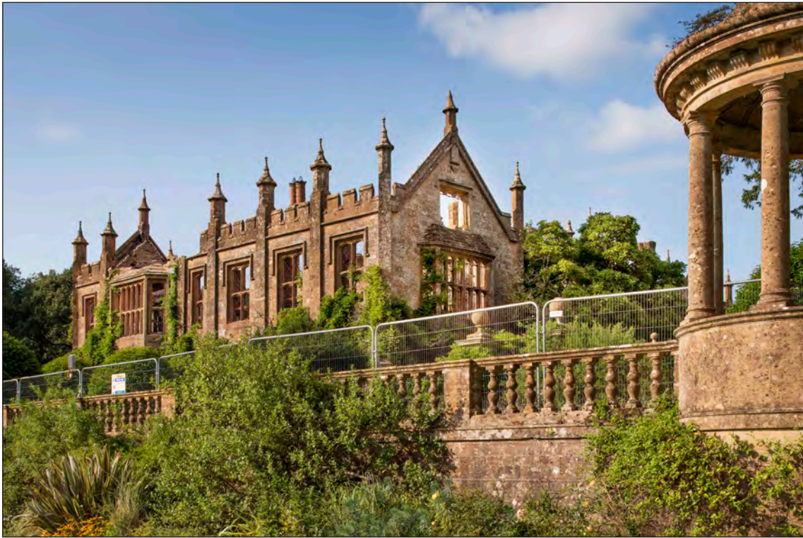
Appendix Two Figure 62: Exterior, south wing, south and east elevations and south terrace, looking north west (DP275952)
