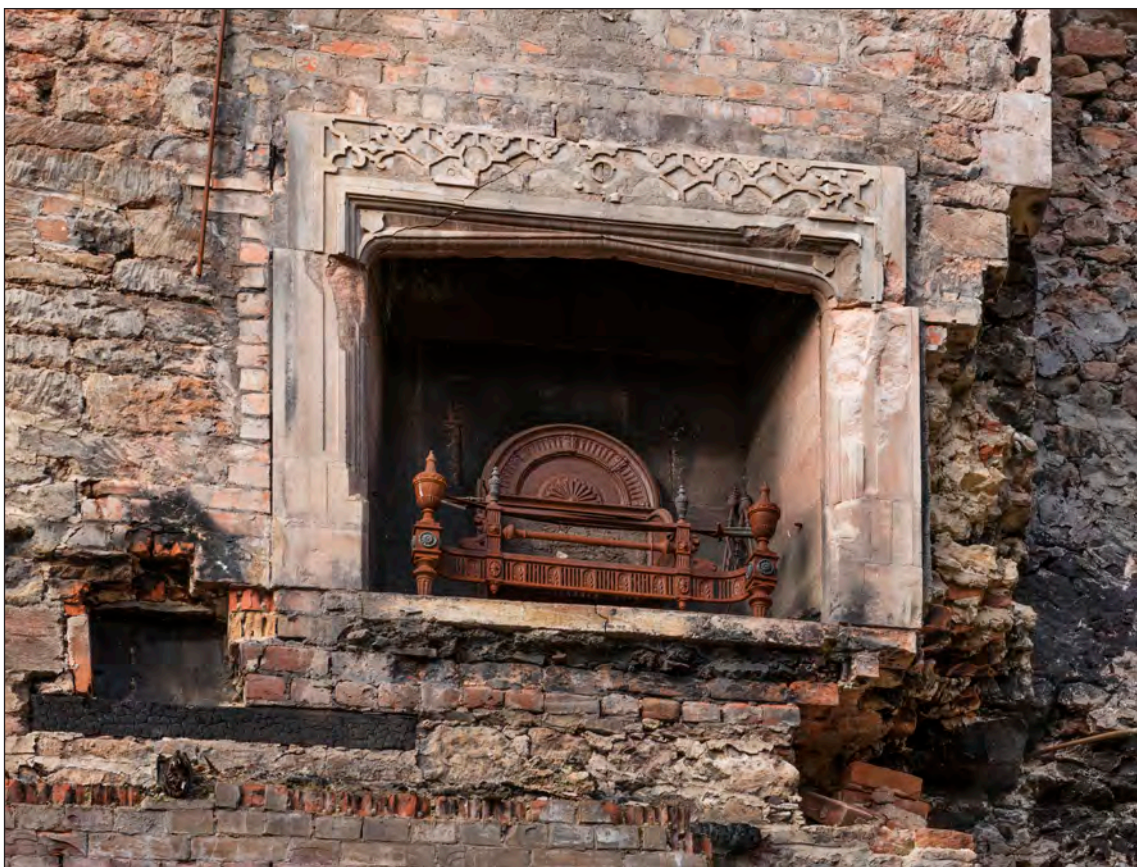
Appendix Two Figure 69: Interior, south wing, first-floor east room, showing detail of fireplace, looking north (DP275959)
