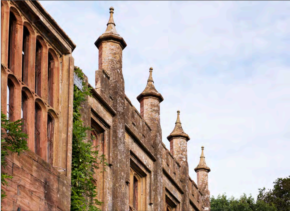
Appendix Two Figure 75: Exterior, south wing, south elevation, detail of parapet, looking north east (DP275965)
