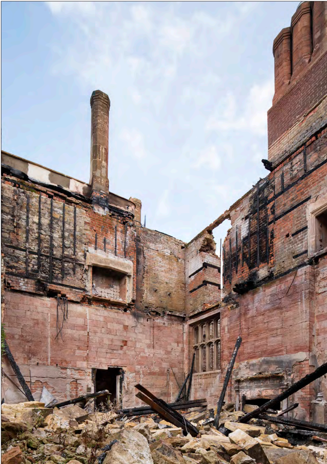
Appendix Two Figure 124: Interior, dining room, north and east elevations, looking north east (DP276014)
