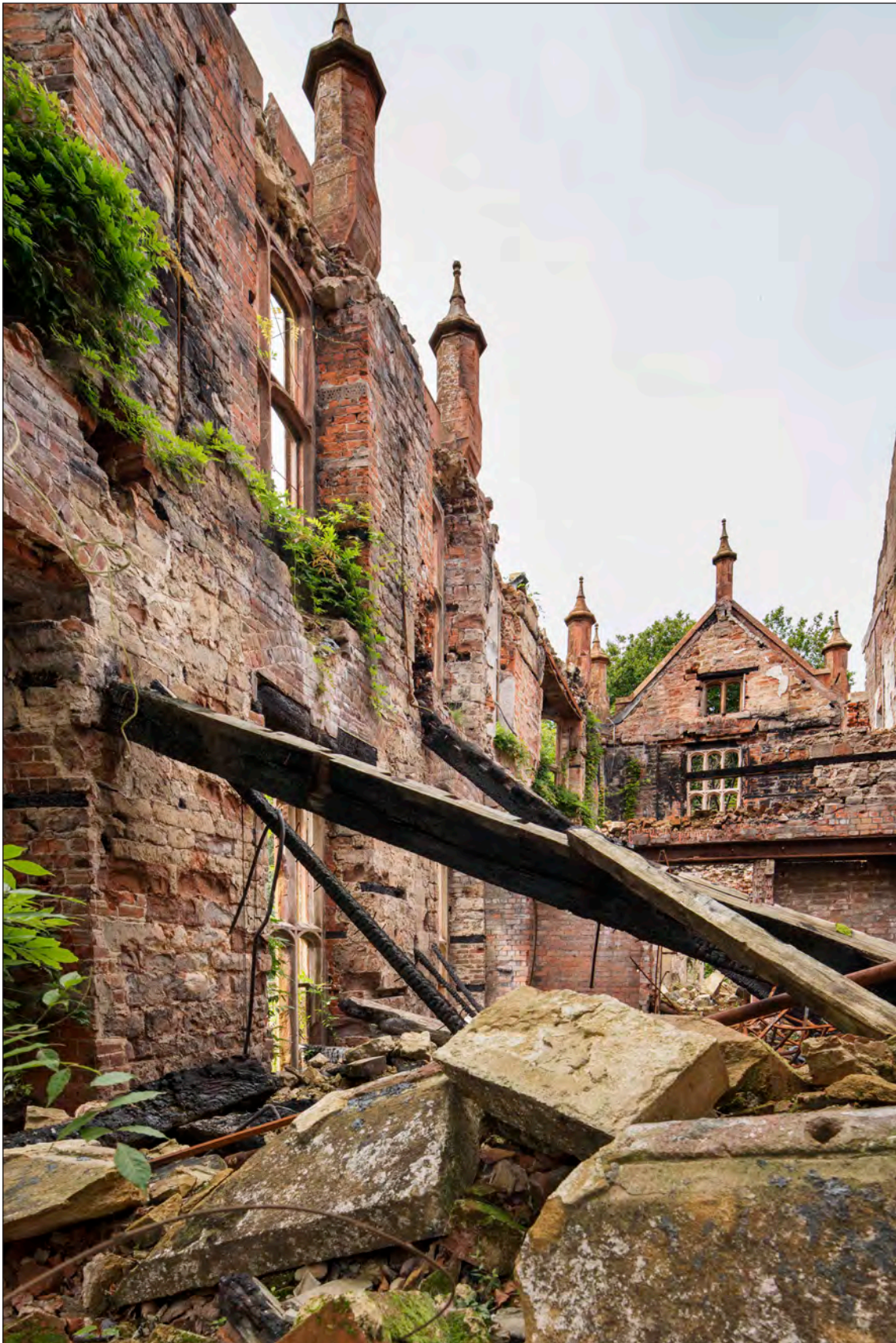
Appendix Two Figure 81: Interior, south wing, south elevation, looking south west (DP275971)
