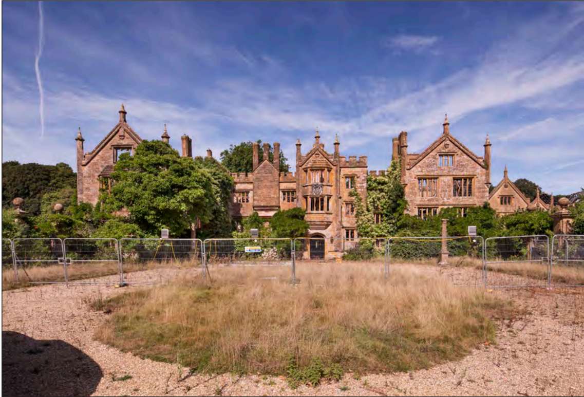
Appendix Two Figure 13: Exterior, east elevation and forecourt, looking west (DP275903)
