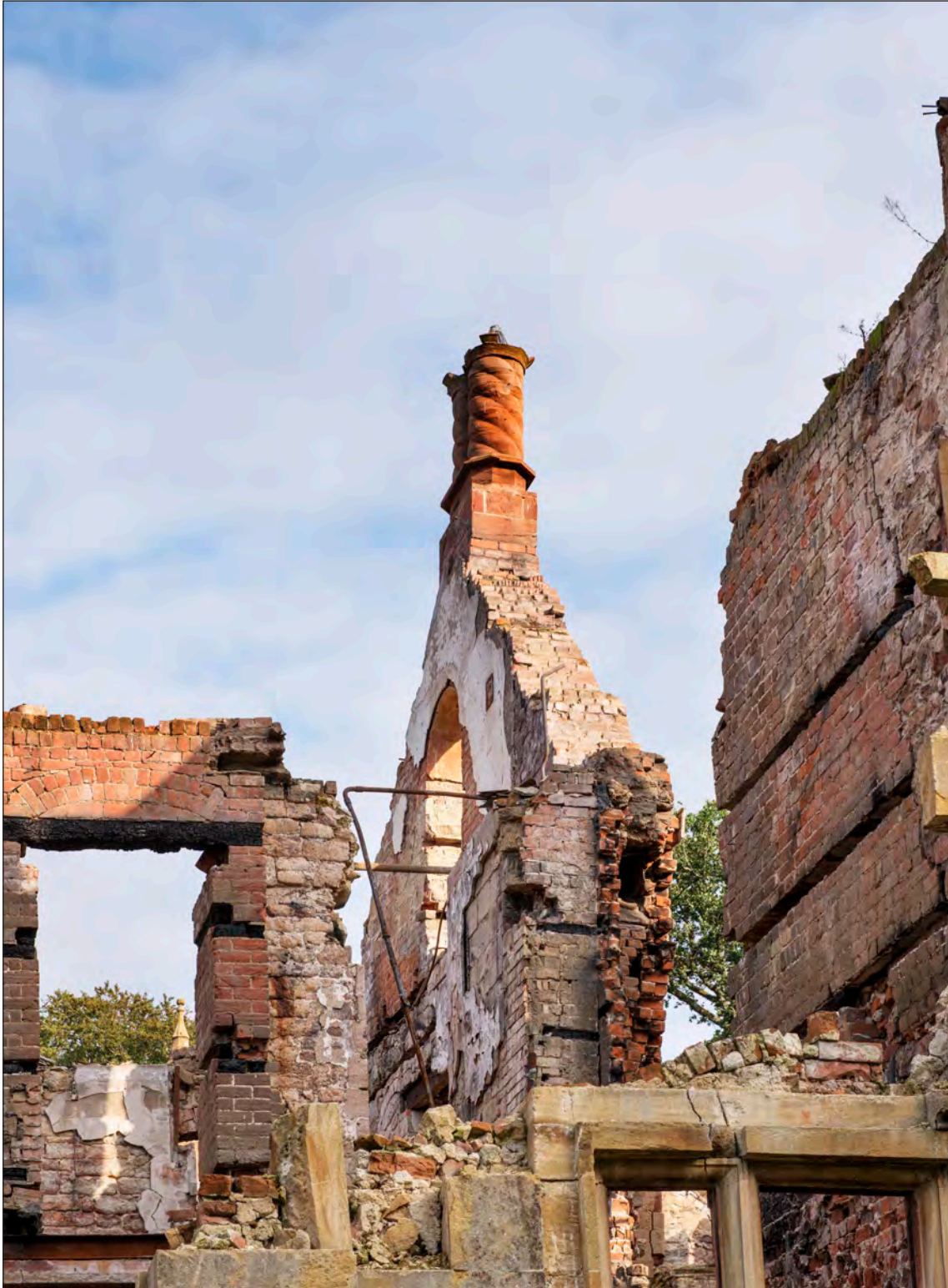
Appendix Two Figure 74: Interior, main range, south elevation and junction with south wing, looking south east (DP275964)
