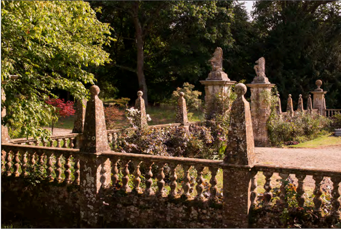
Appendix Two Figure 59: Forecourt, looking southeast (DP275949)
