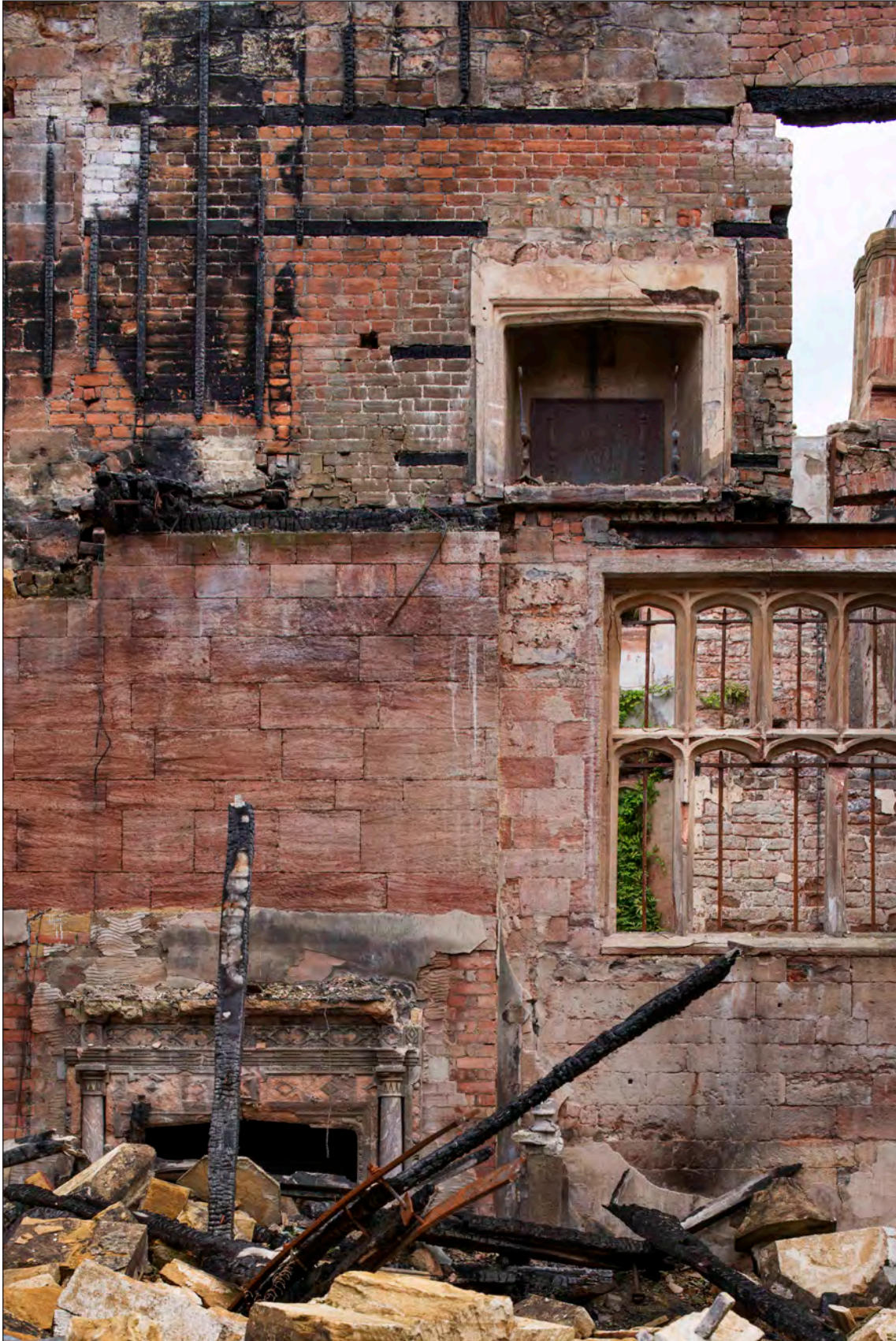
Appendix Two Figure 56: Interior, dining room, east elevation, looking east (DP275946)
