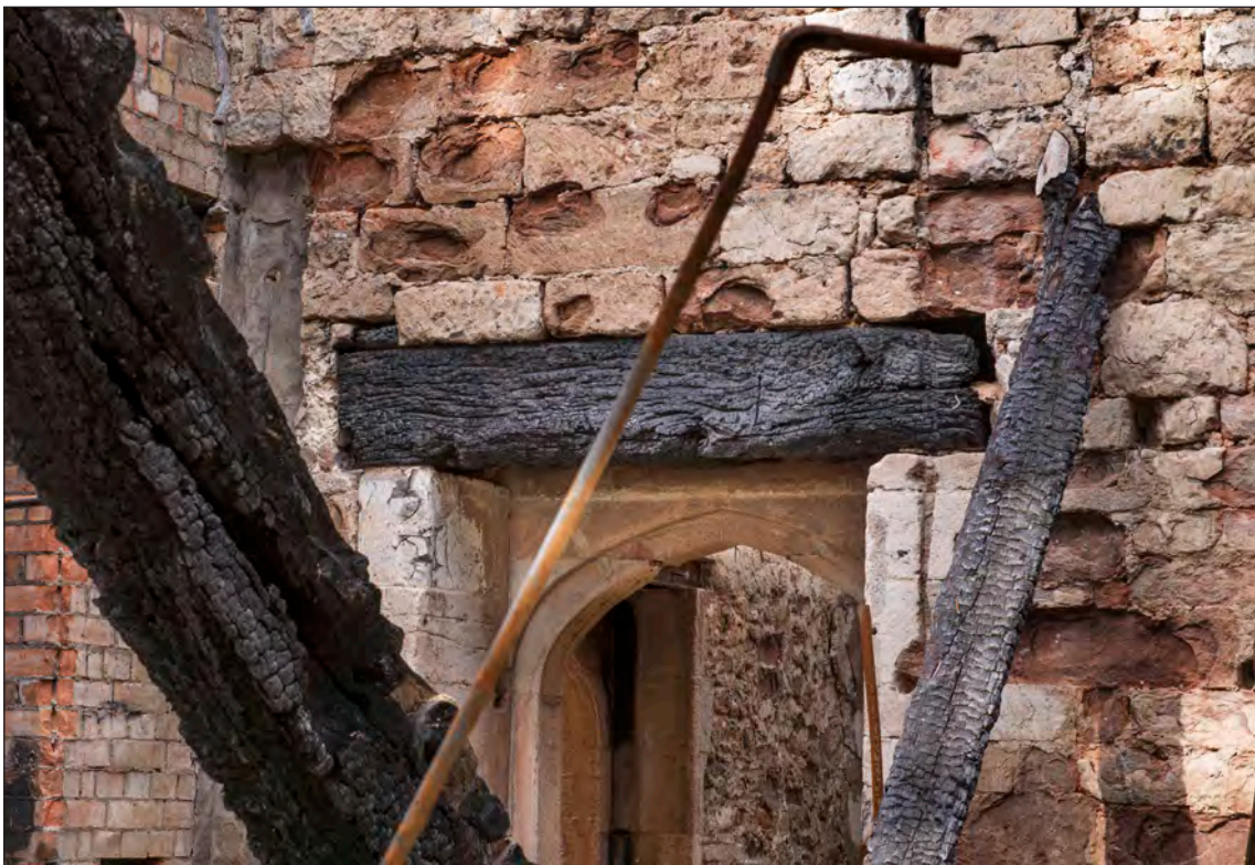
Appendix Two Figure 107: Interior, south wing, north elevation, detail of doorway to south stair, looking north (DP275997)
