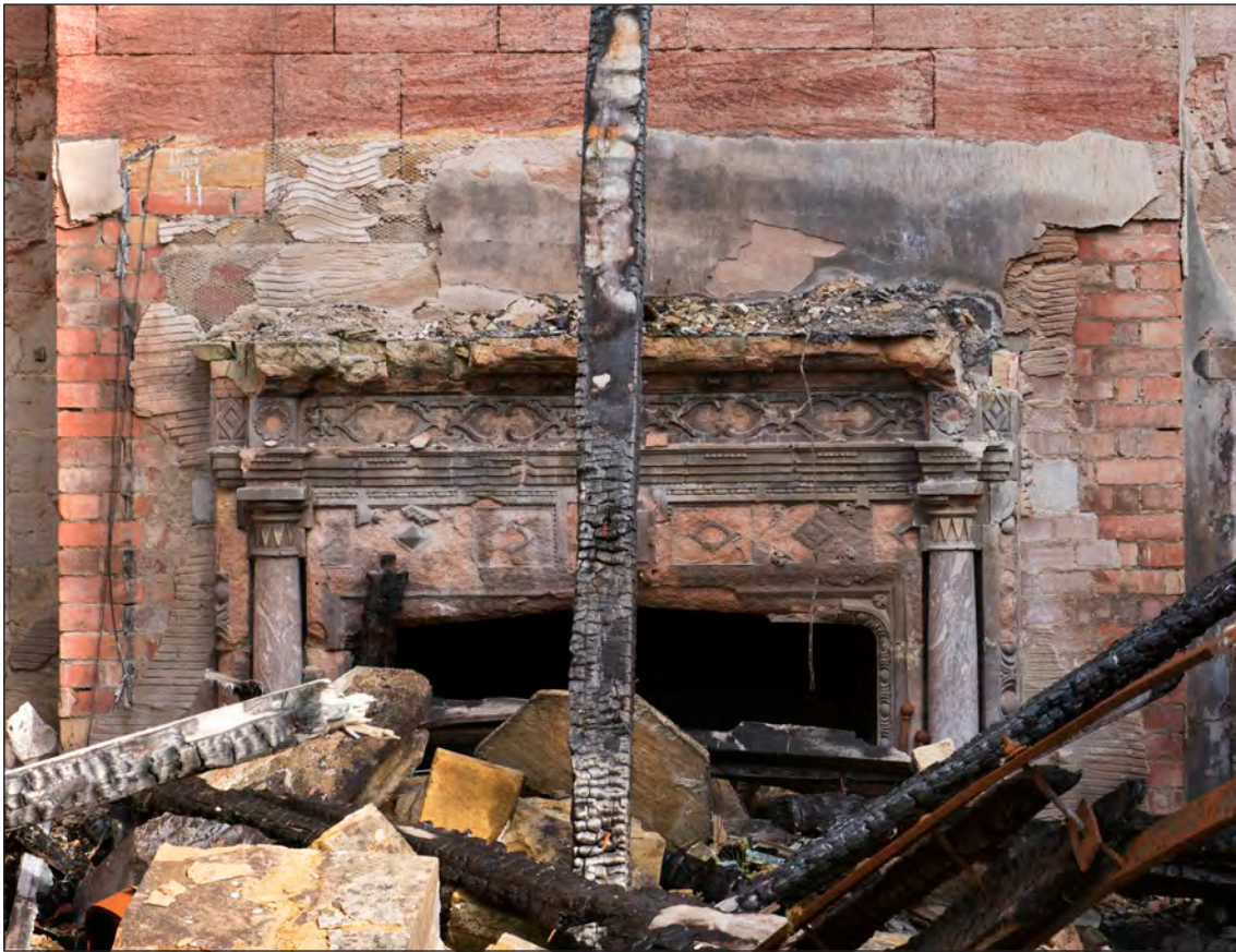
Appendix Two Figure 64: Interior, dining room, detail of fireplace, looking east (DP275954)
