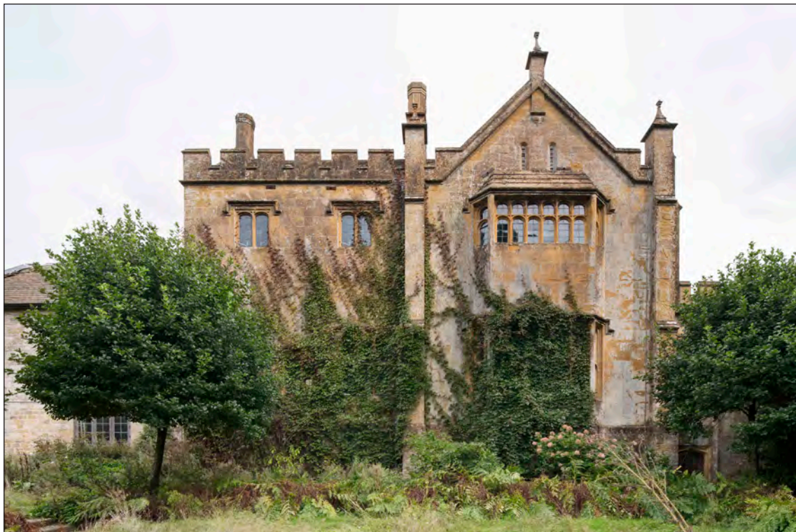
Appendix Two Figure 110: Exterior, service range, west elevation, looking east (DP276000)
