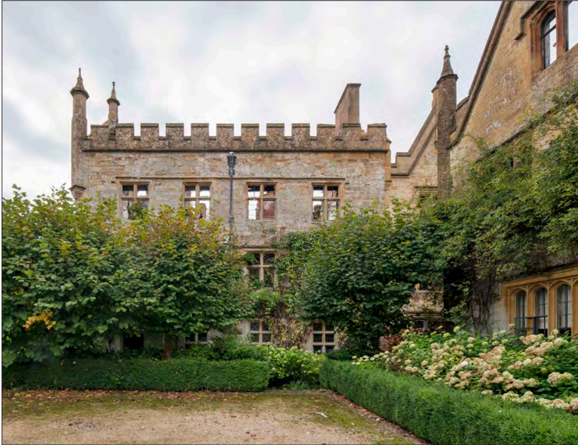
Appendix Two Figure 15: Exterior, north wing, north elevation, looking south (DP275905)
