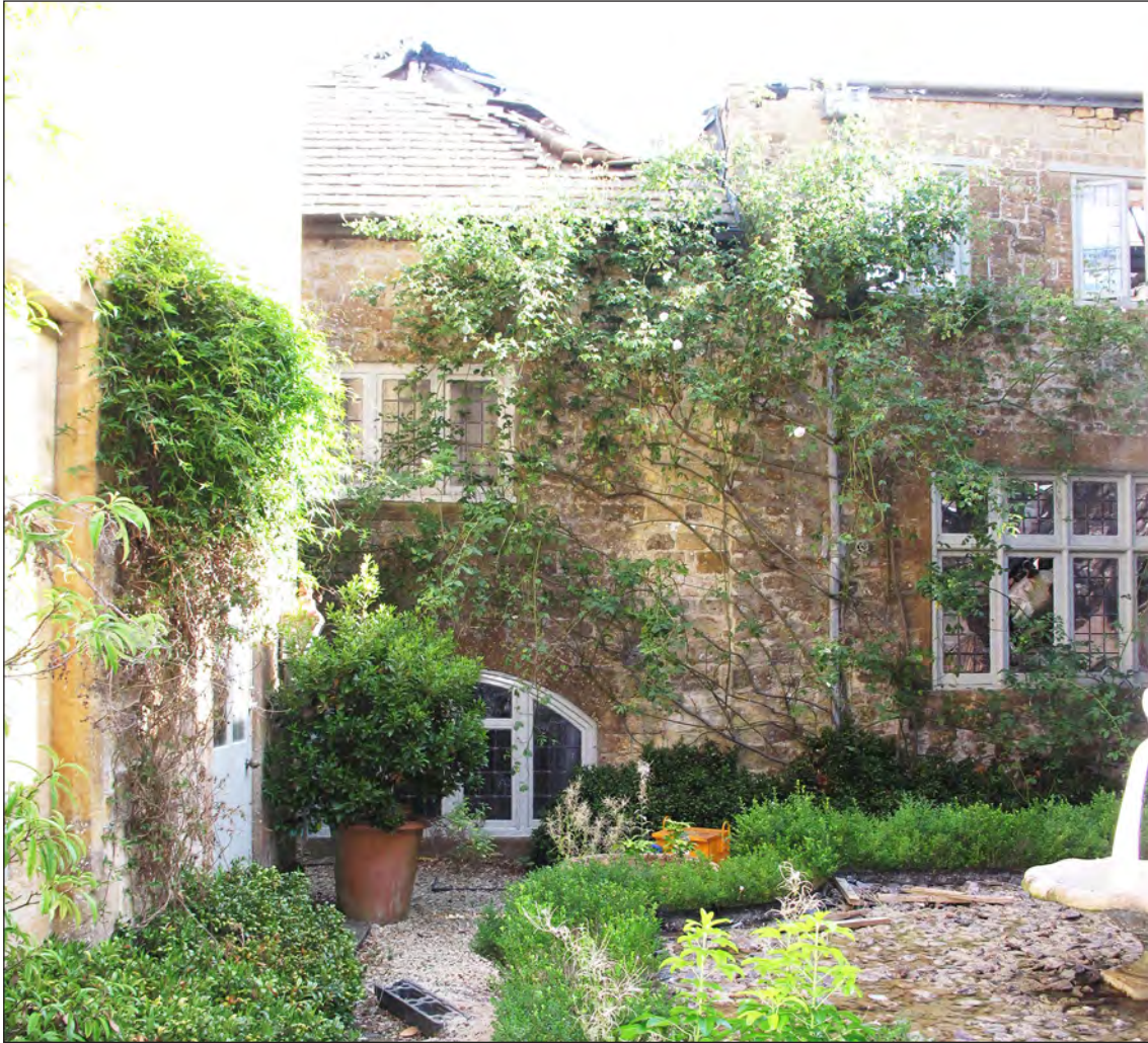
Figure 27 South wall of the stable block from the service courtyard, showing the junction of the east and west ranges of the block (Investigator photograph © Historic England)
