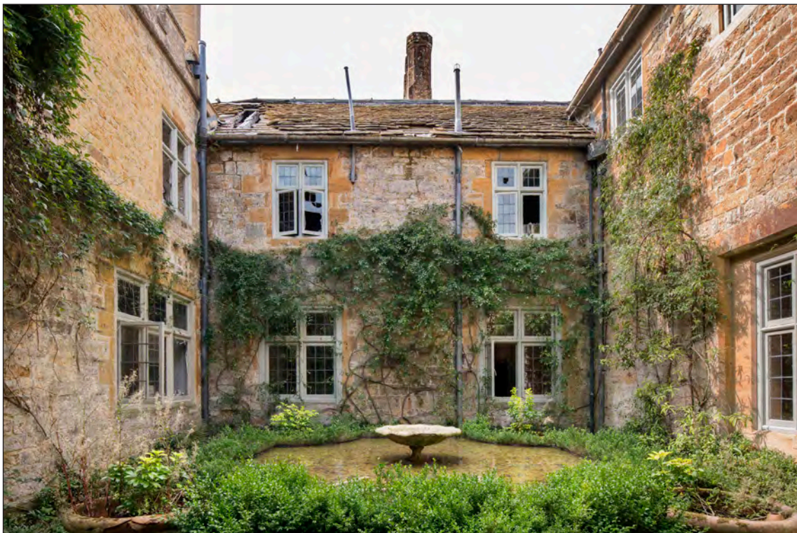
Appendix Two Figure 78: Exterior, service courtyard, service range, north elevation, looking south (DP275968)
