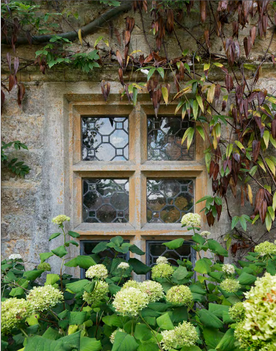
Appendix Two Figure 18: Exterior, north elevation, north wing, detail of central ground-floor window, looking south (DP275908)
