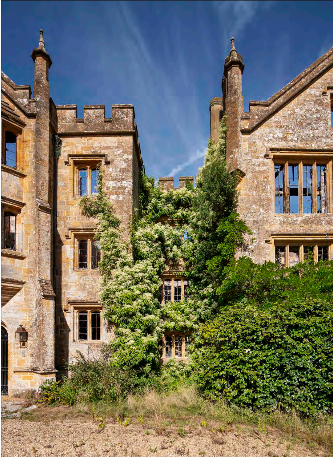
Appendix Two Figure 10: Exterior, north stair and main range, east elevation, looking west (DP275900)
