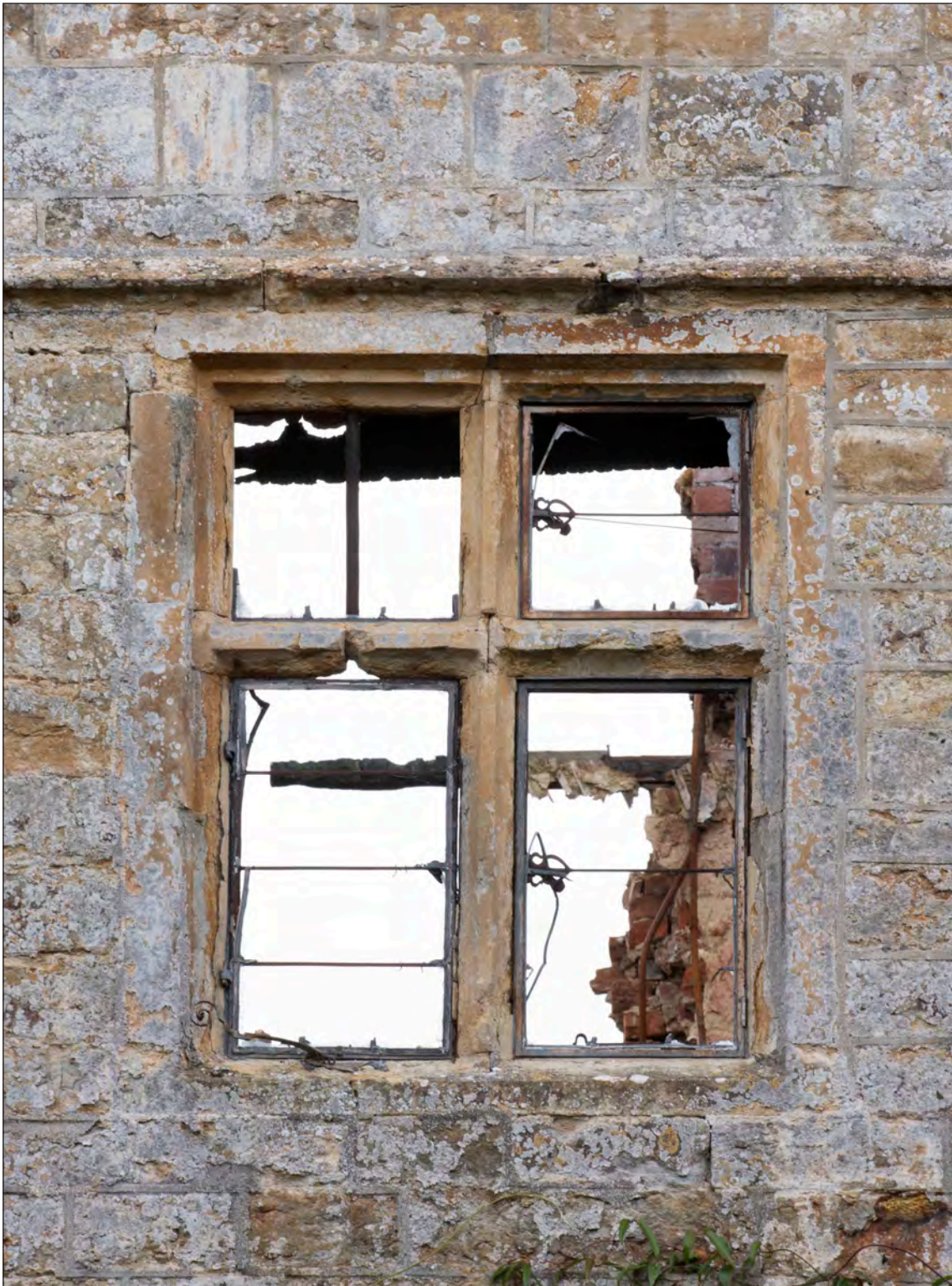
Appendix Two Figure 23: Exterior, north wing, north elevation, detail of second-floor window, second window from west, looking south (DP275913)
