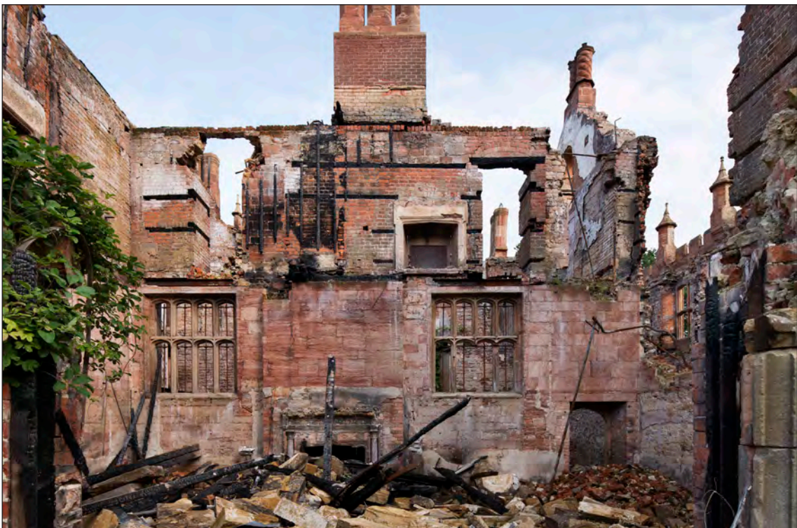
Appendix Two Figure 76: Interior, dining room, west elevation, looking east (DP275966)
