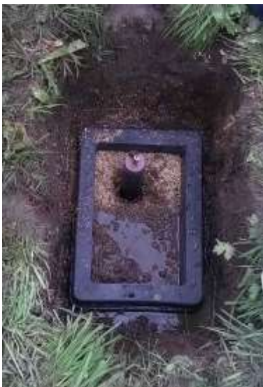
Figure 97 Monitoring site being installed
