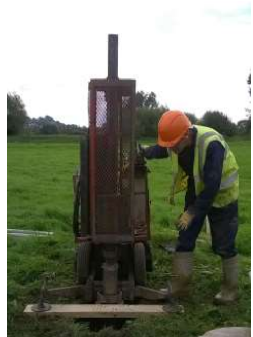
Figure 96 Installation of the new monitoring equipment
