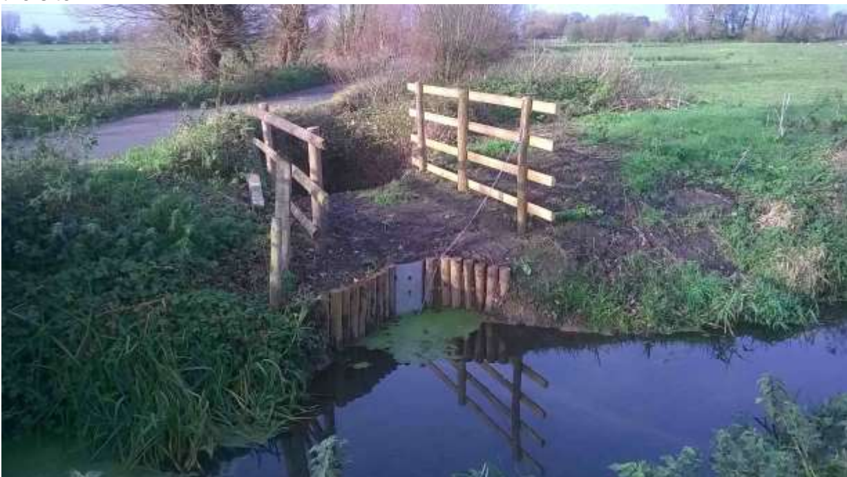
Figure 93 The new inlet to ditch on the western side of the site. Great Withy Rhyne in the foreground
