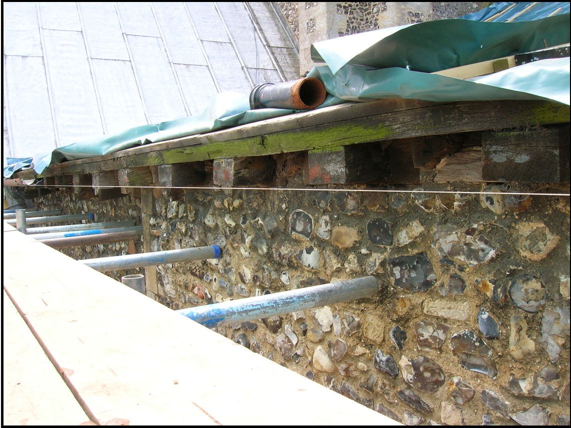
Figure 7: North chapel roof, showing ends of timbers
