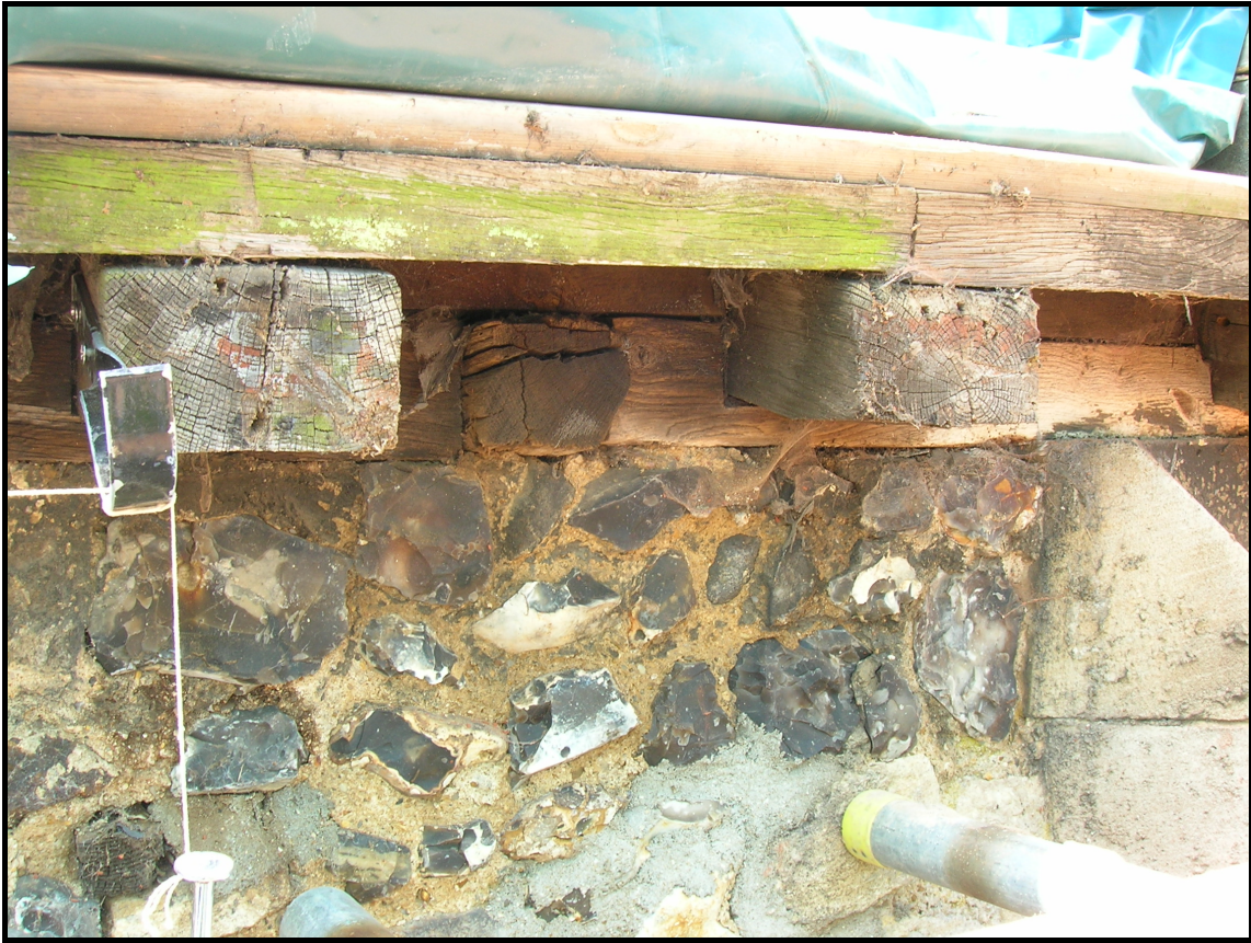
Figure 8: North chapel, exposed timbers, in addition to the main 'joists' are a number of smaller timbers (A)
