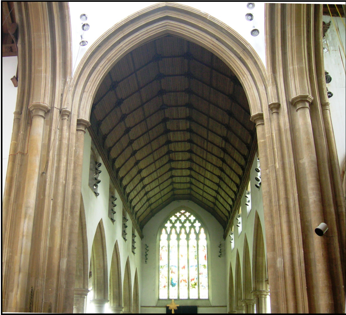
Figure 5: The nave ceiling, as viewed from below
