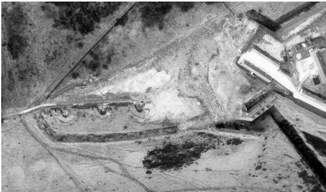
Figure 5 Citadel Battery in 1966 after the Western Outworks ditch had been partially filled in (NMR: MAL/66081/102 )
