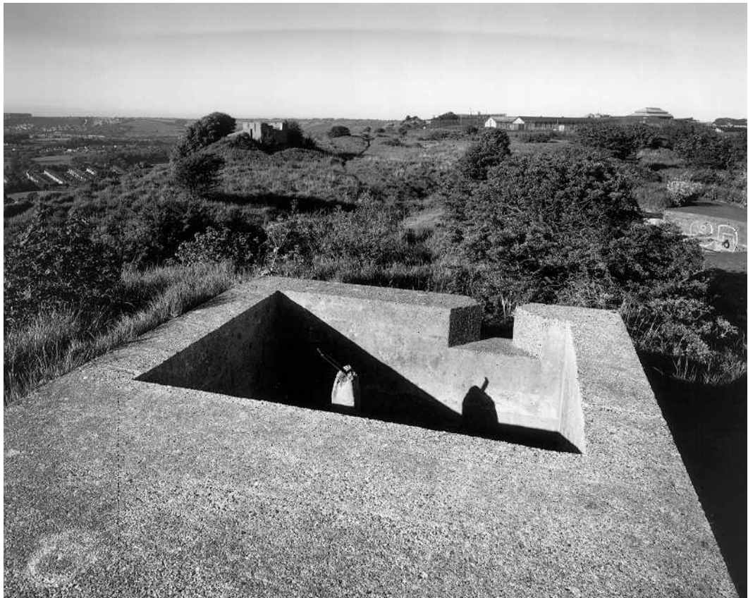
Figure 17 View across Citadel Battery from the top of pillbox 1; in the foreground is the pit for the light anti-aircraft gun (NMR: AA99/09729 © Crown Copyright 1999)
