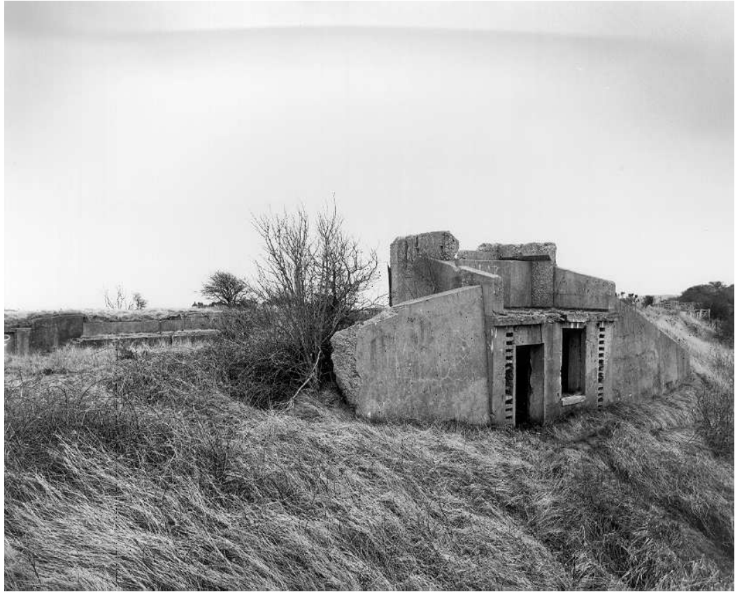
Figure 14 The second Battery Command Post from the rear, showing the telephone room below and the DRF position above (NMR: AA99/09740 © Crown Copyright 1999)
