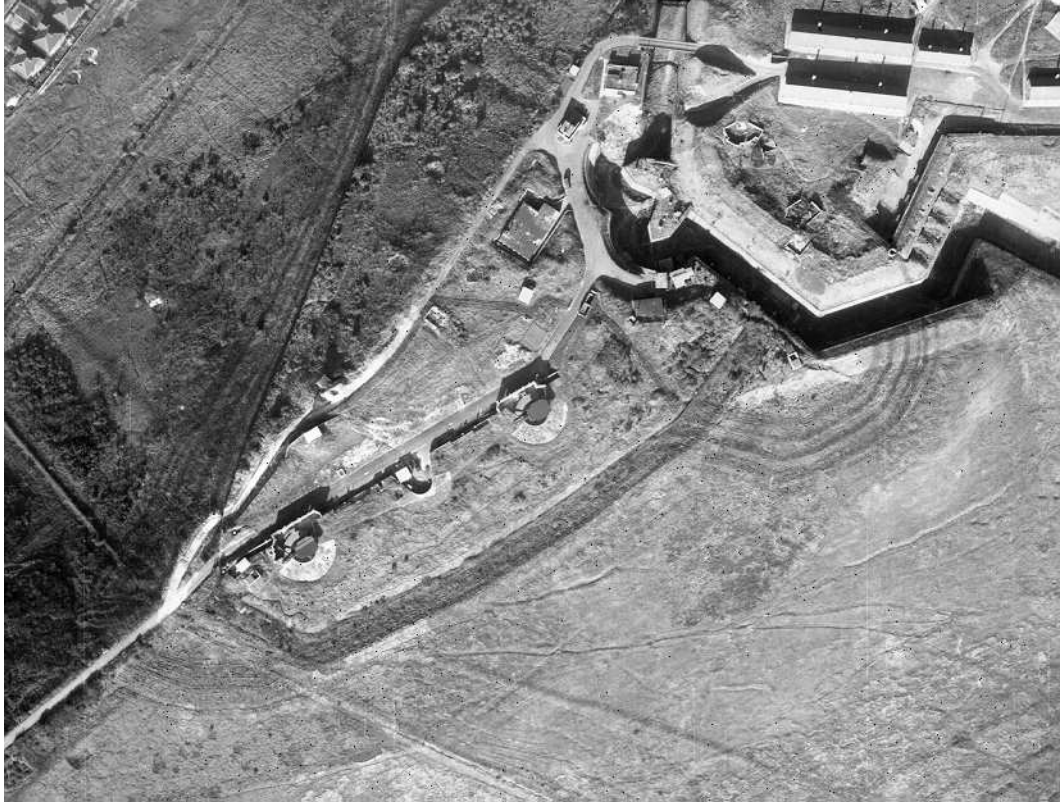
Figure 4 Citadel Battery in 1945 (NMR: 106G/UK/944/Part II/6097) © MOD by kind permission
