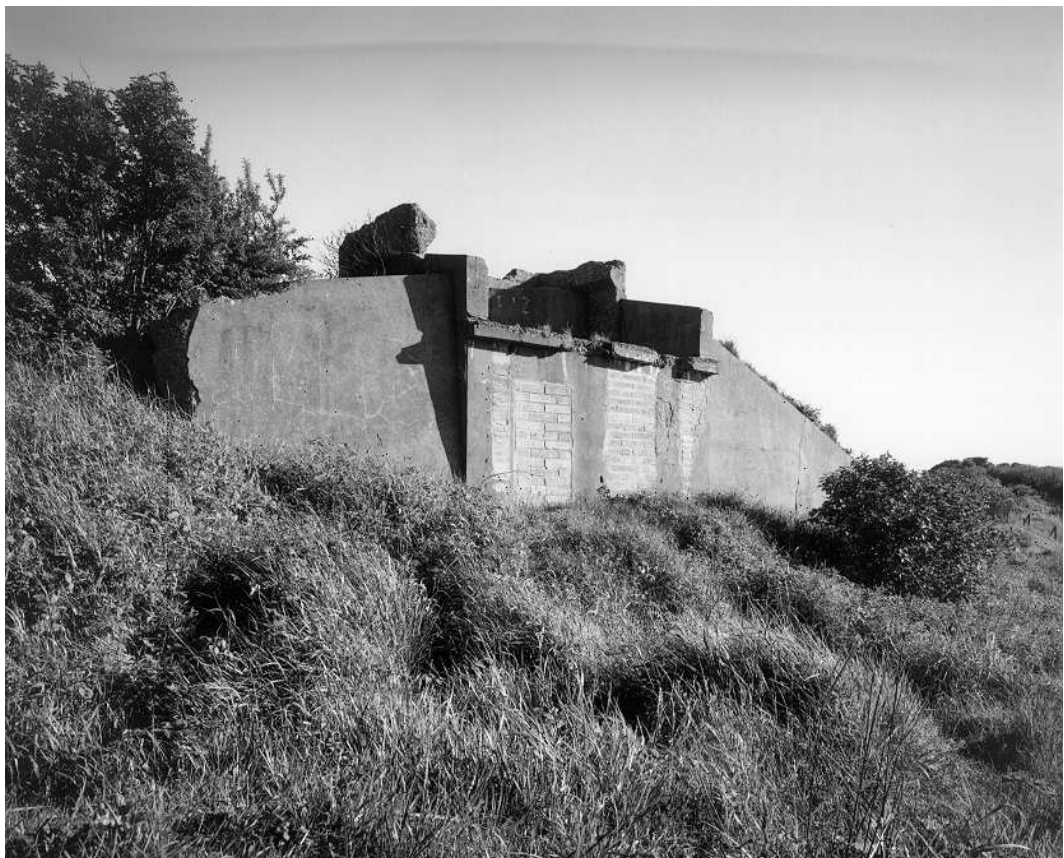
Figure 16 The second Battery Command Post, showing the blocking of the telephone room (NMR: AA99/09735 © Crown Copyright 1999)
