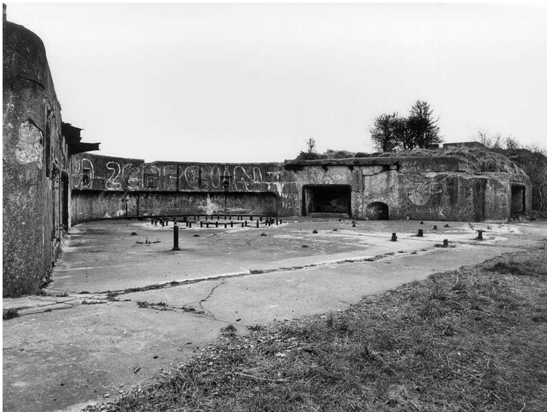
Figure 9 Emplacement for gun no 1, showing the gun floor with holdfast and sawn-off uprights for the steel loading platform and the barbette with shell recess, cartridge recess and tunnel to the hydraulic accumulator (NMR: AA99/19743© Crown Copyright 1999)
