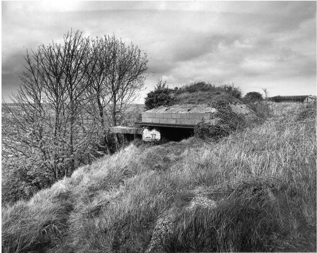
Figure 18 ?Shelter on the north side of Citadel Battery, with a pillbox immediately downslope (NMR: AA99/09739 © Crown Copyright 1999)
