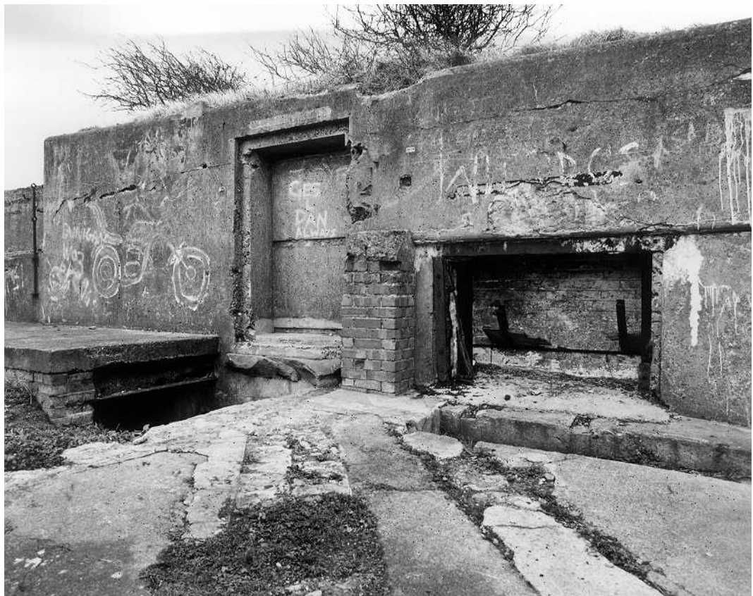
Figure 11 The parapet east of gun emplacement I, showing from right to left, the blocked ammunition lift, dials recess and blocked entrance to underground magazine and shelter (NMR: AA99/09746 © Crown Copyright 1999)
