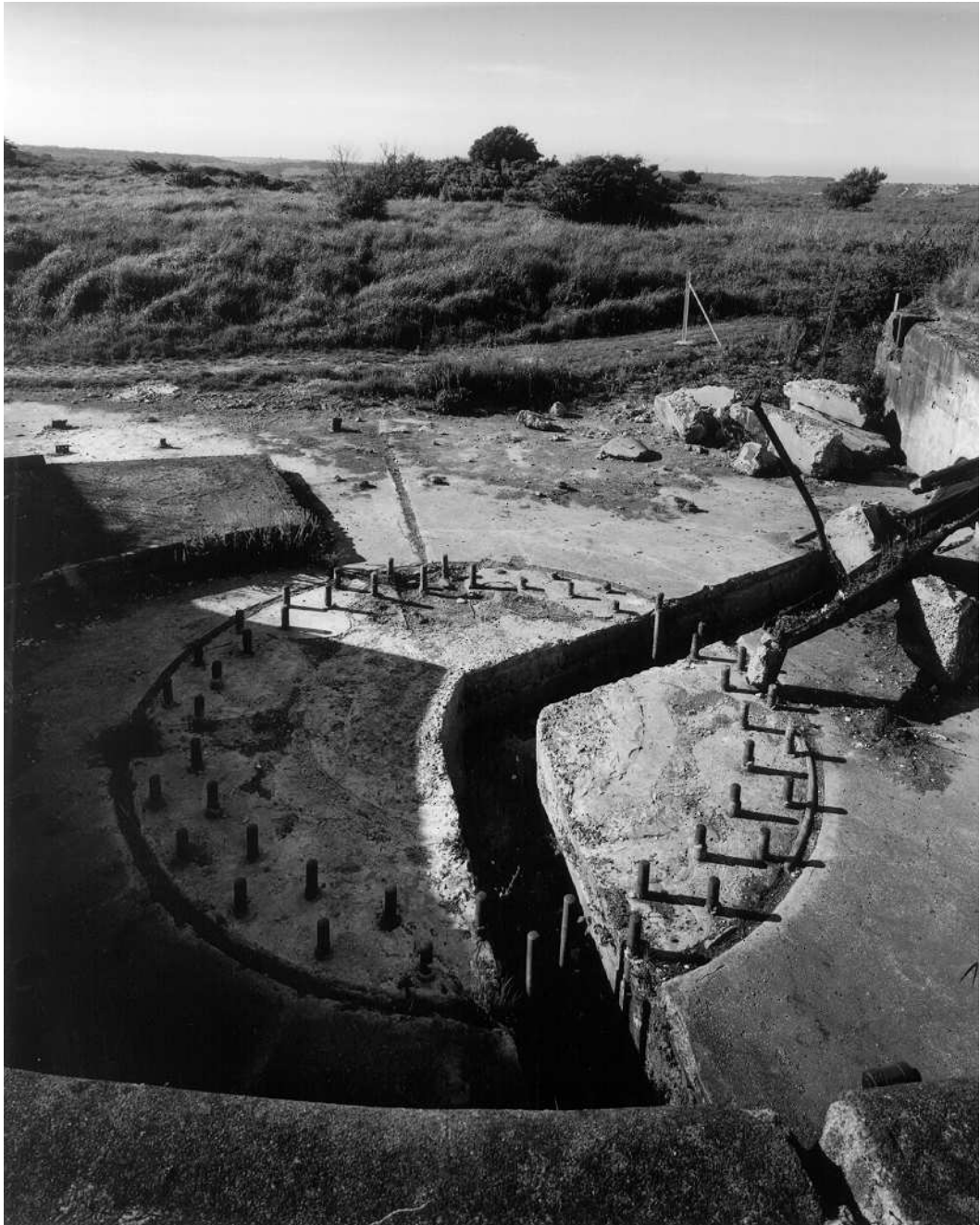
Figure 10 Emplcaement no III; detail showing the metal bolts of the gun holdfast and the gulley which carried hydraulic power to the gun and lift (NMR: AA99/09731 © Crown Copyright 1999)
