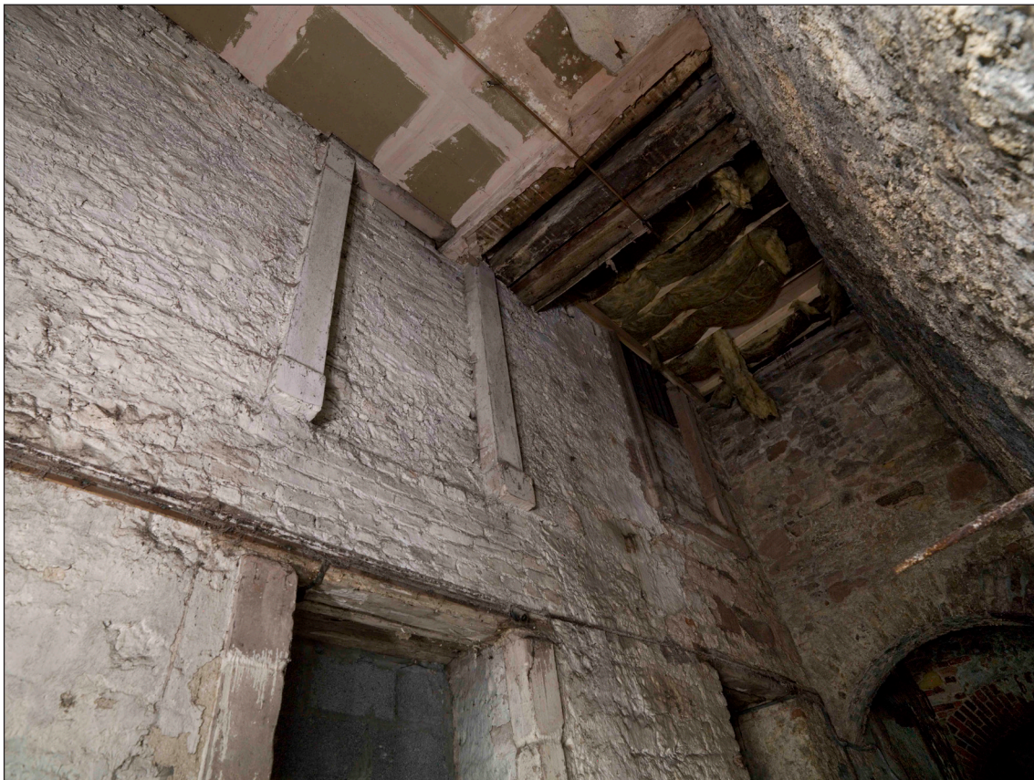
Fig. 40: View of the covered ground-floor passage extending along the north side of the granary, showing original openings (with raised surrounds) in the north wall of what was once the coach house and stables. DP065314 © English Heritage
