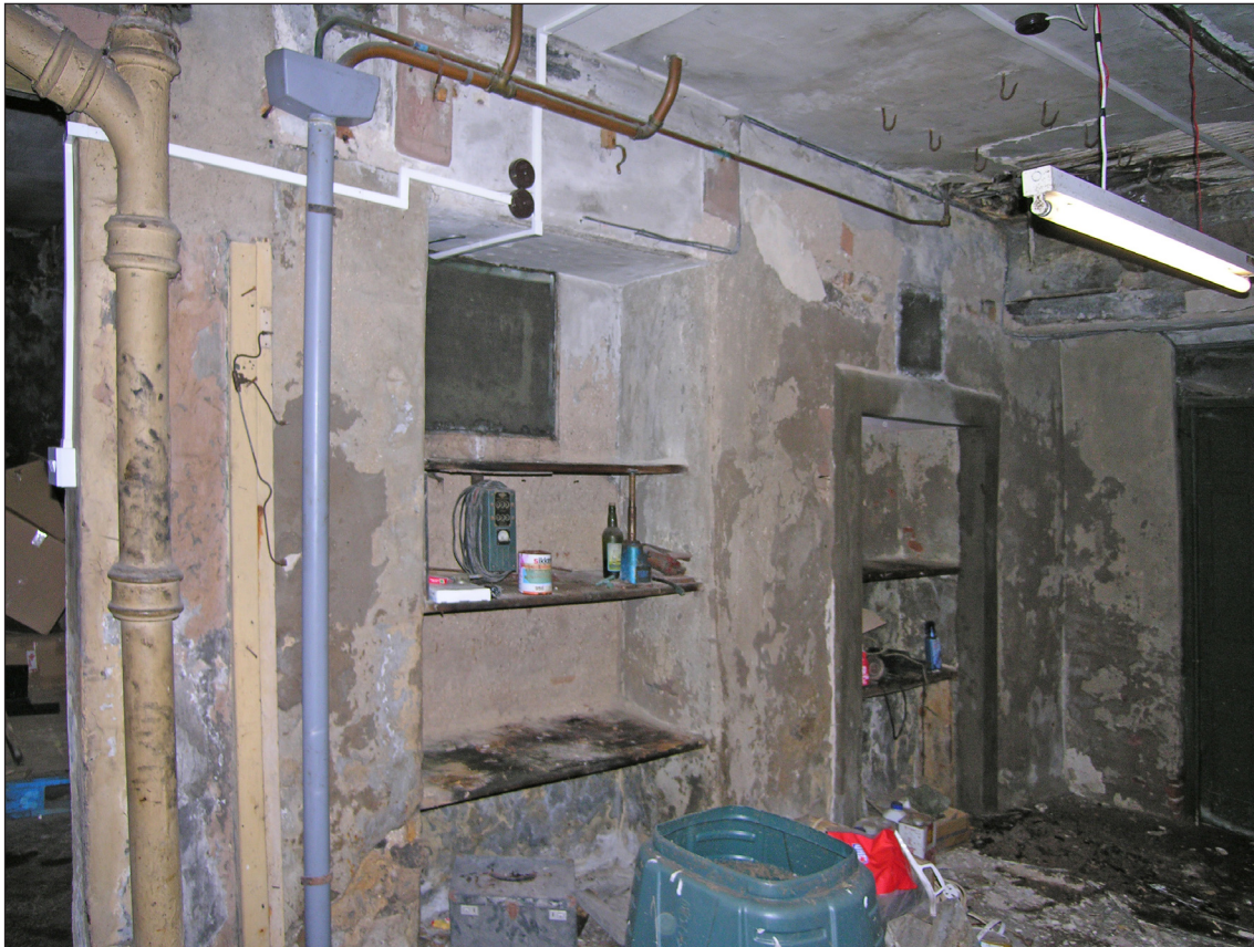
Fig. 42 (below): Blocked ground-floor openings in the southern wall of the granary. © English Heritage
