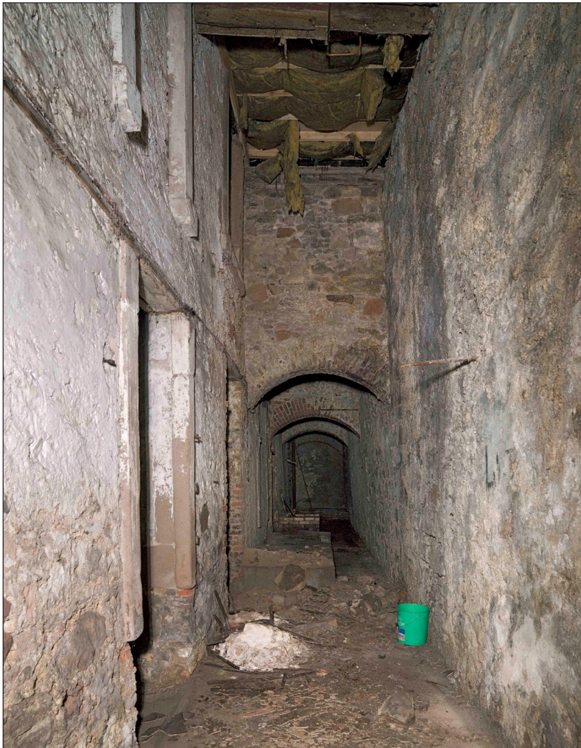
Fig. 45: The passageway on the line of the Cat Well Wall, showing the north wall of the granary to the left. DP065315 © English Heritage
