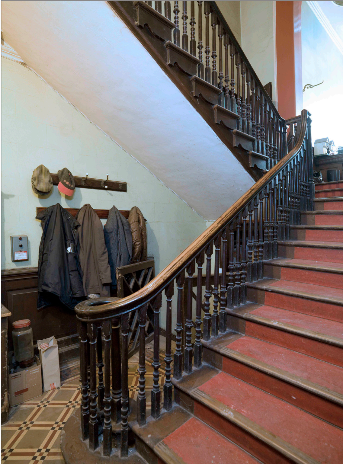
Fig. 17: The principal staircase of 2 Love Lane / 64 West Street with curtail, ramped handrail and three column balusters per step. DP065331 © English Heritage
