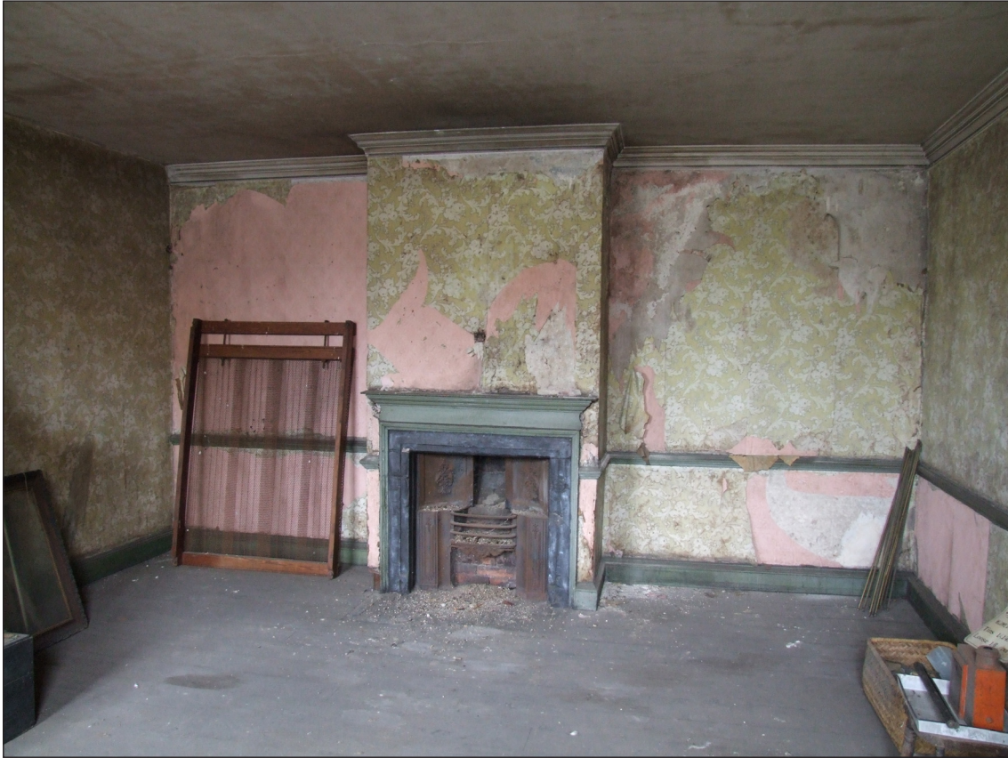
Fig. 26: The larger second-floor bedroom with stone chimney piece, 2 Love Lane / 64 West Street. © English Heritage
