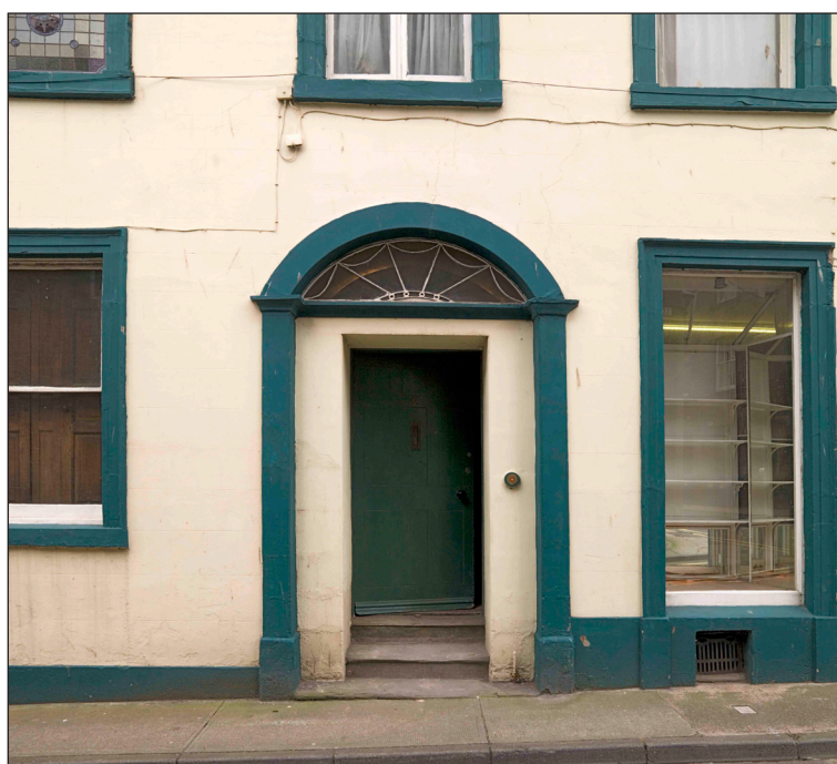
Fig. 30: The early-19th-century doorcase of 2 Love Lane / 64 West Street. DP065311 © English Heritage
