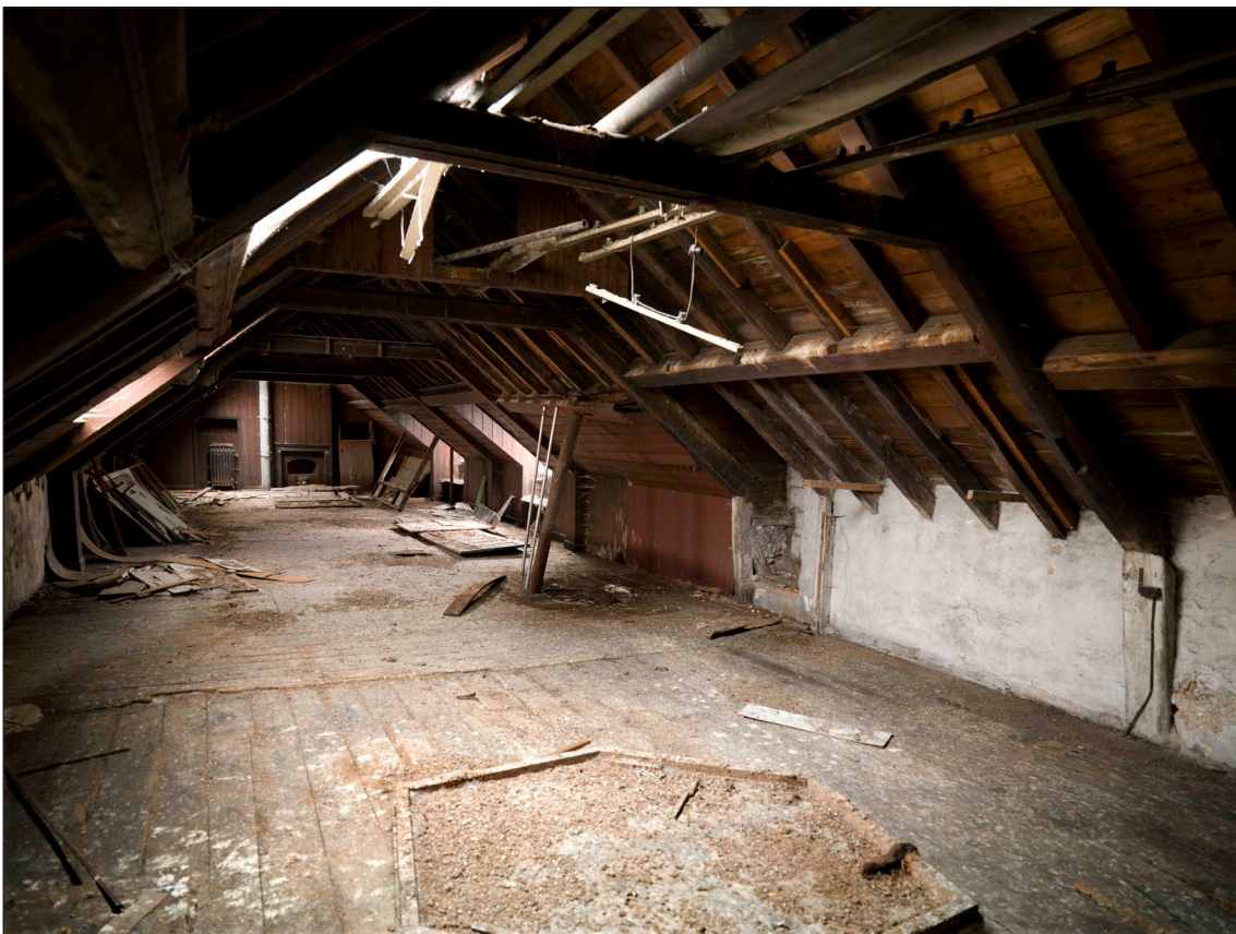
Fig. 48: View of the attic of the granary, showing the collar trusses, looking east, with John Wilson's late 19th-century office at the far end. DP065356 © English Heritage
