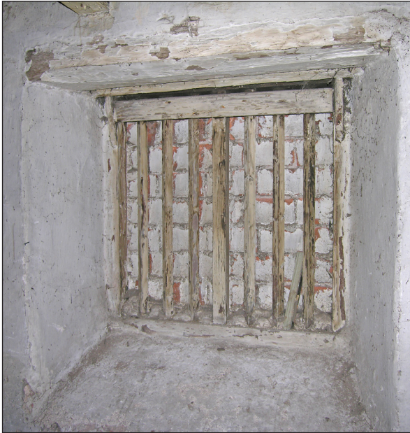
Fig. 46: A window on the second floor of the granary, with timber stanchions. © English Heritage
