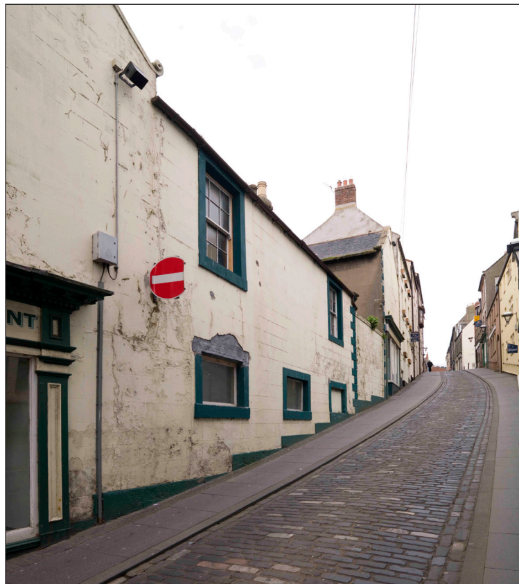
Fig. 34: The billiard room with bedrooms above, added to the rear of 2 Love Lane / 64 West Street. This addition faces onto West Street. DP065337 © English Heritage
