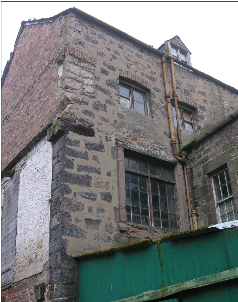
Fig. 43: First floor window with stone surround in the southern wall of the granary west of the outshot. © English Heritage
