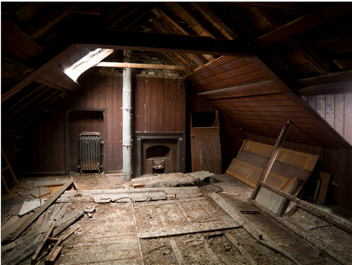
Fig. 51 (below): The tongued-and-grooved boarded office in the attic of the granary. DP065355 © English Heritage
