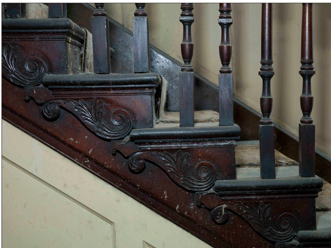
Fig. 68: The carved cheeks of the main, open-string stair in the principal range of 57 West Street / 64-66 Bridge Street. DP065373 © English Heritage
