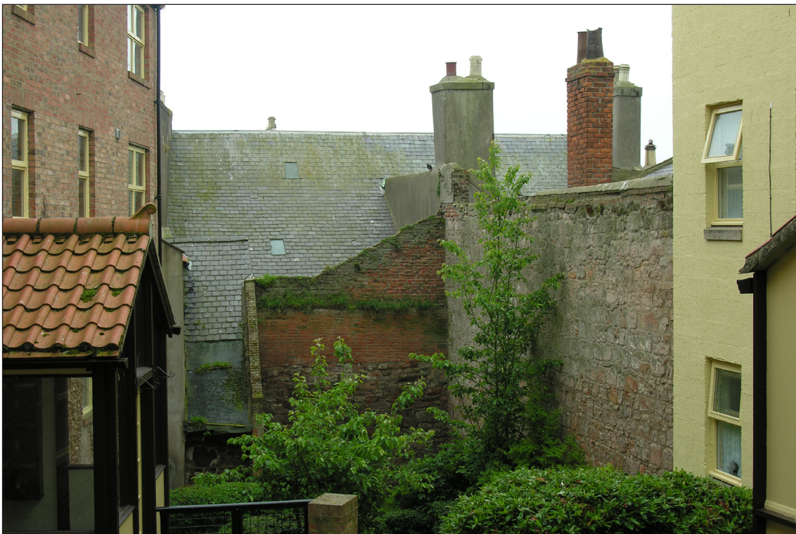
Fig. 60: The rear wall of the rear range and the roof of the principal range of 57 West Street / 64-66 Bridge Street as seen from Easter Wynd. DP065410 © English Heritage
