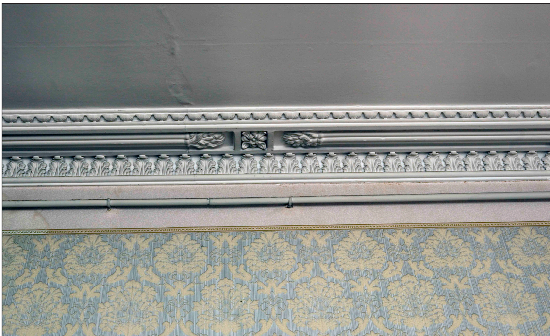
Fig. 31: The drawing room cornice, 2 Love Lane / 64 West Street. DP065318 © English Heritage
