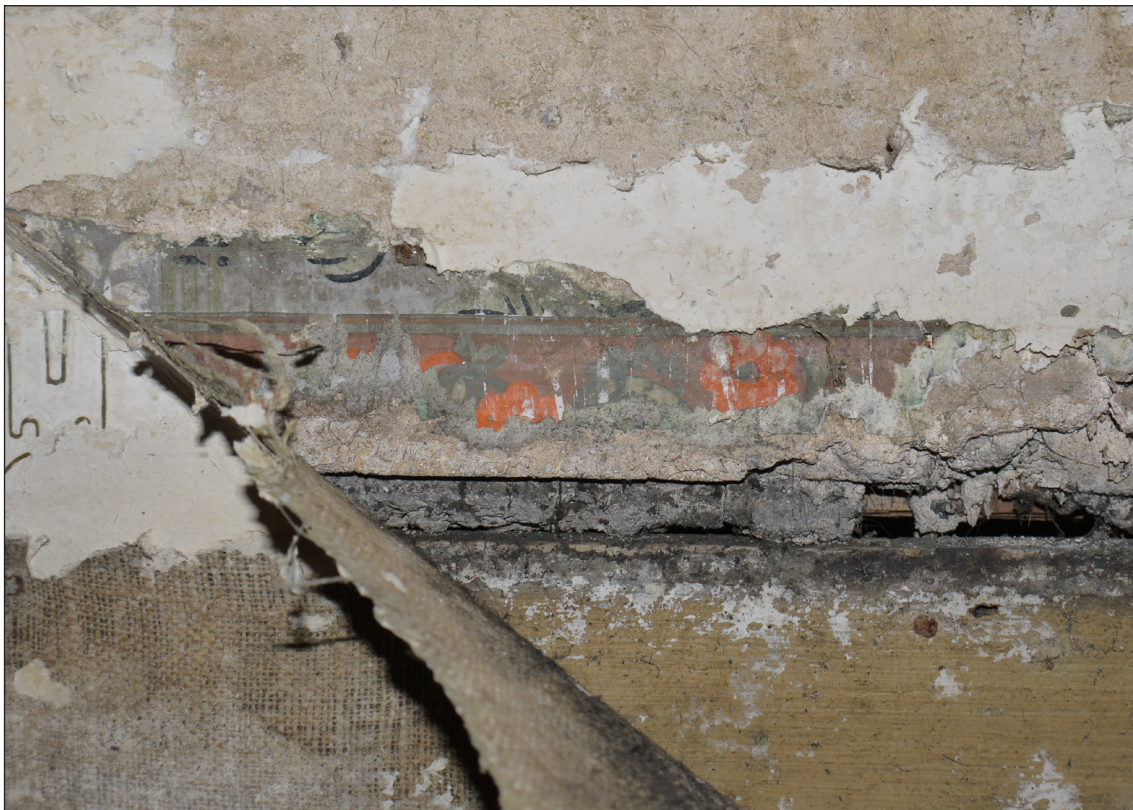
Fig. 69: The wallpaper border at dado-rail height in the west room on the second floor of the principal range, 57 West Street / 64-66 Bridge Street. © English Heritage
