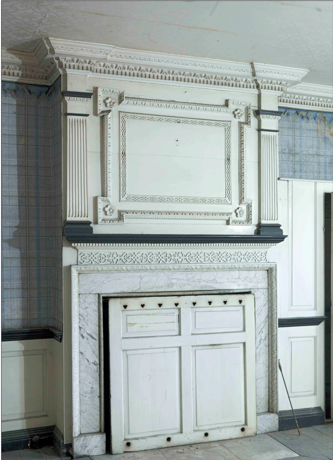
Fig. 70: The chimney piece and over mantel, complete with chimney board, in the large east room on the second floor of the principal range, 57 West Street / 64-66 Bridge Street. DP065380 © English Heritage
