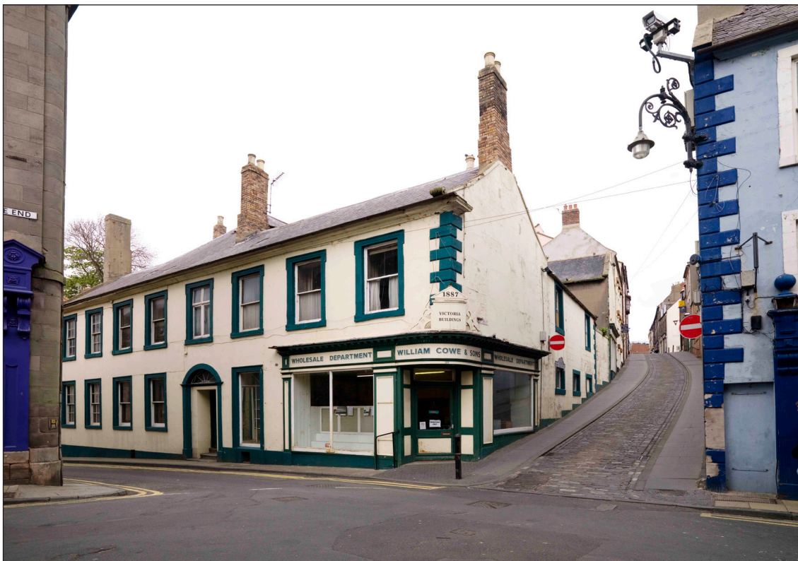
Fig. 11: 2 Love Lane / 64 West Street from the corner with Bridge Street. The slate-roofed building to the rear, running parallel to the house, is 60 West Street. DP065320 © English Heritage
