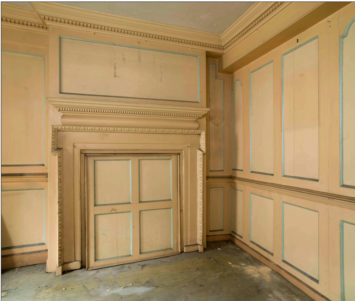
Fig. 63: The wainscotted room on the first floor of the principal range of 57 West Street / 64-66 Bridge Street, complete with chimney board. DP065399 © English Heritage
