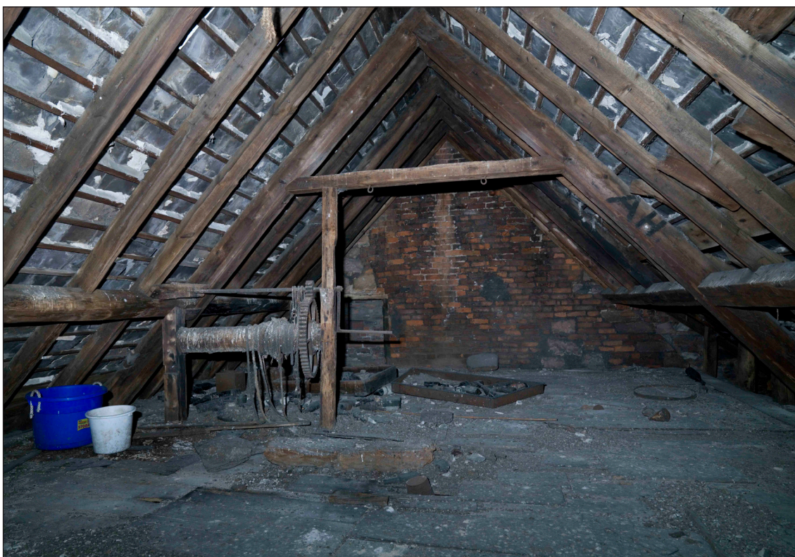
Fig. 74: The roof of the main range of 57 West Street / 64-66 Bridge Street, looking west. The winch is associated with a low loading doorway in the gable beyond. DP065403 © English Heritage
