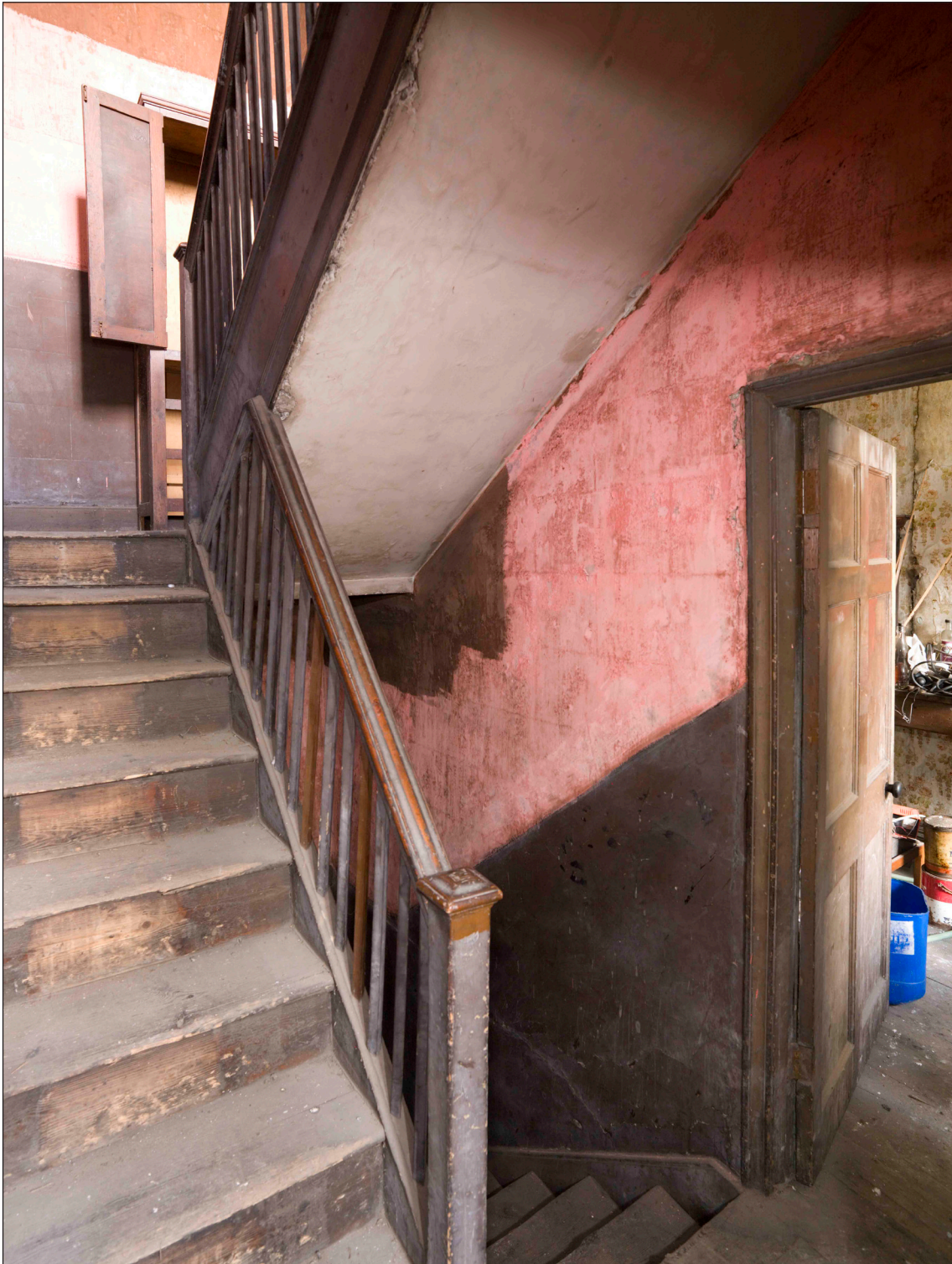
Fig. 21: The second stair of 2 Love Lane / 64 West Street, from the first-floor landing. DP065330 © English Heritage
