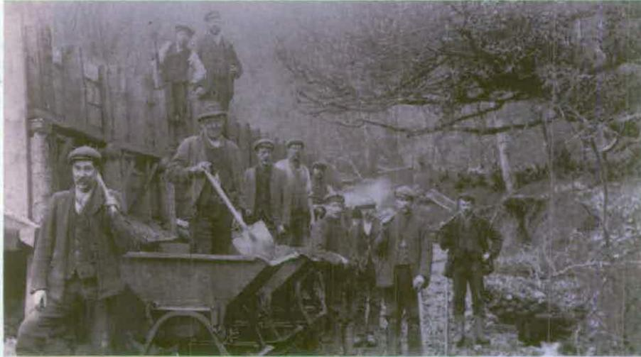
*Figure 3: Colton Pits: working the west adit in 1908. Iron ore was tipped from the mine tramway wagons into these wooden bins. A light railway then took the ore up the incline (Hole Collection).*
