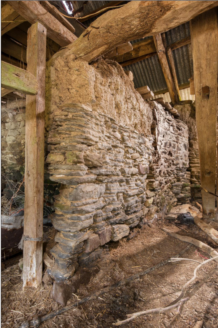
Figure 48 Spine beam in the linhay supporting the joists of the tallet, looking north west [DP220522]
