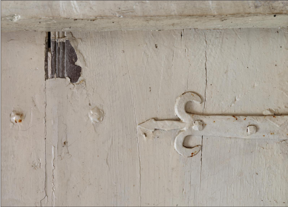
Figure 42 Detail of the door between the first-floor landing and the room over the central hall, showing a decorative moulding visible on the edge of the door plank where the paint has fallen away and the end of the decorative strap hinge [DP220765]
