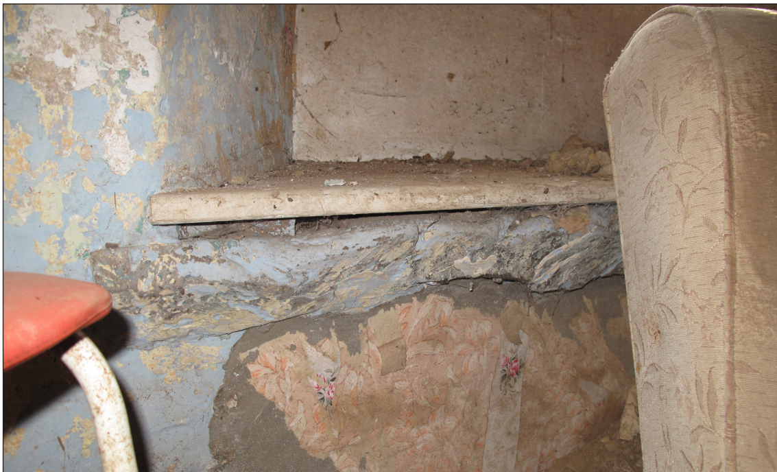
Figure 11 Earlier timber window sill visible underneath the later sill in the surviving hall window [© Historic England Rebecca Lane]
