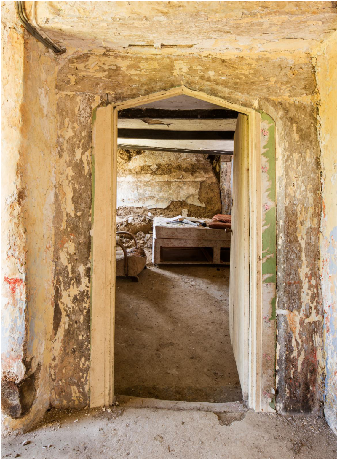
Figure 31 Doorway between the cross passage and the hall, looking west [DP220533]
