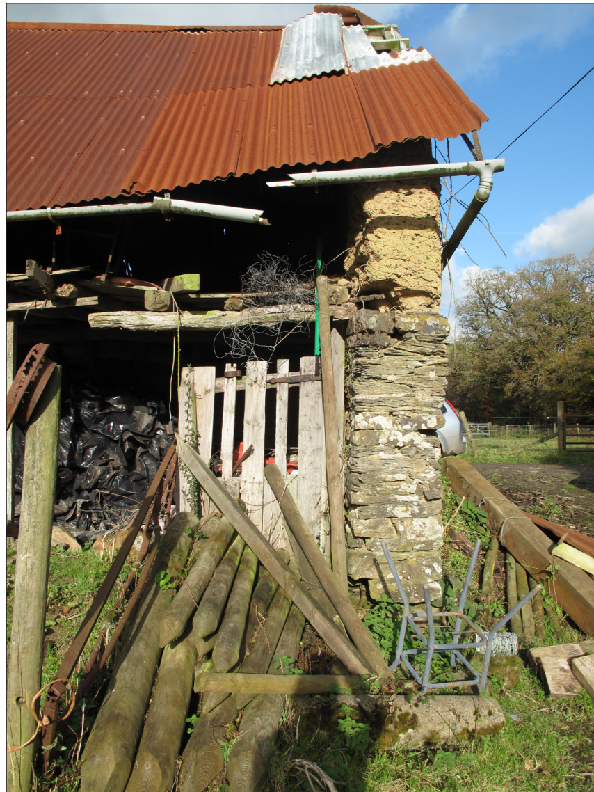
Figure 49 South-east corner of the linhay, looking north. Note the remains of the timber beam which formerly supported the southern end of the tallet [© Historic England Rebecca Lane]
