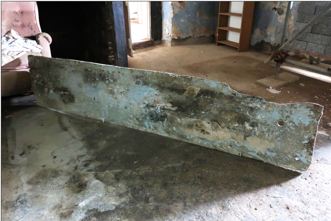
Figure 61 Timber plank found within the cob walling under truss A-A1 (Investigator photograph)
