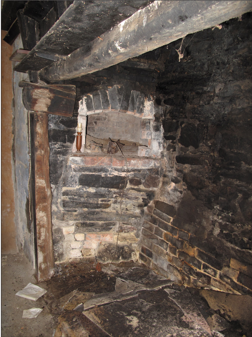
Figure 55 North jamb of the fireplace in the hall, looking north east, showing detail of the opening to the bread oven [© Historic England Rebecca Lane]
