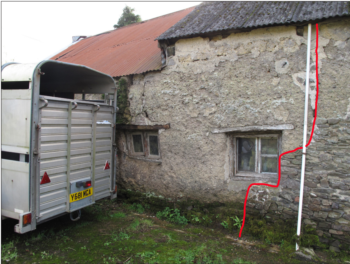
Figure 52 North wall of the farmhouse, looking south east. The uneven junction between the fabric of the original north wall and the later infill section of walling is marked with a red line [© Historic England Rebecca Lane]
