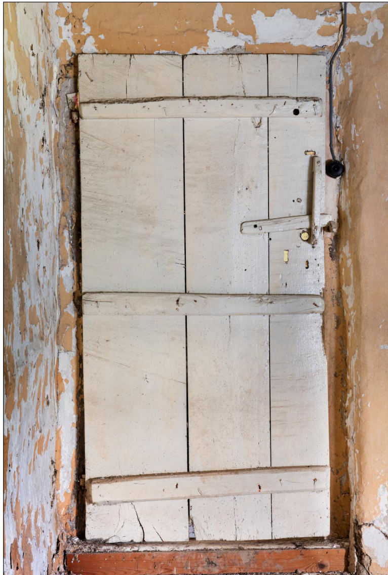
Figure 41 Back of the door between the first-floor landing and the room over the hall [DP220567]
