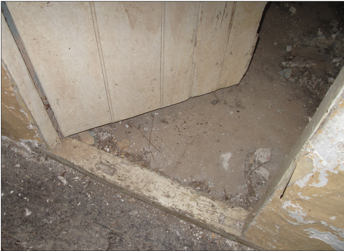
Figure 33 Cross beam in the partition between the eastern room and the cross passage, viewed from the current first-floor landing, looking north east. Note the residual mortices for the studs of the partition, which indicate the doorway is later [© Historic England Rebecca Lane]
