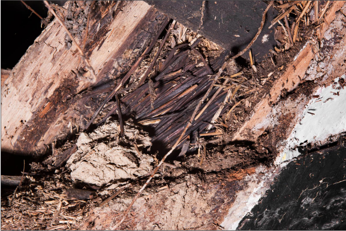
Figure 16 Surviving fragment of smoke-blackened thatch adjacent to the southern principal rafter of truss A-A1 [DP220570]
