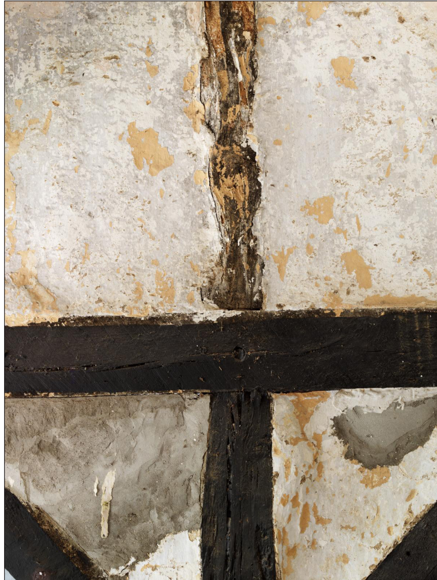
Figure 15 Eastern side of truss A-A1, looking west, showing the junction of the central post and the collar, with a large single peg joining the two [DP220759]
