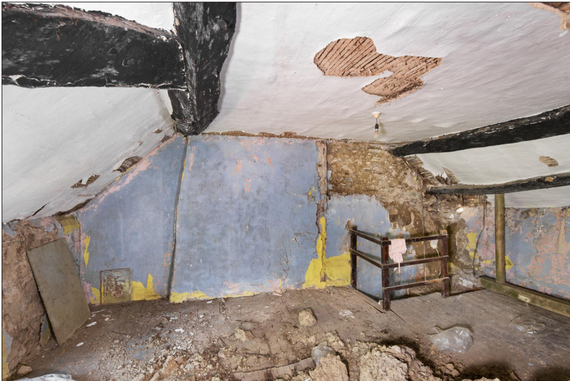
Figure 12 West gable wall, from the first-floor western room, looking west [DP220547]
