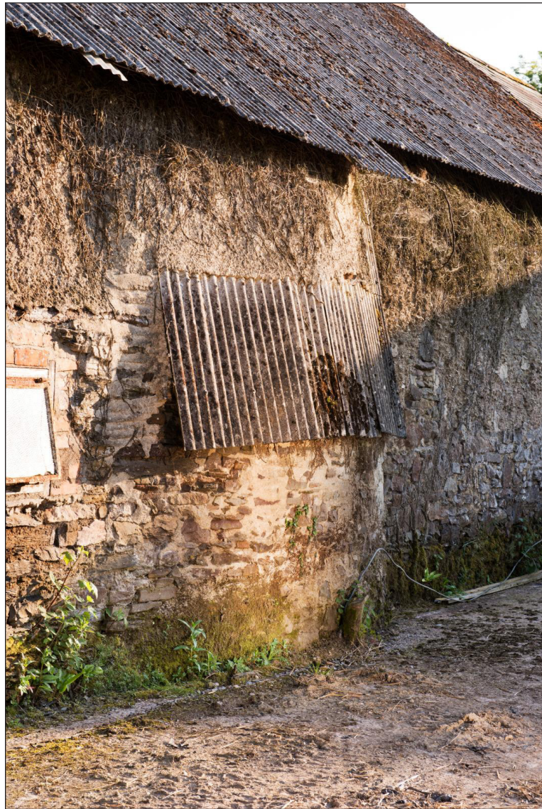
Figure 54 North elevation of the farmhouse, looking south west, showing the curving external wall of the bread oven [DP220577]
