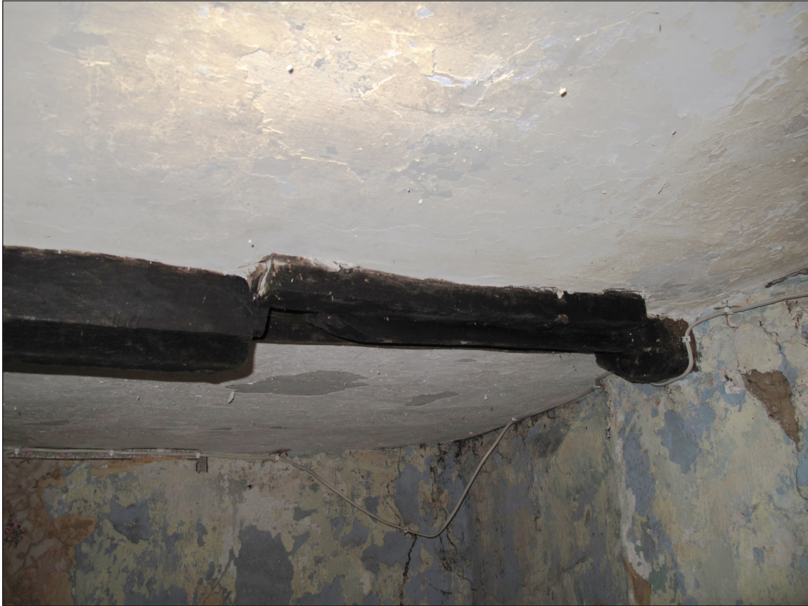
Figure 39 Offset section of the eastern cross beam in the hall, looking south east [© Historic England Rebecca Lane]
