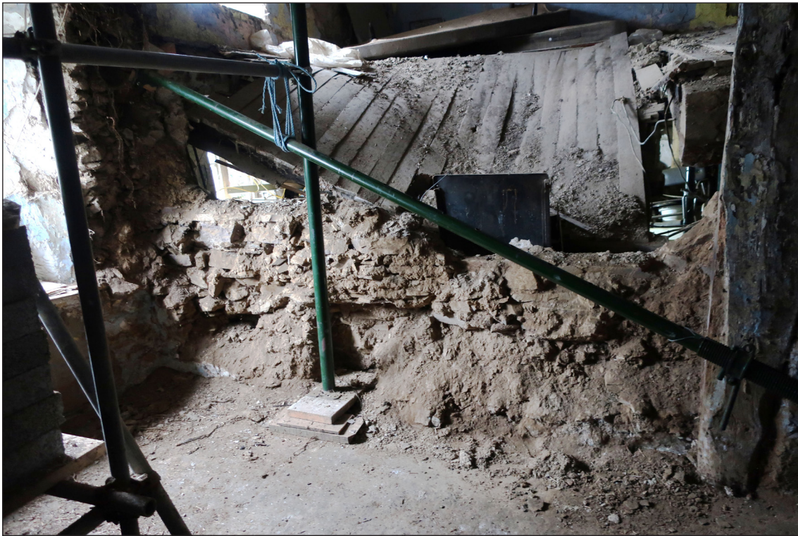
Figure 27 View of collapsed cob wall, built up against the earlier partition under truss A-A1, looking west [© Historic England Rebecca Lane]
