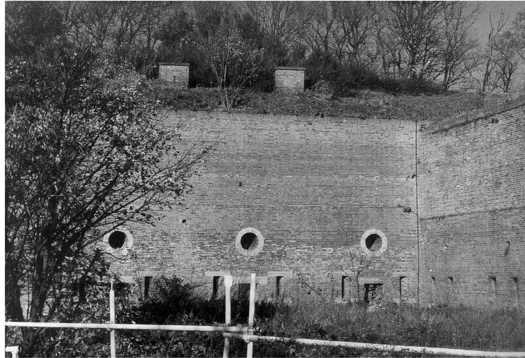
The southern end of the ditch emerges on the steep slope. The scarp is revetted, initially with the same brickwork, except that the top is finished in a quarter-round profile. Erosion at the base reveals a thickness of 1½ bricks set against
