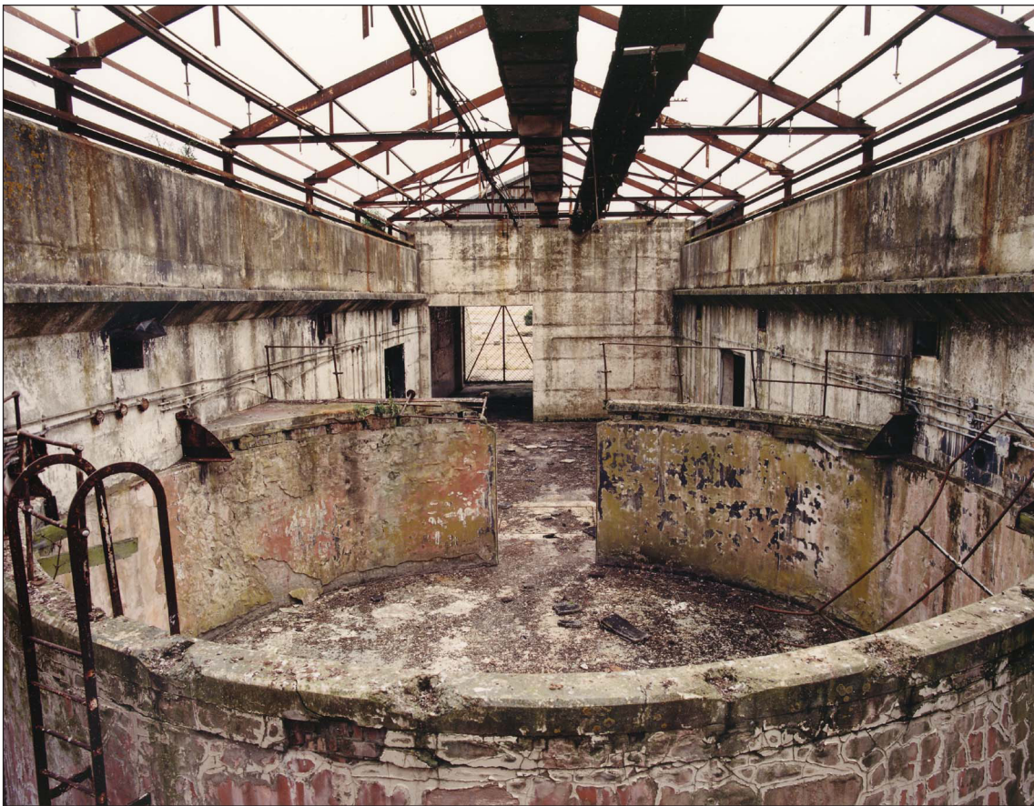
Figure 30: Laboratory I in June 2000, interior showing the centrifuge pit and above it a section of air conditioning conduit. Below the tops of the walls are projecting ledges that carried rails for a travelling crane. (c) English Heritage
