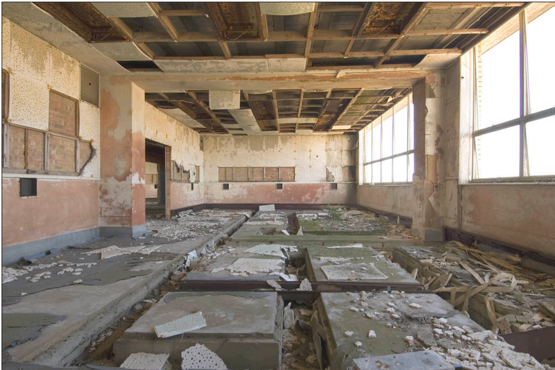
Figure 32: The Control Room E4, showing the large southwestern control room, with subfloor cable ducts and sound proofing boards. (c) English Heritage DP070006
