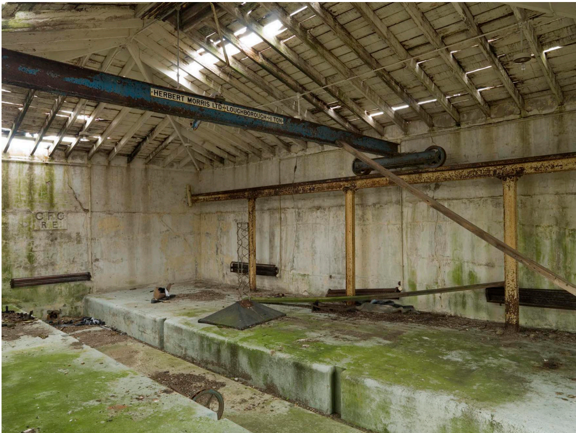
Figure 21: First World War Magazine D2 showing storage platforms and later alterations. (c) English Heritage DP070014
