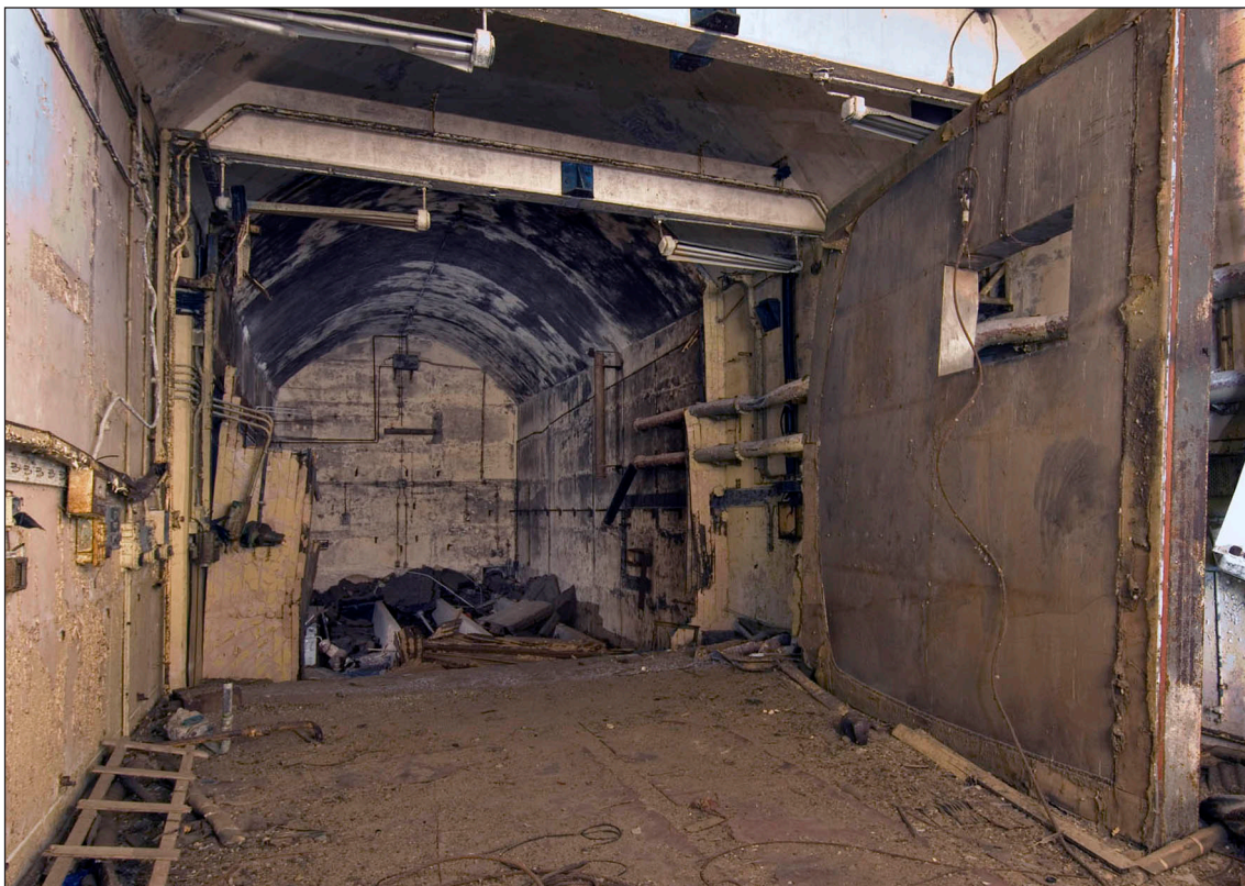
Figure 28: Laboratory 3, interior showing the rear climatic chamber and dismantled sliding door that sealed the chamber. (c) English Heritage DP068471
