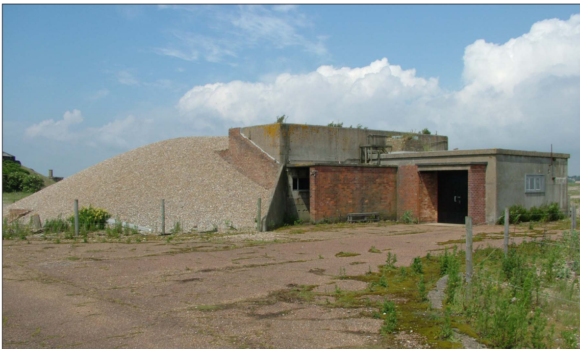
Figure 26: Control Room F4 I27/I67, showing the later brick porch and blast wall. (c) English Heritage
