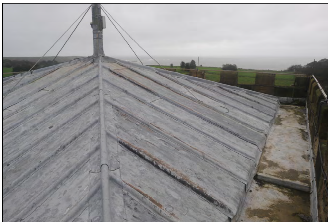
Figure 3. General view of south side of tower roof showing roll joints in lead
