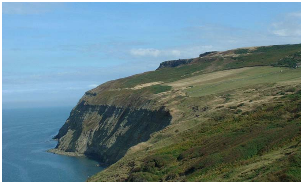
Figure 3. View of Loftus Alum Works from the west, showing the profile of the cliffs
