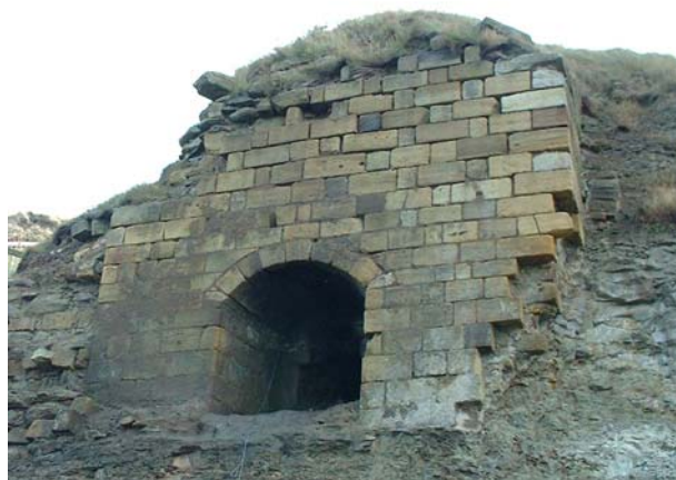
Figure 33. Photograph of the arch adjacent to the steps down to Hummersea Beach. This may be the remains of a kiln or boiler, possibly associated with the building shown in 19th century photographs.
