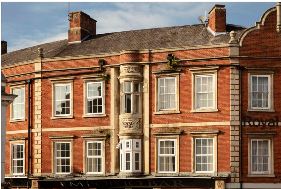
Figure 33: Oriel window on the west street elevation [DP300995]
