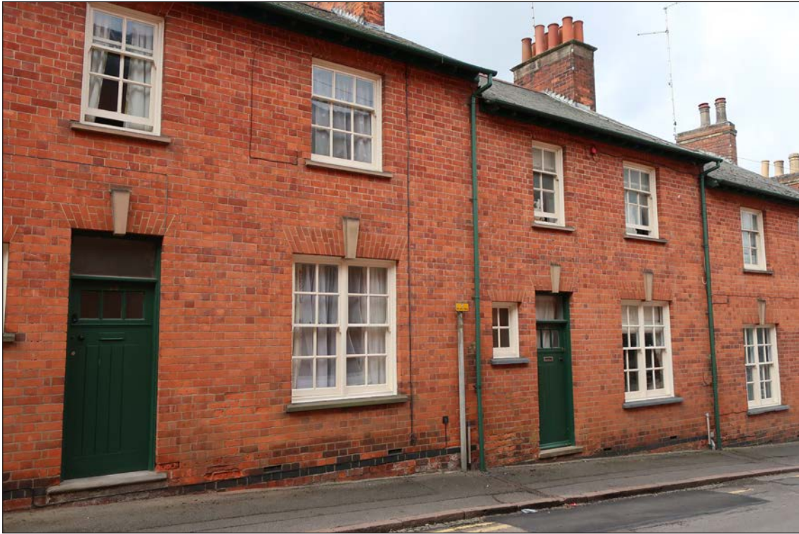
Figure 21: Numbers 23-25 West Street [© Historic England, Aimee Henderson]
