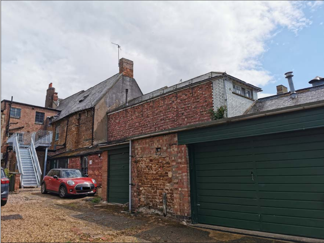
Figure 28: North elevation as seen from the courtyard of numbers 1-7 High Street [© Historic England, Aimee Henderson]
