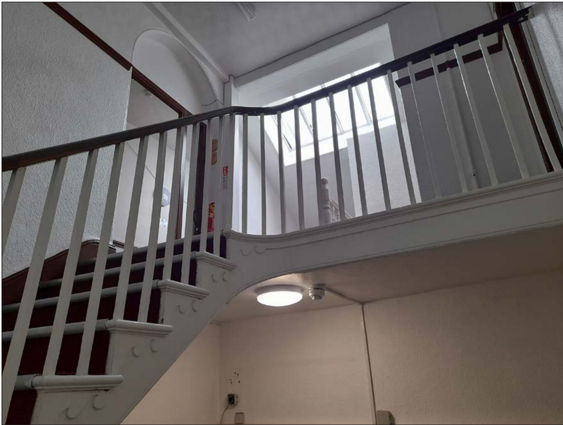
Figure 30: North stair, second-floor landing when viewed from below [© Historic England, Aimee Henderson]
