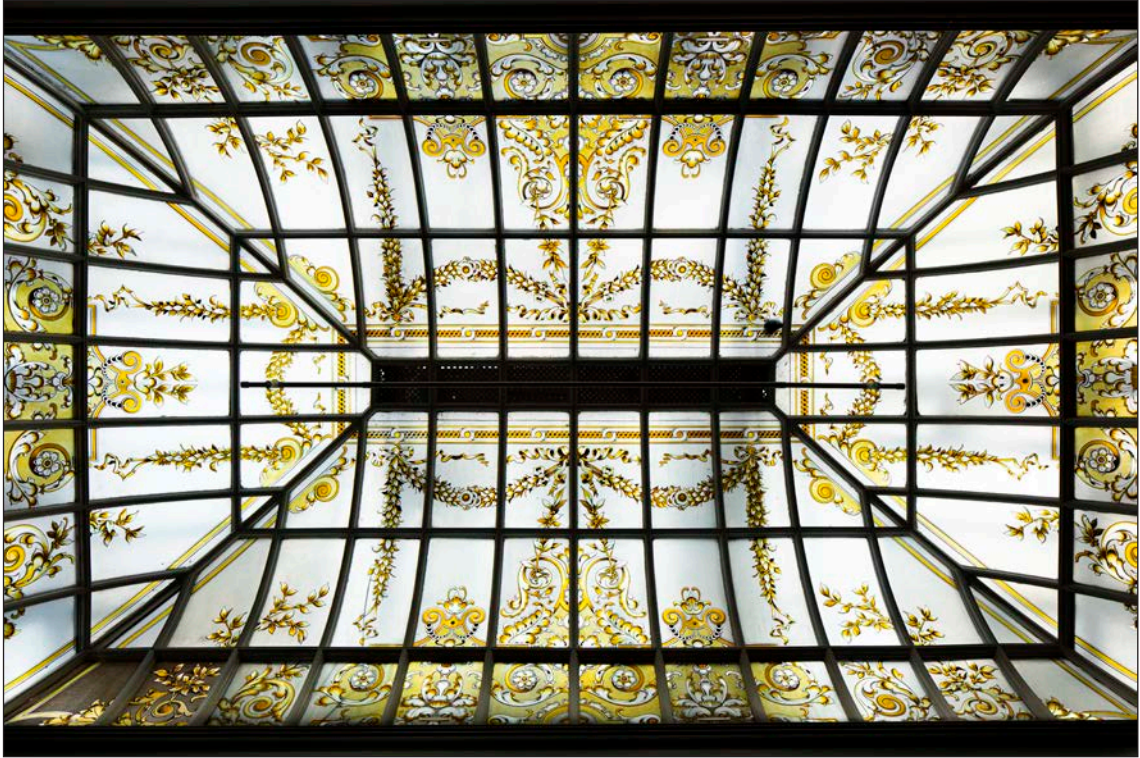
Figure 41: Glazed roof above the restaurant [DP311850]
