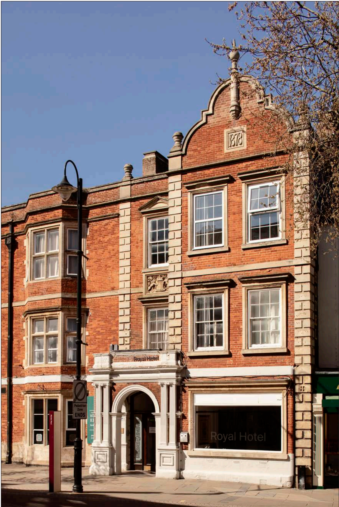
Figure 4: Northern gable with date stone and entrance porch [DP300771]
