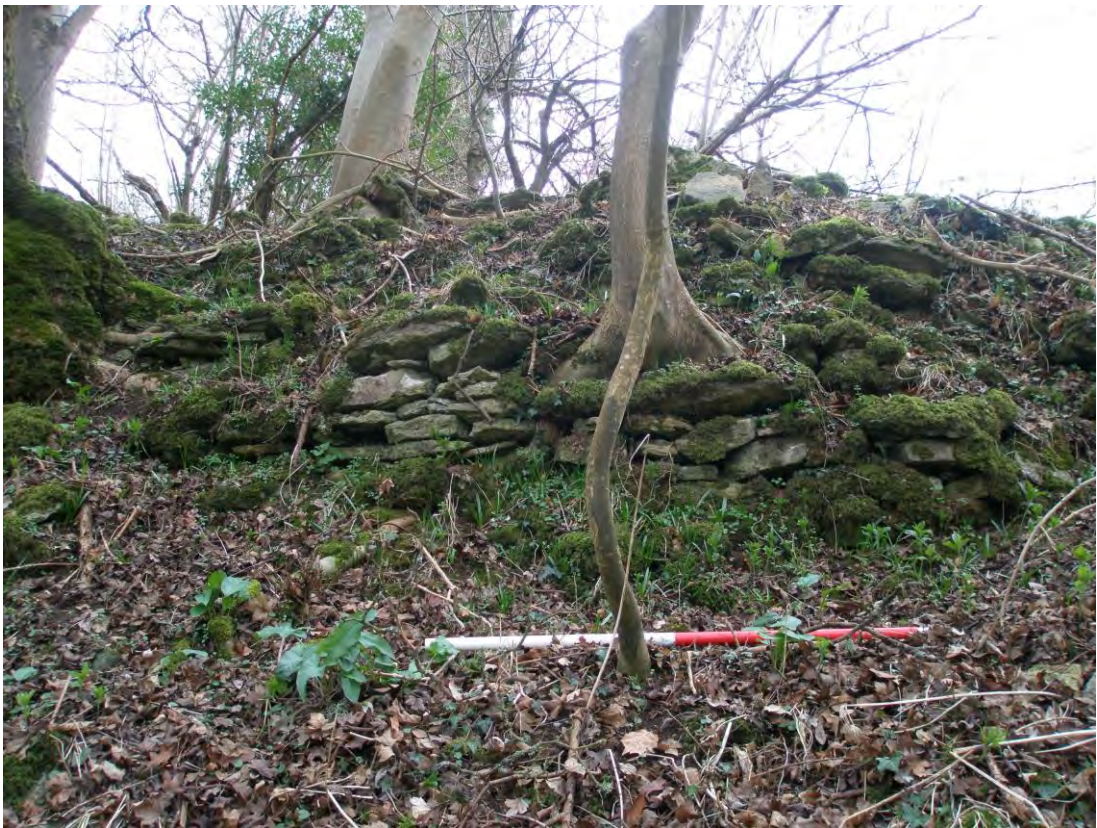
Figure 15: Revetment walling on top of the ringwork bank (6 on survey plan)
