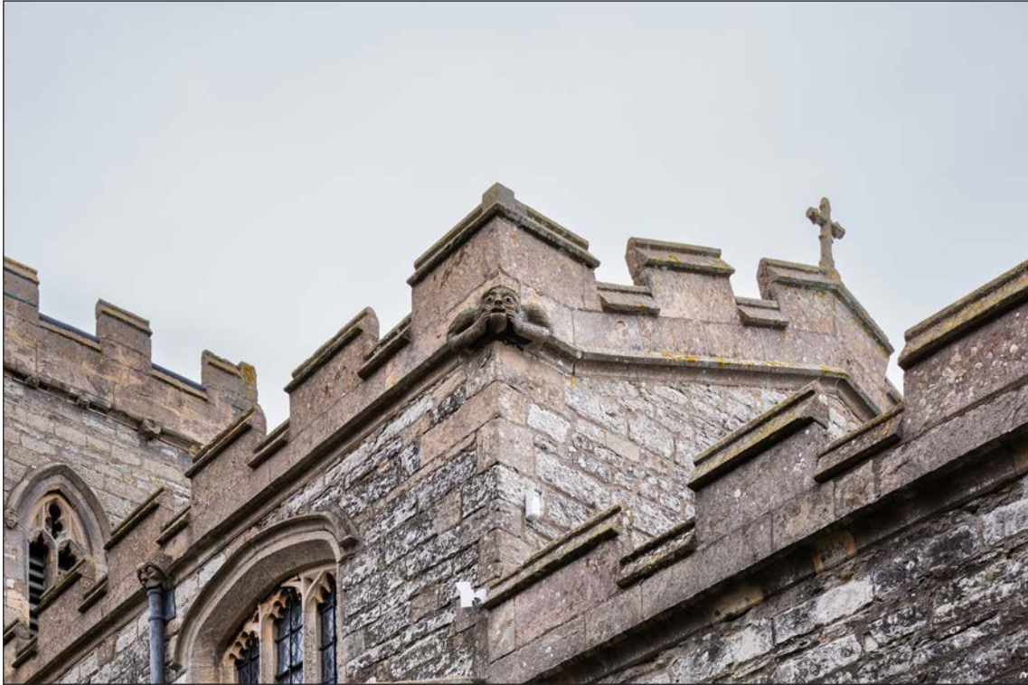
Figure 4: Grottesque, southeast corner of the nave. Note also the stone gargoyle above the rainwater downpipe [DP311810]
