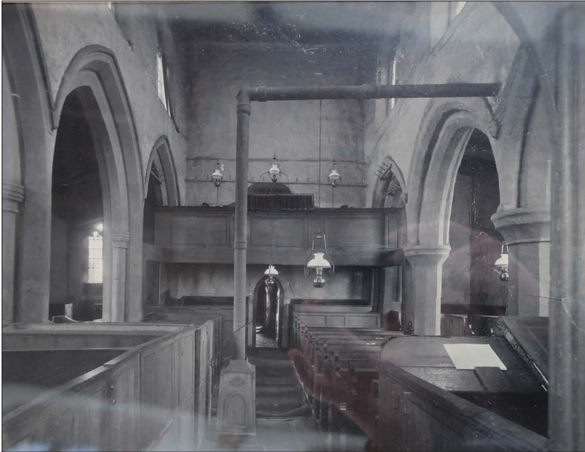
Figure 13: Church interior looking west c. 1900, note the infilled tower arch with the gallery above and surviving box pews [St Wilfrid's North Muskham PCC] 74
