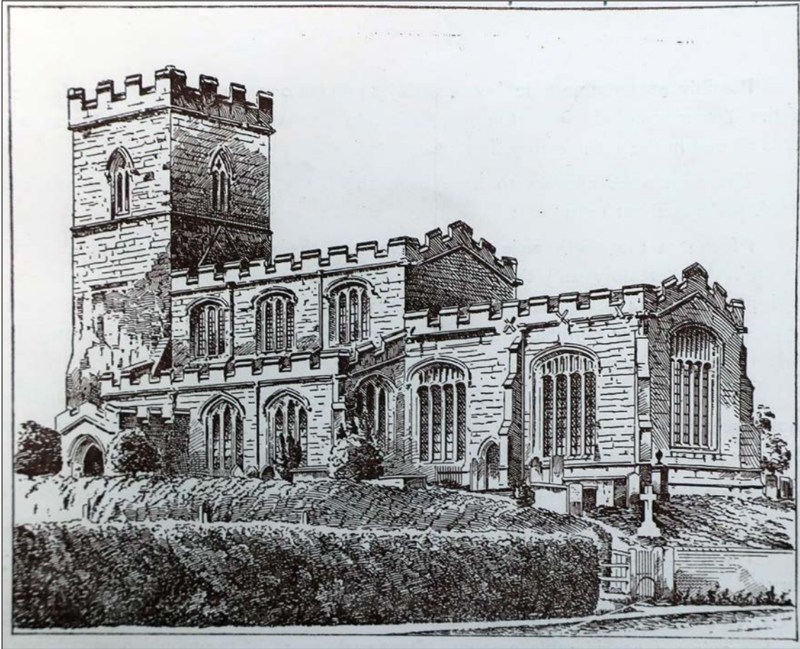
Figure 14: Drawing of St Wilfrid's North Muskham, 1904, note the hashed lines suggesting render on the lower stage of the tower. [Nottinghamshire Archives DR/1/1/2/1711A/15]
