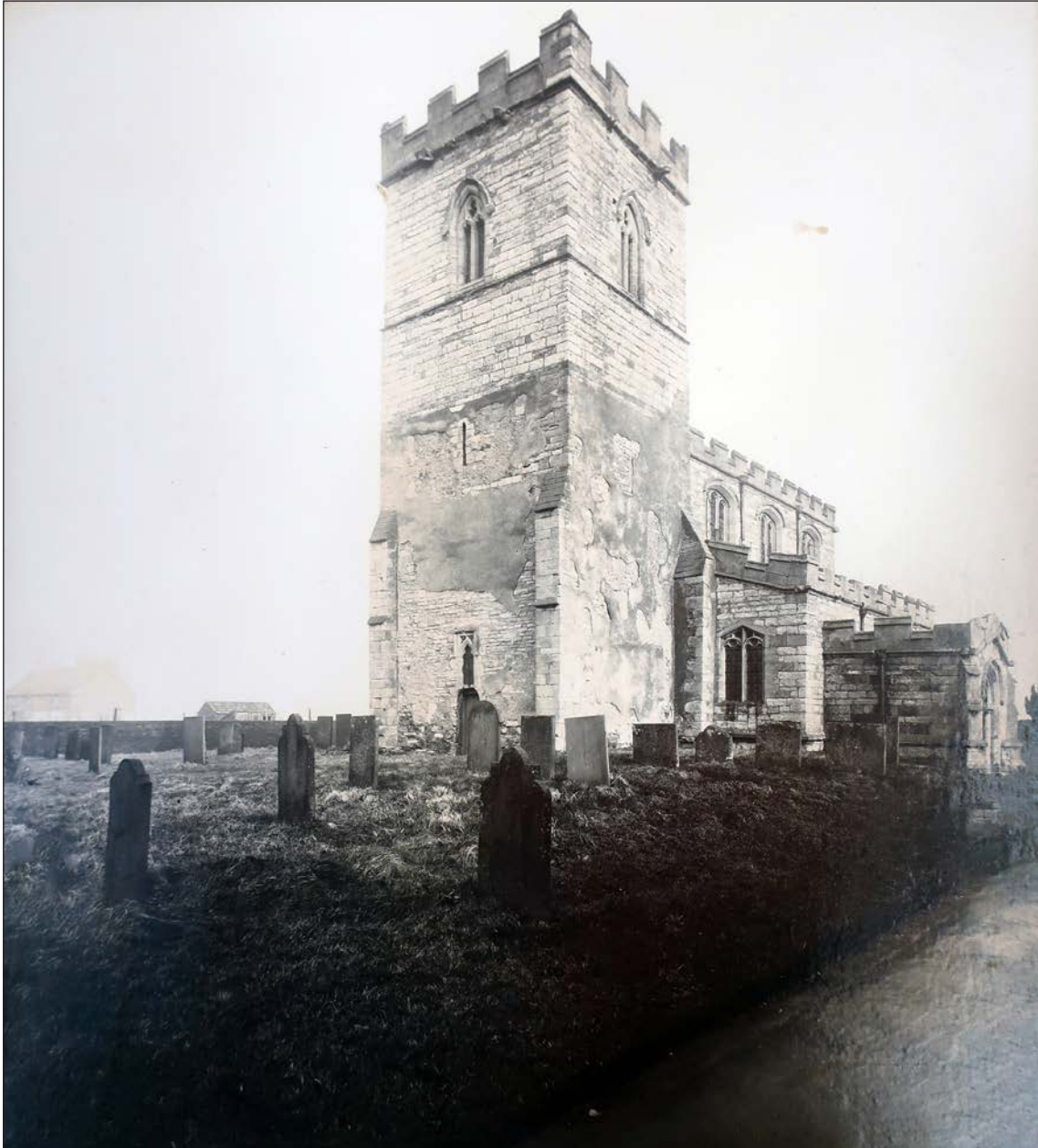
Figure 15: Undated photograph (estimated to be c. 1900) showing render on the exterior of the tower [St Wilfrid's North Muskham PCC]
