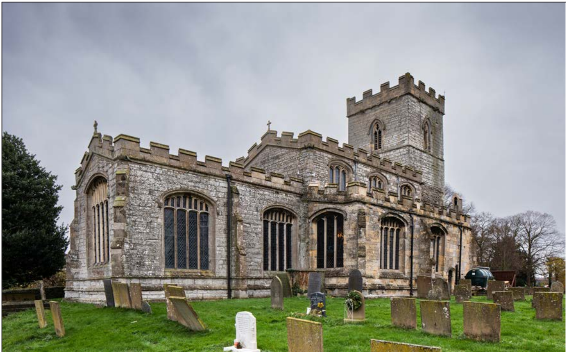
Figure 3: Nave and chancel from North [DP311806]
