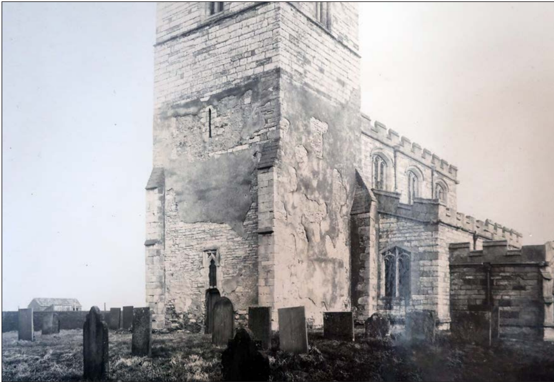
Figure 16: Undated photograph (estimated to be c. 1900) showing render on the exterior of the tower (detail). Note also the now blocked door in the western elevation. [St Wilfrid's North Muskham PCC]
