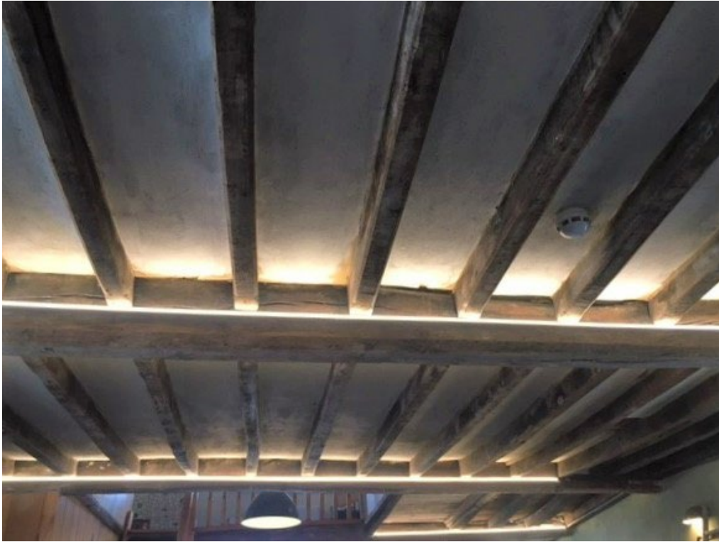
Figure 4: Rear range; ceiling structure, photograph taken from the south (Alison Arnold)
