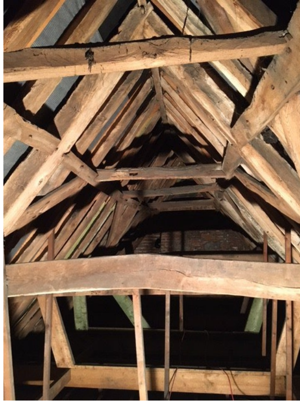
Figure 2: Truss 3, photograph taken from the east (Alison Arnold)
