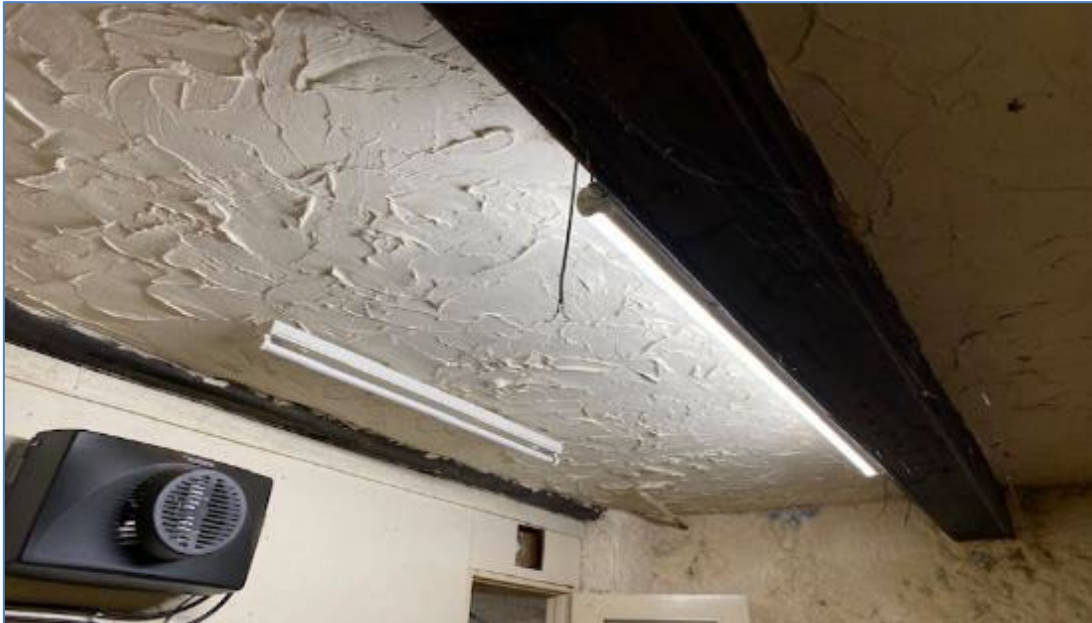
Figure 8: Cellar ceiling (No 27), photograph taken from the south-west (Alison Arnold)
