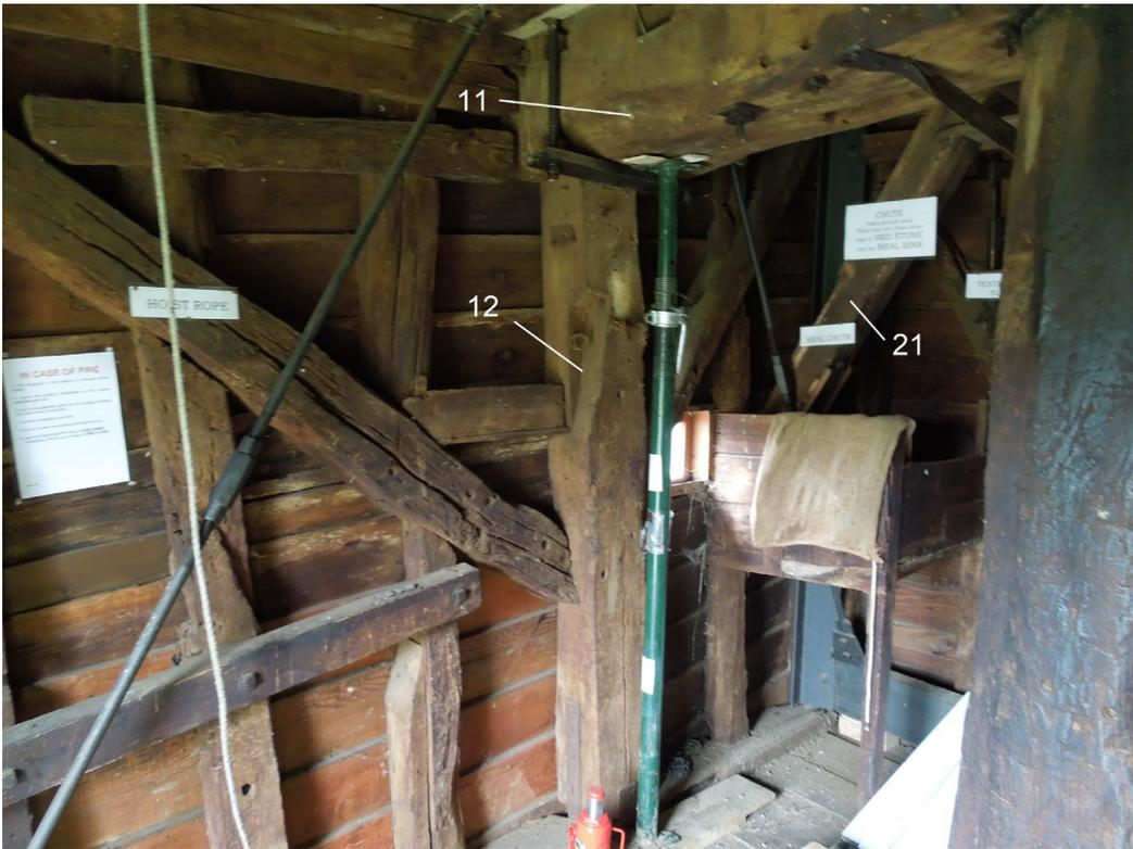
Figure 3: Photograph looking at the left centre of the buck, indicating the left vertical post (bourn12) with the crown-tree (bourn11) and front diagonal brace (bourn21, photograph by Martin Bridge)
