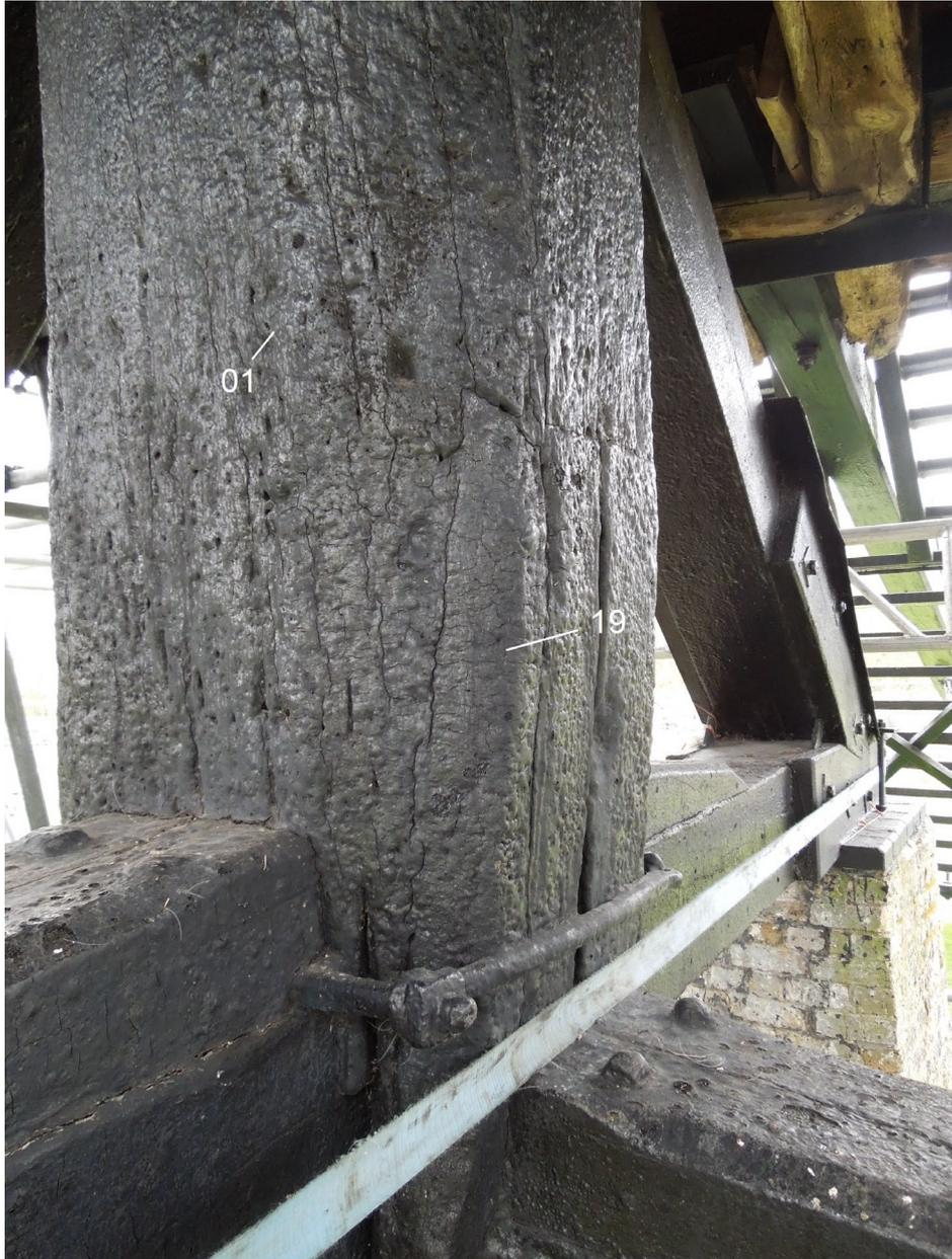
*Figure 5: View of the main post (bourn01), looking towards the rear of the mill (currently east, with the mill immobile) and indicating the patch at the base of the main post (bourn19)(photograph by Martin Bridge)*
