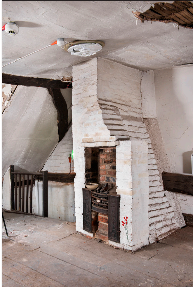
Figure 40 Interior, second floor, south room, inserted fireplace. [DP219886]
