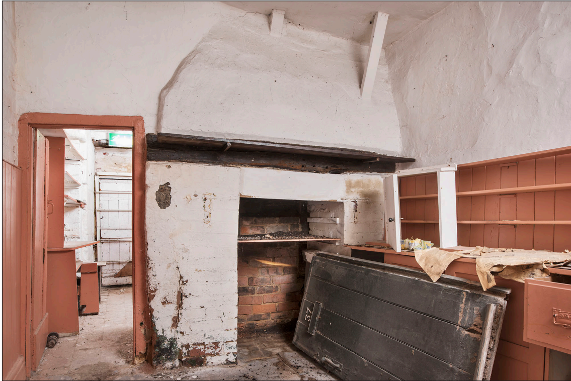
Figure 28 Interior, ground floor, south room showing inserted fireplace. [DP219912]
