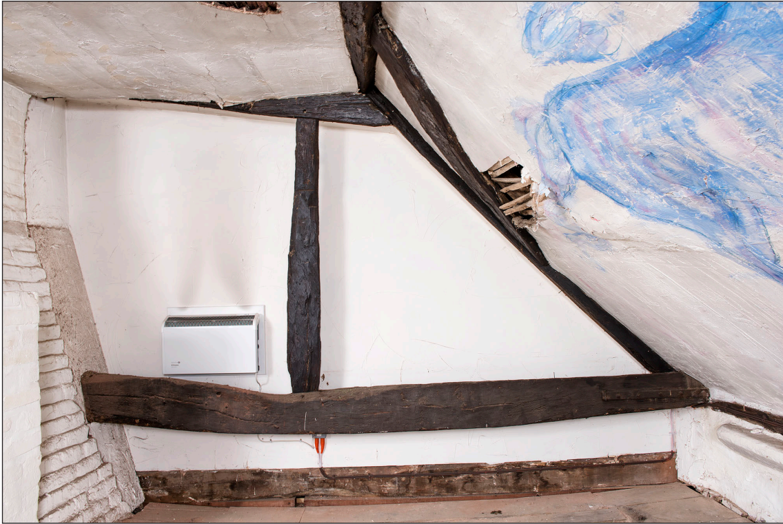
Figure 33 Interior, second floor, south room, showing detail of south truss. [DP219887]
