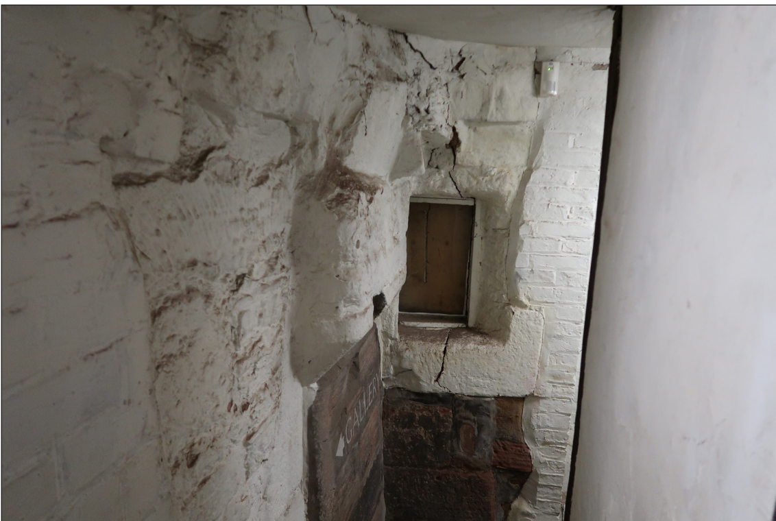
Figure 20 Interior, east elevation, ground floor, north room, showing jamb of doorway and stonework around the high level window feature. [Rebecca Lane © Historic England]
