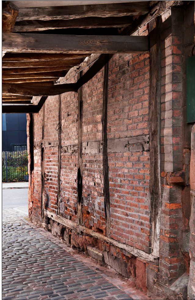
Figure 25 Exterior, north elevation of passageway. [DP219943]
