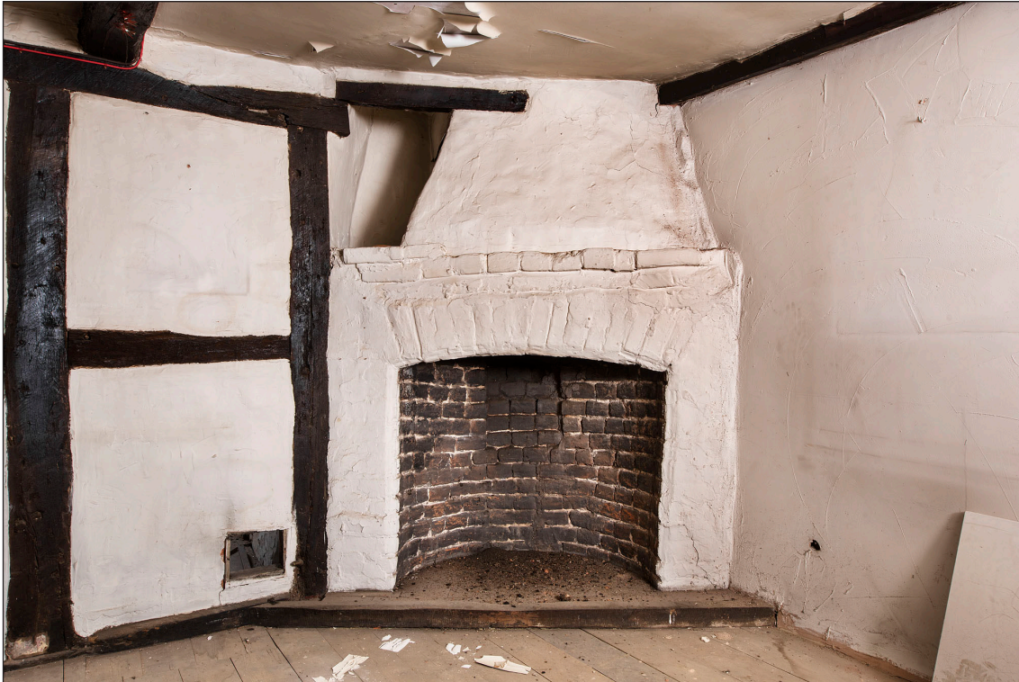
Figure 38 Interior, first floor, south room, showing inserted fireplace. [DP219903]
