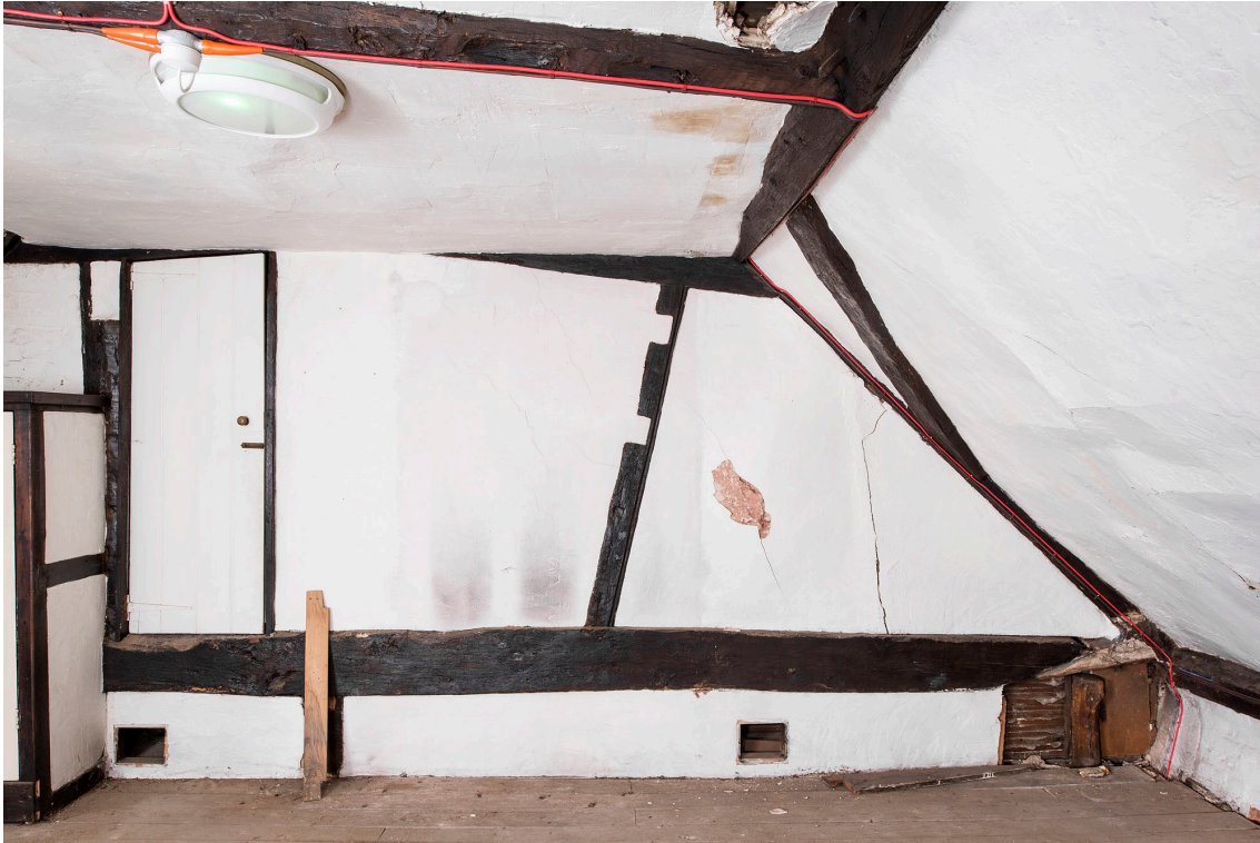
Figure 32 Interior, second floor, north room showing detail of central truss. [DP219895]
