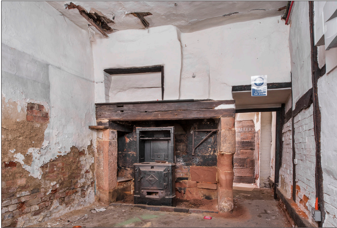
Figure 27 Interior, ground floor, north room showing inserted fireplace. [DP219918]
