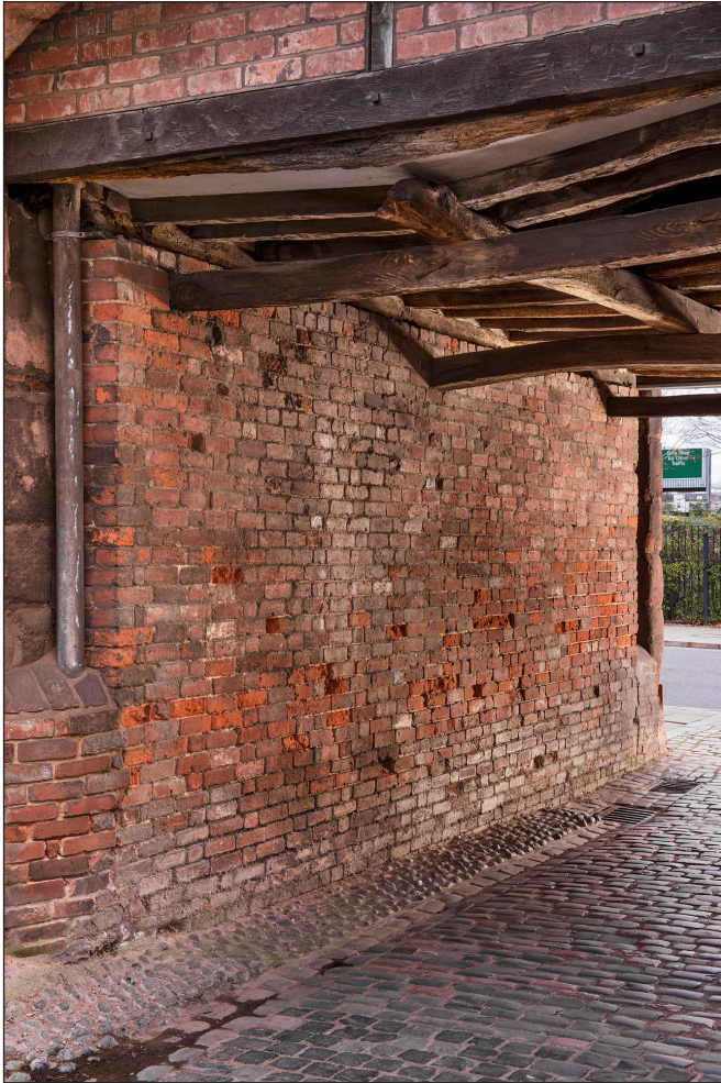
Figure 39 Exterior, south wall of passageway showing brick reconstruction. [DP219944]
