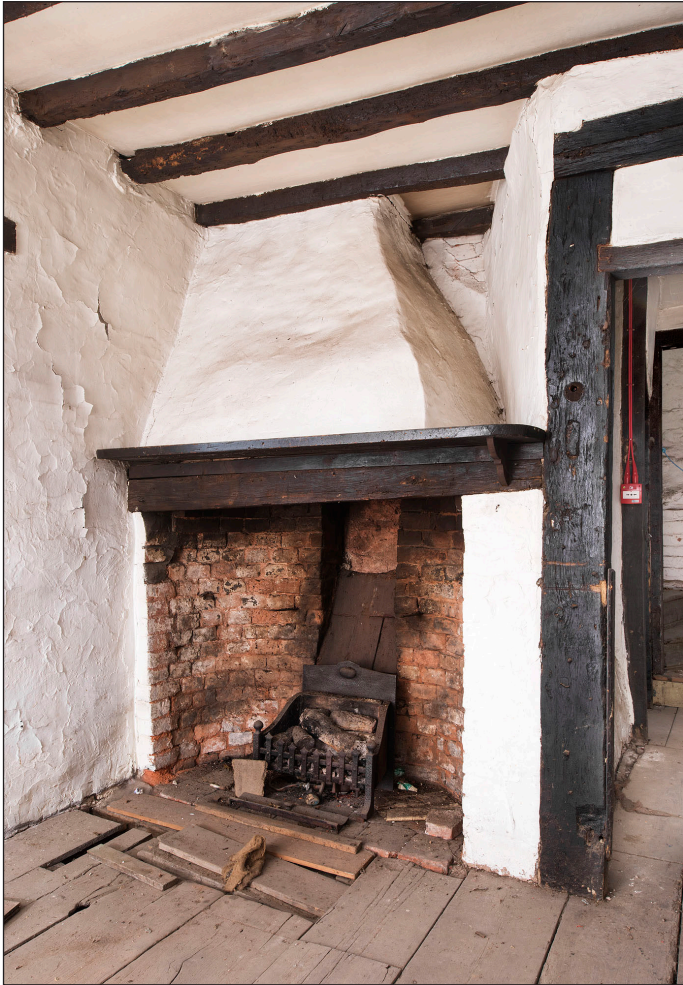
Figure 37 Interior, first floor, north room, detail of inserted fireplace. [DP219903]
