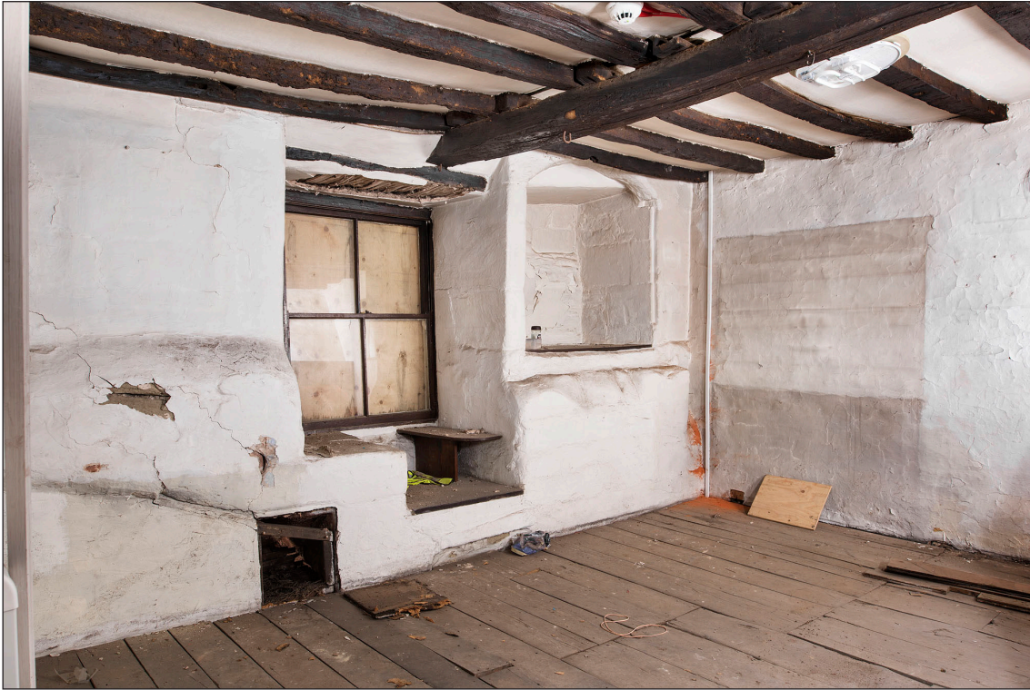
Figure 15 Interior, west elevation, first floor, north room. [DP219900].
