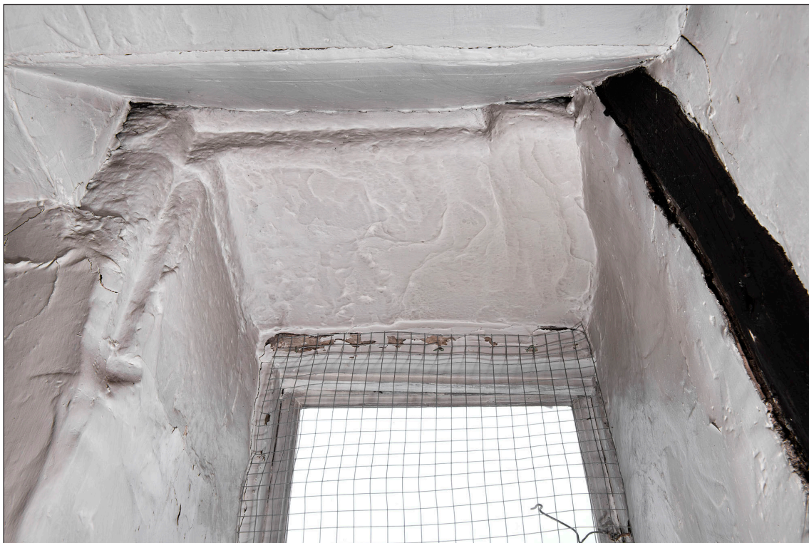
Figure 24 Interior, east elevation, first floor, north room, showing rebate around high-level window opening. [DP219930]
