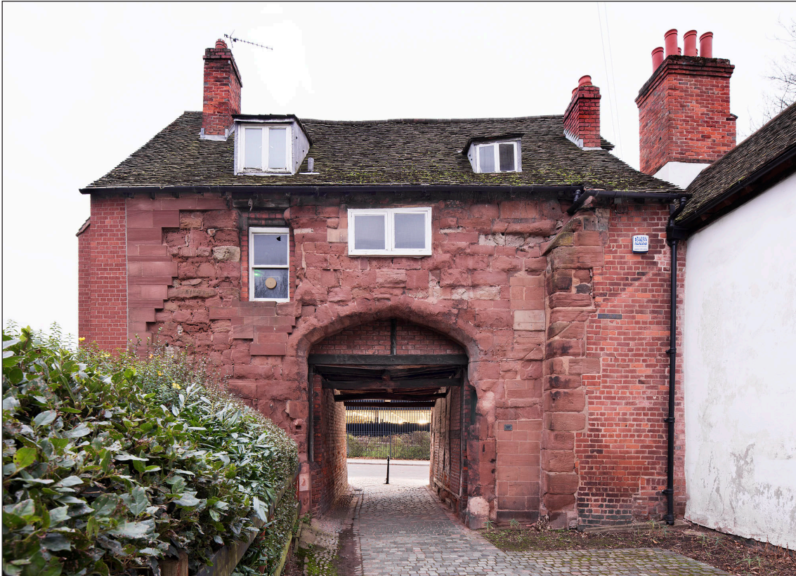
Figure 10 East elevation showing the main archway, the blocked north doorway and the truncated chimney stack. The south doorway is obscured. [DP219945]
