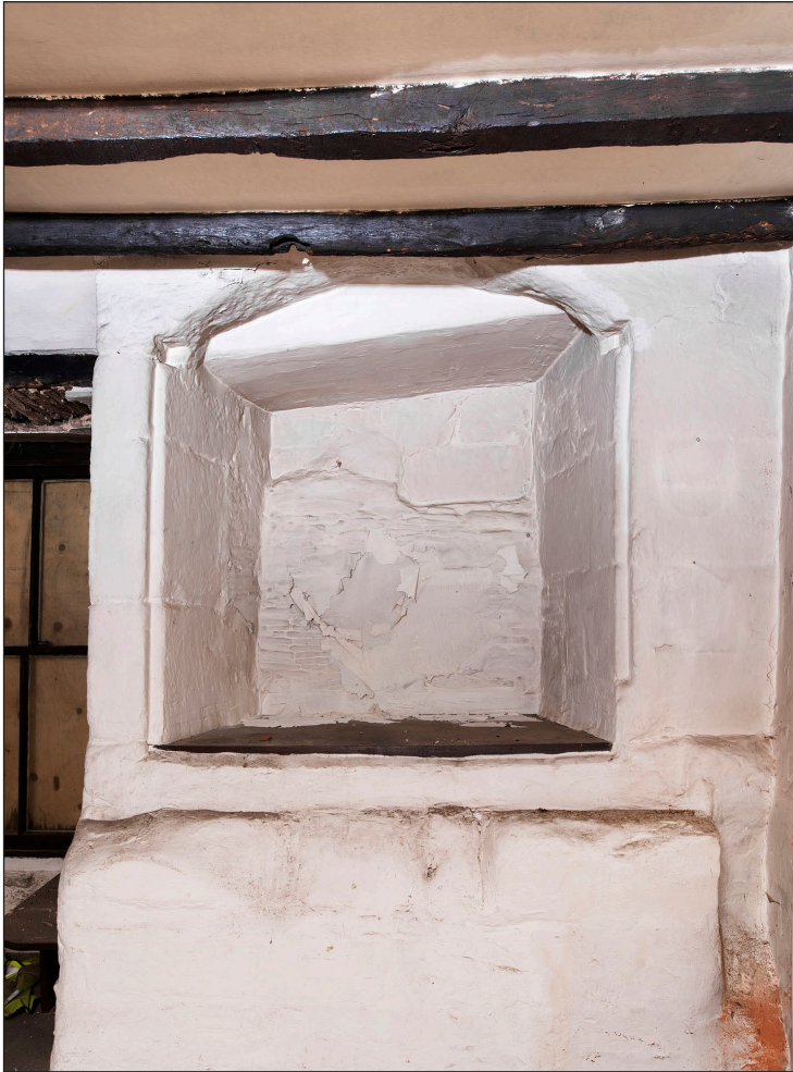
Figure 16 Interior, west elevation, first floor, north room, detail of cupboard. [DP19904]
