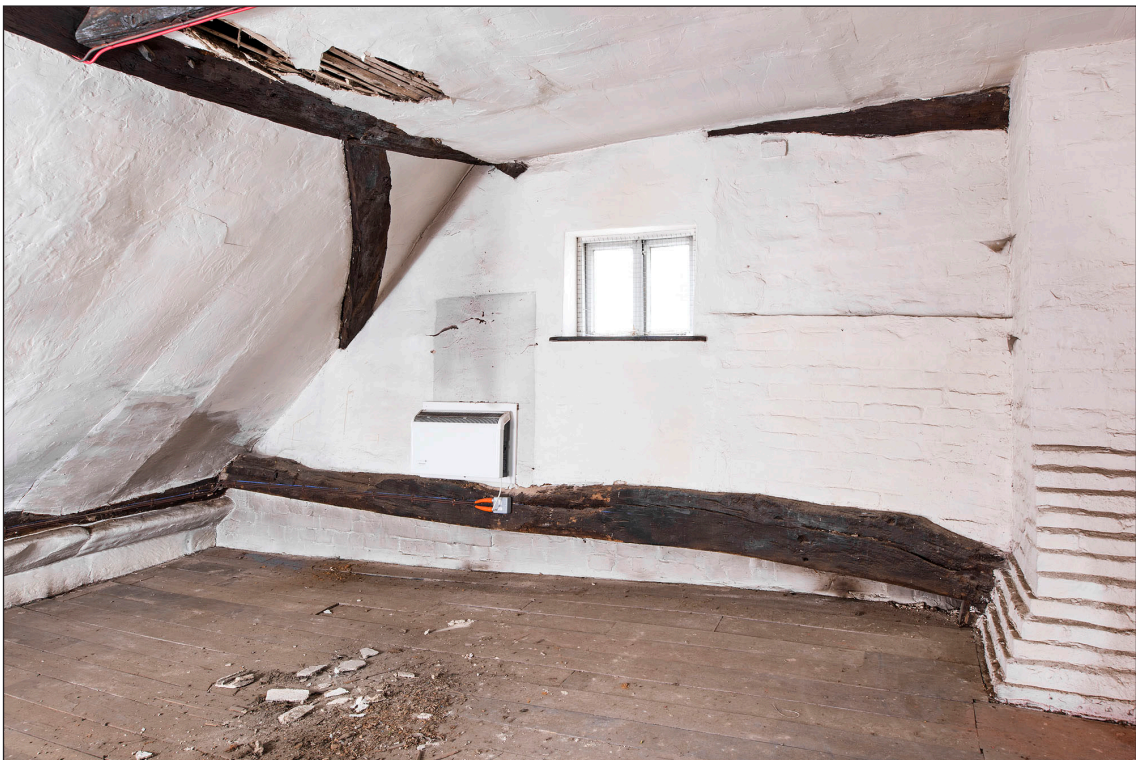
Figure 34 Interior, second floor, north room, showing northern truss. [DP219896]
