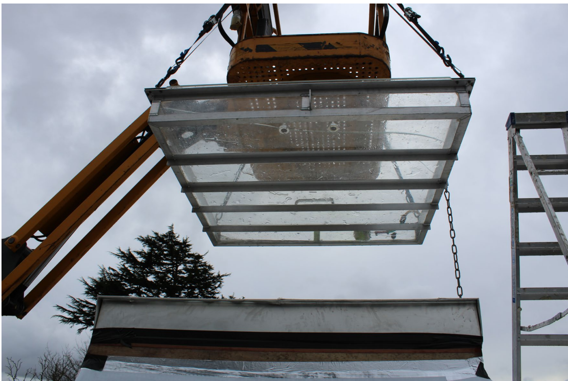
Photo B3: Water tank suspended below mobile platform before being put in position
