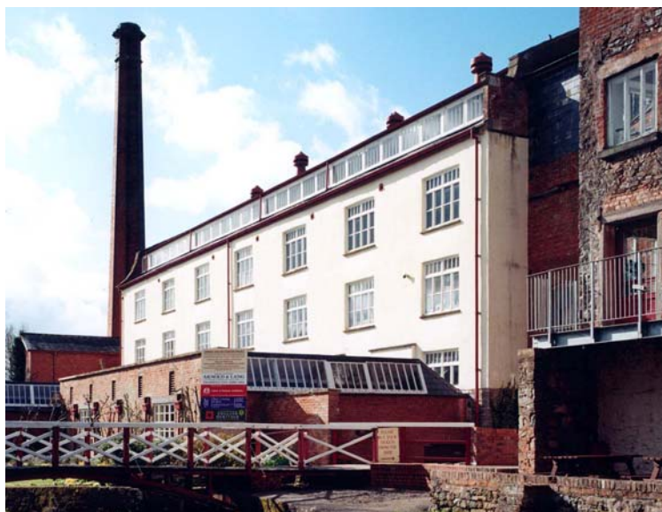
Fig 3. The main mill from the south east. The lower three storeys date from c1800.
