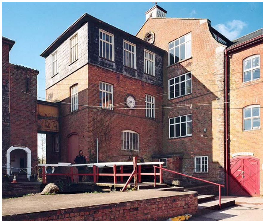
Fig 13. The wheelhouse from the north east.
