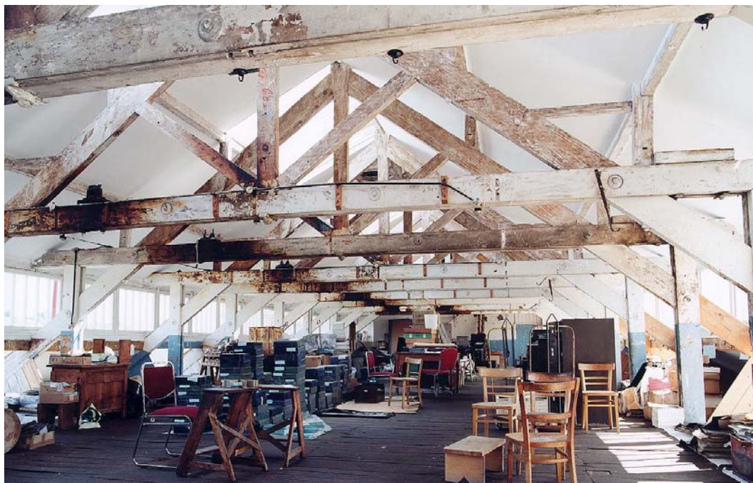
Fig 9. The attic from the west end.
