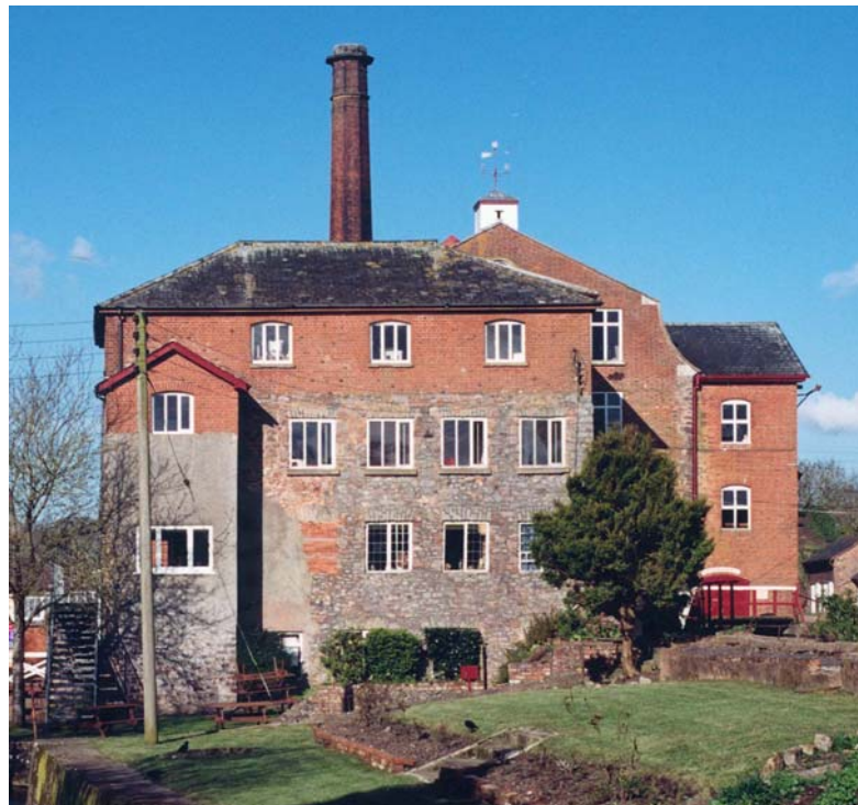
Fig 2. The grist mill from the east. Parts of the lower walls and the north end probably date from before c1800.
