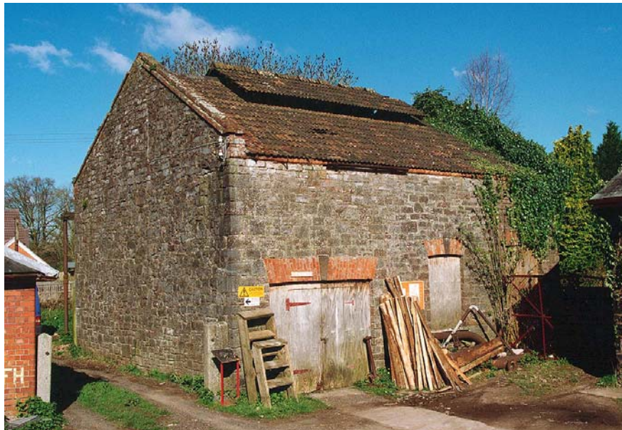
Fig 20. The gas retort house.
