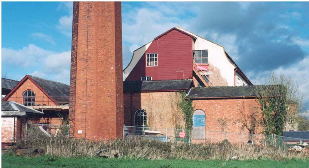
Fig 14. The west end of the site, showing (L – R) the economiser, boiler house, chimney, beam-engine house, rope race and beam-engine house extension.
