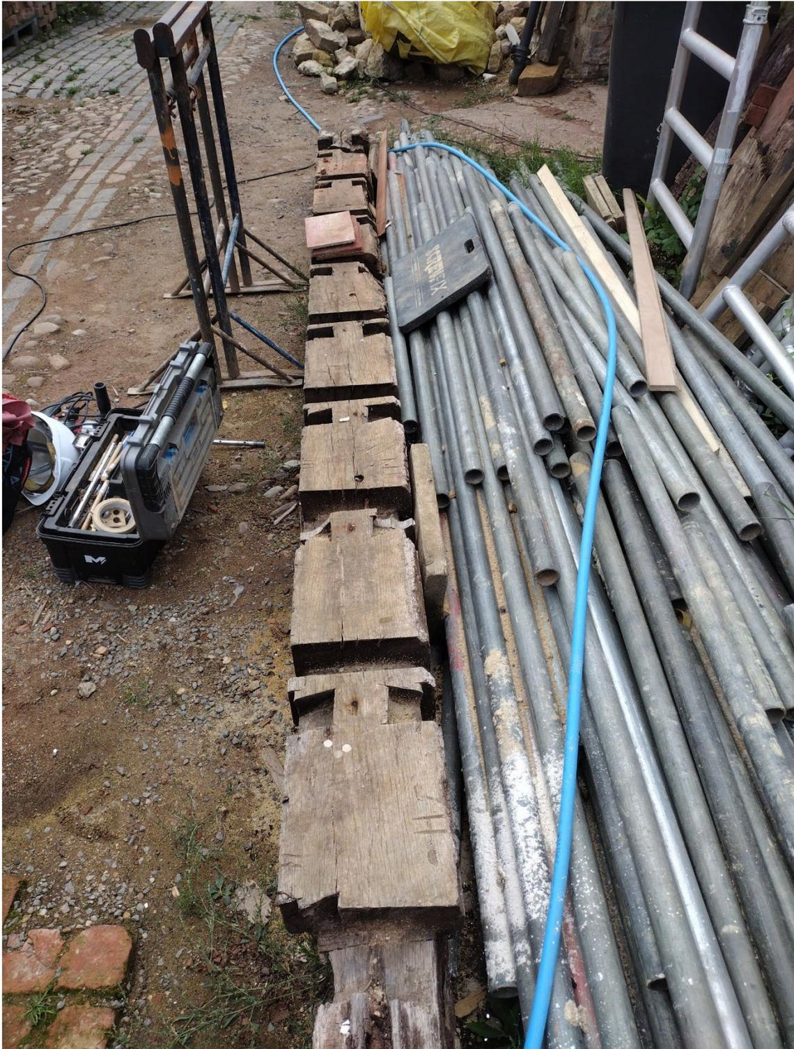
*Figure 4: The ex situ cellar beam, showing the half dovetail joist housings and sapwood on the top right corner of the beam (photograph Martin Bridge)*
