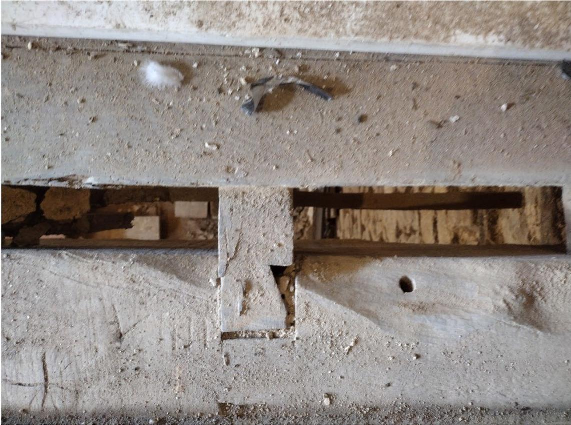
*Figure 3: View from above of the floor beam (tows02) showing the sample hole in the complete sapwood, and the half dovetail joint between the joist and the beam, found also in the tiebeams and the cellar beam (photograph Martin Bridge)*
