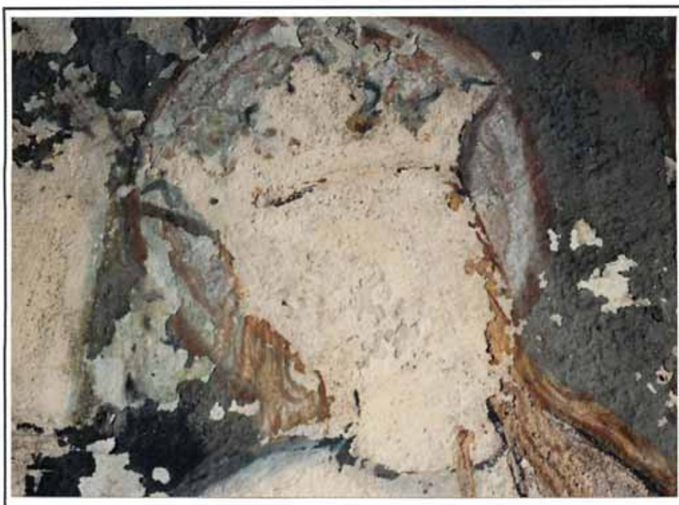
Plate 6: Horsham St Faith Priory. Foundation Scenes: detail of St Faith. Flaking of the paint layer ( whether related to the original technique or to added materials ) is aggravated by the cycling of salts. Fixatives ( sizes ) have been applied here, but have not 'taken' - probably due to the high moisture content of the surface [ see JAMES 1988 ].
