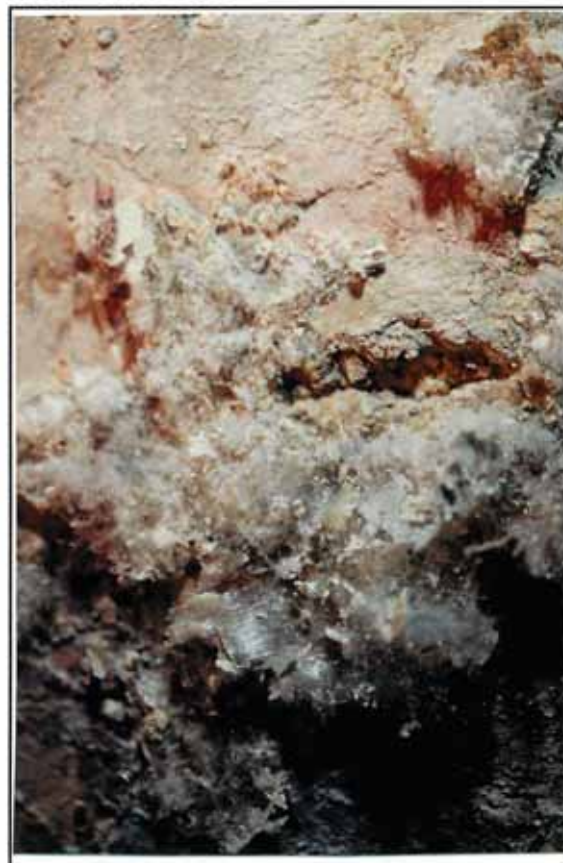
Plate 3: Cleeve Abbey; detail of masonry pattern in dorter. Less soluble salts cause disruption ( such as powdering and flaking ) of the paint layer and even of the render during cycles of crystallisation and solubilisation [ see MATTEINI 1991 ].
