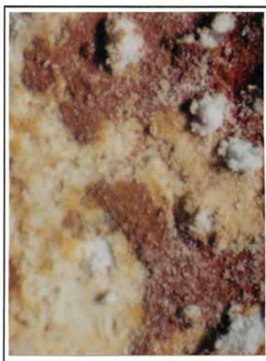
Plate 7: Horsham St Faith Priory. Detail of Foundation Scenes. The growth of salt crystals in the pores of the render can cause pitting and spalling of the paint layer [ see ARNOLD + ZEHNDER, 1991 ].
