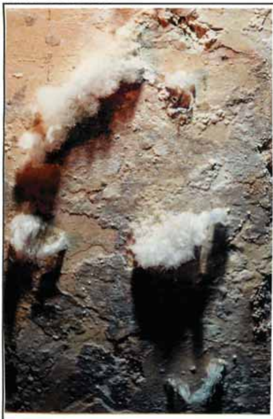
Plate 2: Cleeve Abbey; detail of the masonry pattern in the dorter. Very soluble salts can form efflorescences on the surface of the painting; the type of efflorescence is governed by environmental conditions as well as salt type [ see ARNOLD + ZEHNDER, 1991 ].
