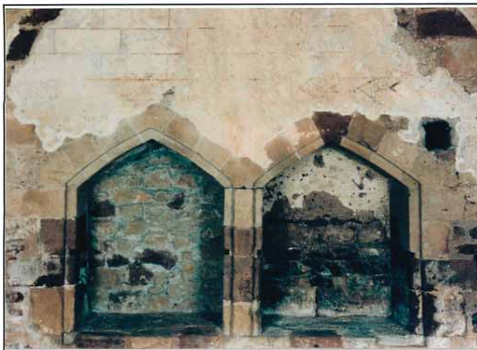
Plate 13: Cleeve Abbey, Somerset: south wall of Sacristy. Environmental monitoring of the ambient conditions in the sacristy suggests that the west side of the wall receives considerably more radiant energy than the east side, especially in spring ( note that no surface temperature measurements were made at this site ). It is arguable that this differential is at least implicated in the selective way the painted border has altered.
