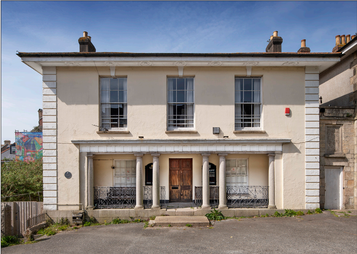
Figure 2: The former Redruth Savings Bank in 2021. [DP276704]
