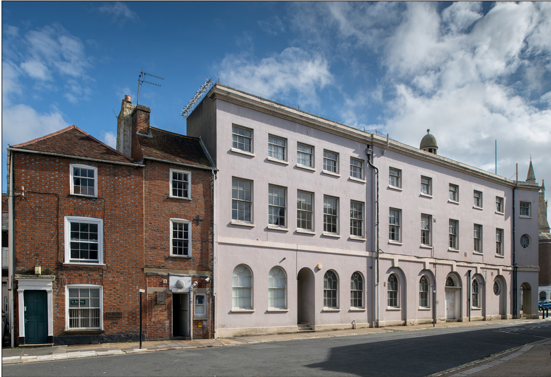
Figure 4: The Quay Street elevation, looking south-west. [DP301380]
