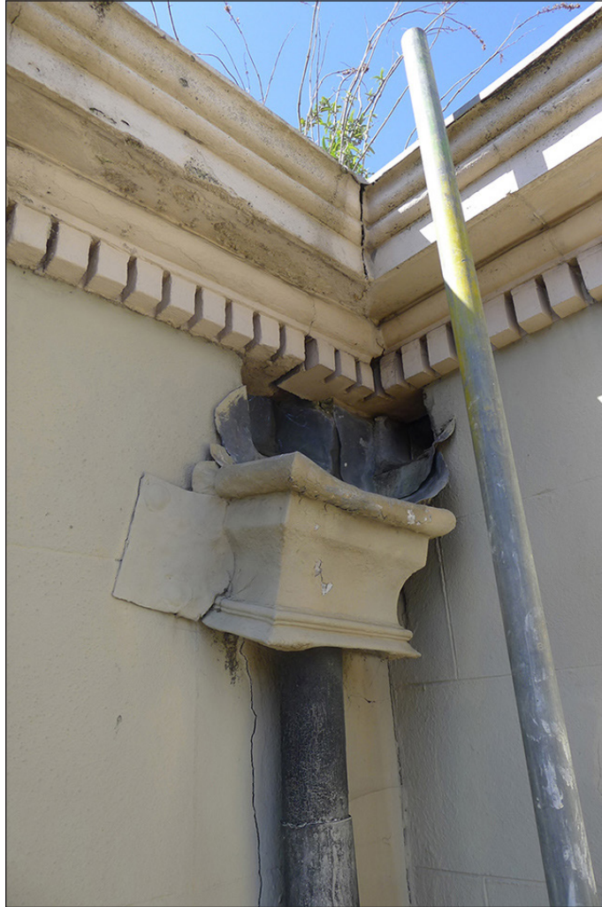
Figure 35: The historic lead hopper and lead downpipe in the angle of the High Street elevation. [Photograph by Oxley Conservation Ltd]
