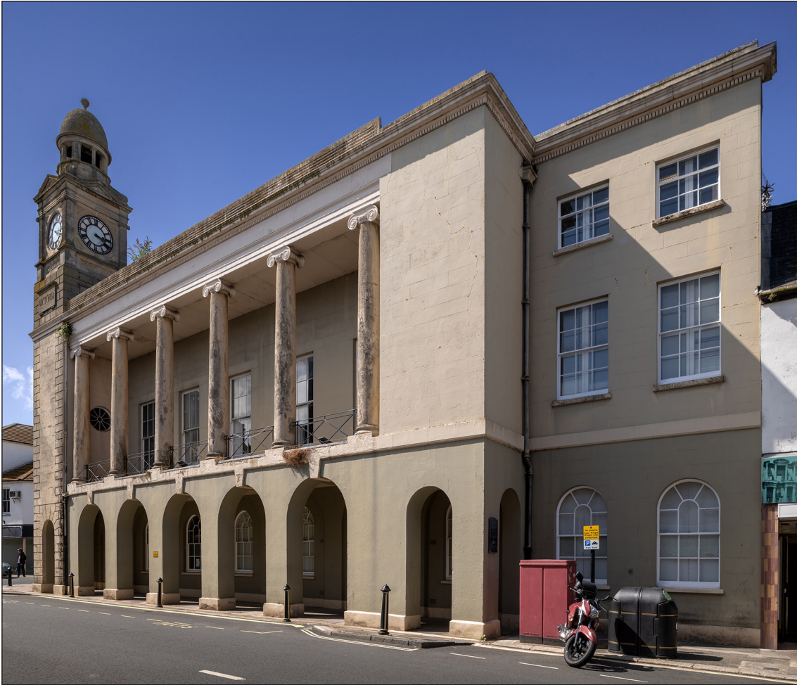
Figure 3: The south elevation from the south-east. [DP301379]
