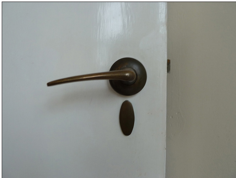
Figure 42: A 1960s door handle with keyhole escutcheon and cover in a first-floor office facing Quay Street.
