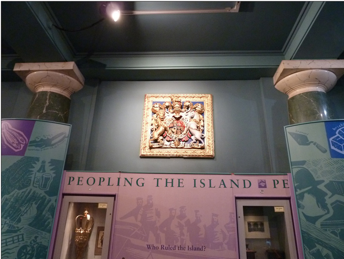
Figure 28: The fibrous plaster columns of 1957-8 in their positions of 1967-8. (The Newport coat of arms is part of the Museum collections and has no historic link to the Guildhall.)
