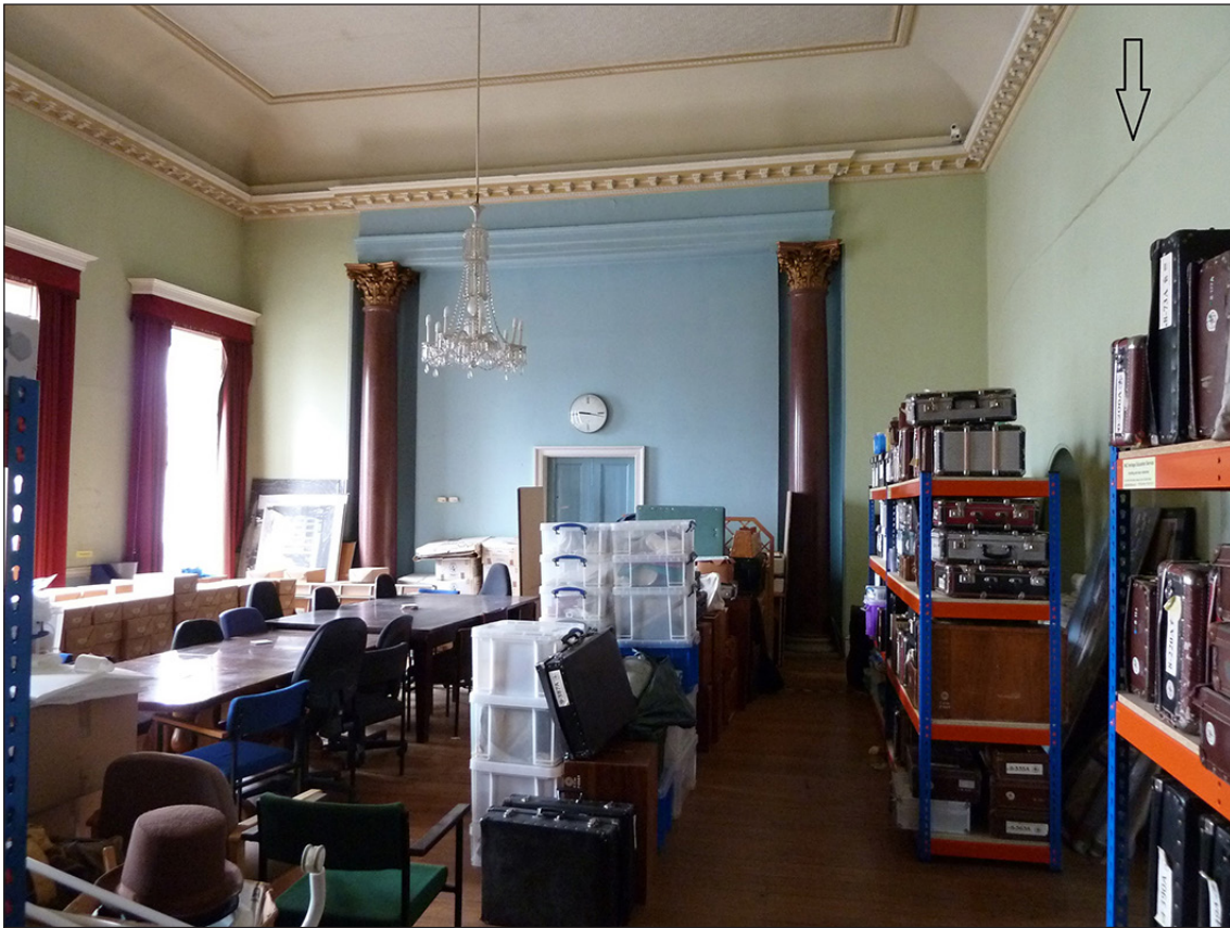
Figure 17: The Town Hall room, with an arrow pointing out the horizontal feature which may relate to a former balcony or gallery in this room.
