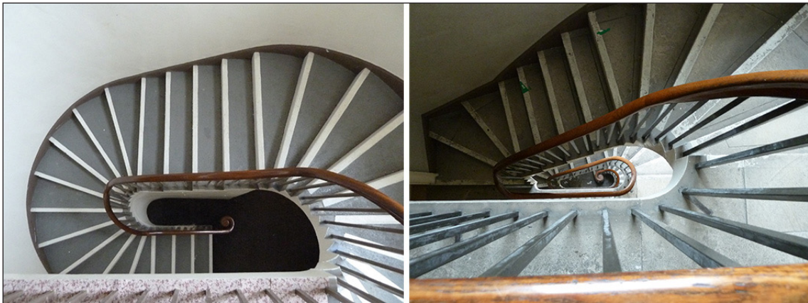
Figure 37: The principal staircase photographed from the first floor looking down (left); and the smaller staircase, looking down from the second floor (right).
