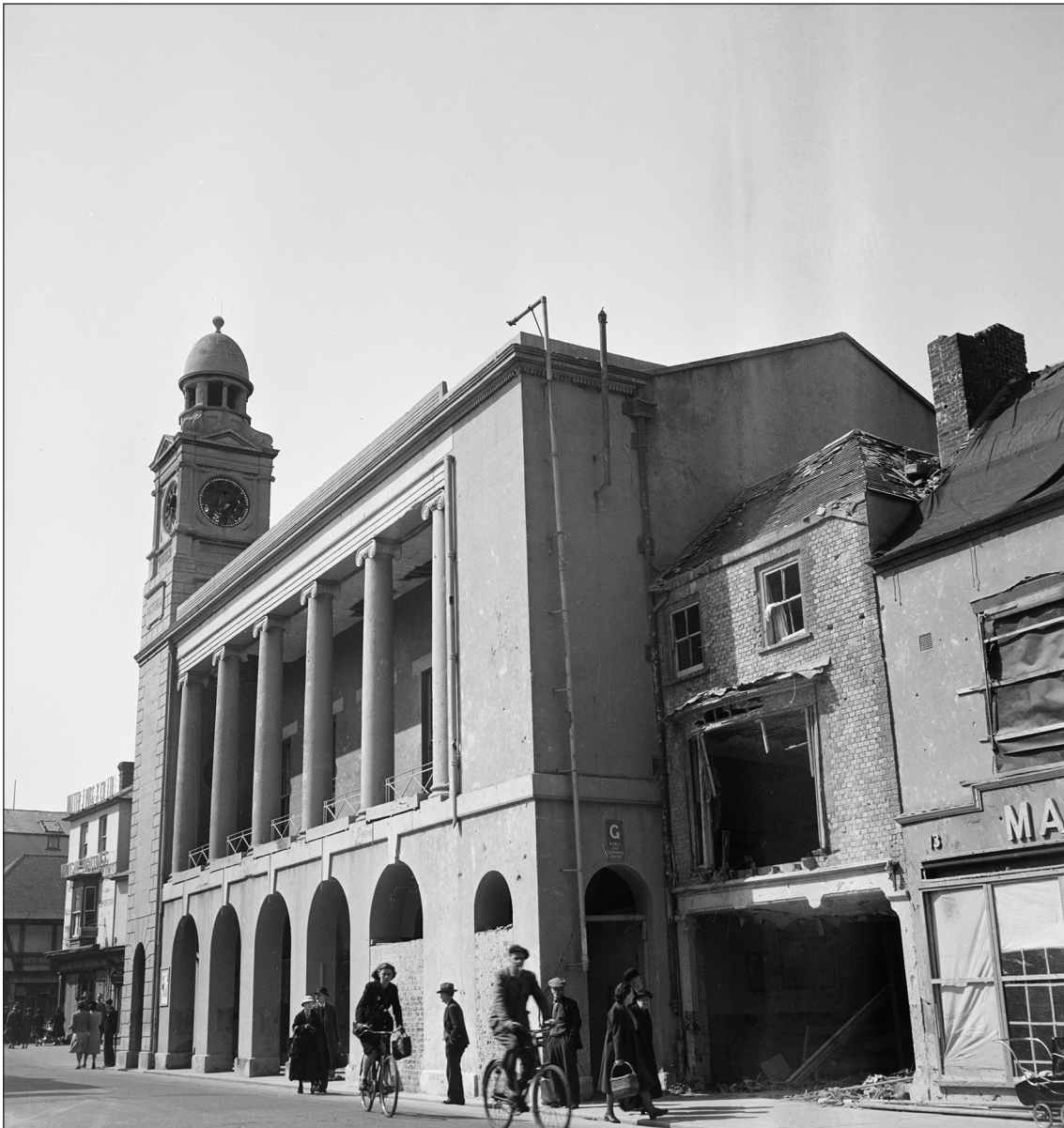
Figure 23: The Guildhall and 136 High Street in a photograph taken by O. G. S. Crawford in the winter of 1943-4. [AA53/04334]
