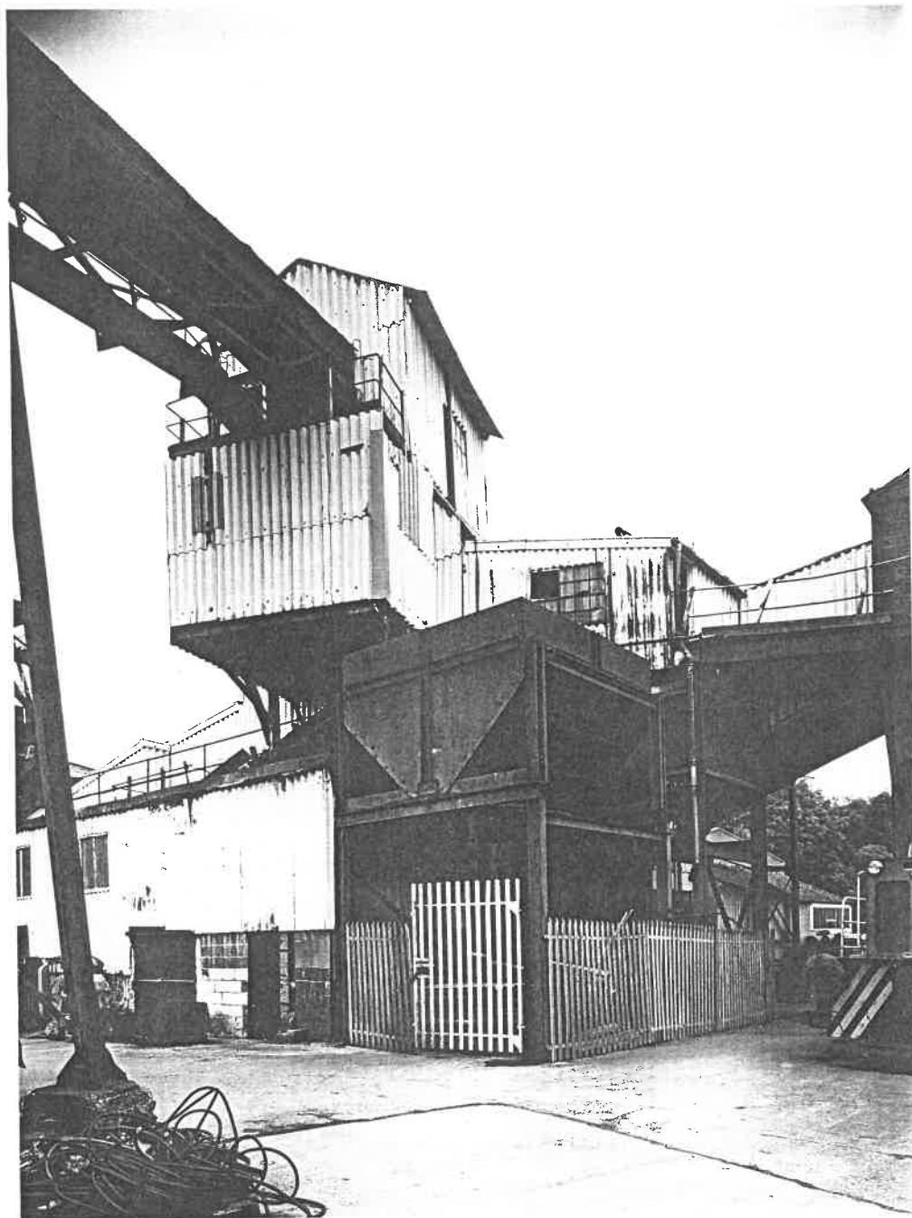
Fig 30 Caphouse Pit. Detail of screens building and associated bunkers, with conveyor from drift approaching from left. RCHME AA97/4976.
