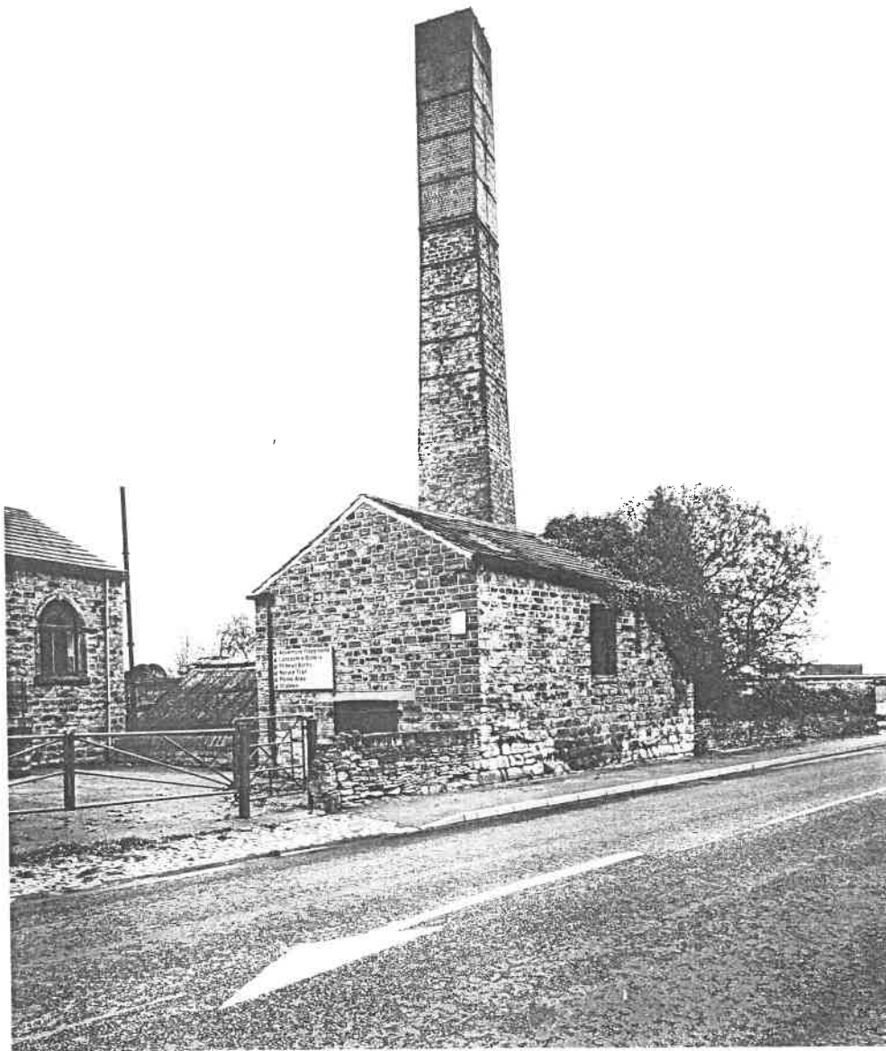
Fig 26 Caphouse Pit. Store adjacent to entrance yard in front of steam winding engine house. RCHME AA97/4969.
