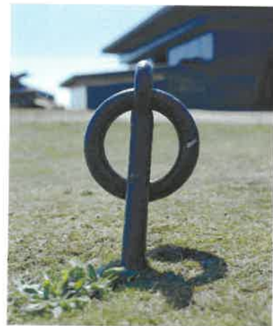
Figure 52 No III gun: one of the metal ringbolts on the apron of the emplacement (NMR: AA051421)
