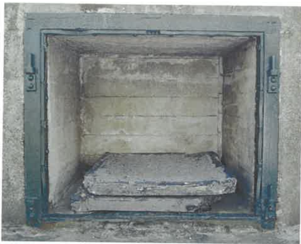
Figure 80 Second World War no 2 gun: two tiles of plastic armour inside an ammunition recess; the tiles formed part of the anti-strafting cover above the gunhouse (NMR: AA051397)
