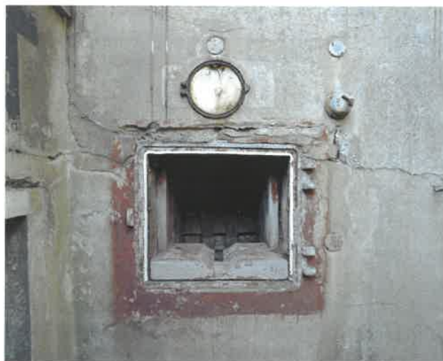
Figure 26 No II gun: the opening for the band lift which brought cartridges up from the magazine below; note the electric light fitting above (NMR: AA051389)
