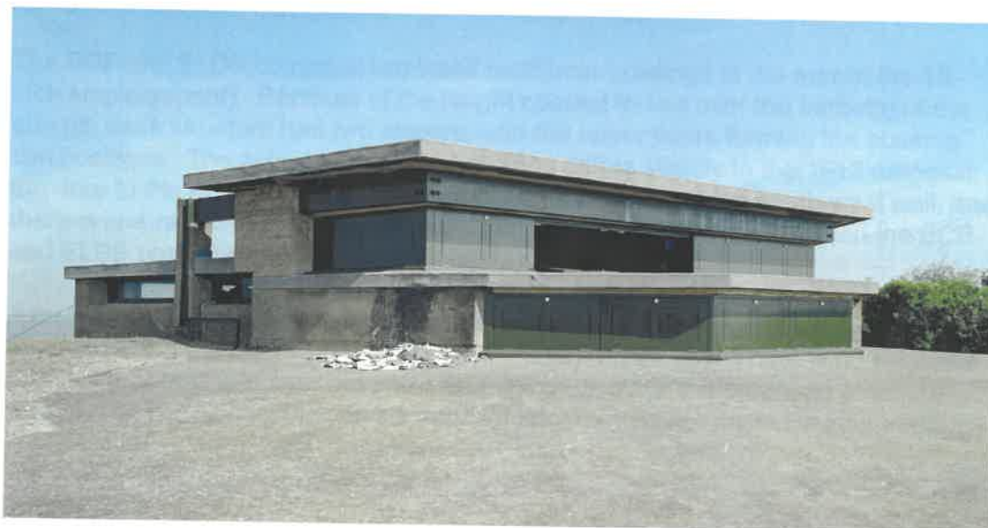
Figure 56 The CD BOP in the old 10-inch emplacement (NMR: AA051372)
