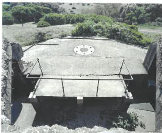
Figure 29 No II gun: the concrete platform inserted after the removal of the 6-inch gun in 1943 (left); and detail of the holdfast (right) (NMR: AA051392/AA051388)
