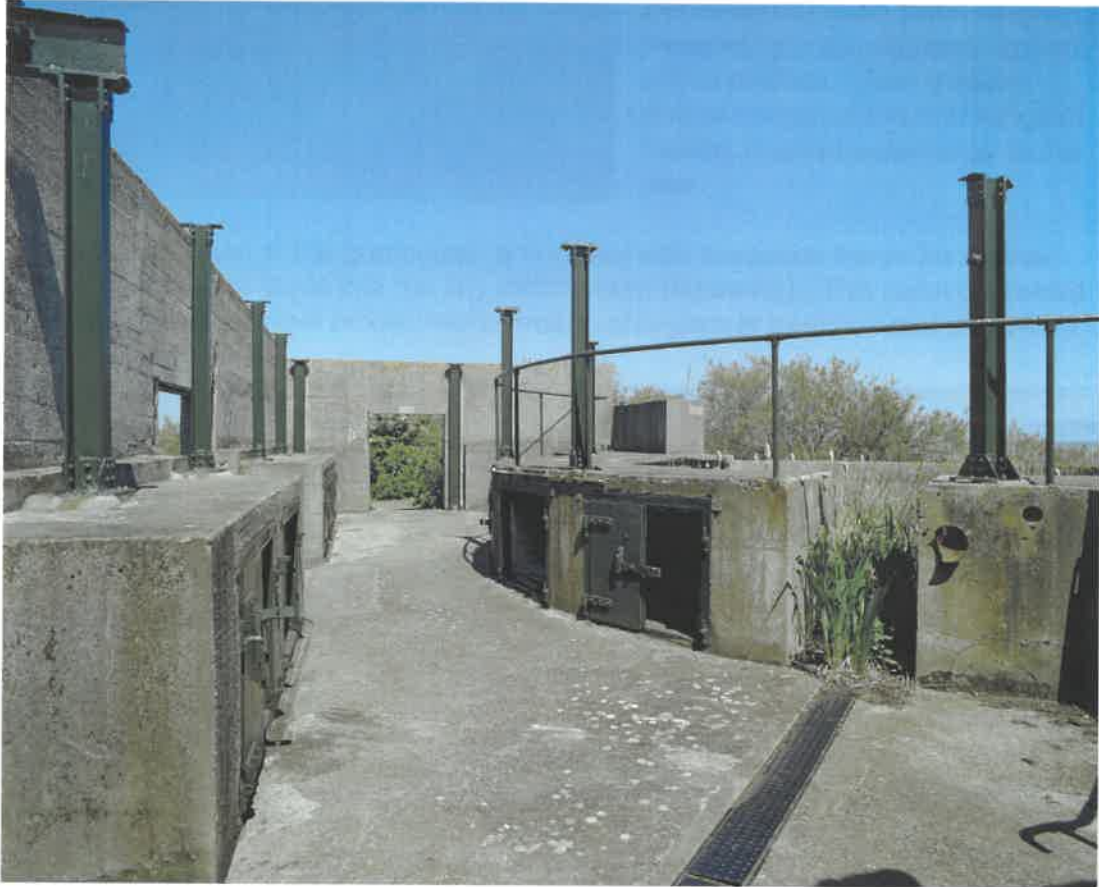
Figure 79 Second World War no 2 gun: the gunhouse, with the raised gun floor to the right and the remaining piers which supported the anti-strafting cover (NMR: AA051401)
