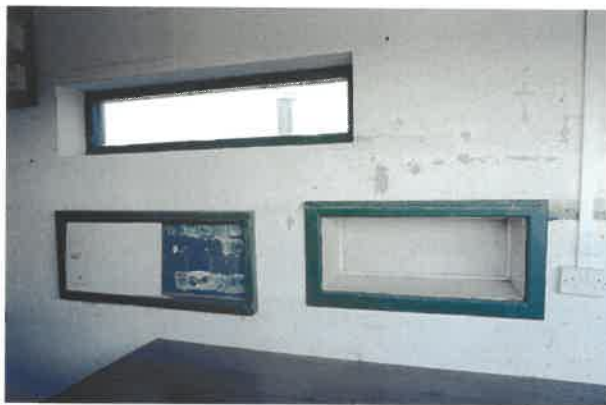
Figure 59 CD BOP: communication hatches between the rooms (NMR: AA051374)
