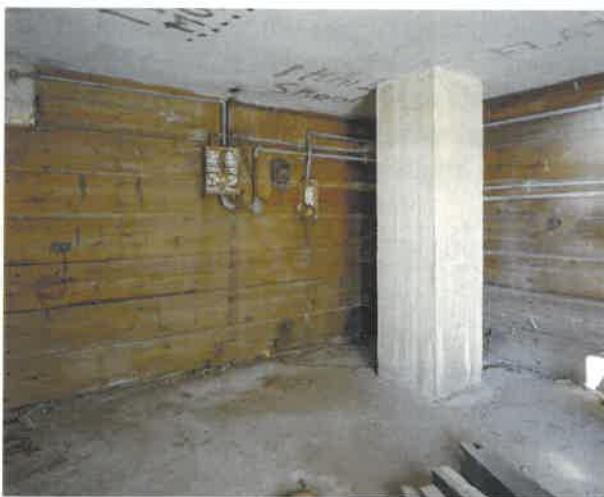
Figure 64 CD BOP: the space (B) beneath the BCP post, showing the base of the 1913/14 DRF pillar and wooden panelling which supported electric wiring and fuse boxes (NMR: AA051417)
