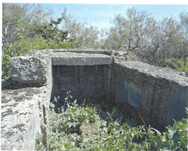
Figure 93 Position-finding cell: the remains of the structure (NMR: AA051428)
