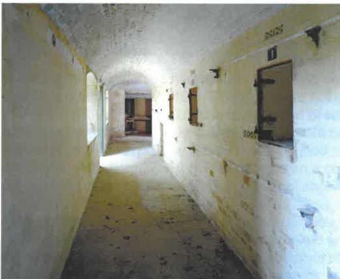
Figure 43 6-inch Magazine: the corridor of the magazine, looking towards Shell store 2. The lamp recesses and issue hatch are for Cartridge store 2; the remains of brackets for later shelving are also visible (NMR: 051406)
