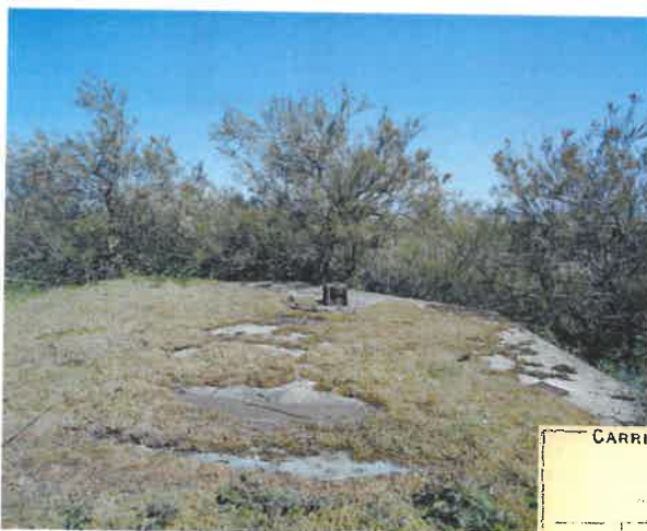
Figure 91 Practice Battery: one of the Vavasseur emplacements, heavily overgrown (left) (NMR: AA051430) and a detailed elevation of the garrison carriage for a 5-inch Vavasseur Mk II, very similar to the 6-inch variety (right) (Treatise on Military Carriages, War Office, 1911)
