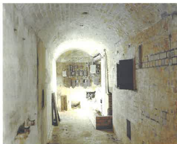
Figure 69 10-inch Magazine: the corridor, showing the doors of the lamp recesses in the right-hand wall (NMR: AA051440)
