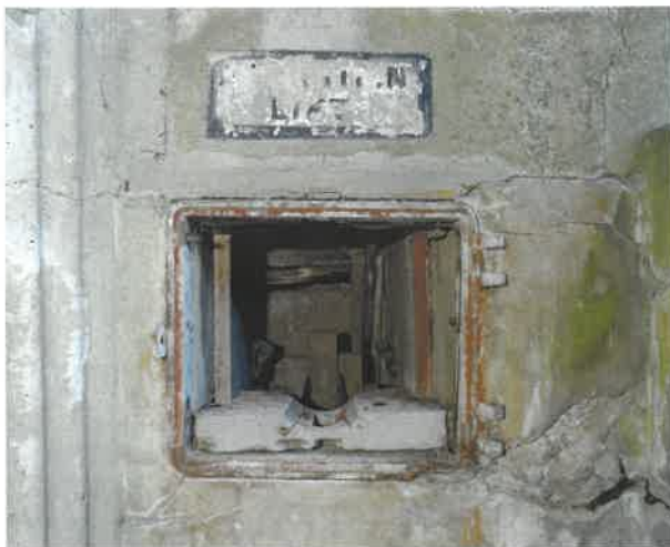
Figure 17 No 1 gun: the opening at gun floor level for the band lift which transported cartridges from the magazine (NMR: AA051380)
