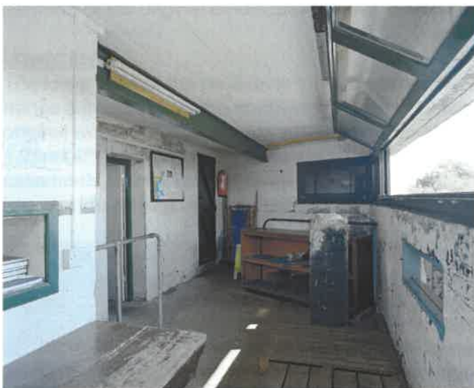
Figure 61 CD BOP: interior view, with (at right) the observation embrasure across the front wall (NMR: AA051373)
