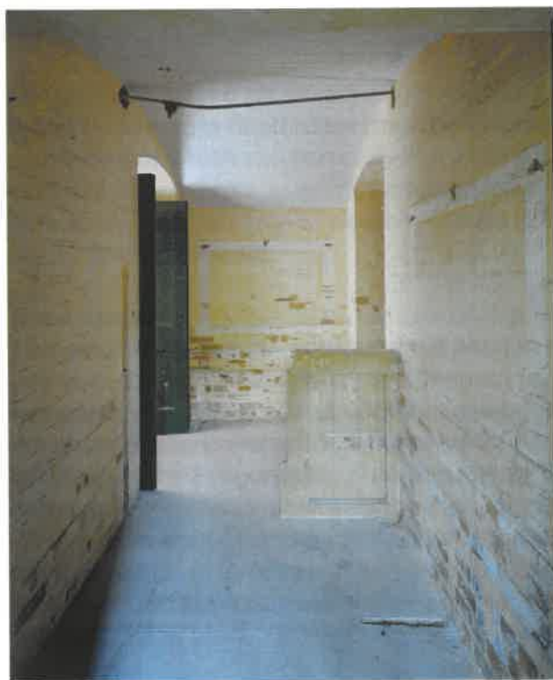
Figure 47 6-inch Magazine: the shifting lobby, with the entrances to both cartridge stores at the far end beyond the remains of the wooden shifting barrier (NMR: AA051412)
