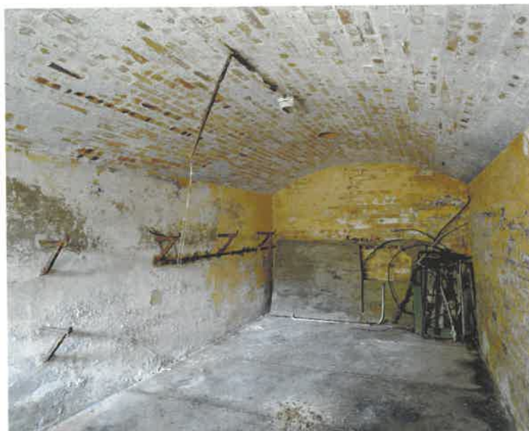
Figure 74 The Artillery Store for the 10-inch gun (NMR: AA051437)
