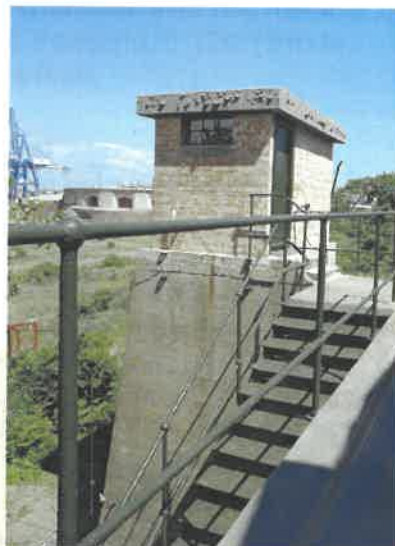
Figure 30 BC Post: view from the south- west, with Landguard Fort in the background (NMR: AA051385)
