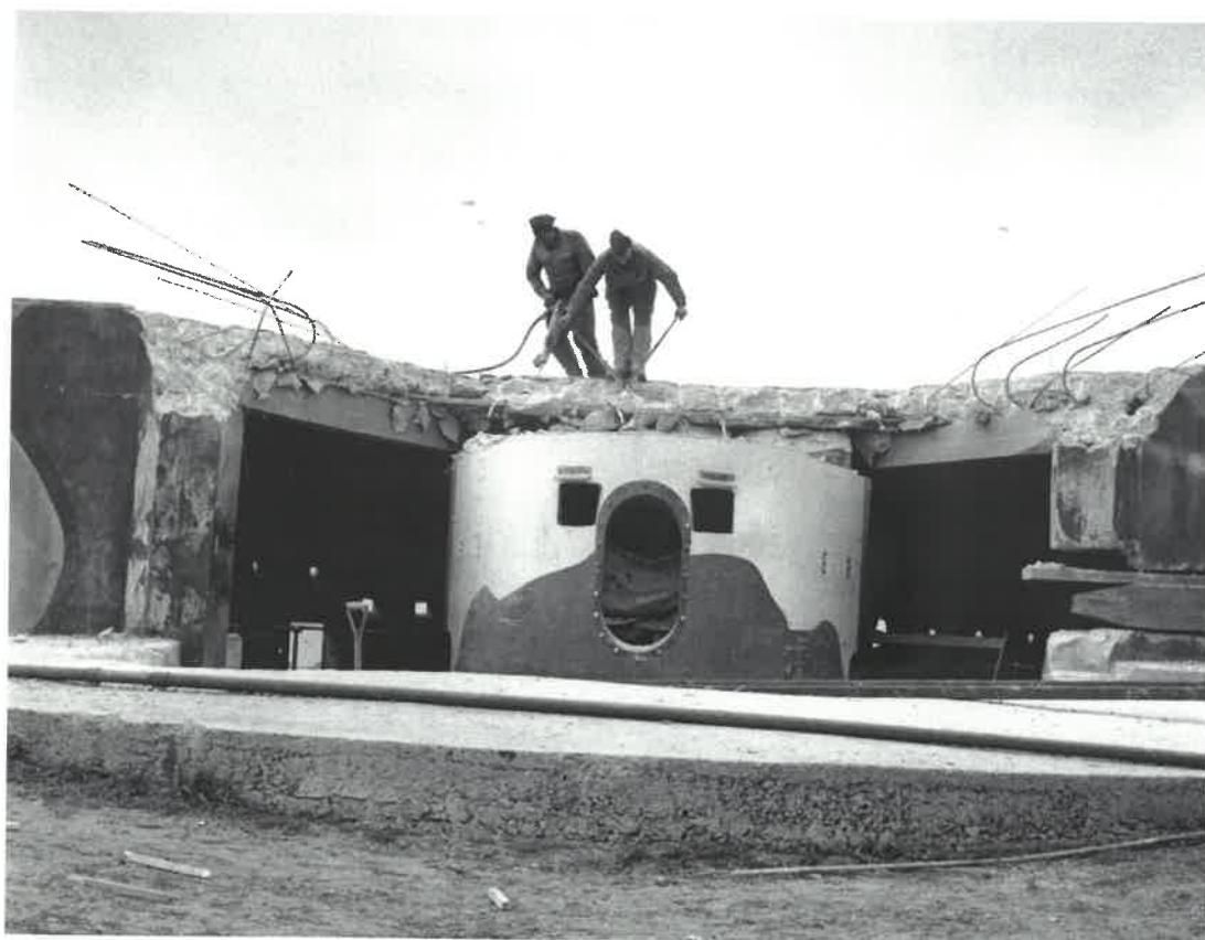
Figure 28 No II gun: Royal Engineers breaking the casemate in order to remove the gun in 1943; note the wooden prop on the right-hand side of the casemate, probably associated with the removal of the gun (IWM: H28717; reproduced with the kind permission of the Imperial War Museum)
