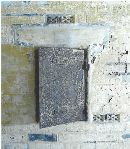
Figure 44 6-inch Magazine: lamp recess door in the corridor of the magazine (NMR: AA051420)
