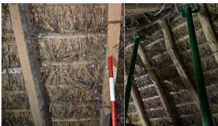
Figure 1 Contrasting rafters with square cut beams in the phase 1a extension (left) and more roughly shaped beams of the original roof (right).
