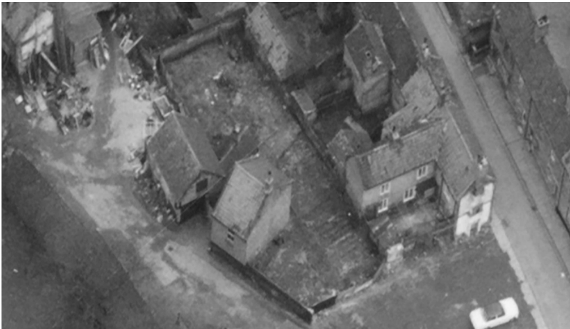
Fig 18: Part of the Ship Yard area in 1968 showing evidence of demolition and dereliction. The former interior wall of a house on Vicarage Street (showing white) can be seen bottom right of the image. Detail of MAL/60068 159 24-FEB-1968. Photo by Meridian Airmaps Ltd. Copyright Norfolk County Council.
