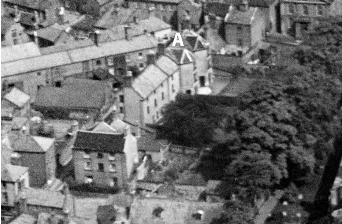
Fig 43: The vicarage and associated houses to the north of the church seen from the west in 1928. The vicarage is marked A, Vicarage Street runs diagonally from the bottom left, the churchyard is to the right. Detail of EPW021294 MAY 1928 © Historic England (Aerofilms Collection).
