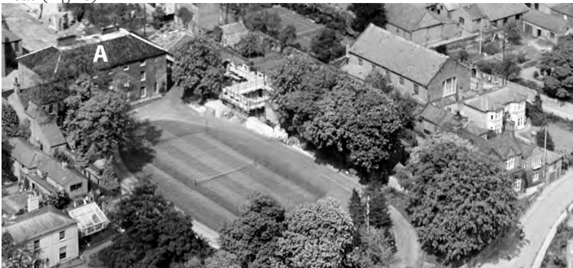
Fig 78: The southern part of Paston Grammar School site seen in 1928 from the south-west, with Grammar School Road bottom right. The letter A marks the main school building (the Nelson Building). Detail of EPW021292 MAY 1928 © Historic England (Aerofilms Collection).
