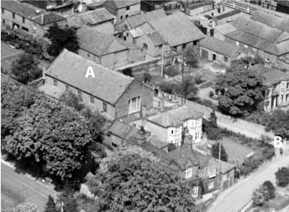
Fig 91: The southern end of Bank Loke in 1928. The letter A marks the hall, B marks the southern entrance to Bank Loke. Grammar School Road is bottom right. Detail of EPW021292 MAY 1928 © Historic England (Aerofilms Collection).
