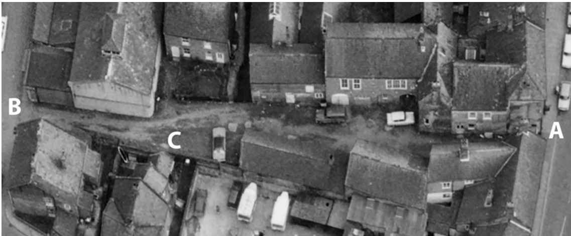
Fig 37: Old Bear Yard looking east in 1968. The letter A marks the entrance from Market Street, B the entrance from Vicarage Street. C marks an area of demolition; compare with Fig 35. Detail of MAL/68006 146 24-FEB-1968. Photo by Meridian Airmaps Ltd. Copyright Norfolk County Council.
