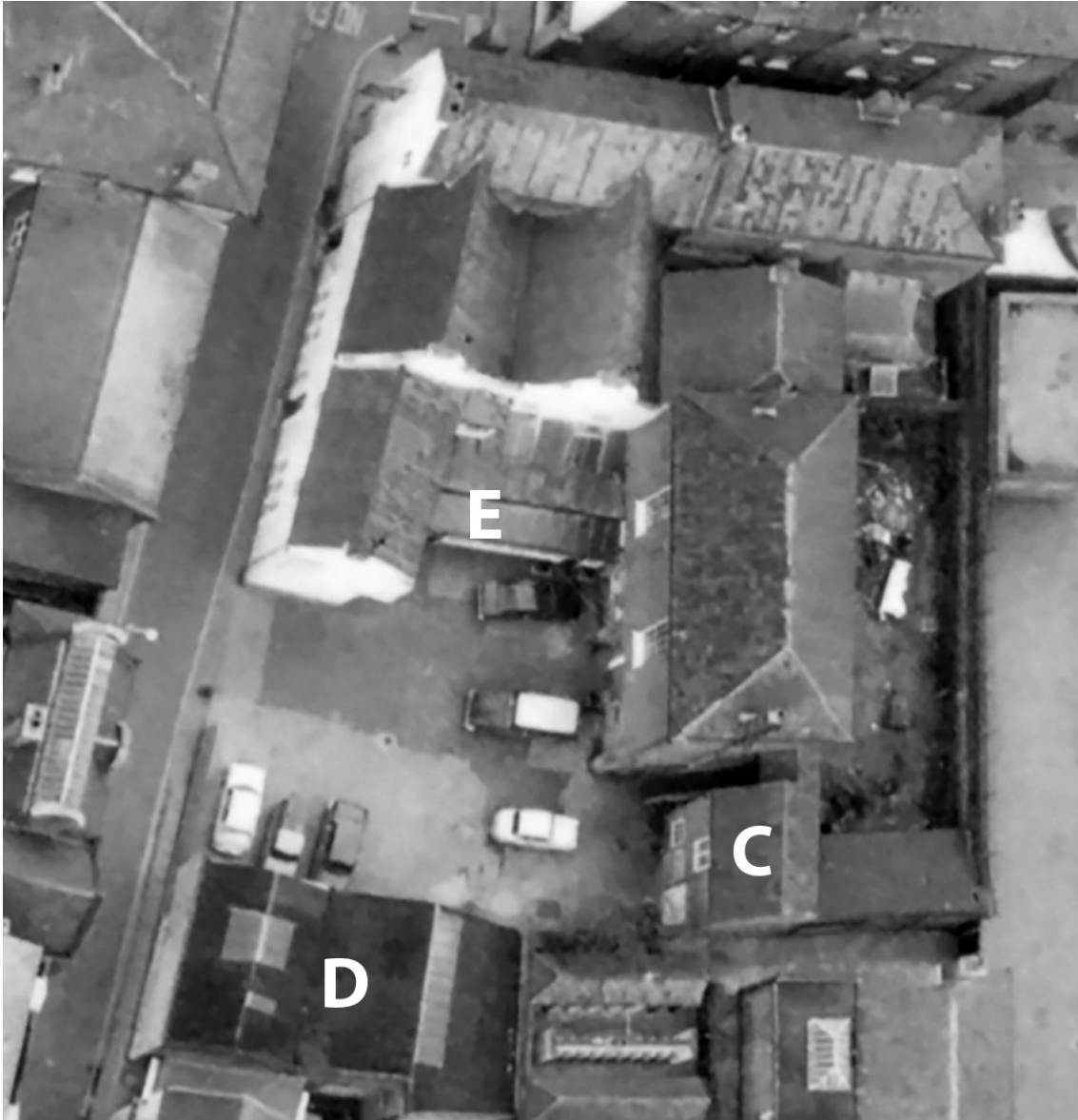
Fig 74: The King's Arms Hotel in 1968 showing the opened-out yard creating a car park and the new buildings (C and D) and the extension (E). Detail of MAL/68006 157 02-FEB-1968. Photo by Meridian Airmaps Ltd. Copyright Norfolk County Council.
