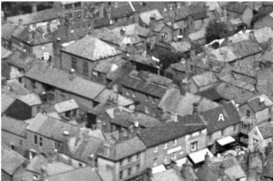
Fig 8: Mitre Tavern Yard seen from the south-west in 1928. The letter A is 6 Market Place and the entrance to the yard is below the A and to the left of the awning. The yard extended to a junction with Vicarage Street marked B. Detail of EPW021295 MAY-1928 © Historic England (Aerofilms Collection).
