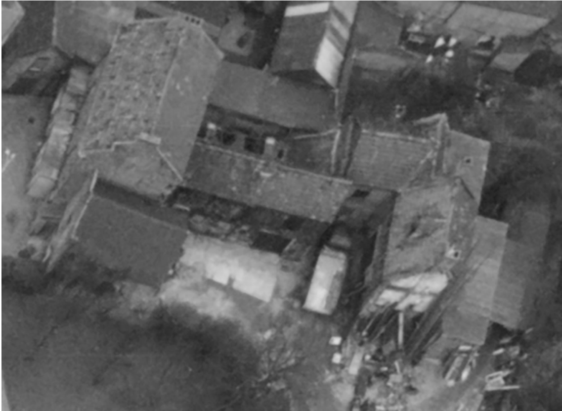
Fig 17: A view taken in 1968. The northern end of The Butchery is on the left of this image. The former interior wall of the terrace partially demolished in the 1930s can be seen showing white on the lower right side of the image. Detail of MAL/60068 159 24-FEB-1968. Photo by Meridian Airmaps Ltd. Copyright Norfolk County Council.
