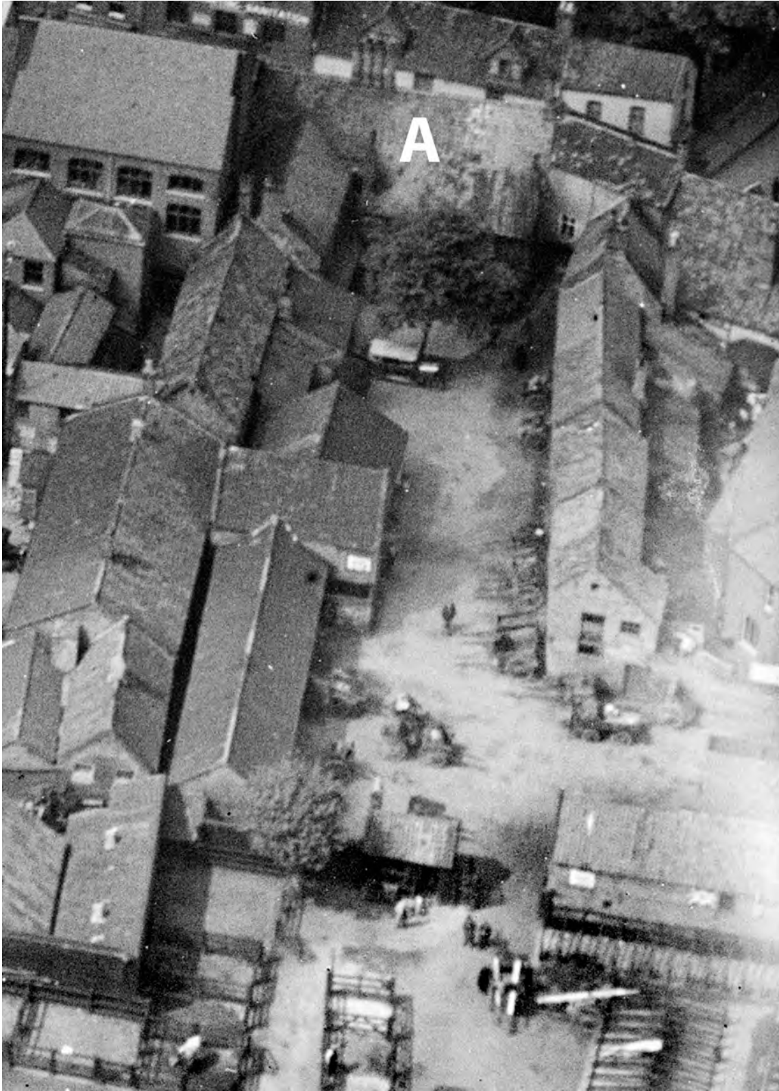
Fig 90: The Cross Keys Hotel yard and the Cattle Yard from the south taken in 1928. The Cross Keys Hotel is marked A. Detail of EPW021290 MAY 1928 © Historic England (Aerofilms Collection).
