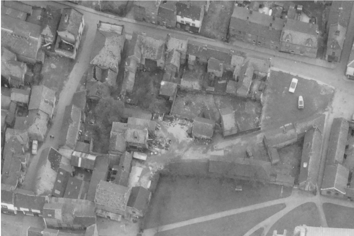
Fig 15: By 1968 the eastern end of the site had been demolished (the open area towards top right with two parked cars). This photograph also shows more clearly the derelict state of some of the buildings with some missing roof tiles. Detail of MAL/60068 158 24-FEB-1968. Photo by Meridian Airmaps Ltd. Copyright Norfolk County Council.
