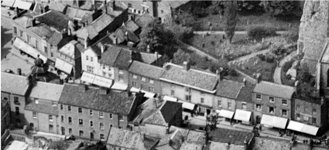
Fig 105: The central and western end of the Market Place from the south-east. Detail of EPW021290 MAY 1928 © Historic England (Aerofilms Collection).
