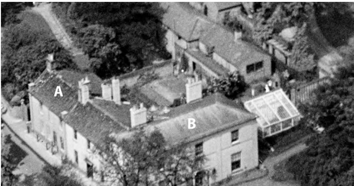
Fig 76: Buildings on King's Arms Street in 1928. Of these 15 Kings Arm's Street survives (A), its neighbour and the larger house at right angles to the road (B) and its greenhouse have since been demolished. Detail of EPW021292 MAY 1928 © Historic England (Aerofilms Collection).
