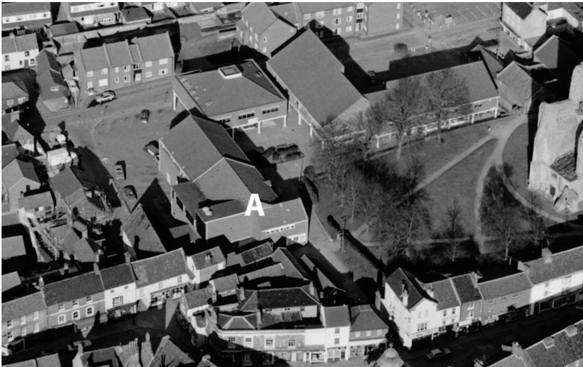
Fig 20: St Nicholas Court precinct in 1986. The buildings centred on A were built after 1972 (compare with Fig 19). Detail of TG2830/C/AZQ8 02-MAR-1986. Photo by D. Edwards Copyright Norfolk County Council.
