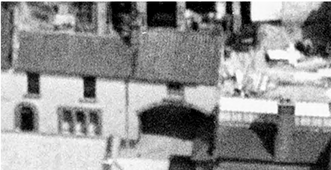
Fig 71: The archway into the King's Arms Hotel yard seen from the west. Detail of EPW021294 MAY 1928 © Historic England (Aerofilms Collection).
