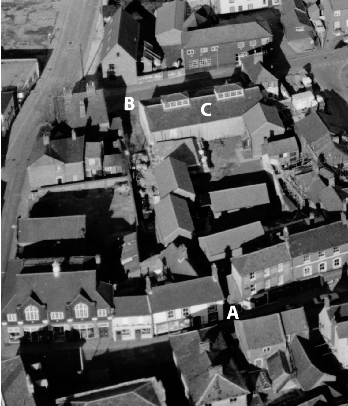
Fig 40: Old Bear Court housing development seen in 1986. The letter A marks the former entrance to Old Bear Yard from Market Street, B the former entrance from Vicarage Street. C marks the Church Rooms. Detail of TG2830/C/AZQ8 2-MAR-1986. Photo by D. Edwards Copyright Norfolk County Council.
