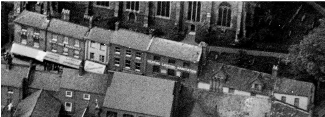
Fig 104: The eastern end of the Market Place from the south-east. Detail of EPW021290 MAY 1928 © Historic England (Aerofilms Collection).
