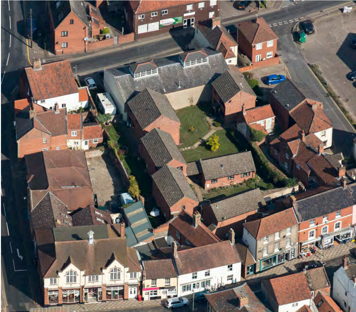
Fig 41: Old Bear Court on the site of Old Bear Yard seen in 2020. Detail of 33933_002 22-SEP-2020 © Historic England Archive.
