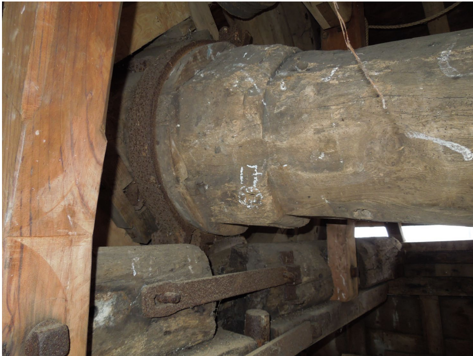
Figure 7: The windshaft, with the position of core kibw17 highlighted in chalk (photograph by Martin Bridge)
