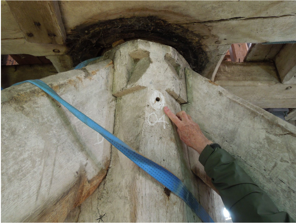
Figure 6: Position of the core from the main post (kibw04) being indicated. (photograph by Martin Bridge)
