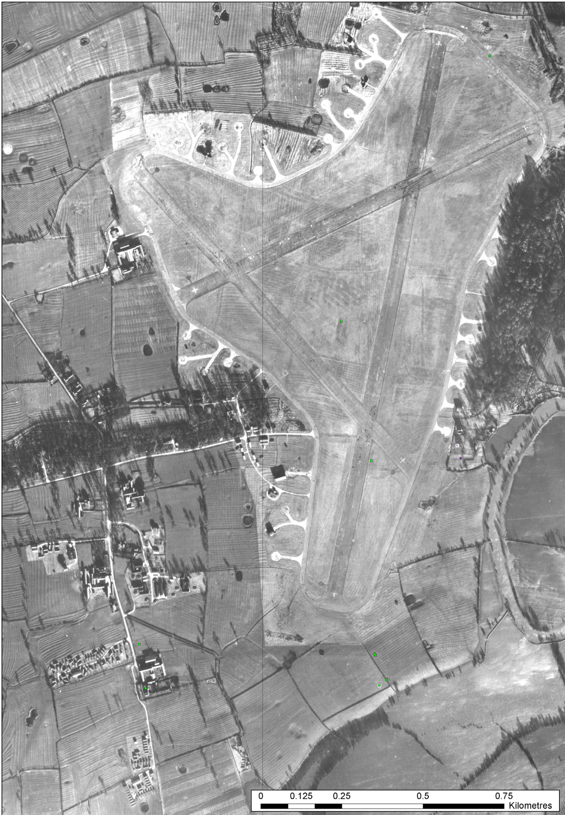
Fig 15: Vertical photograph of RAF Poulton. RAF 30287/ FFO-0077 04-FEB-1945 © Historic England Archive
