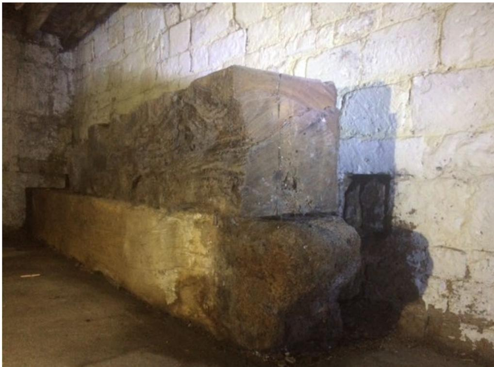
*Figure 3: Ex situ main beam thought to have come from the South Wing, photograph taken from the east (Photograph: Alison Arnold)*
